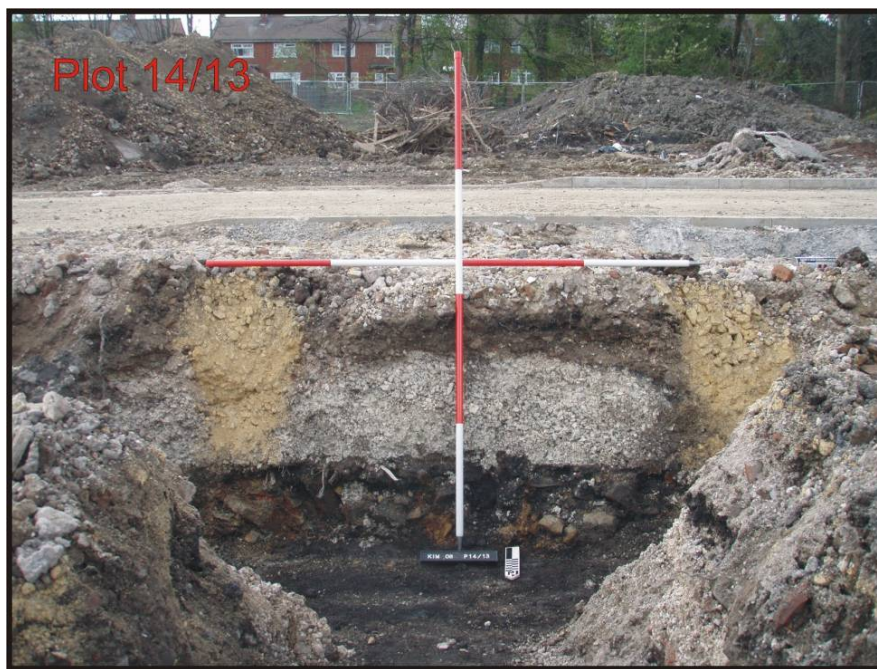
Fig. 10: North-facing section of the foundations. A demolition layer packed with building materials can be seen in the bottom of the section under a 0.40 m thick layer of aggregate.
