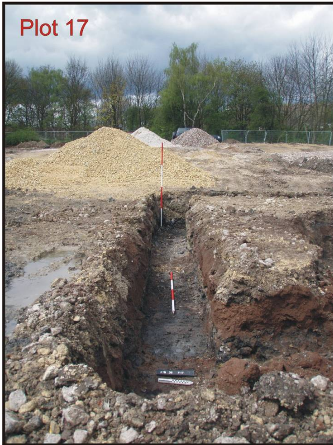
Fig. 18: Foundation for the southern wall of Plot 17.
