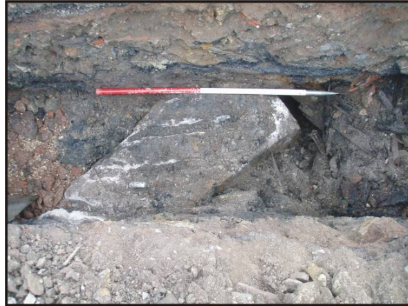
Fig. 20: Concrete block used as foundations.
