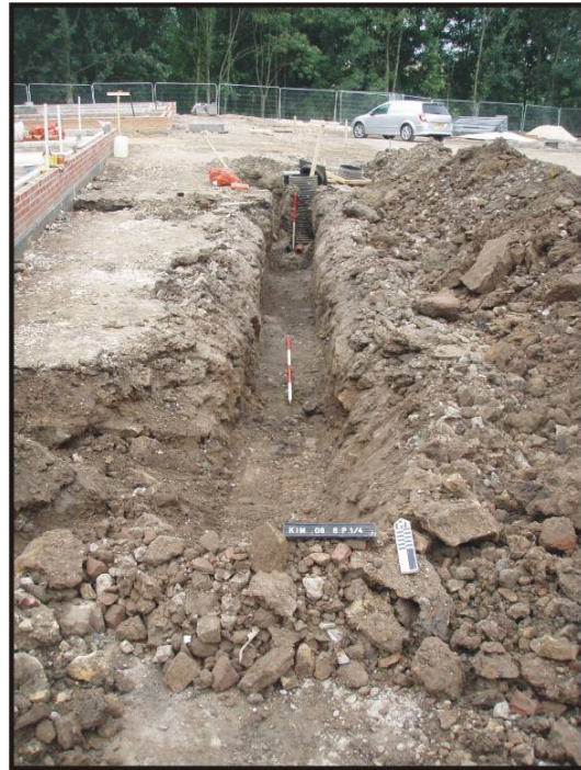
Fig. 22: Sewage trench running north-south on the eastern side of Plots 1-4.
