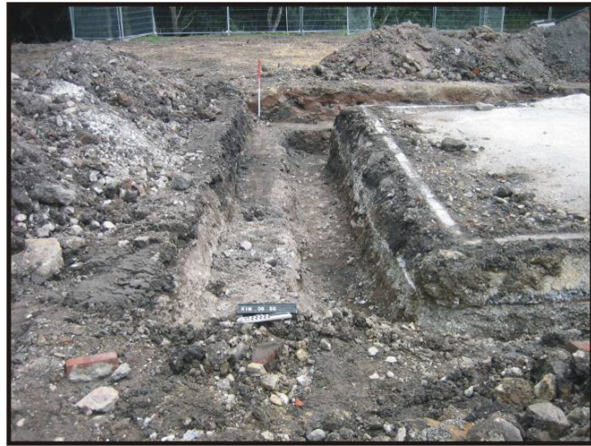
Fig. 25: General services trench, east side.
