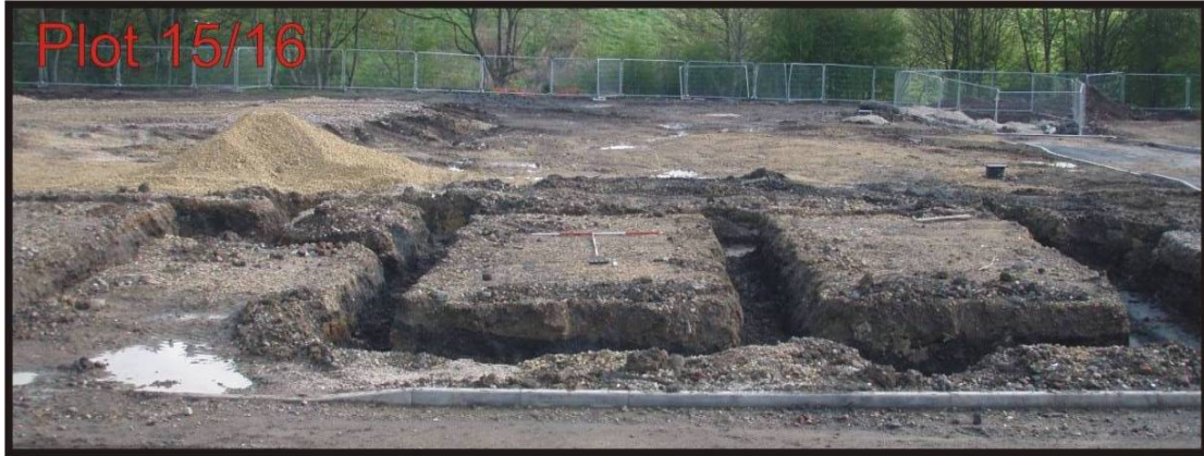
Fig. 15: General view of Plots 15-16 looking north.
