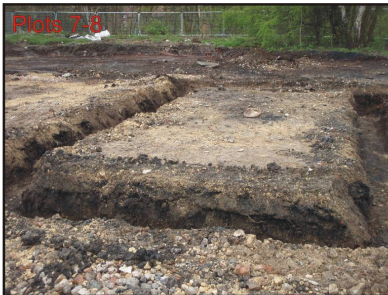
Fig. 7: General view of the foundations of Plot 7 (looking west).
