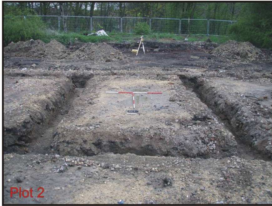
Fig. 5: General view of the foundations of plot 2.
