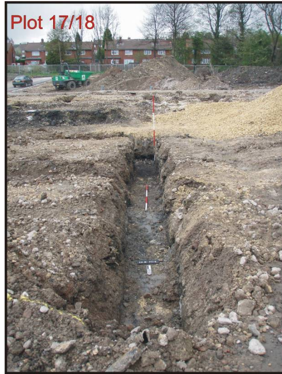
Fig. 16: Foundation trench for the west wall of Plots 17 and 18.
