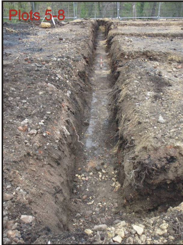
Fig. 8: General view of the foundations of the west wall (looking north).
