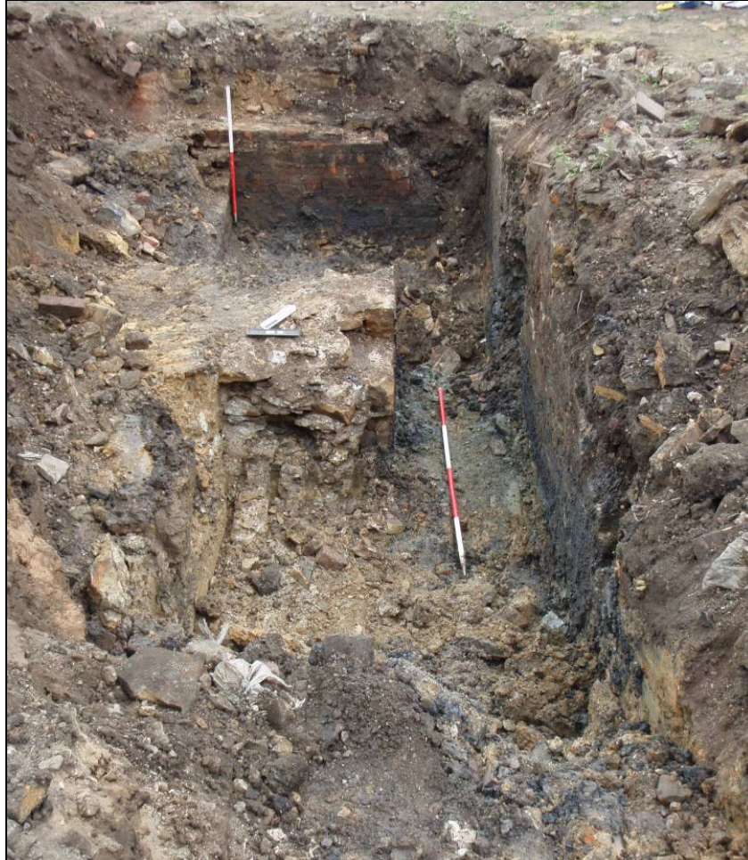
Fig. 4: Trench excavated to remove contamination. Facing west.
