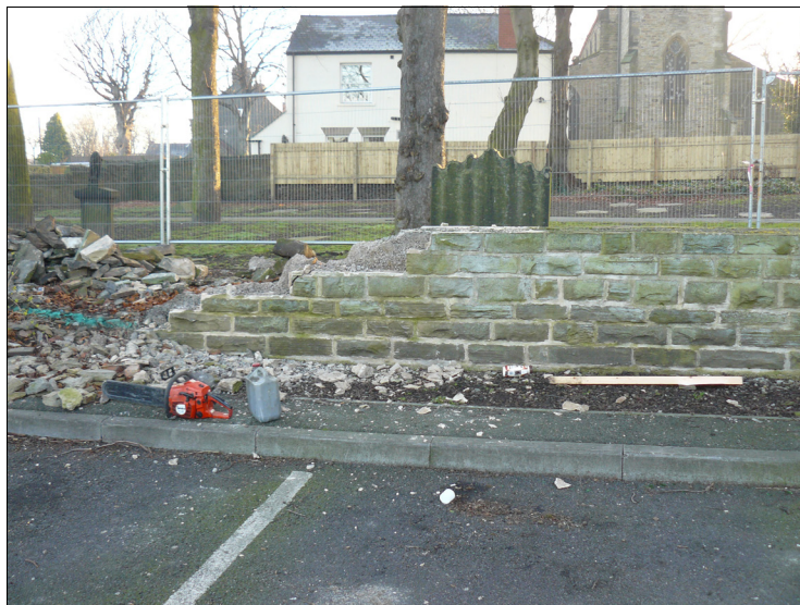
Fig 4: Tarmac pavement. Facing east.
