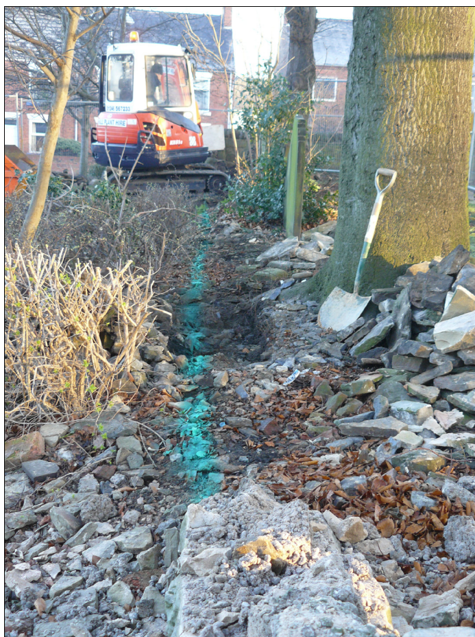
Fig 3: Trench line to be excavated. Facing north
