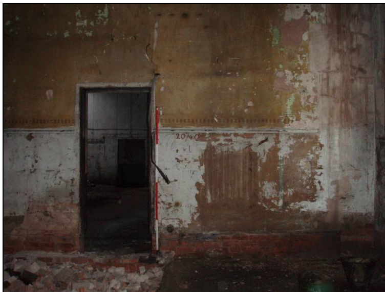
Fig. 13 Western doorway in the south wall giving access to the chapel from the school room. The brickwork at base of wall demotes height of original sloping floor level. (Scale: 2m)
