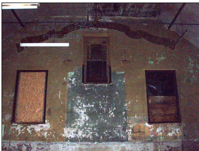
Fig. 10 East wall of the chapel showing the three boarded up windows.
