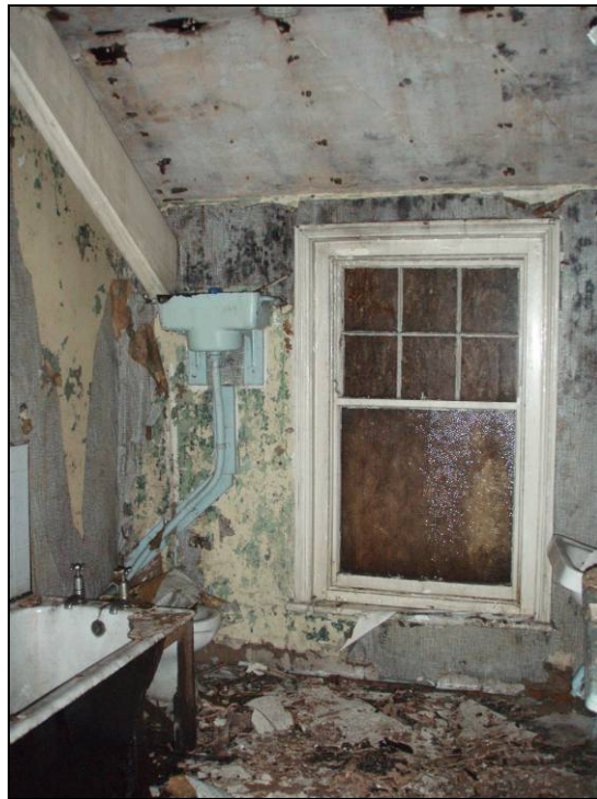
Fig. 48 The bathroom in the 1908 extension.
