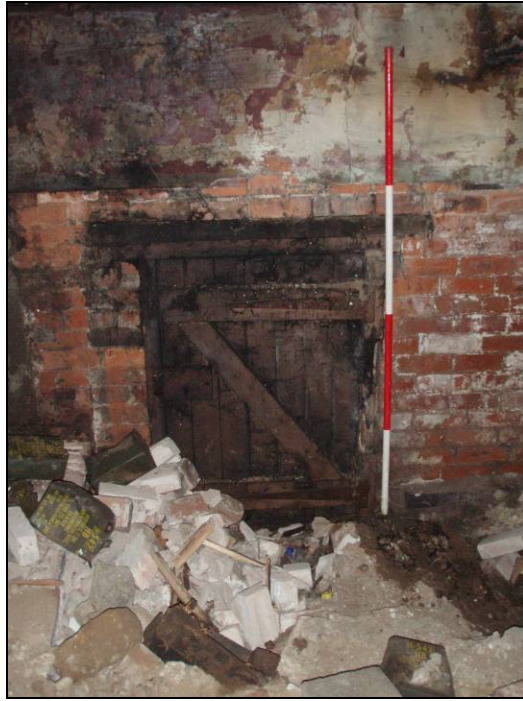
Fig. 18 Wooden doorway that gave access to the space below the altar platform. (Scale: 2m)
