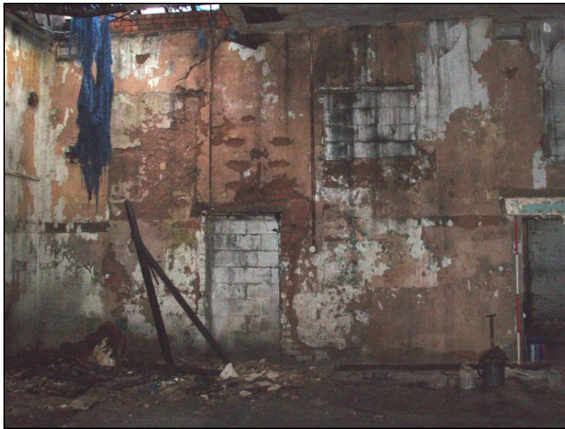
Fig. 20 The east wall of the schoolhouse showing the in-filled windows and doorway. (Scale: 2m)
