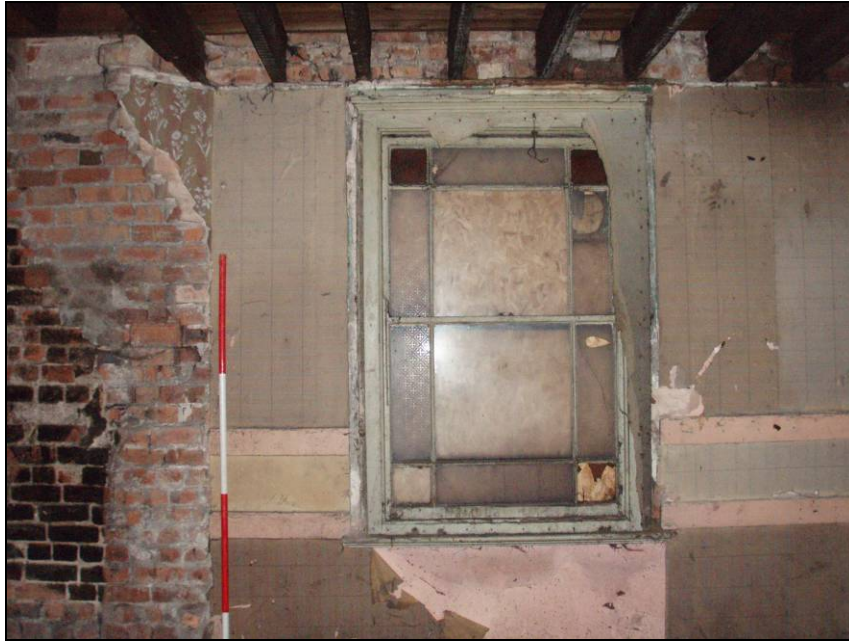
Fig. 29 One of the sash windows flanking the chimney breast on the east wall of the rectory. (Scale: 0.5m graduations)
