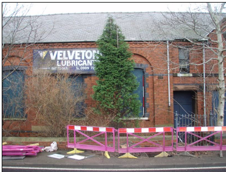
Fig. 60 West exterior elevation of schoolhouse, looking east. (Scale: 2m)
