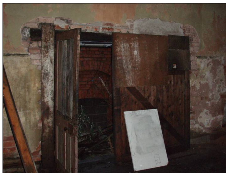
Fig. 35 Doorway in west wall of the upper storey of the rectory.
