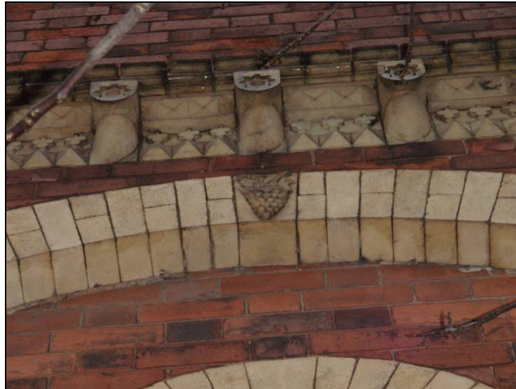
Fig. 52 Detail of the window frame showing the carved grapes detail.
