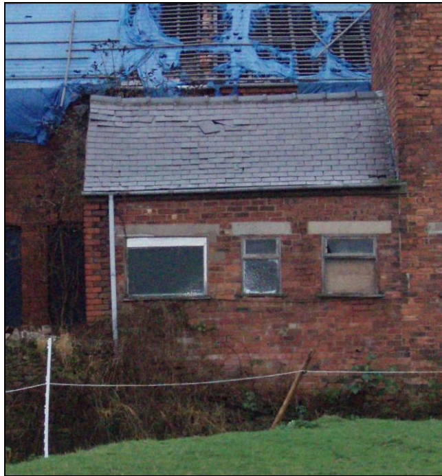
Fig. 65 East elevation of the office and toilet block showing where the wall abuts the rectory wall.
