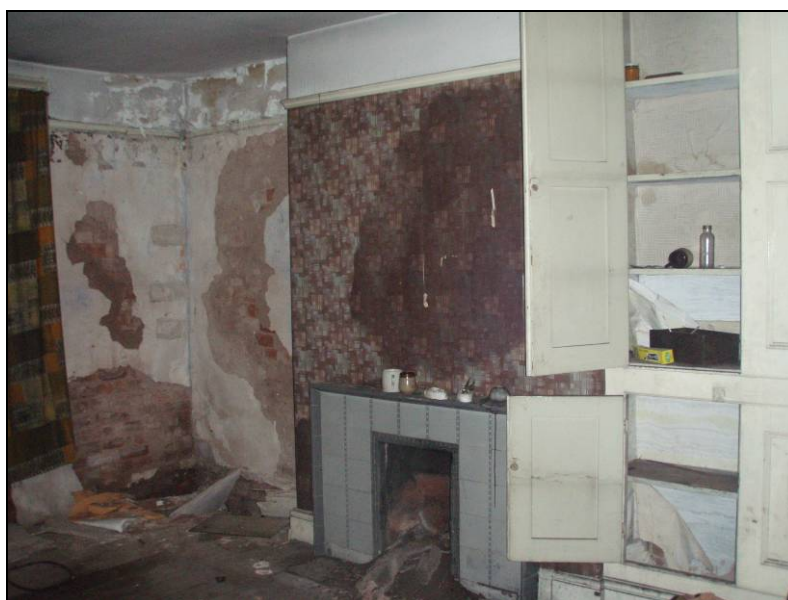
Fig. 45 Room Two of the 1908 extension, looking north-west.
