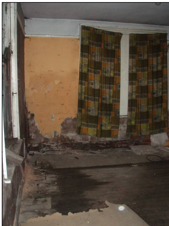
Fig. 44 Room Two of the 1908 extension looking west.
