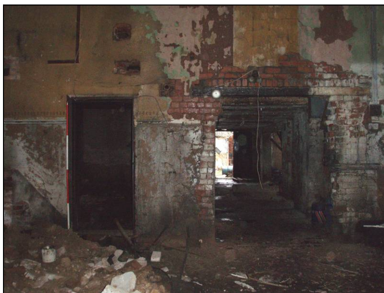
Fig. 14 The second smaller doorway in the south wall adjacent to the modern entrance to the passage. (Scale: 2m)
