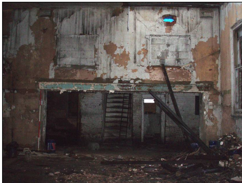
Fig. 21 The east wall of the schoolhouse showing the in-filled windows and the new entrance. (Scale: 2m)
