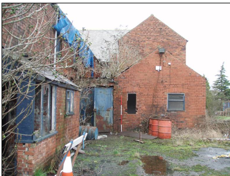
Fig. 64 South elevation of the toilet block, looking north.
