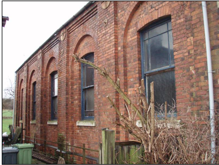
Fig. 57 North exterior elevation of the chapel.
