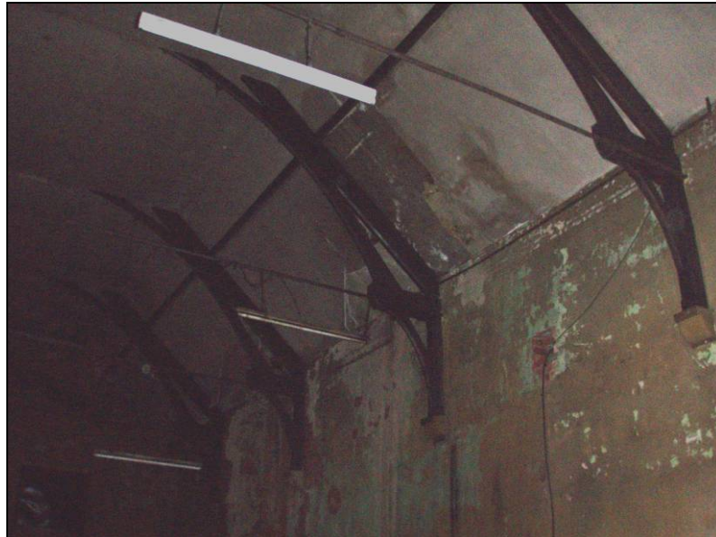
Fig. 7 Interior of Chapel showing the wooden ceiling beams on the south side.
