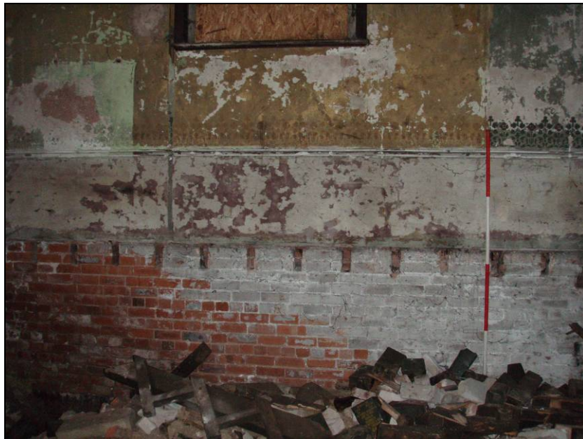
Fig. 17 East wall of the chapel showing the height of the altar and the position of the supporting struts. (Scale: 2m)
