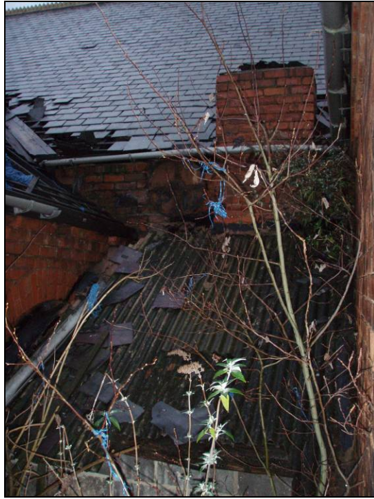
Fig. 36 View from the doorway overlooking the boiler room (note chimney).
