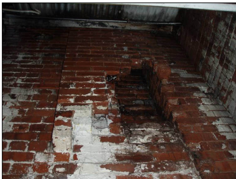
Fig. 25 Chimney breast located on the other side of the south wall of the chapel above the large entrance.
