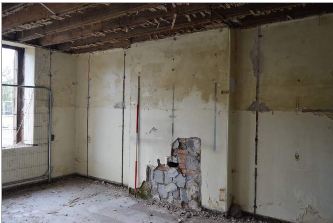
Plate 32: South room with blocked hearth (facing south east). Scale 2m.
