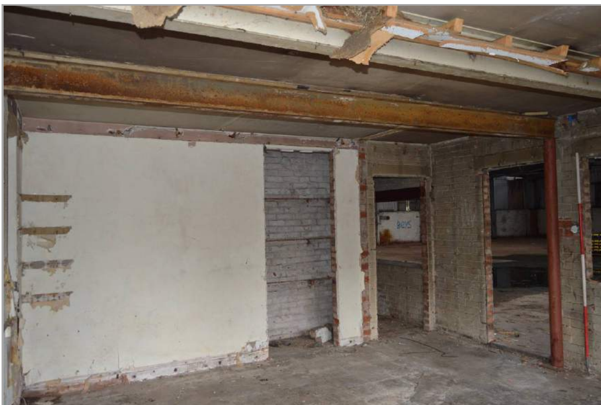
Plate 92: Interior of Building 4 (facing south east).
