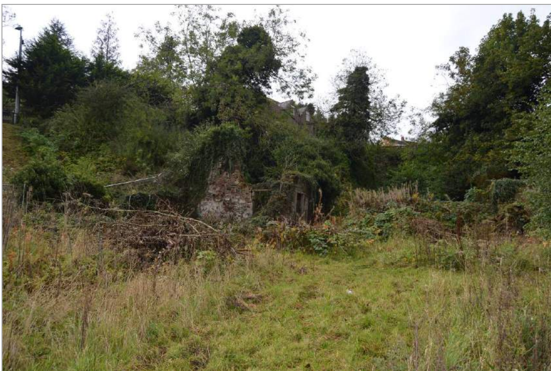
Plate 4: Former mill buildings located to the south western extents of the haulage site (facing south west).
