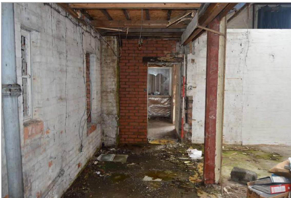
Plate 75: Interior space of linking structure, Building 3 (facing east). Scale 2m.
