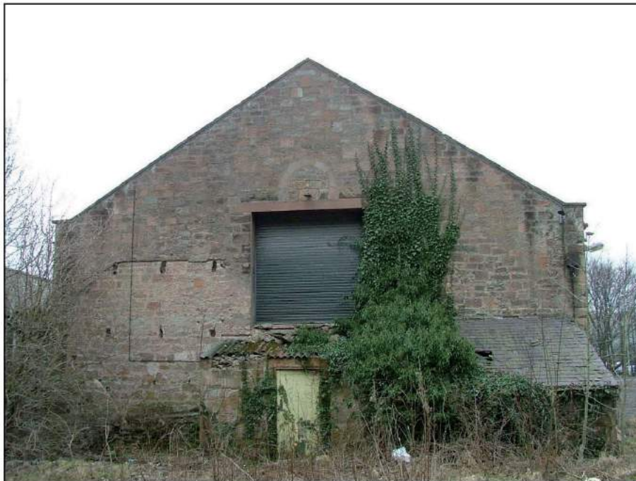
Plate 27: West elevation of Building C
