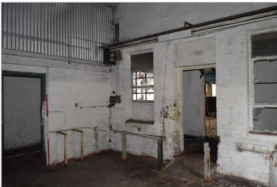
Plate 97: Interior of Building 4 (facing south east). Scale 2m.
