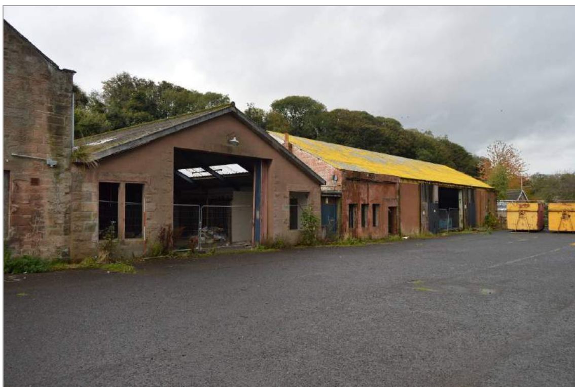
Plate 3: Buildings to the north on the former haulage depot facing north west. Scale 2m.
