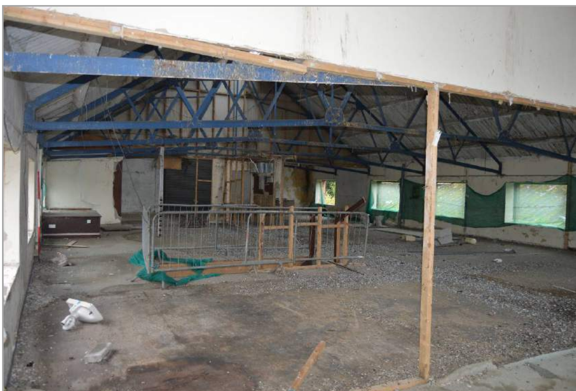
Plate 54: View of Building 1, first floor (facing north west). Scale 2m.
