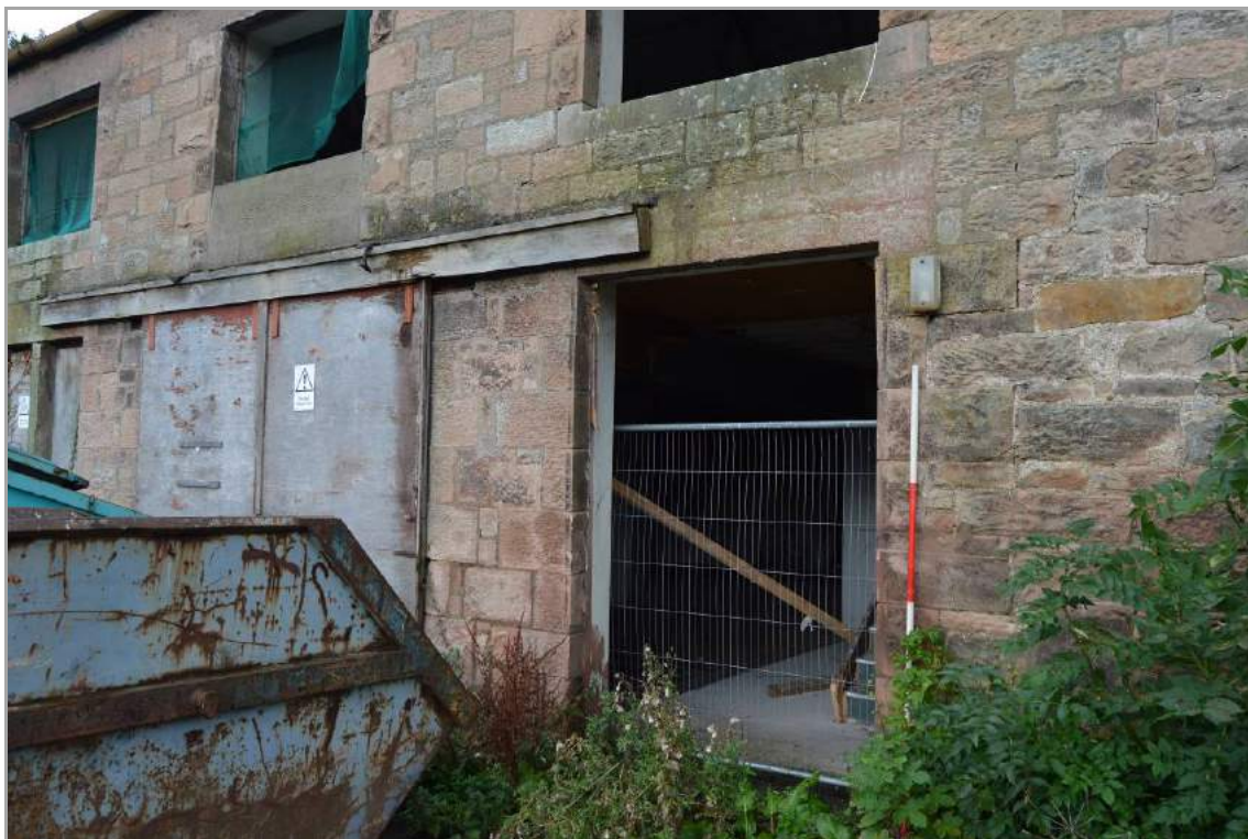
Plate 17: View of doorways in south elevation (facing north west). Scale 2m.
