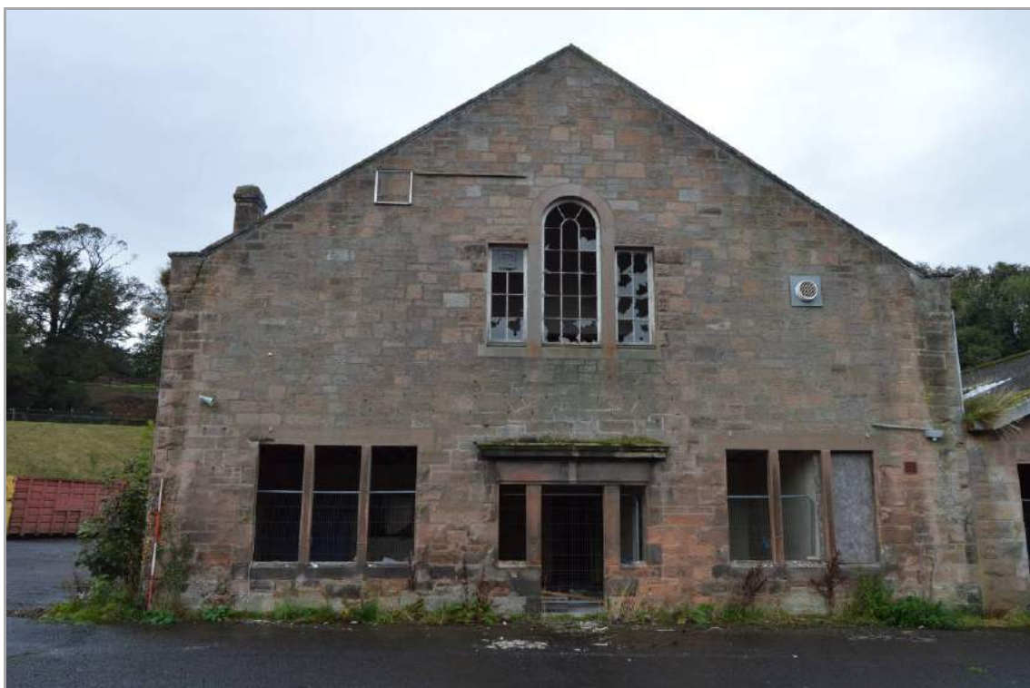
Plate 7: East elevation (facing west). Scale 2m.
