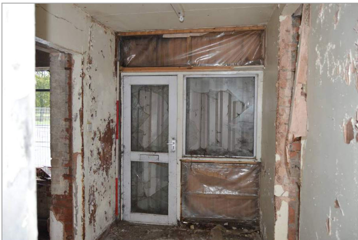
Plate 74: Interior of east elevation of linking structure, Building 3 (facing west). Scale 2m.
