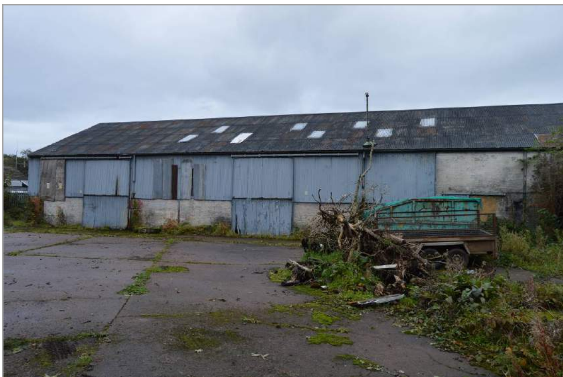
Plate 83: West elevation of Building 4 (facing north east). Scale 2m.
