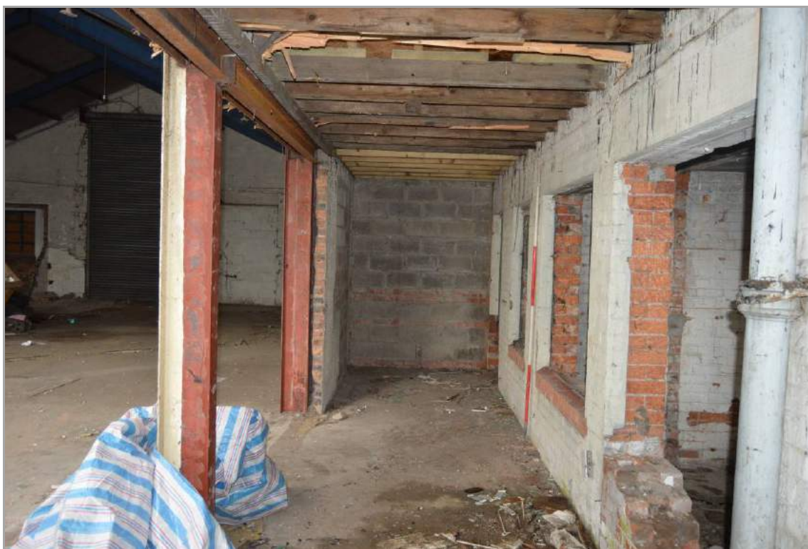
Plate 76: Interior of linking structure, Building 3 (facing west). Scale 2m.
