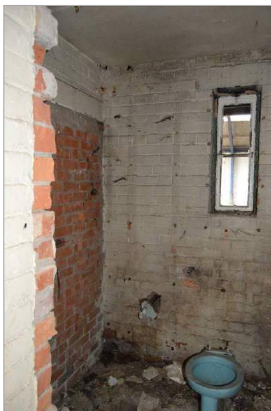
Plate 93: Interior of Building 4 (facing south east).
