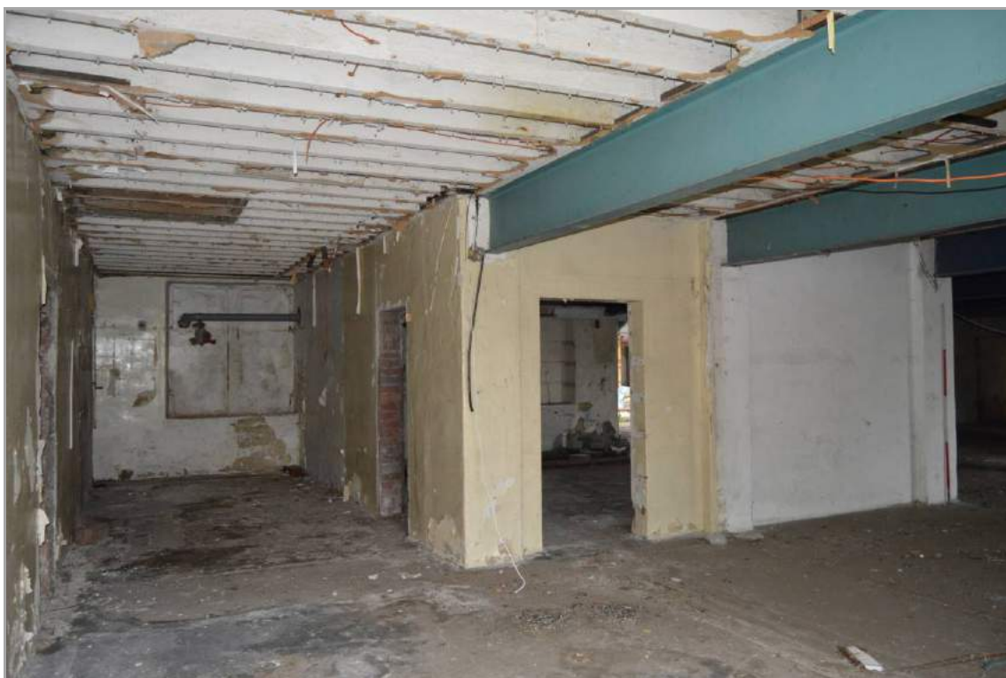
Plate 46: Interior dividing walls (facing north east). Note the blocked window marking the original exterior wall of Building 1. Scale 2m.
