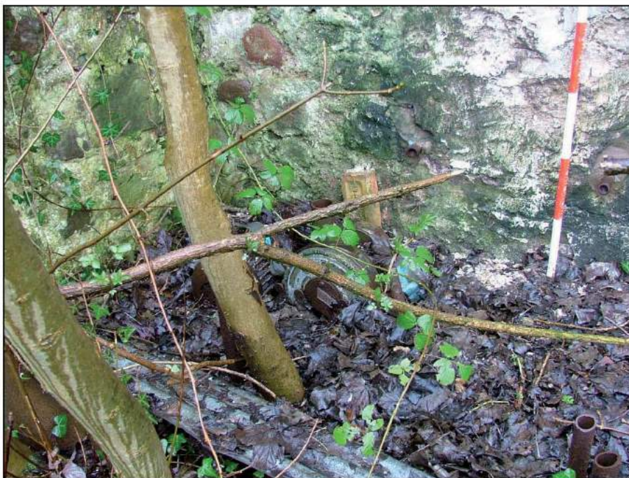
Plate 17: Former motor located within the east room of Building B
