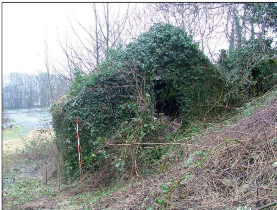
Plate 14: West elevation of Building B (Scale = 2m)
