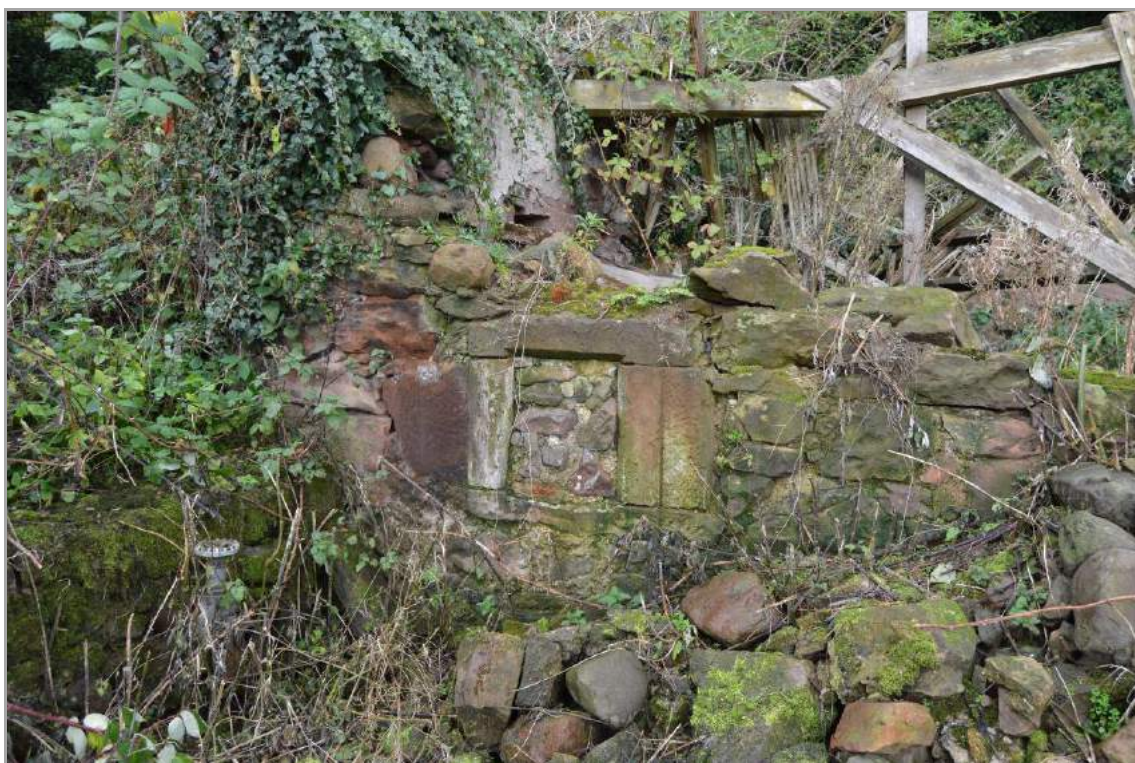
Plate 104: Former Mill Building A, detail of blocked window to remaining south elevation.
