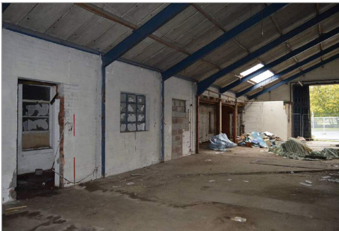
Plate 69: Interior of north elevation to Building 2 (facing north east). Note the knocked through section, a former internal room. Scale 2m.
