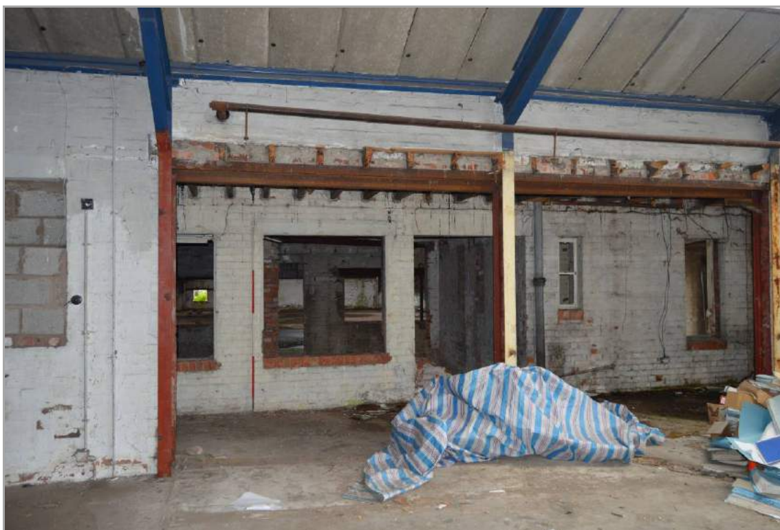
Plate 70: Interior of Building 2, knocked through into Building 3 (facing north). Scale 2m.
