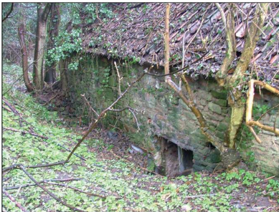
Plate 8: West elevation of Building A
