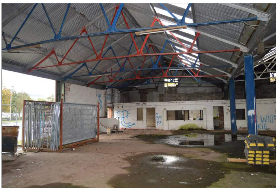
Plate 89: Interior of Building 4 (facing south east).
