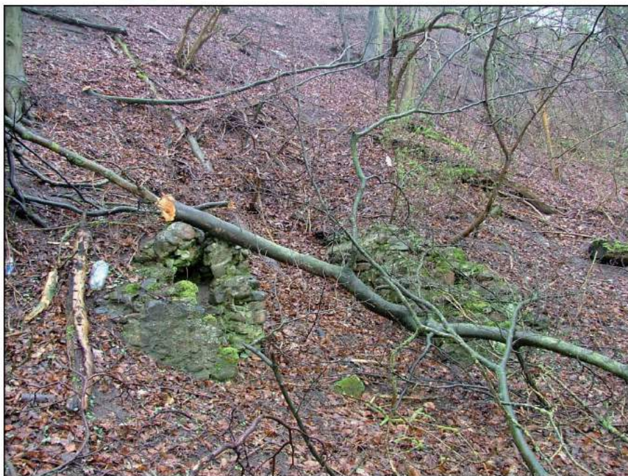
Plate 36: Remains of a building located on the slope of Cardingmill Plantation
