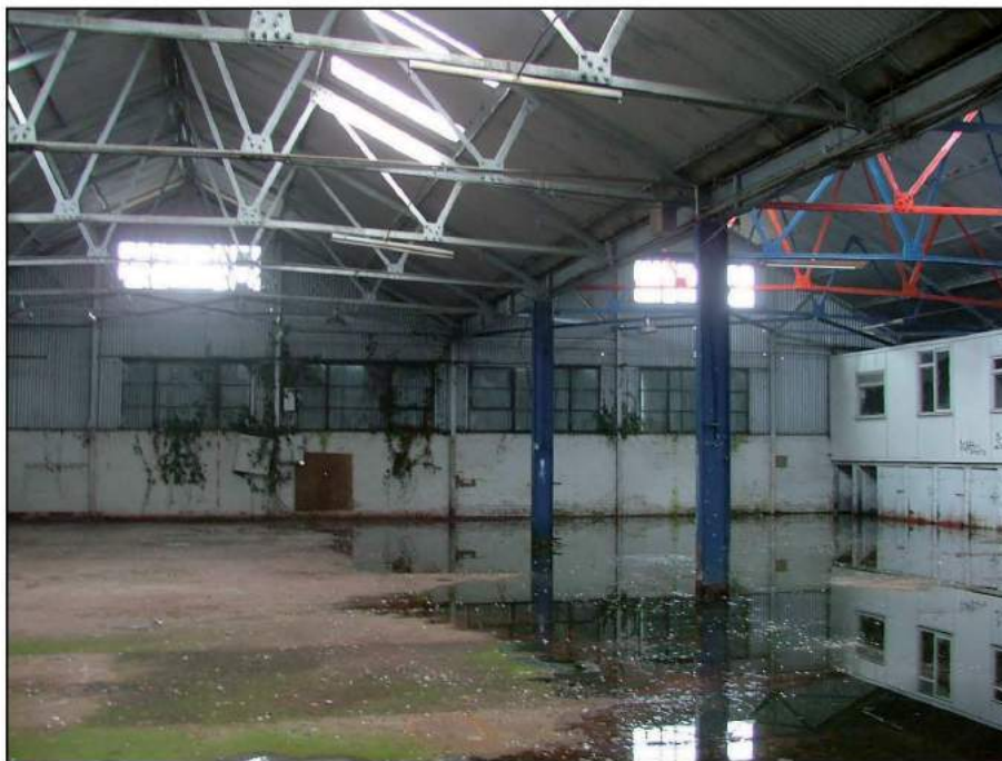
Plate 33: View looking north of the interior of Building E
