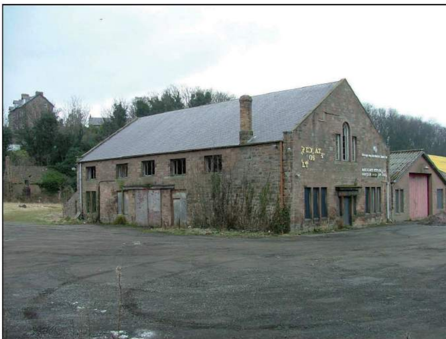
Plate 20: View looking north-west showing Building C
