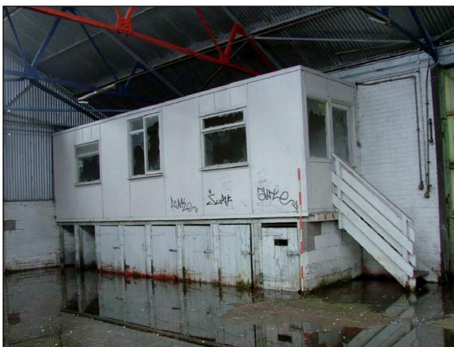
Plate 34: The north-east corner of the interior of Building E (Scale = 2m)
