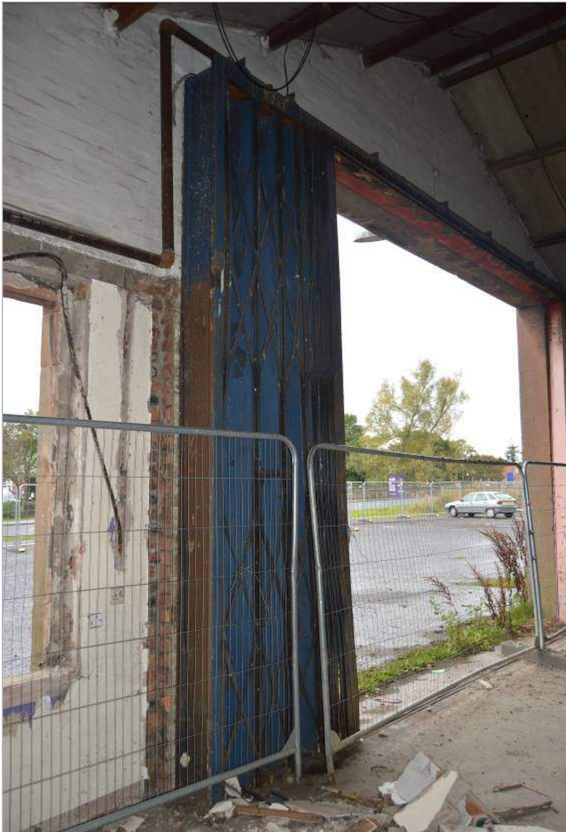
Plate 72: Detail of concertina door from interior of Building 2 (facing east).
