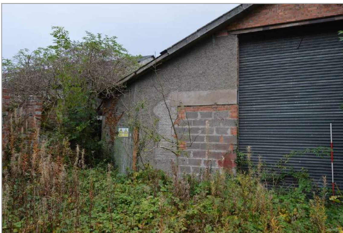
Plate 61: Rear, west elevation of Building 2 showing blocked former entrance (facing north east). Scale 2m.
