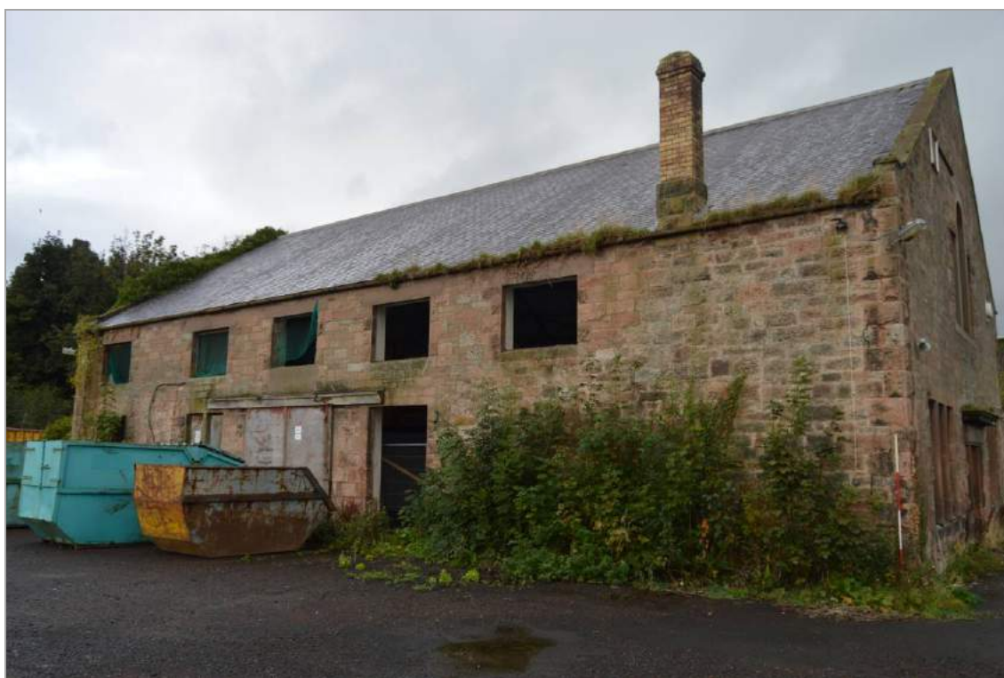
Plate 15: Oblique view of south elevation Building 1(facing south west). Scale 2m.
