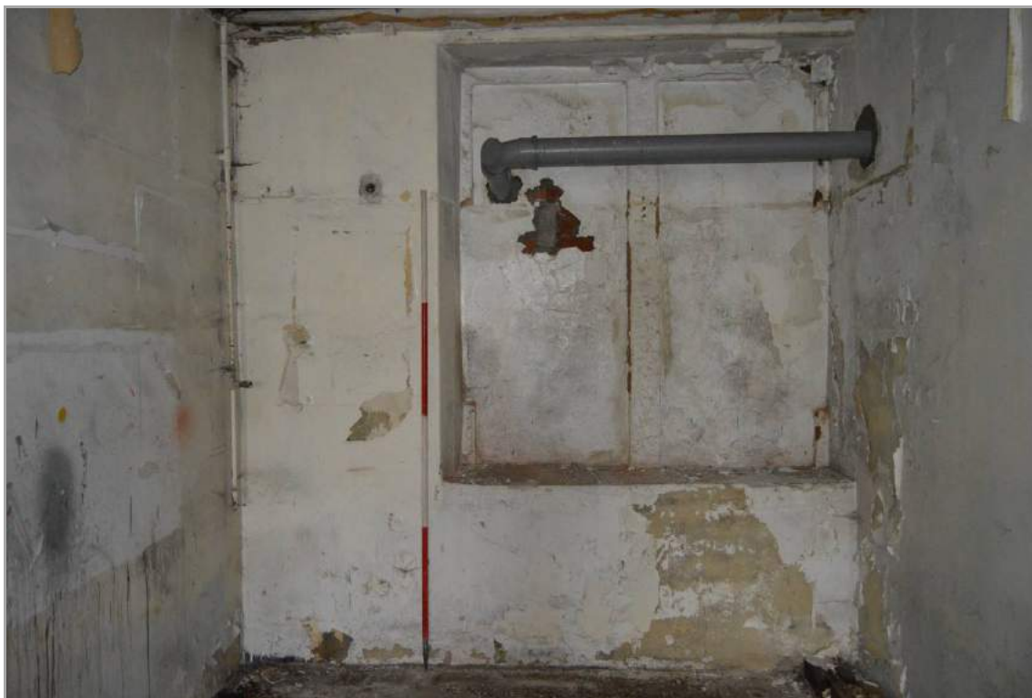
Plate 47: Detail of brick blocked stone mullioned window (facing north). Scale 2m.
