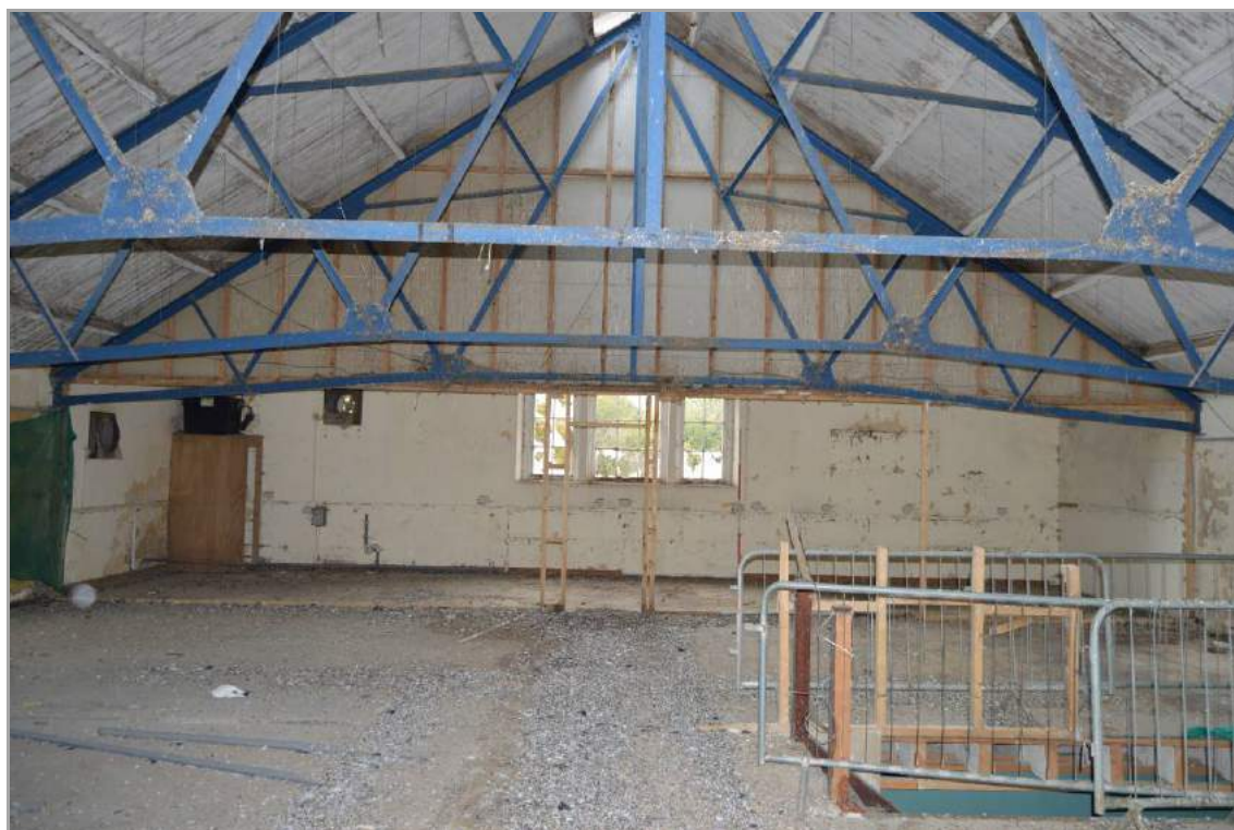
Plate 50: General view of first floor of Building 1 (facing east). Scale 2m.
