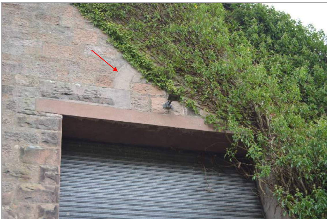
Plate 25: Blocked arched window above first floor good entrance (facing north east).
