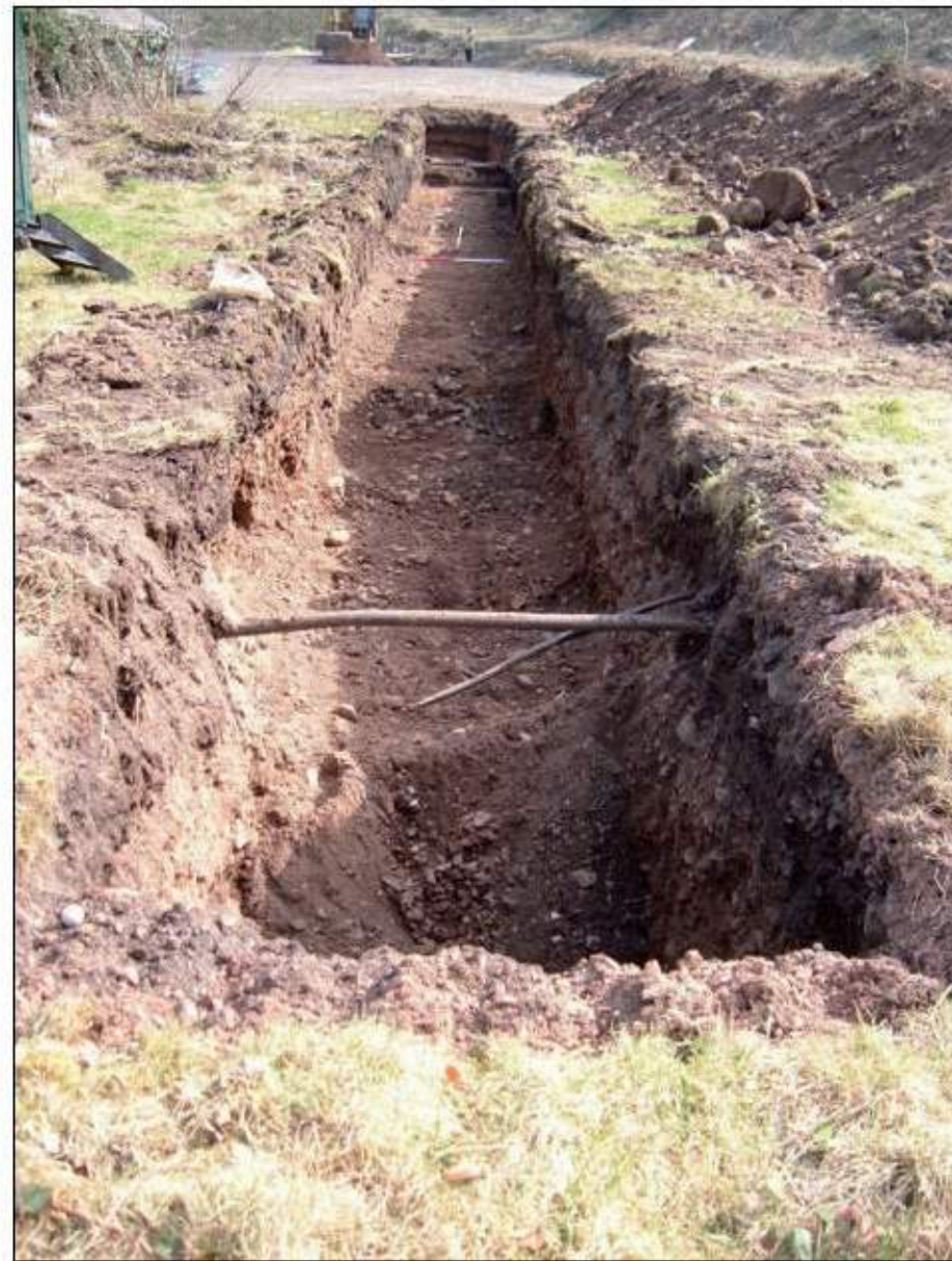
Plate 1: View southeast of Trench 1
