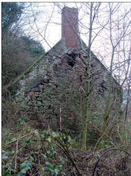
Plate 6: South elevation of Building A (Scale = 2m)
