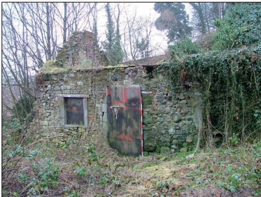
Plate 12: North elevation of Building B (Scale = 2m)
