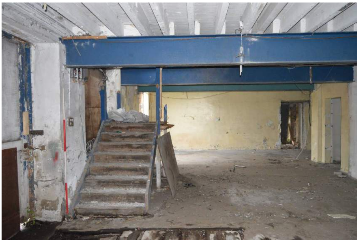
Plate 44: Dog-leg staircase to first floor of Building 1 (facing west). Scale 2m.
