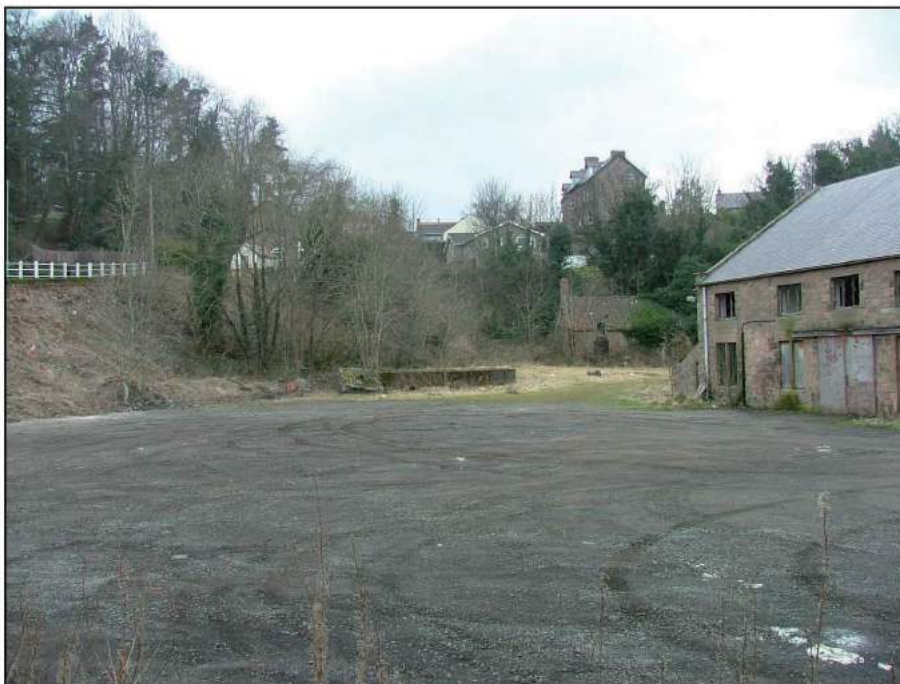
Plate 19: View looking west showing Building A (the cottage) in the background, with part of the south elevation of Building C to the right of photograph
