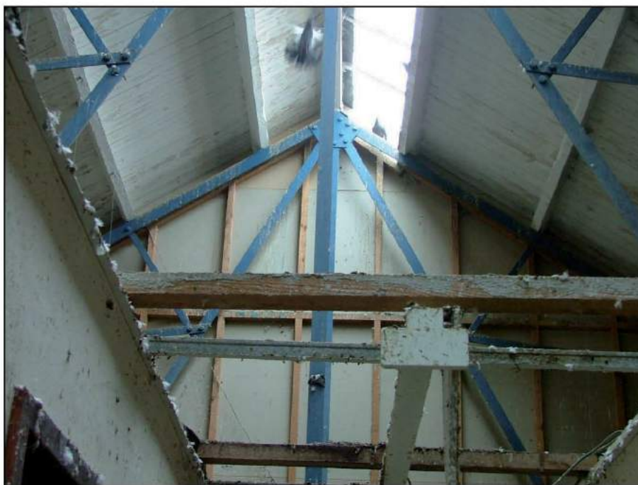
Plate 28: Detail of the internal roof structure of Building C
