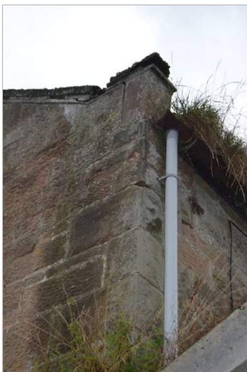
Plate 14: Kneeler detail to north east corner of Building 1 (facing north west).
