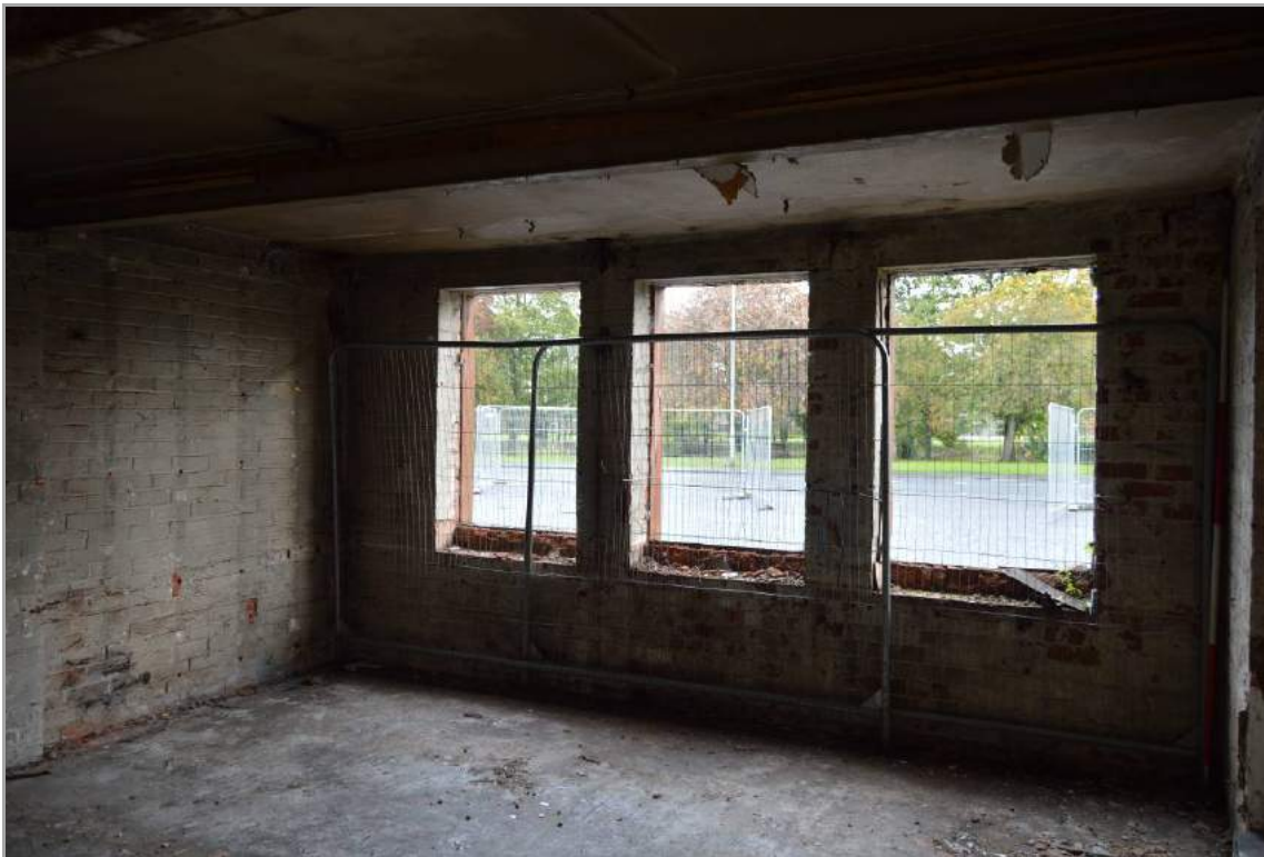
Plate 90: Interior of Building 4 (facing south east).
