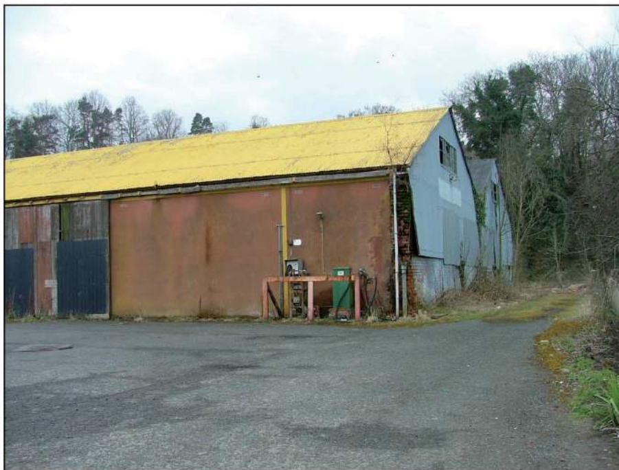
Plate 31: View looking west showing the two gables of Building E
