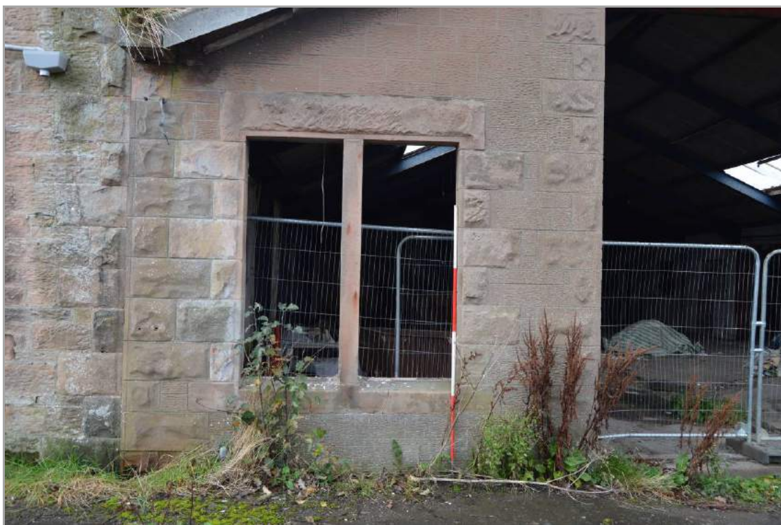
Plate 58: South window to east elevation of Building 2 (facing west). Scale 2m.
