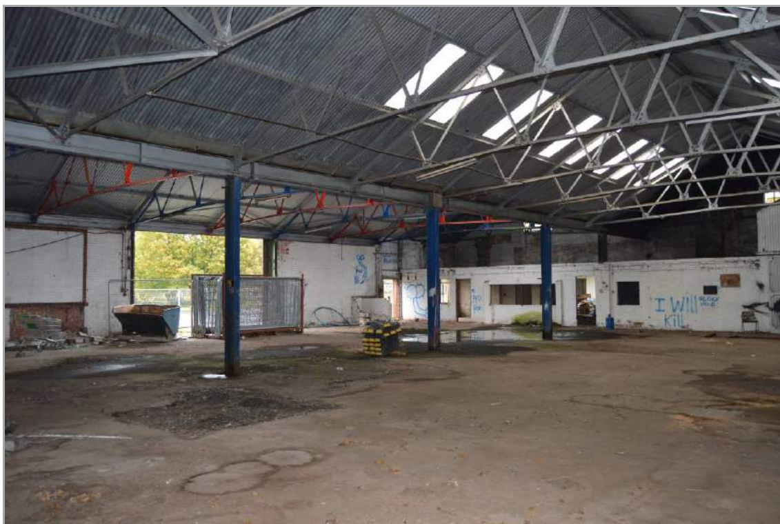
Plate 85: Interior of Building 4 (facing south east).
