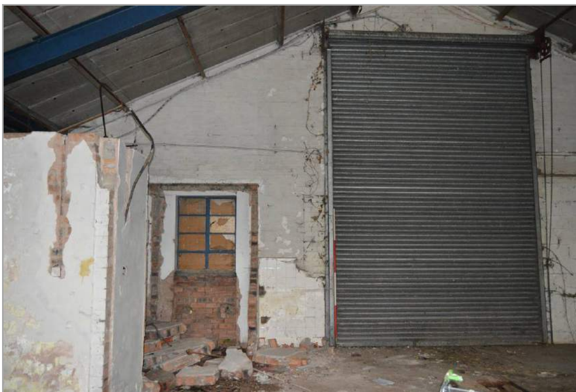
Plate 66: Interior of Building 2 (facing west). Scale 2m.
