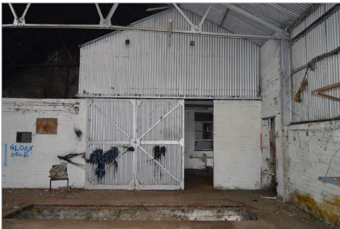
Plate 96: Interior of Building 4 (facing south east). Note the vehicle inspection pit. (Scale 2m)
