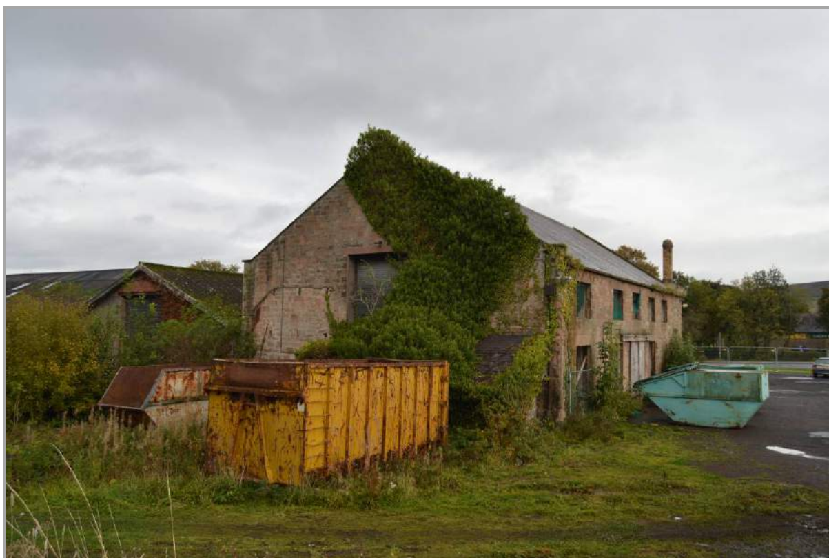
Plate 22: View of west elevation of Building 1 (facing east).
