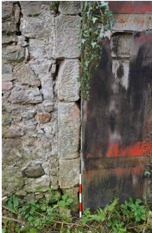
Plate 110: Dressed quoin stone door jamb (facing south). Scale 2m.
