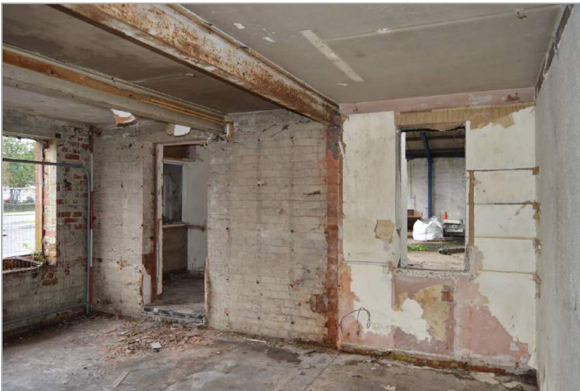
Plate 91: Interior of Building 4 (facing south east).
