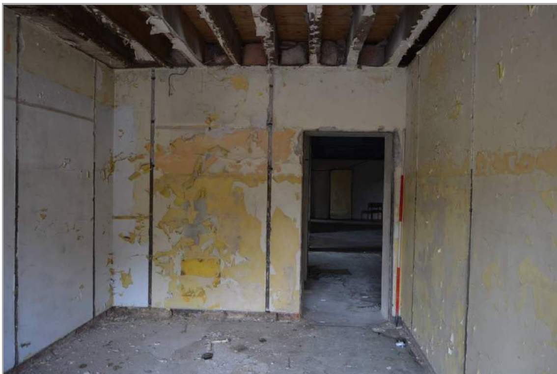
Plate 35: Hallway (facing west). Scale 2m.
