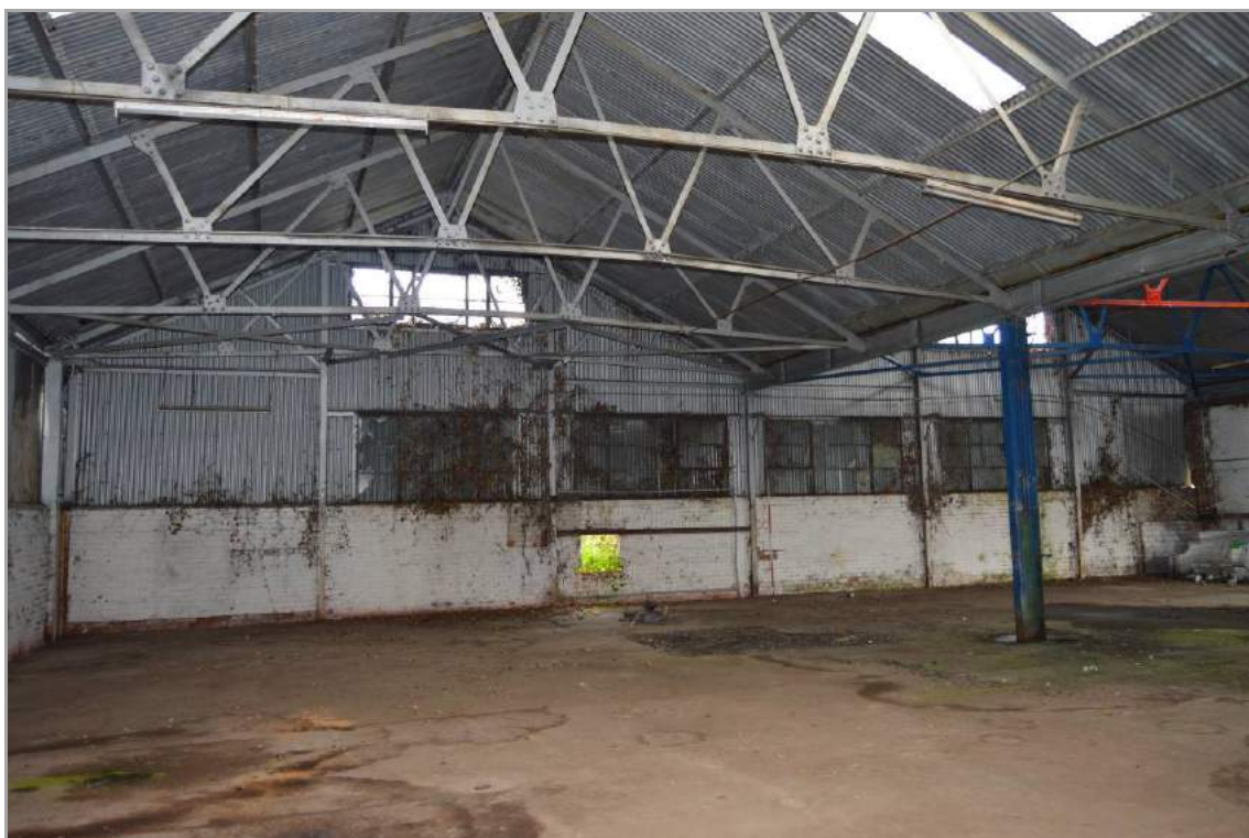
Plate 86: Interior of Building 4 (facing north). Scale 2m.
