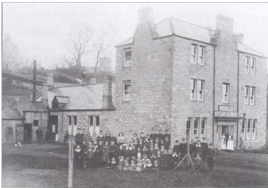
Figure 2: Photograph of the steam laundry building.
