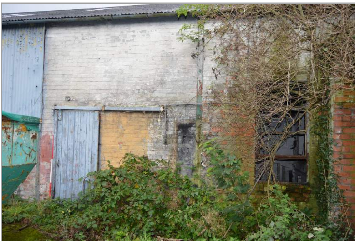
Plate 84: West elevation of Building 4 (facing north east). Scale 2m.
