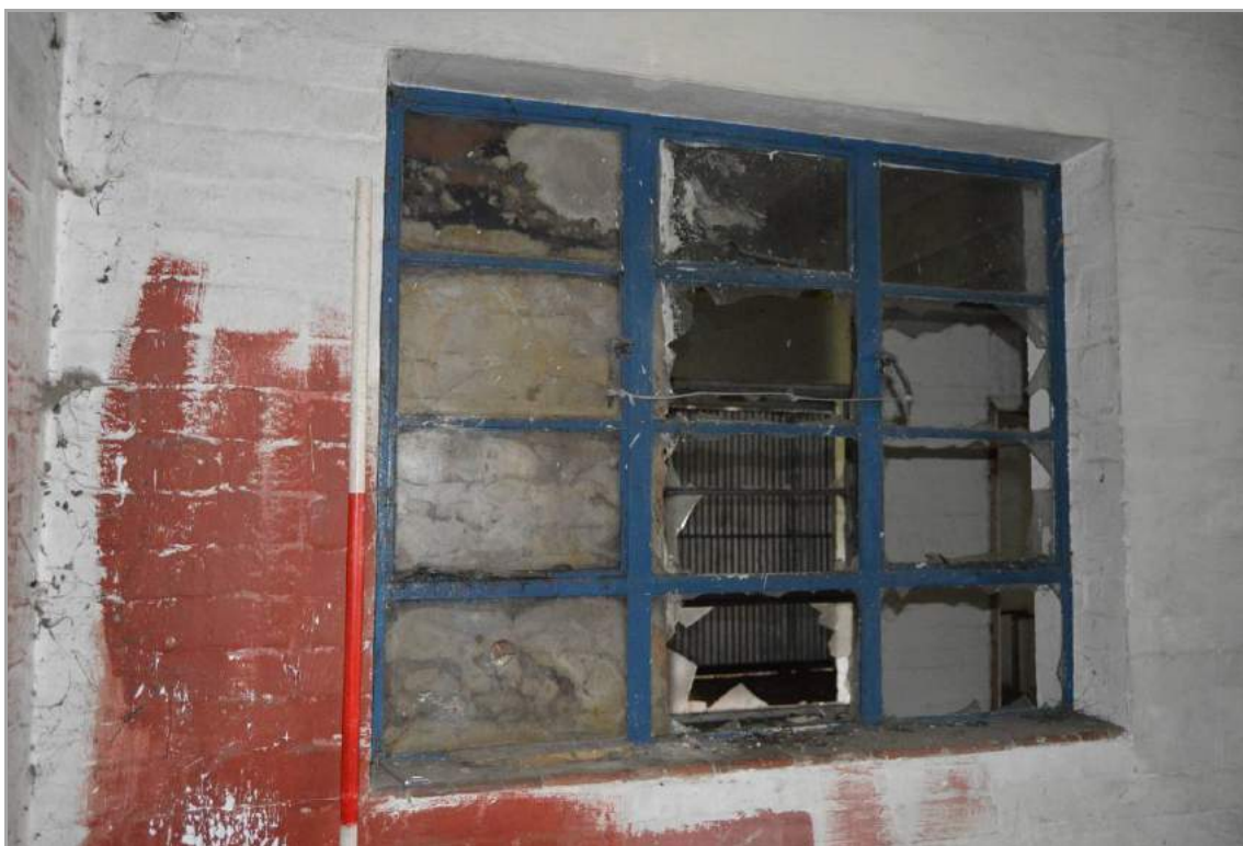
Plate 68: Crittal window to Building 2 (facing north). Scale 2m.
