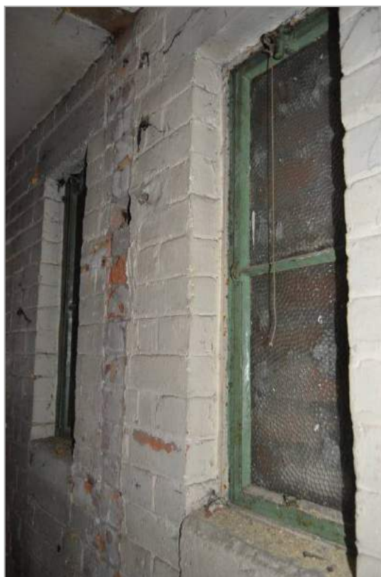
Plate 94: Interior of Building 4 (facing south east).
