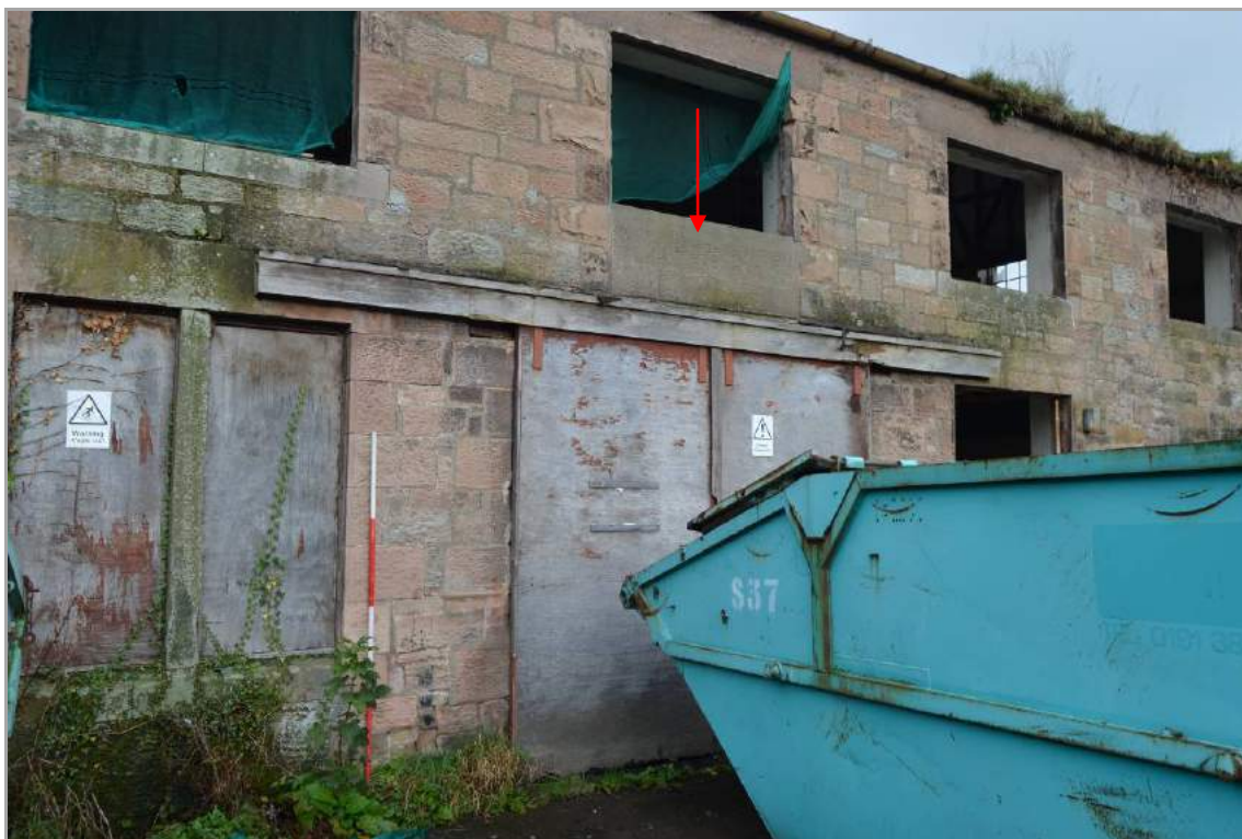
Plate 19: View of doorways in south elevation (facing north west). Scale 2m.
