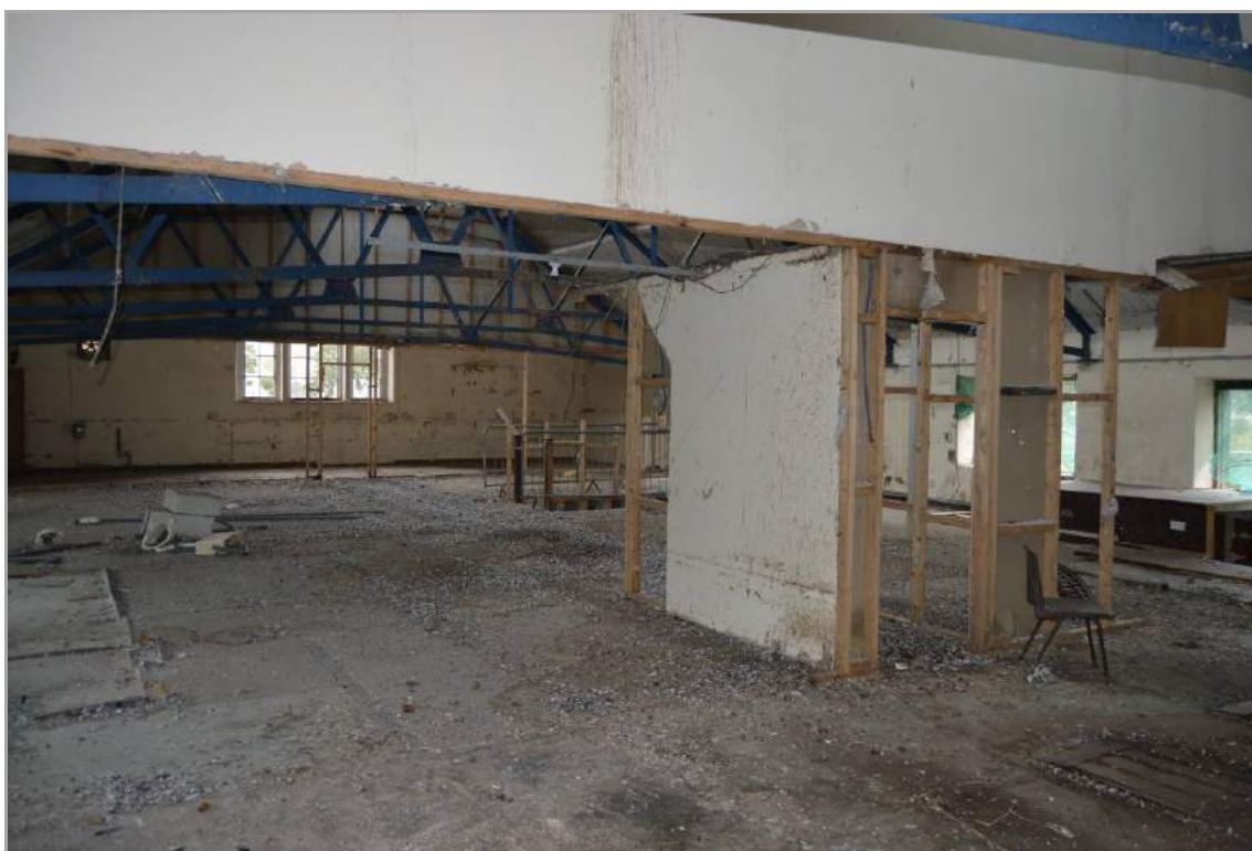
Plate 56: Building 1 first floor (facing south west). Scale 2m.
