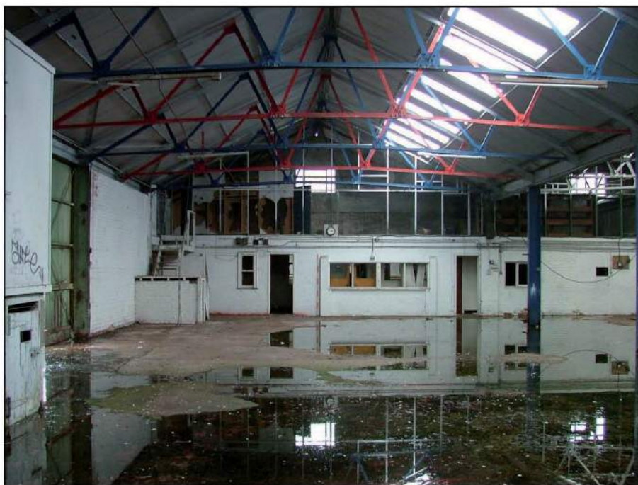
Plate 32: View looking south showing the range offices within Building E
