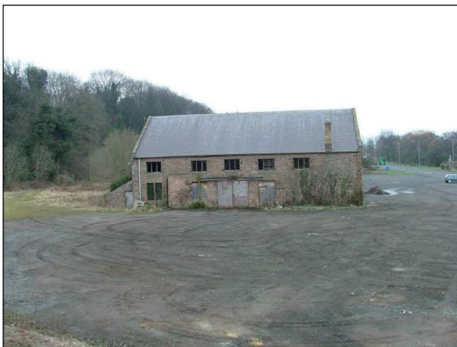
Plate 26: South elevation of Building C
