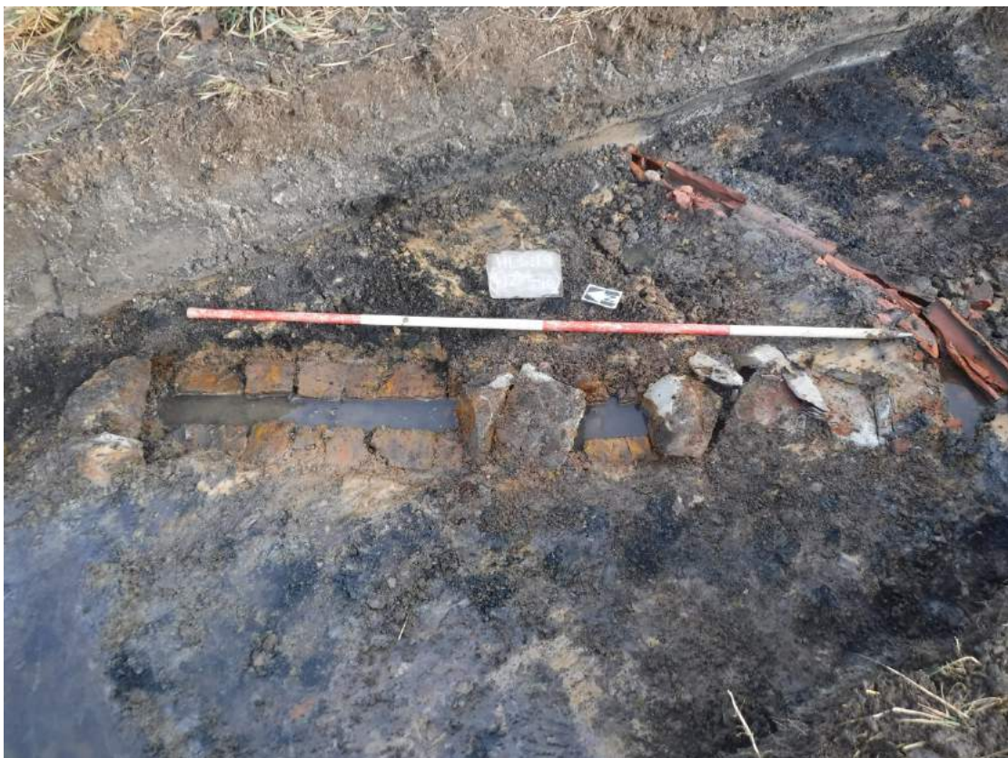
Figure 17. 19 th century brick-constructed culvert with sandstone capping, laid within construction cut [412], truncated by ceramic land drain (411). Scale: 2m.
