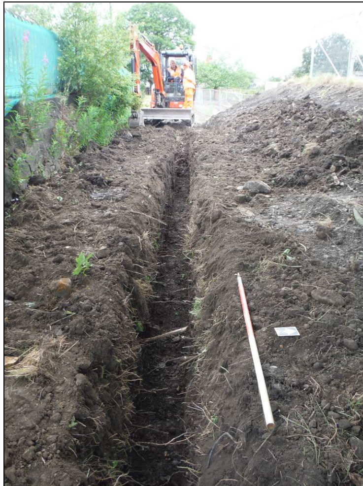
Figure 20. View looking west across Trench 1 (Scale = 1 x 1m in 0.5m graduations).
