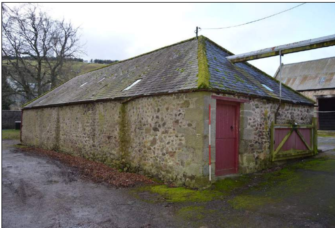
Plate 80: North east aspect of the east farm range. Scale 2m.
