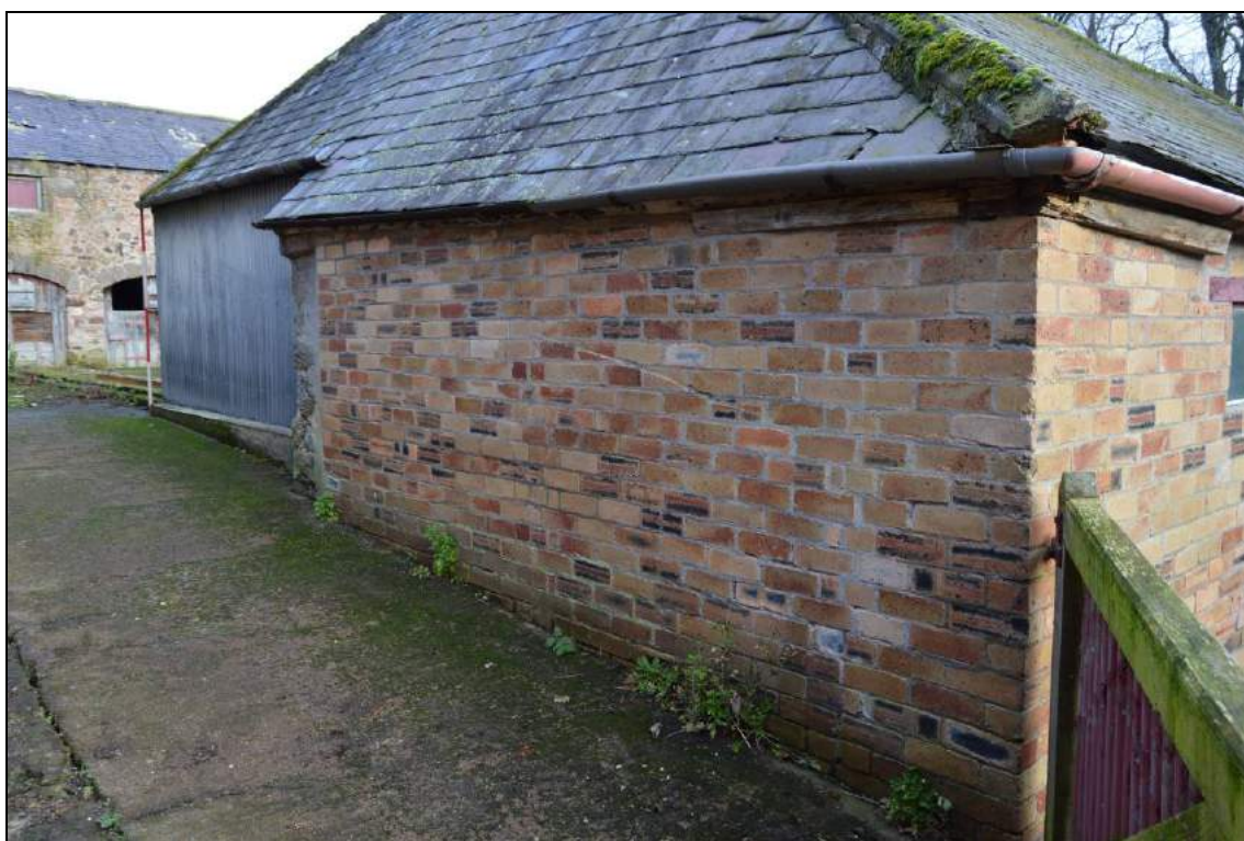
Plate 96: South shelter shed. Scale 2m.
