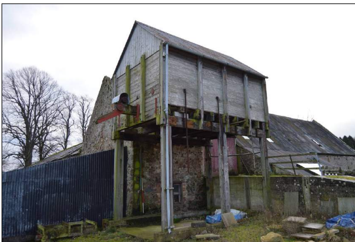
Plate 97: Grain tower (facing south east). Scale 2m.
