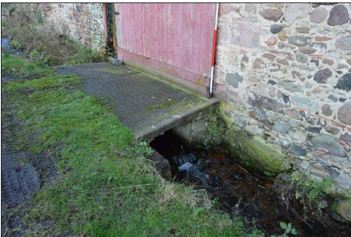
Plate 72: Concrete bridge (over former mill race) south elevation of south animal shed showing (facing north west). Scale 2m.
