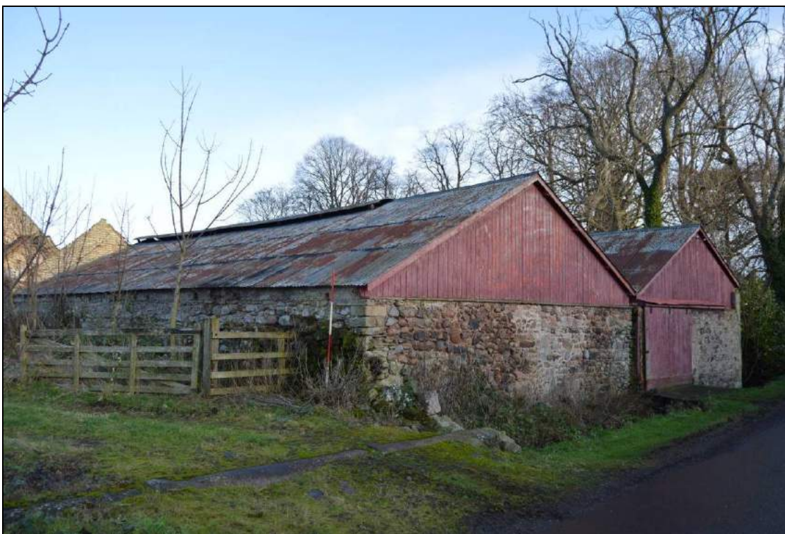
Plate 73: South elevation (facing north east). Scale 2m.
