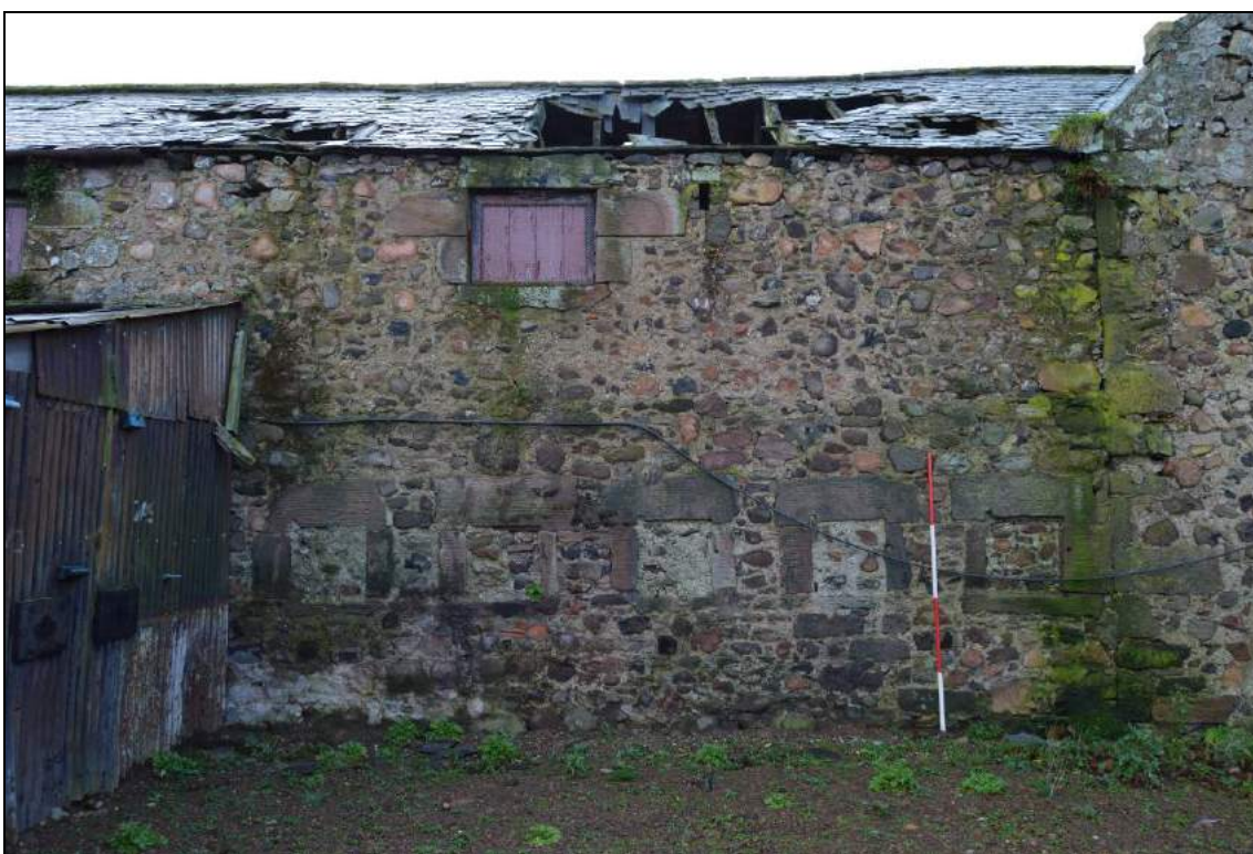
Plate 17: Five of the cow-house apertures to the north elevation of the granary range (facing north west). Scale 2m.
