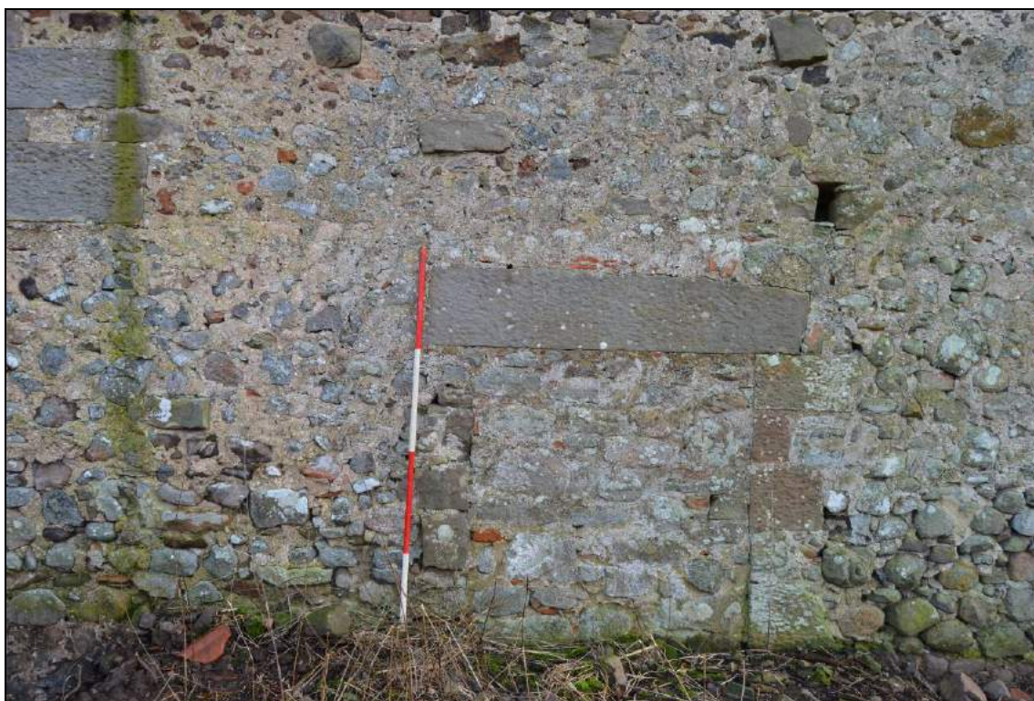
Plate 36: Blocked apertures in west elevation. Scale 2m.
