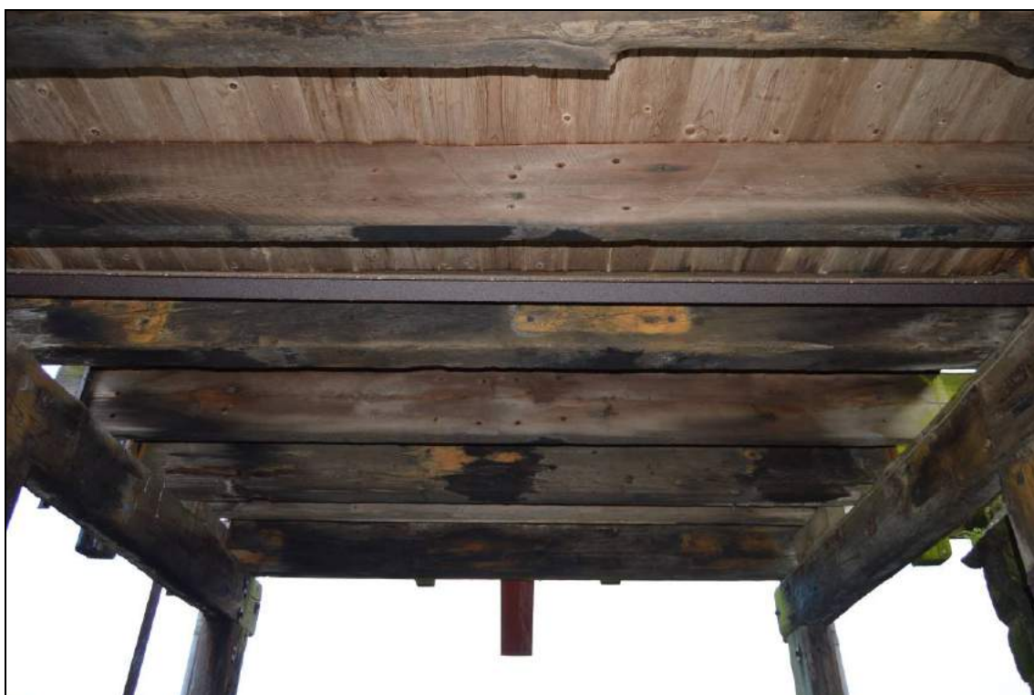
Plate 99: Underside of grain tower floor (facing north).
