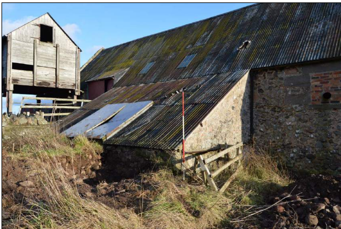
Plate 37: West elevation of barn (facing north east) with a grain silo extension to foreground. Scale 2m.
