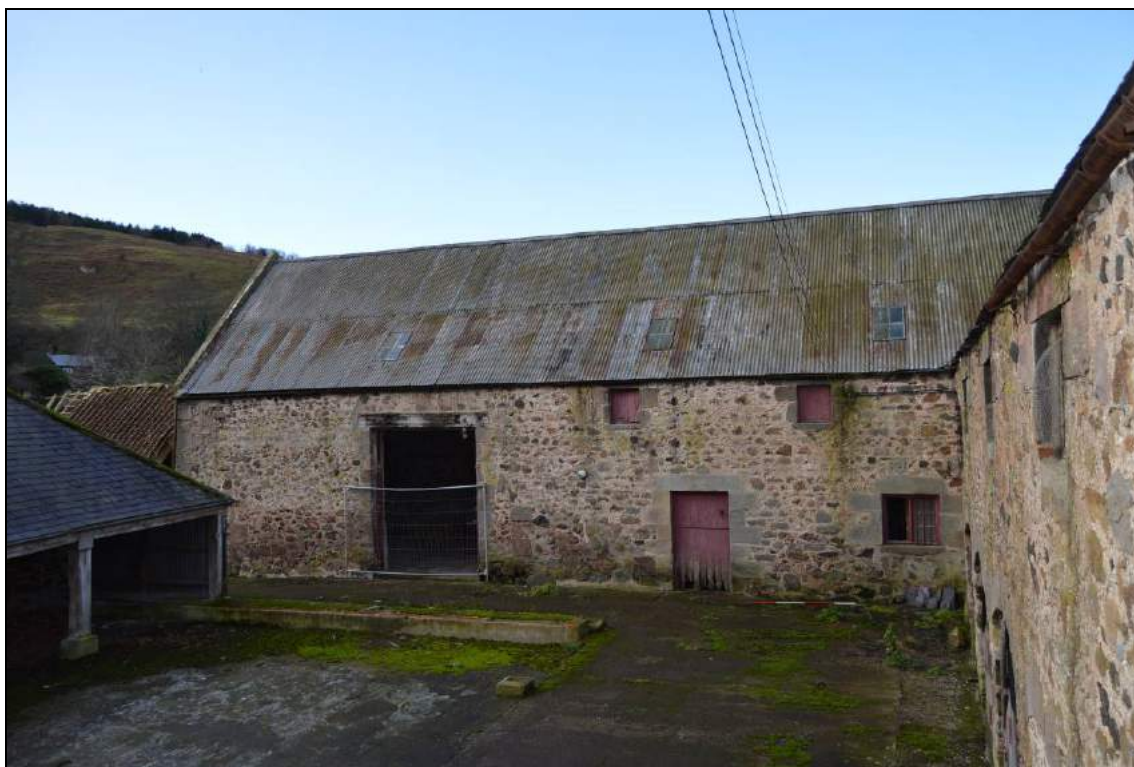
Plate 29: East elevation of the barn (facing west). Scale 2m.
