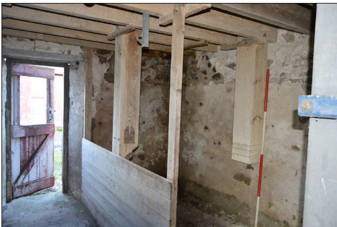
Plate 49: Grain chutes on the ground floor, fed from the first floor hopper above (facing north east). Scale 2m.
