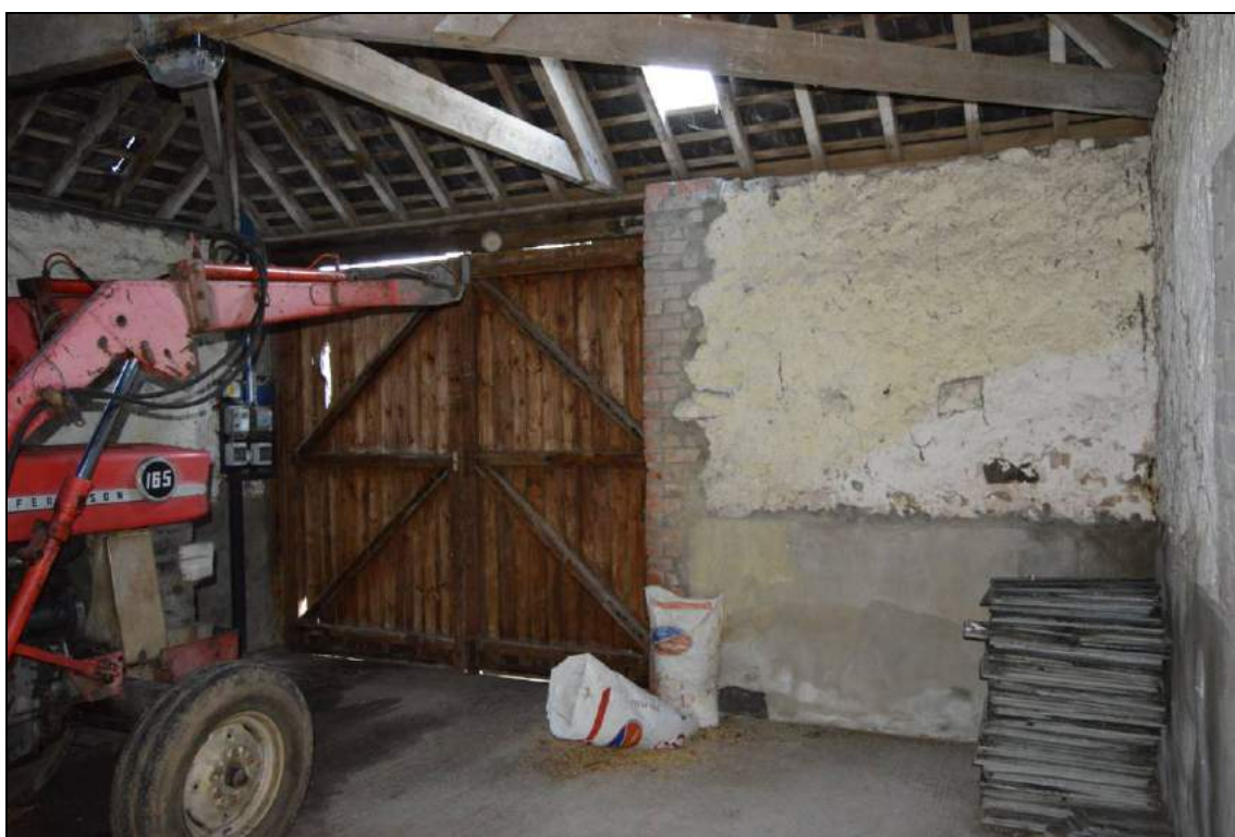
Plate 87: Interior of Building 5 (facing south). Scale 2m.
