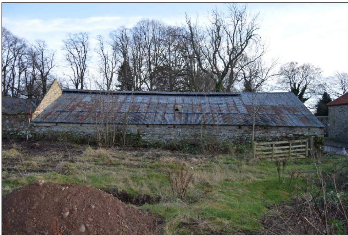
Plate 74: West elevation (facing south east). Scale 2m.
