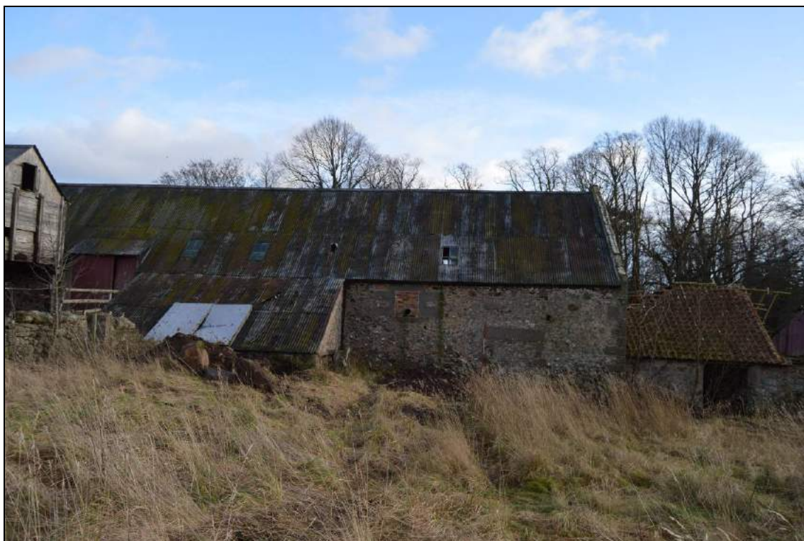
Plate 35: West elevation of barn. Scale 2m.
