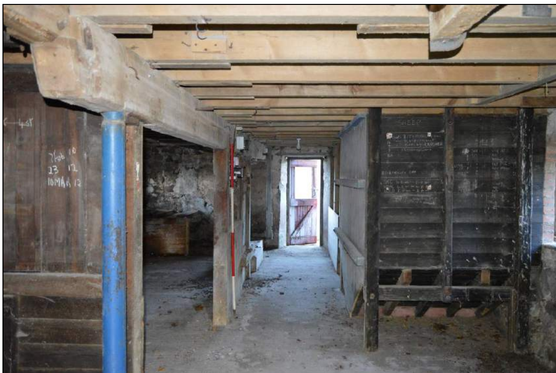
Plate 48: Interior of the barn's ground floor. (facing north). Note the timber grain hopper to the right. Scale 2m.
