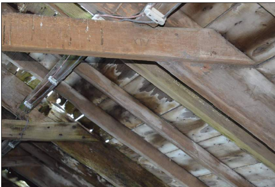
Plate 28: Detail of wooden truss over the granary level (facing east).
