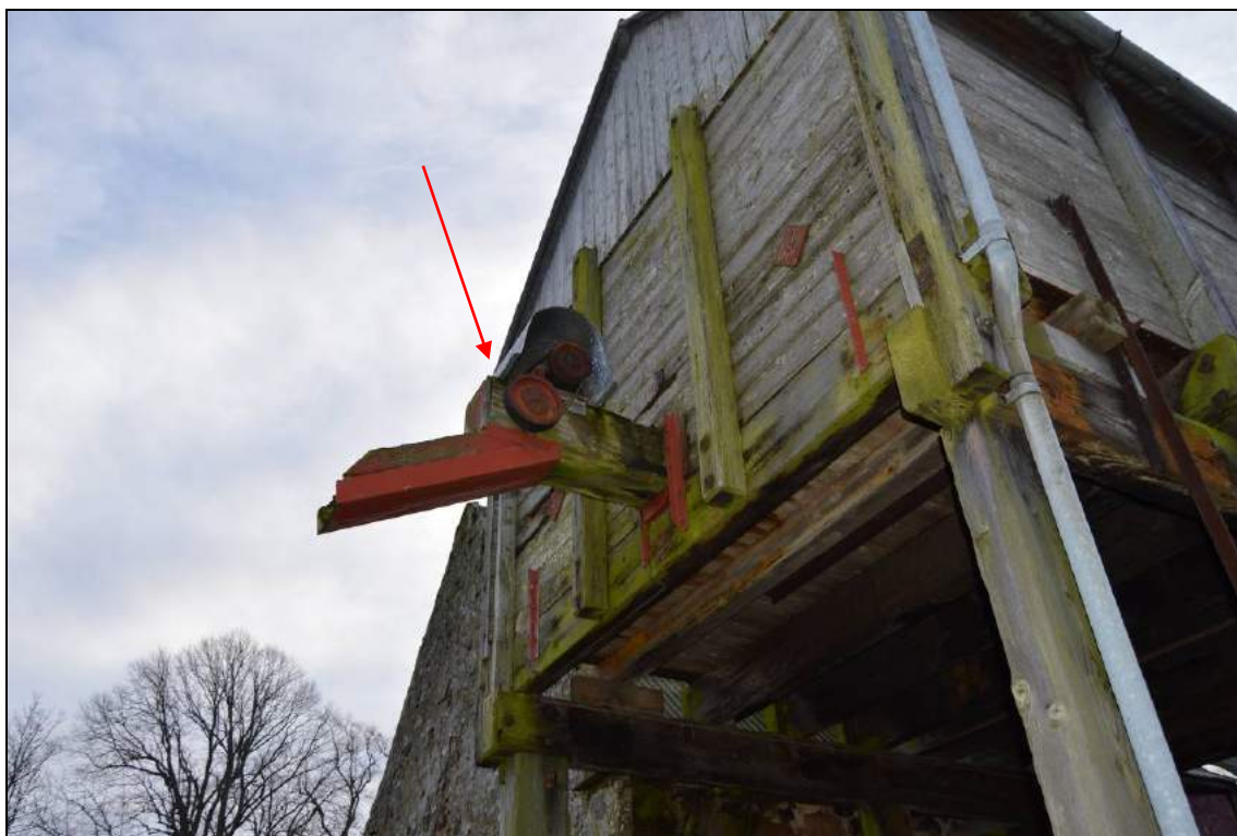
Plate 98: North elevation of grain tower with mechanised conveyor chute (facing east).
