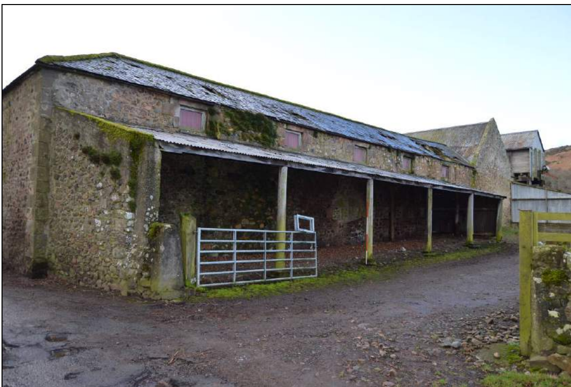
Plate 101: Shelter shed (facing south west). Note. Scale 2m.
