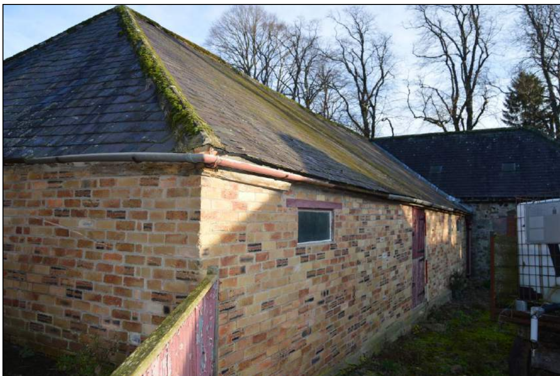
Plate 95: South shelter shed. Scale 2m.
