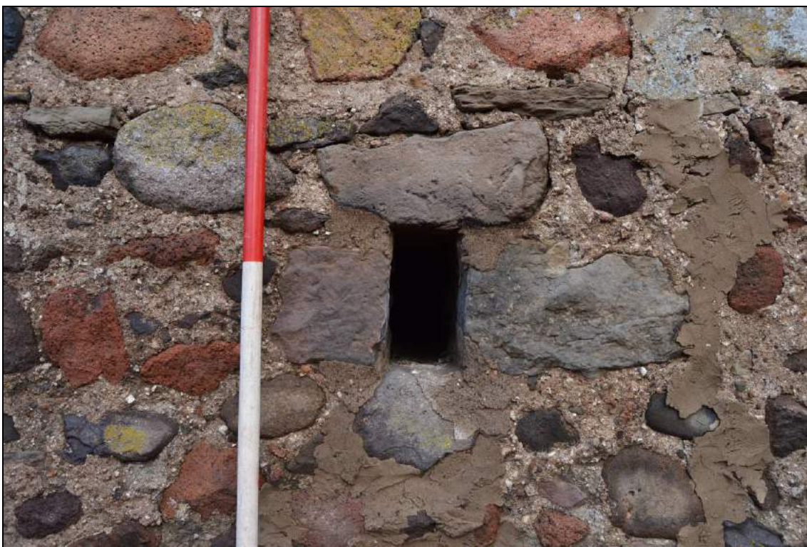
Plate 14: Vent slot detail (facing north west).
