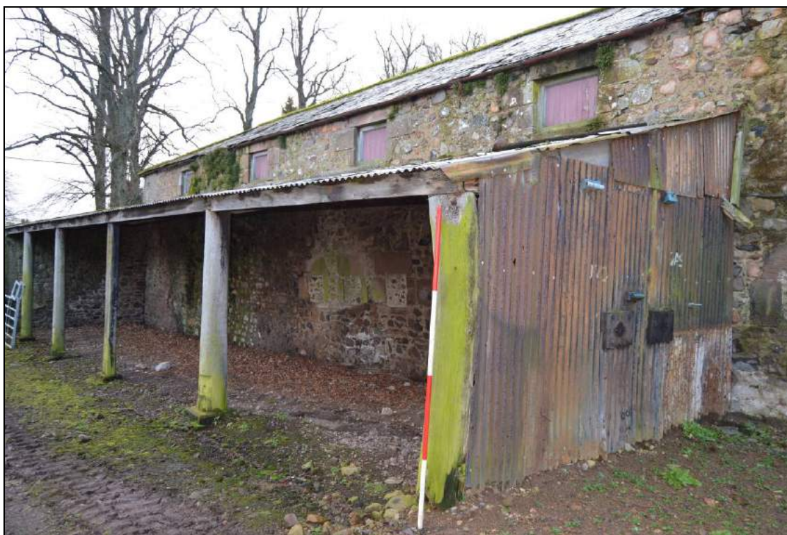
Plate 100: Timber and corrugated metal shelter along the north elevation of the cow-house/granary (facing south east). Scale 2m.
