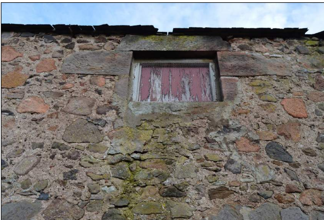
Plate 13: First floor window in east elevation (facing west).
