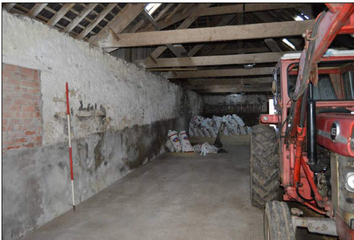
Plate 86: Interior of Building 5 (facing north). Scale 2m.
