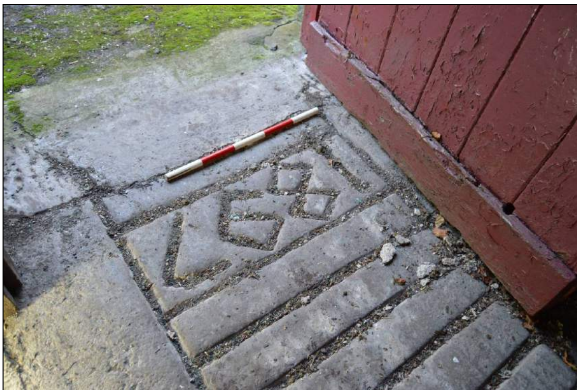
Plate 88: Date cast in the concrete floor (facing north east). Scale 0.5m.
