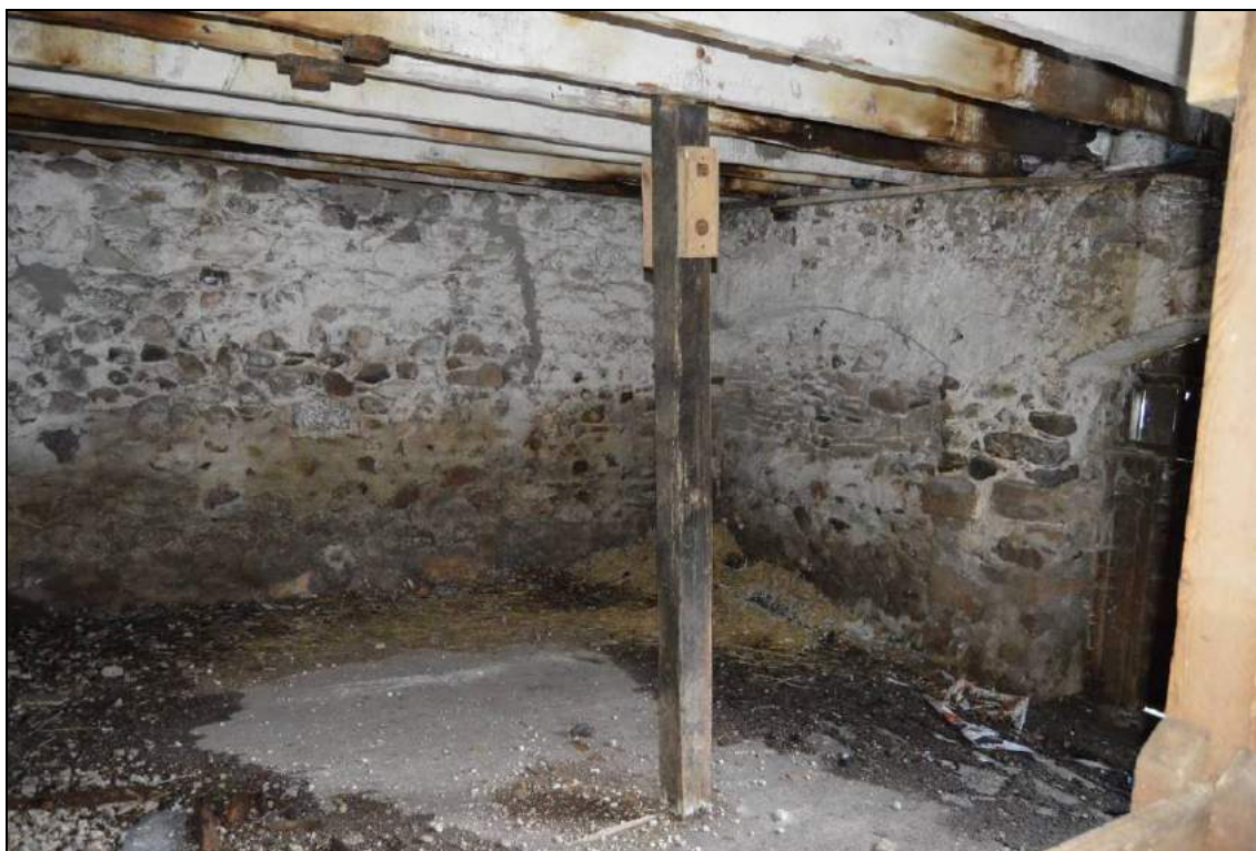
Plate 25: Ground floor of cow house (facing east). (Scale 2m).
