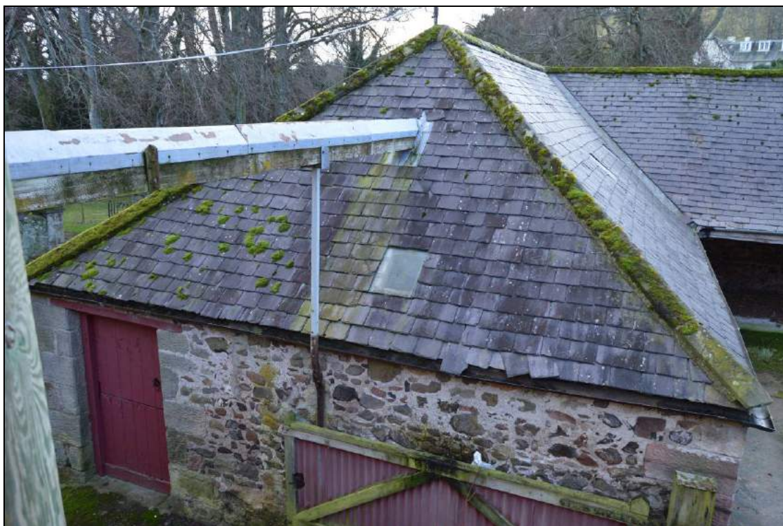
Plate 81: North hip of roof to the east farm range.
