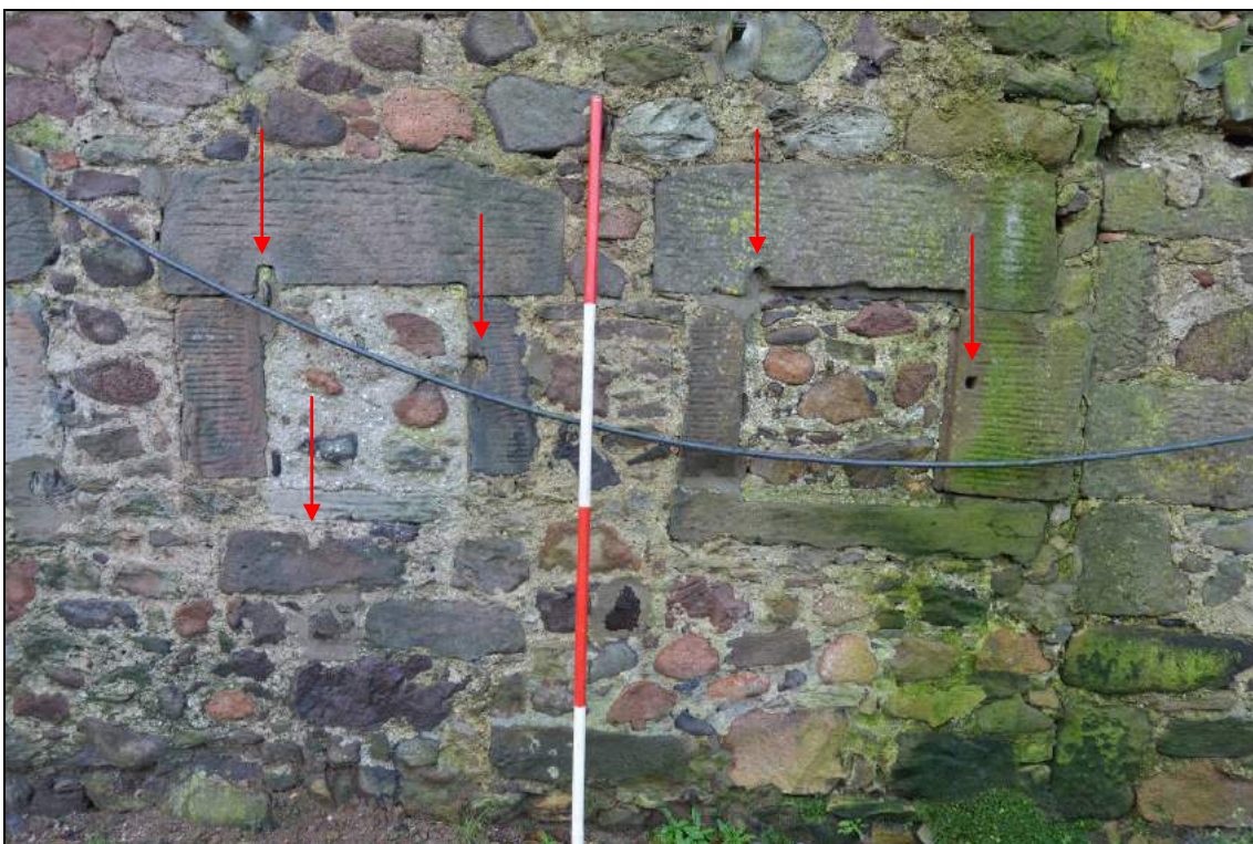
Plate 18: Detail of cow-house apertures to the north elevation (facing south). Note the hinge and latch slots for shutters. Scale 2m.
