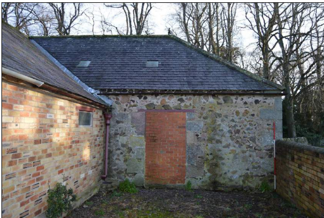
Plate 83: West elevation (facing south east) showing blocked doorway. Scale 2m.
