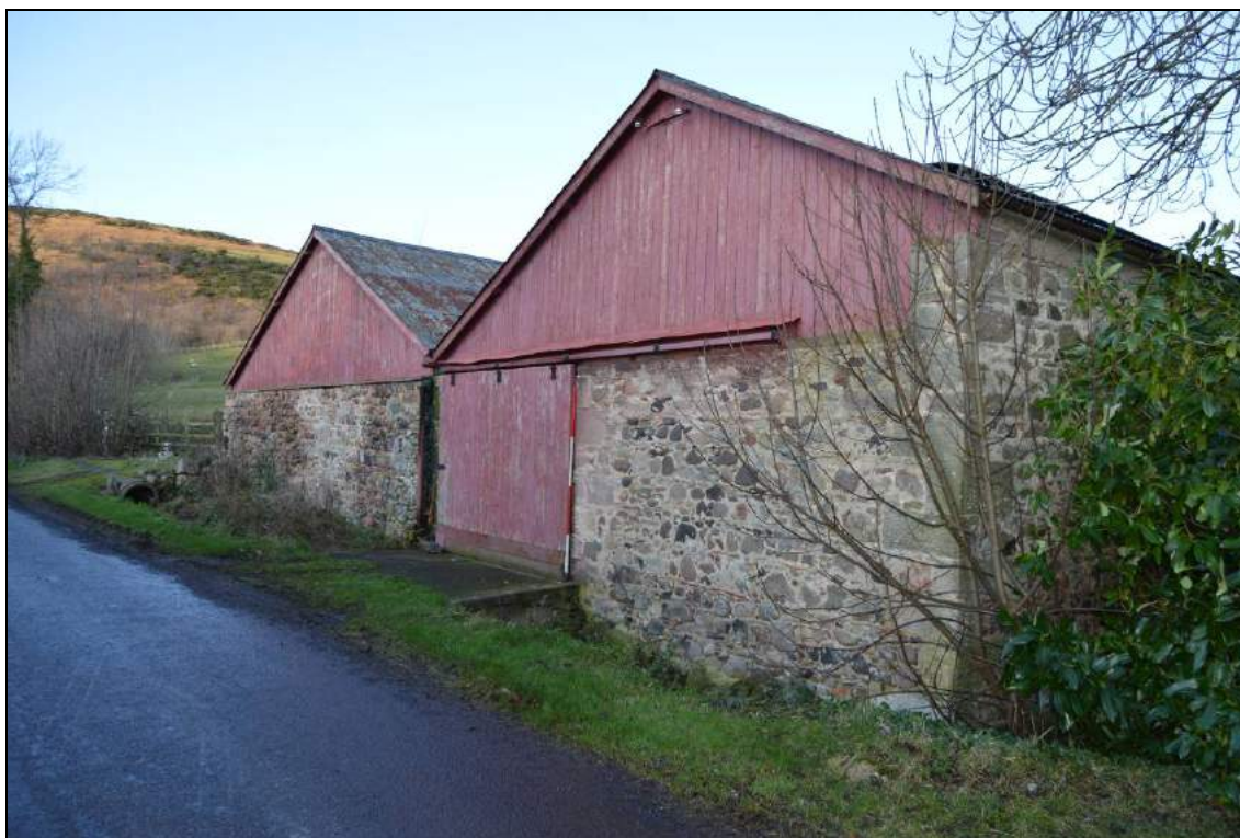
Plate 70: South elevation of south animal shed (facing south east).
