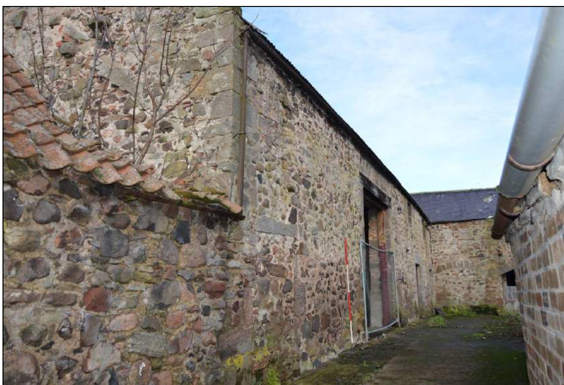
Plate 32: East elevation of the barn (facing west). Scale 2m.
