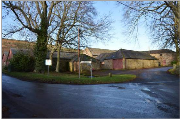
The buildings at North Yearle Steadings from the south east, Earle, Northumberland.
