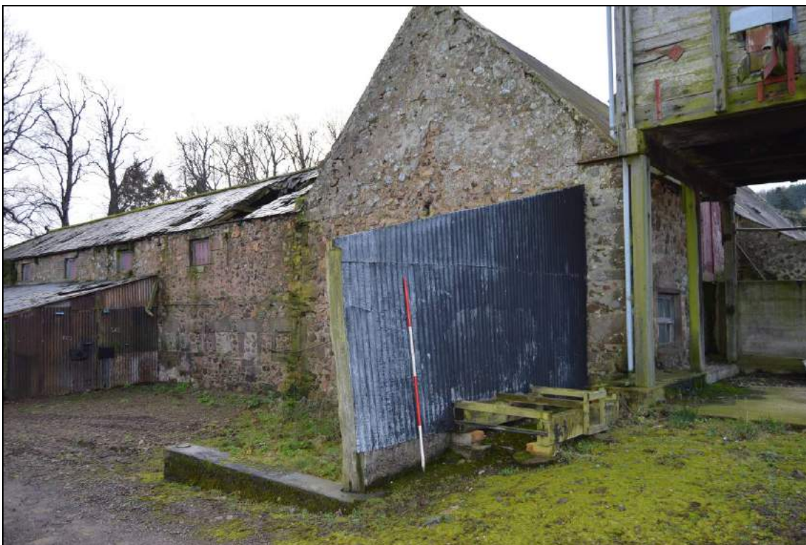
Plate 40: North elevation of barn (facing south). Scale 2m.
