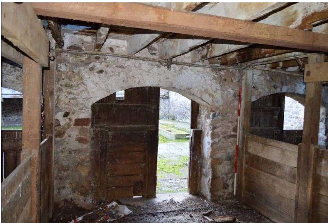
Plate 20: Division of animal stalls inside cow house (facing east). Scale 2m.
