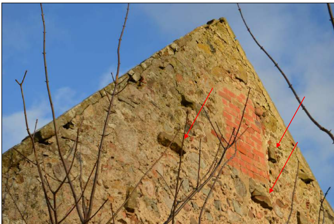
Plate 34: South elevation of the barn with pronounced tie stones (facing north east).
