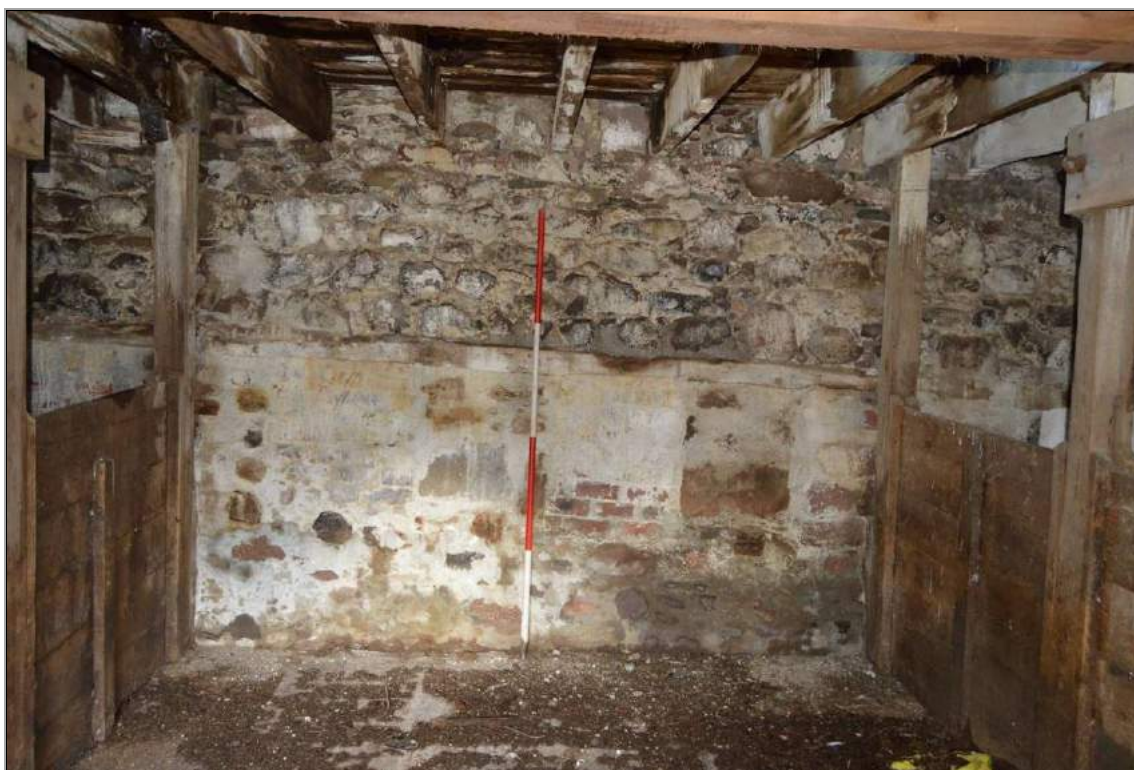
Plate 23: South room with blocked apertures (facing south east). Scale 2m.
