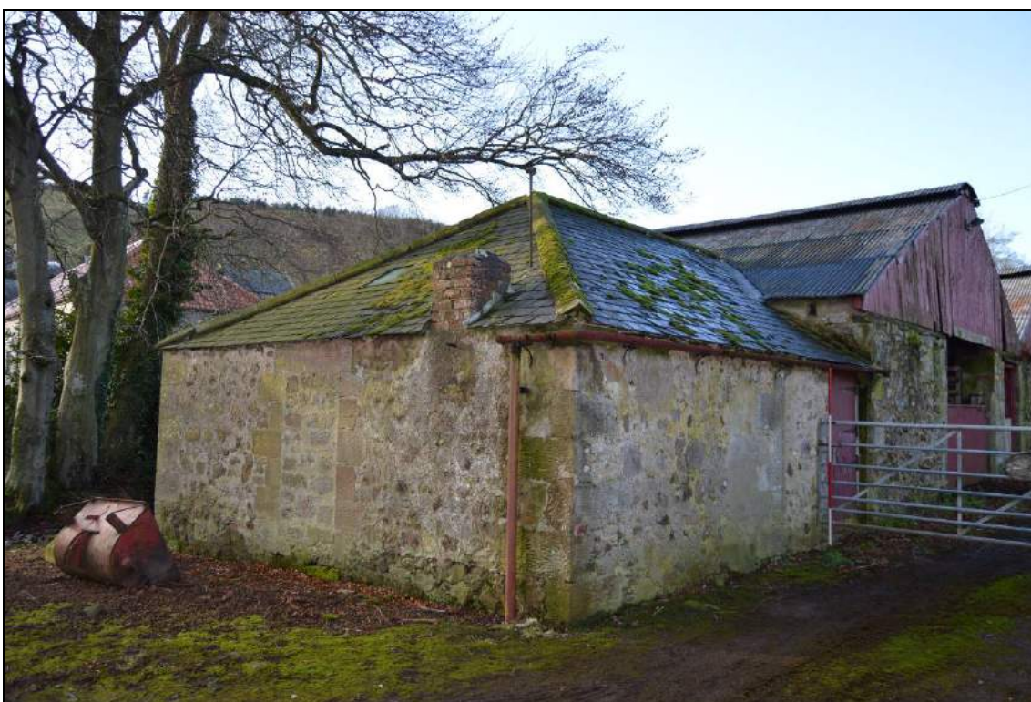
Plate 67: Projecting wing of south animal shed (facing south west). Scale 2m.
