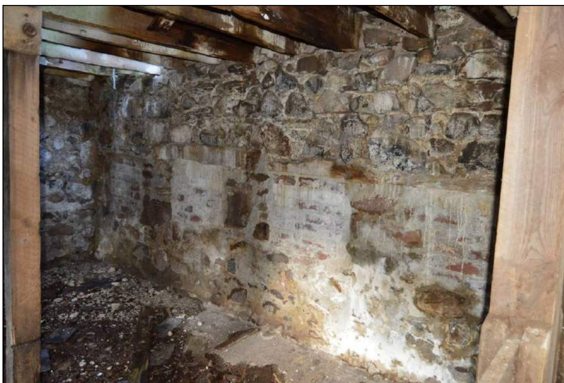
Plate 22: South room (facing east). Scale 2m.
