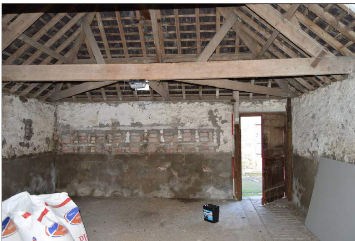
Plate 85: Interior of Building 5 (facing north). Note the brick blocked apertures in the far wall. Scale 2m.
