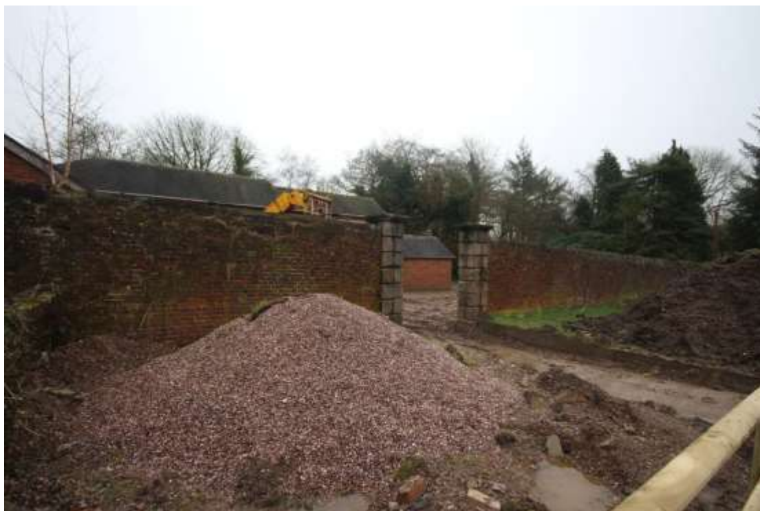
Plate 125: Interior view of the eastern wall of the Walled Garden, facing south east.
