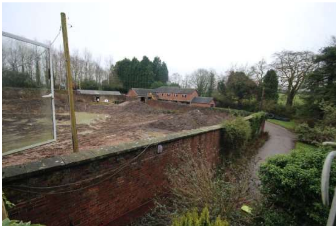
Plate 123: View of the south eastern quarter of the Walled Garden, facing north east. This photograph was taken from the first floor of the Coachman's Halt.
