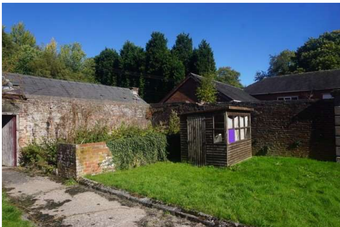
Image 3: View of the north eastern corner of the walled garden, including the remains of the now lost glasshouse base, facing north east. Source: CTD Architects.
