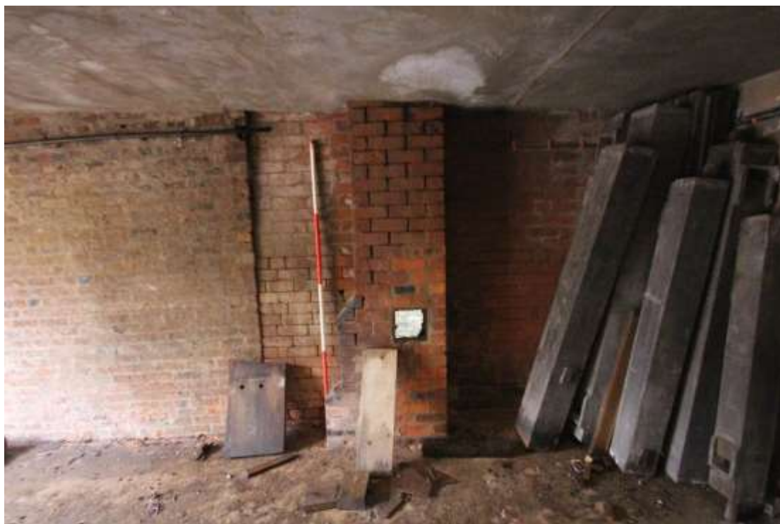
Plate 121: View of the northern side of the western wall inside the small workshop building, facing west. Scale 2m. Note the building break to the left of the scale, defining the original wall and the newly built extension.
