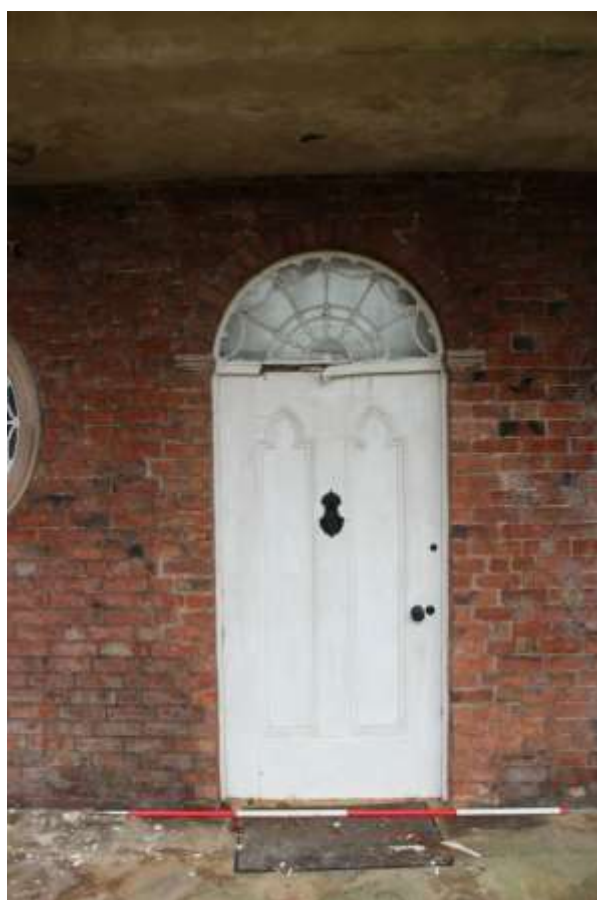
Plate 18: Detailed view of the western front door, facing east. Scale 2m.
