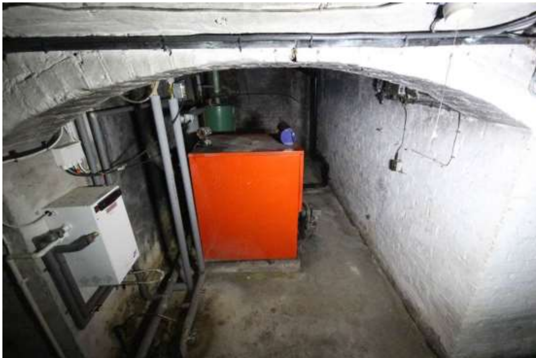
Plate 83: Looking into the Boiler Room from the corridor, facing west.
