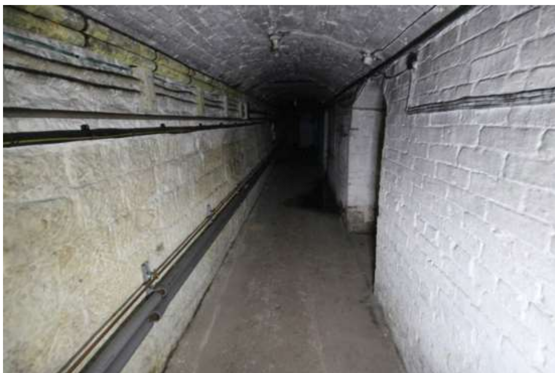
Plate 69: View of the north-south corridor in the Basement, facing south. Note the way in which the concrete floor here seems to cover a line of masonry, suggesting it has been raised.
