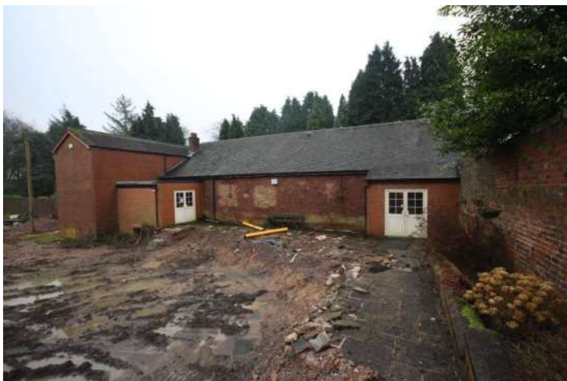
Plate 97: View of the northern elevation of the Halcyon Room, facing south. This northern wall has been reused and is likely part of the original stable block that once stood here.
