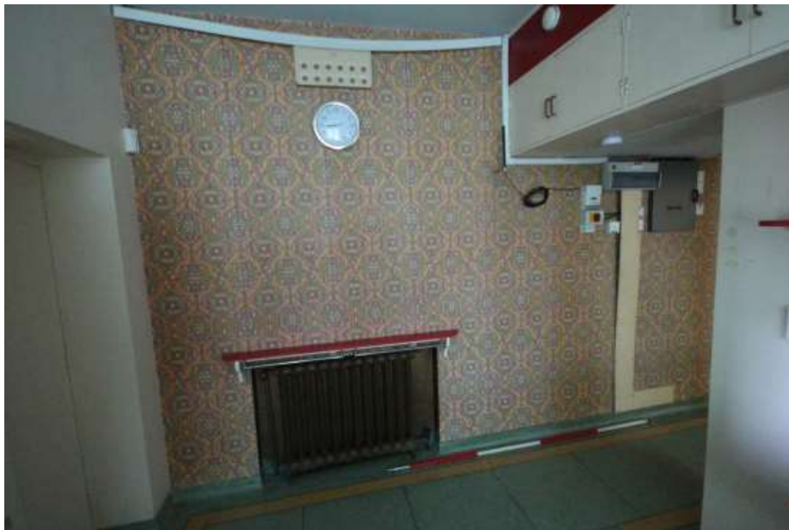
Plate 53: View of the western wall of the Utility Area, taken from the Kitchen facing west. Scale 2m.
