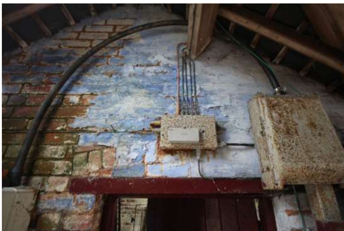
Plate 108: Detailed view looking above the doorway to the western room of the Potting Shed, facing west. Note the relieving archway above the door.
