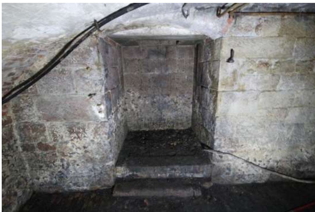
Plate 74: Detailed view of the alcove and former doorway in the northern elevation of the northern store, facing north. Scale 2m.
