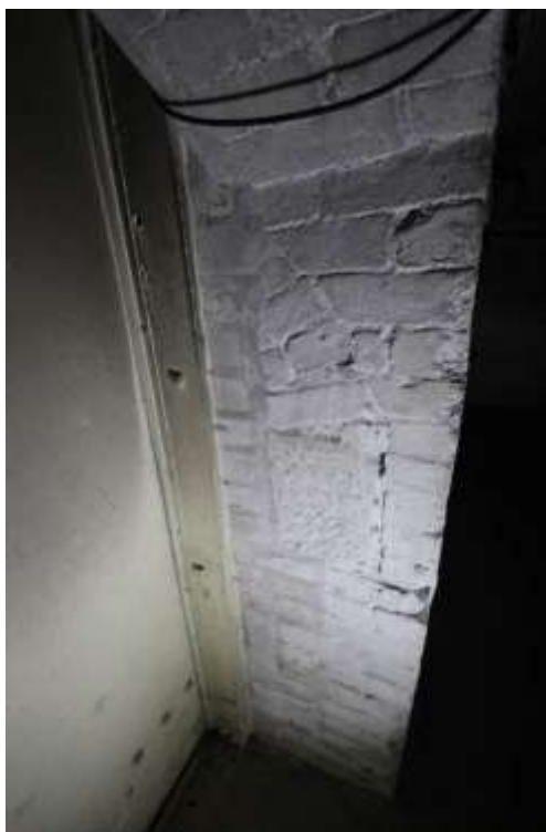
Plate 79: Detailed view of the blocked opening visible immediately next to the Wine Cellar doorway, facing north west.
