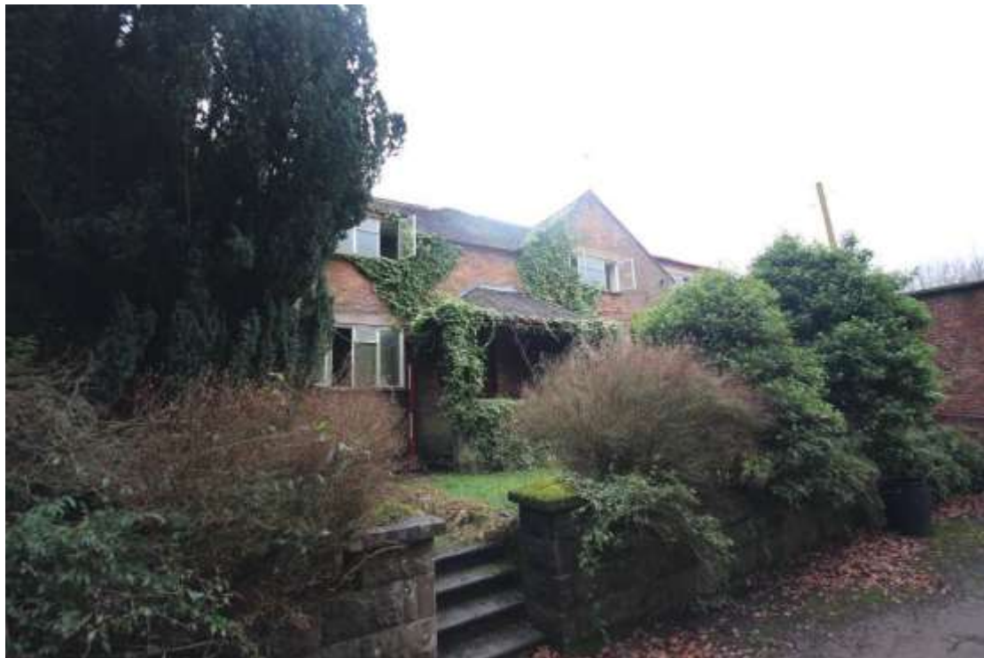
Plate 126: View of the eastern elevation of the Coachman's Halt, facing west. Scale 2m.
