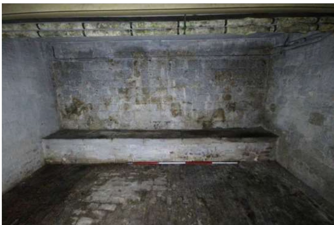
Plate 86: View of the southern elevation of the southern Store room, facing south. Scale 2m. The raised bench visible here contains three relieving arches.
