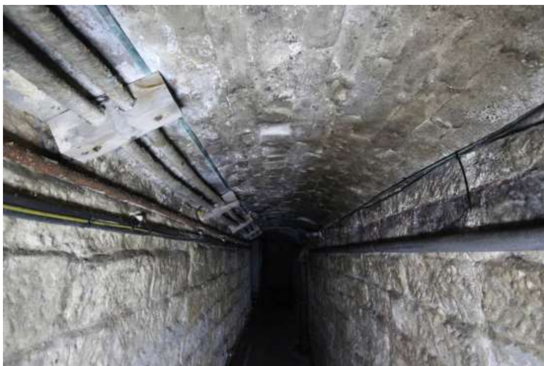
Plate 67: View of the corridor running east-west in the Basement, facing west.
