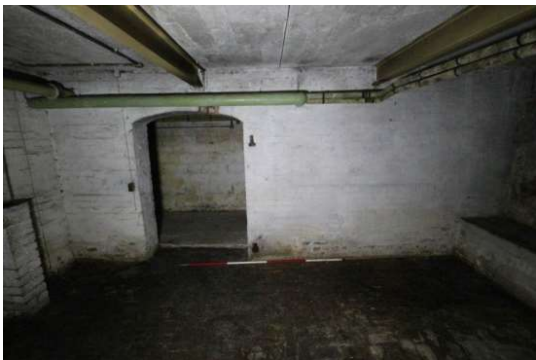
Plate 90: View of the eastern elevation of the southern Store room, facing east. Scale 2m. Note the remaining iron pintel and latch fastener, this is evidence of a former doorway.
