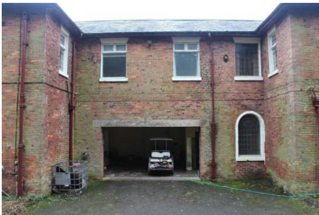
Plate 7: View of the central northern elevation of Block A, facing south. Scale 2m.
