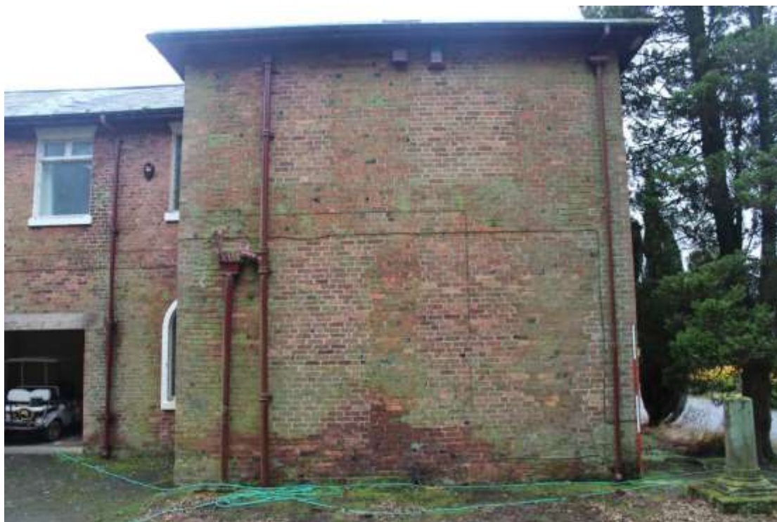
Plate 5: View of the western wing's northern elevation, facing south. Scale 2m.
