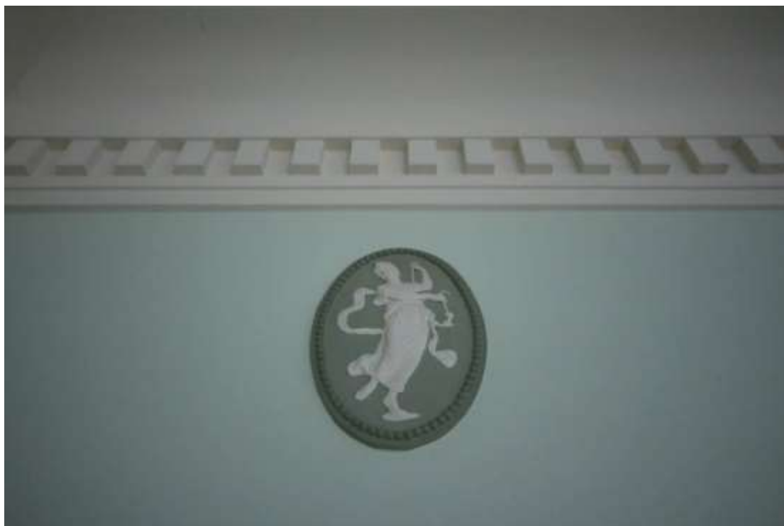
Plate 52: Detailed view of the dogtooth cornice and plaster roundel in the northern elevation of the Dining Room, facing north.
