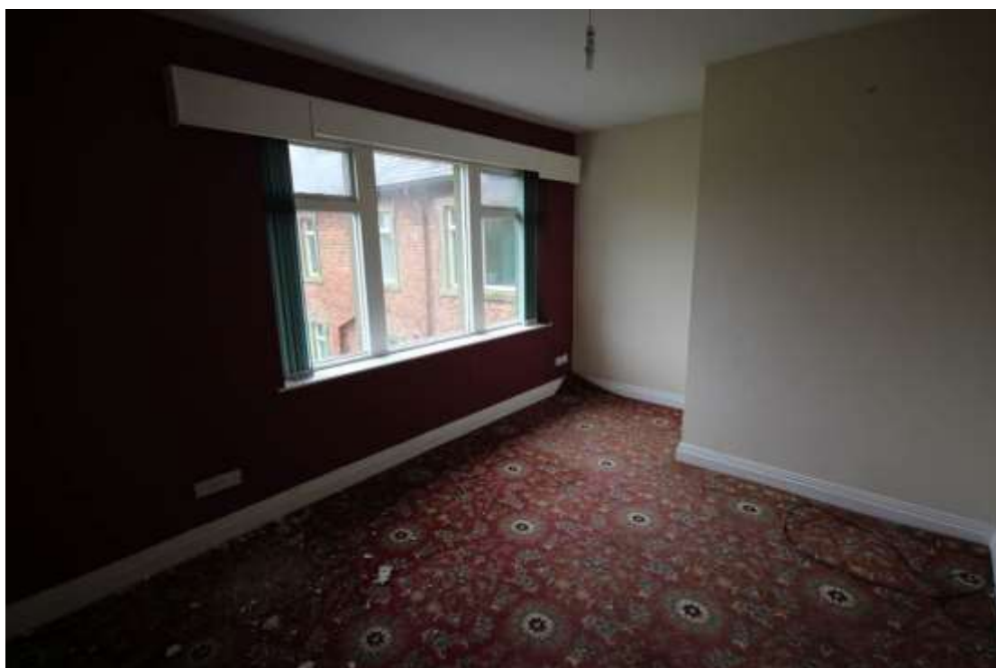
Plate 37: View of the first floor Sitting Room in the eastern part of Block A, facing south west.
