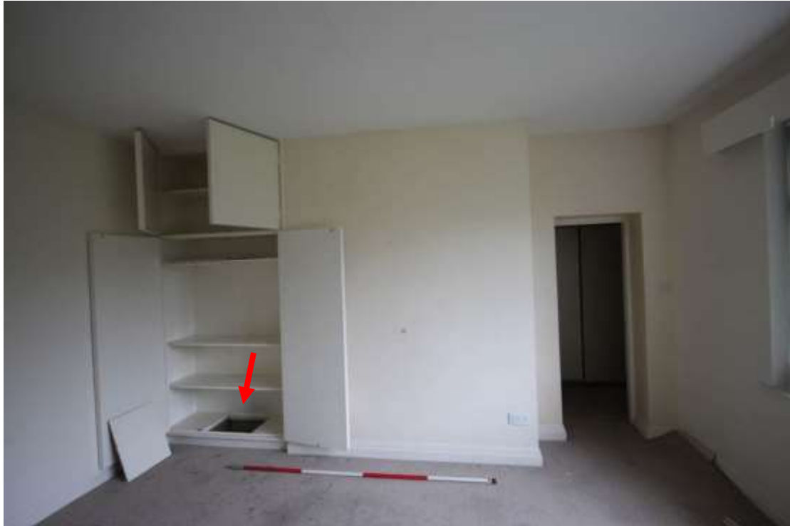
Plate 59: View of the northern part of Bedroom 1, facing north. Scale 2m. The arrow indicates the access to the Crawl Space underneath this room.
