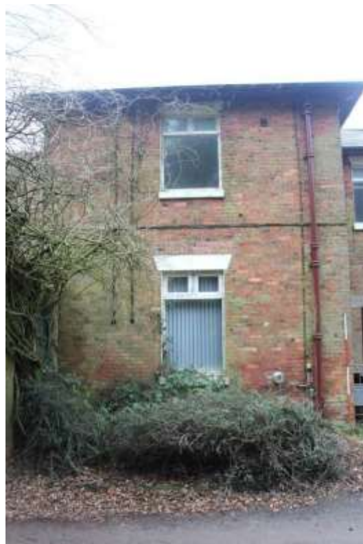
Plate 8: View of the eastern wing's northern elevation, facing south. Scale 2m.
