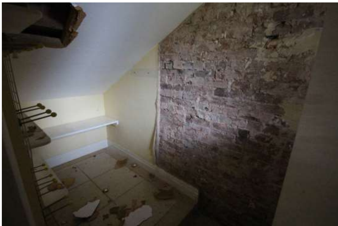
Plate 44: View of the storage area in the Porch, facing east.
