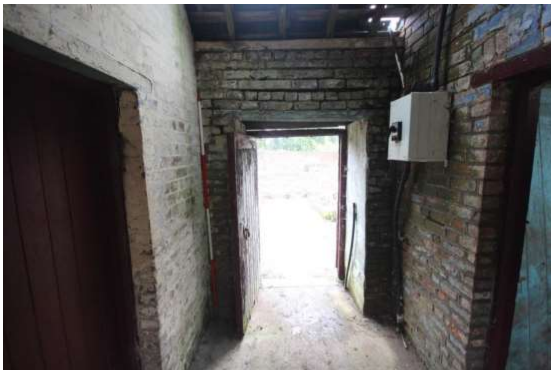
Plate 107: View of the southern doorway leading into the central corridor of the Potting Shed, facing south. Scale 2m.
