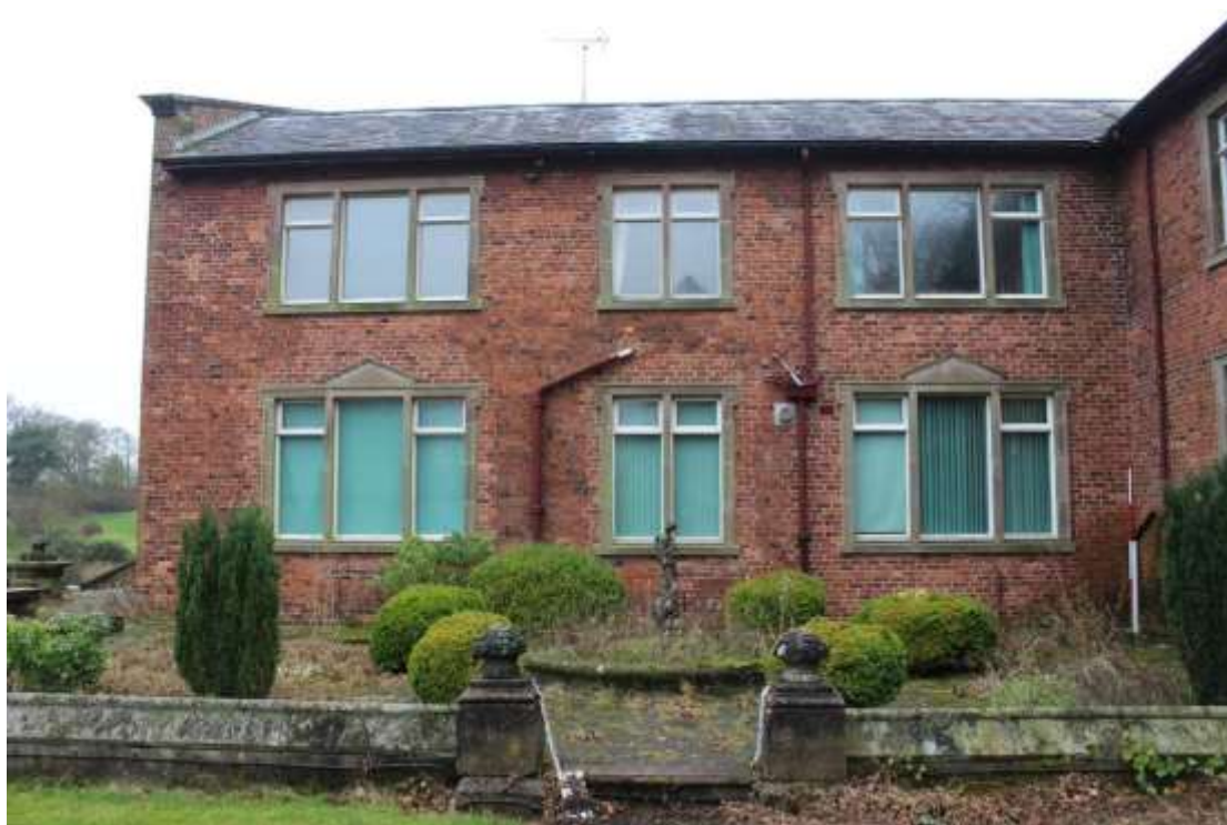
Plate 15: View of the eastern elevation of Block B, facing west. Scale 2m.
