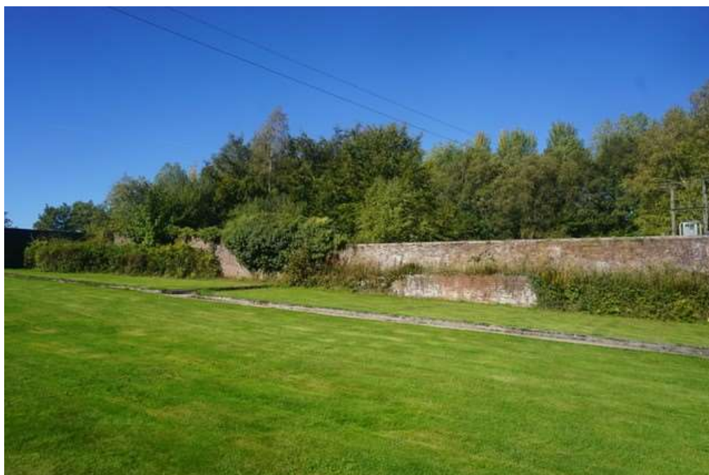
Image 1: The glasshouse bases along the internal northern wall of the Walled Garden, facing north west. Source: CTD Architects.
