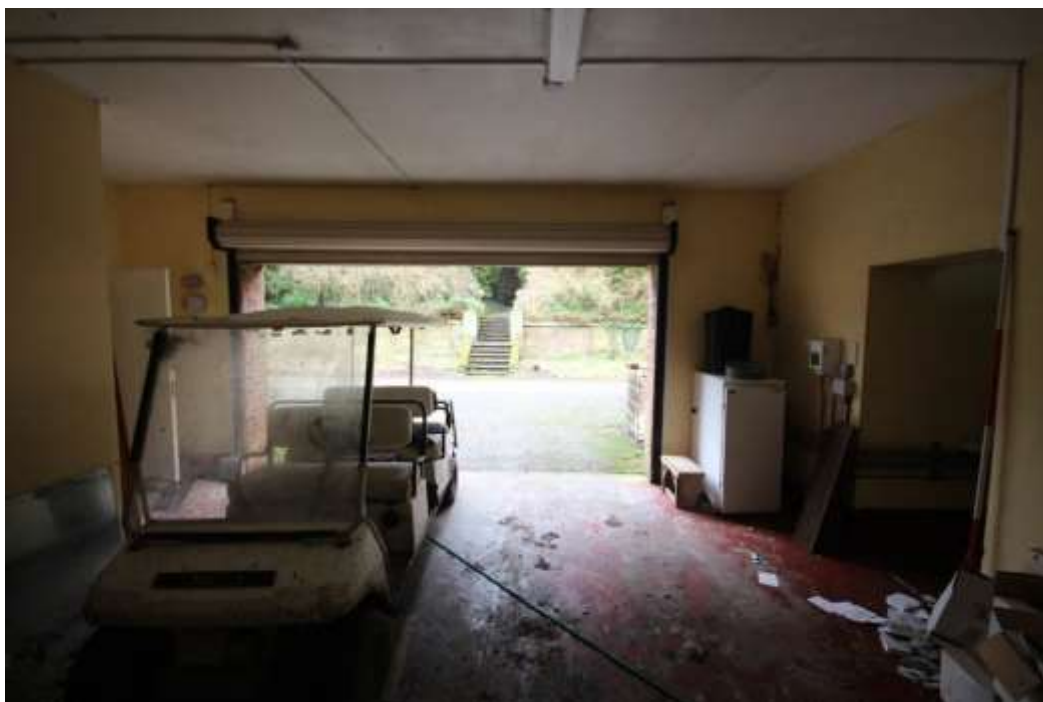
Plate 26: View of the northern half of the garage, facing north.
