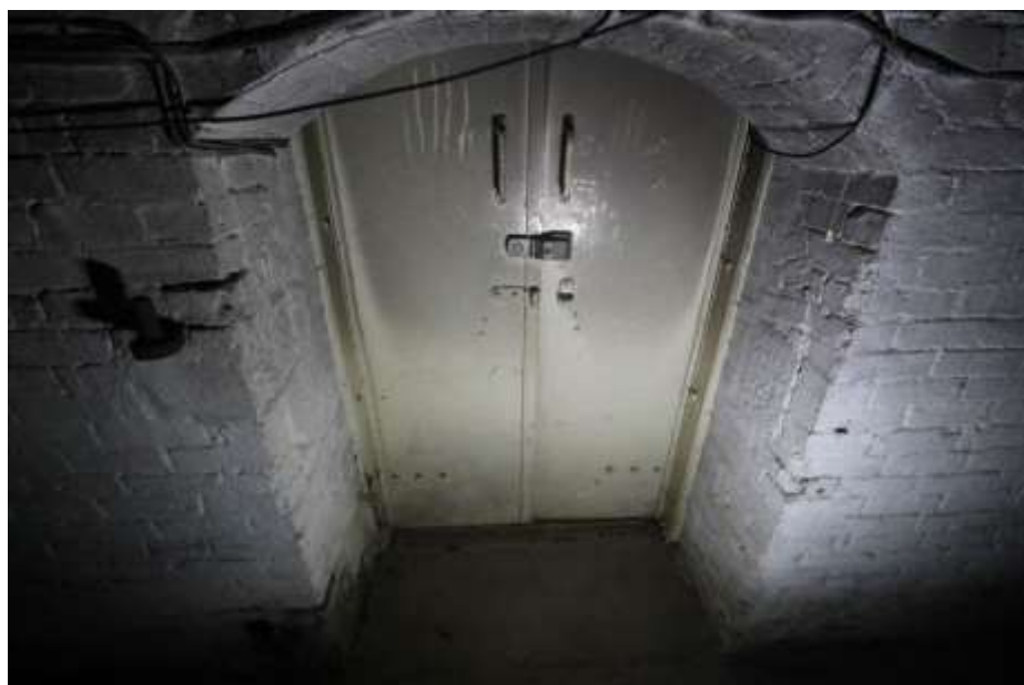
Plate 78: View of the doorway leading into the wine cellar, facing west. Note the iron pintel visible to the left of this opening.
