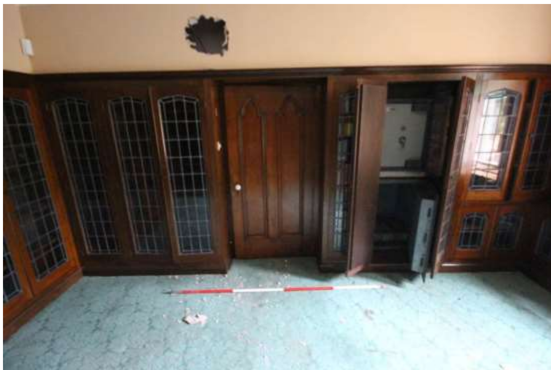
Plate 24: View of the library, facing south. Scale 2m.
