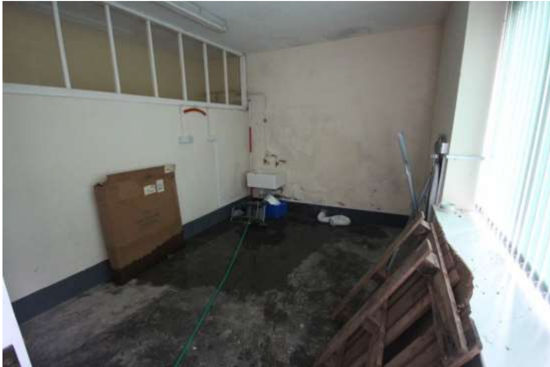
Plate 27: View of the laundry room, facing north east.
