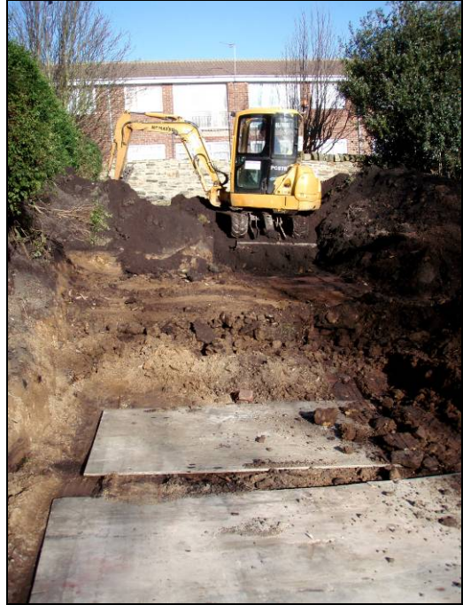
Mini-digger removing topsoil from the north section.
