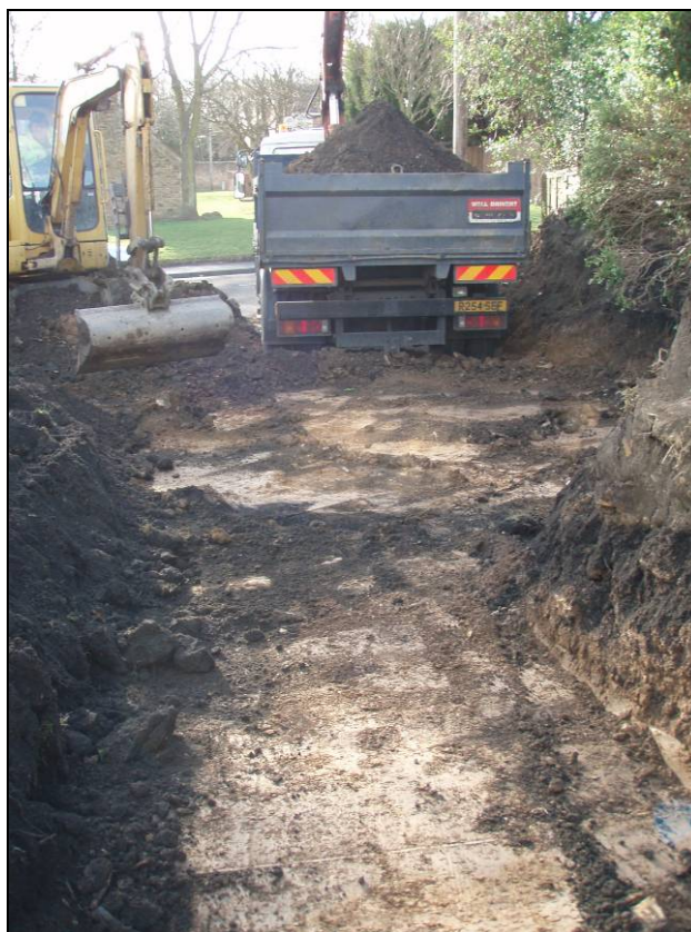
Fig. 4 excavation of topsoil down to natural sand.
