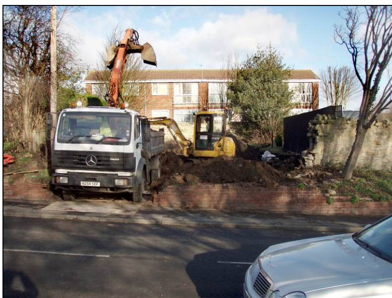
Fig. 3 North view of the study area showing site access.
