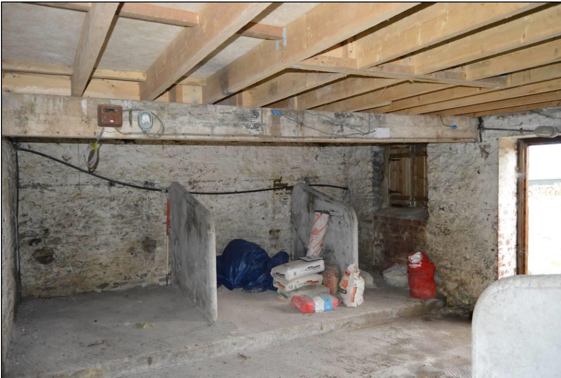
Plate 22: Ground floor of building 1 (facing south east). Scale 1m.
