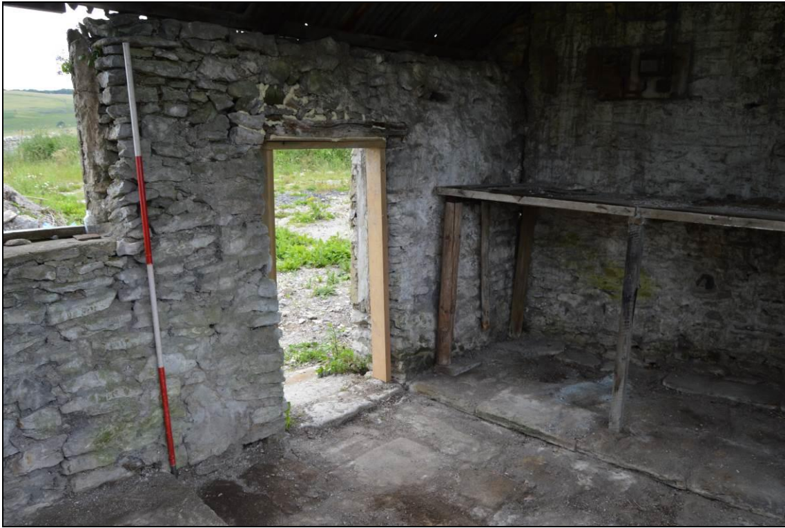
Plate 41: Interior of building 2 (facing south west).
