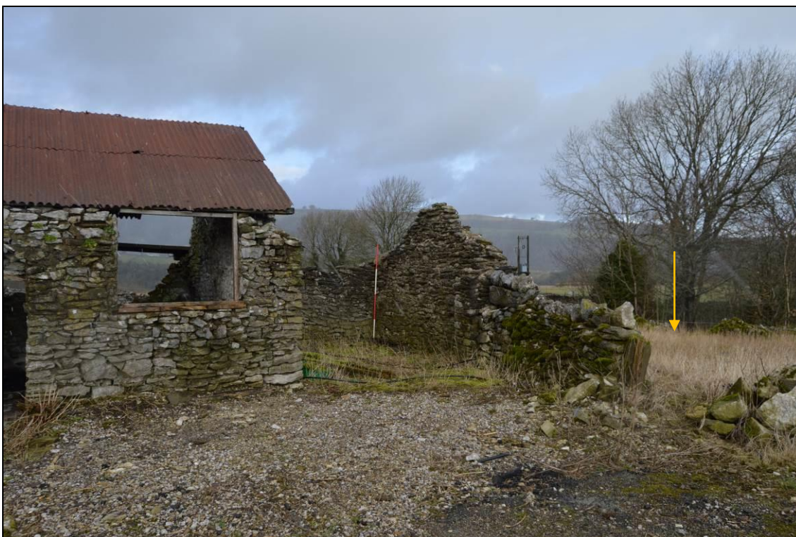
Plate 49: Building 3 and part of the enclosure wall (facing north east). To the right, the small eastern enclosure (indicated) which building 3 originally adjoined. Scale 2m.
