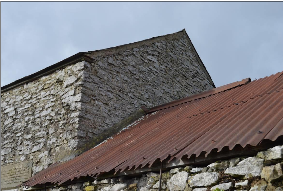
Plate 20: East elevation from the foldyard (facing north west).
