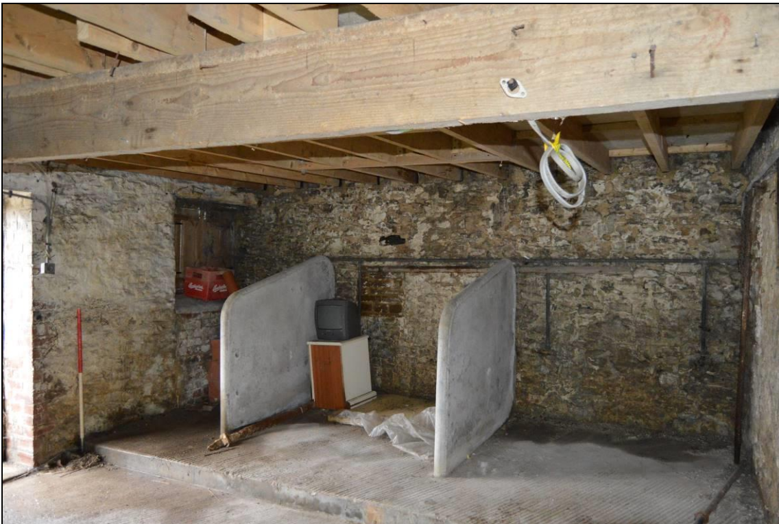
Plate 23: Ground floor of building 1 (facing south east). Scale 1m.
