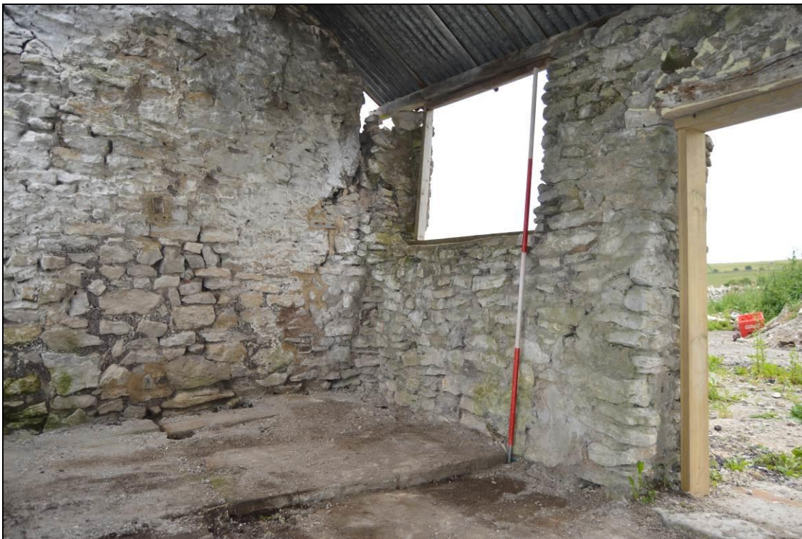
Plate 40: Interior of building 2, (facing south east). Scale 2m.
