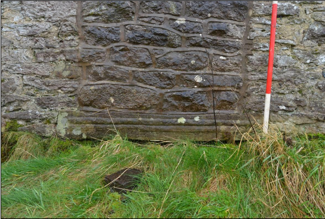
Plate 7: Moulded stone step to blocked doorway in north elevation. Scale 2m.
