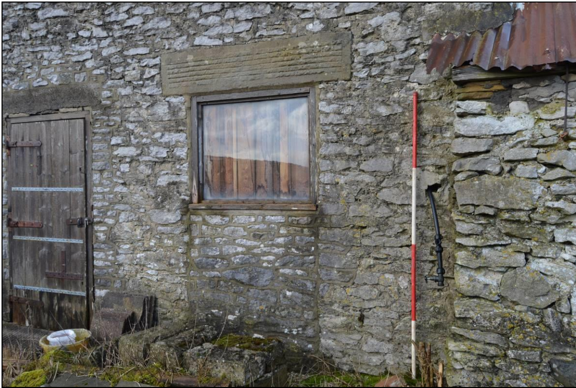
Plate 15: Former east door to the south elevation, facing north. Scale 2m
