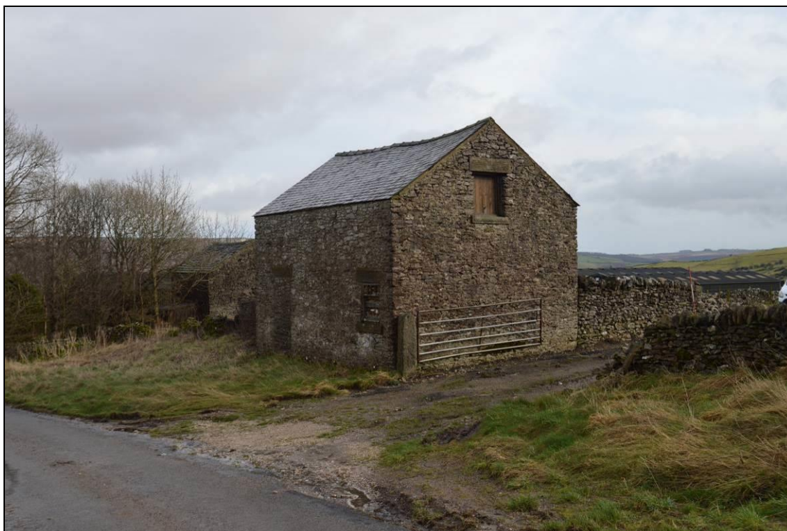
Plate 1: The former outfarm buildings from Middleton Lane (facing south east).
