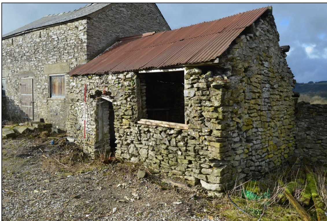
Plate 36: South elevation of building 2 (facing north west). Scale 2m.
