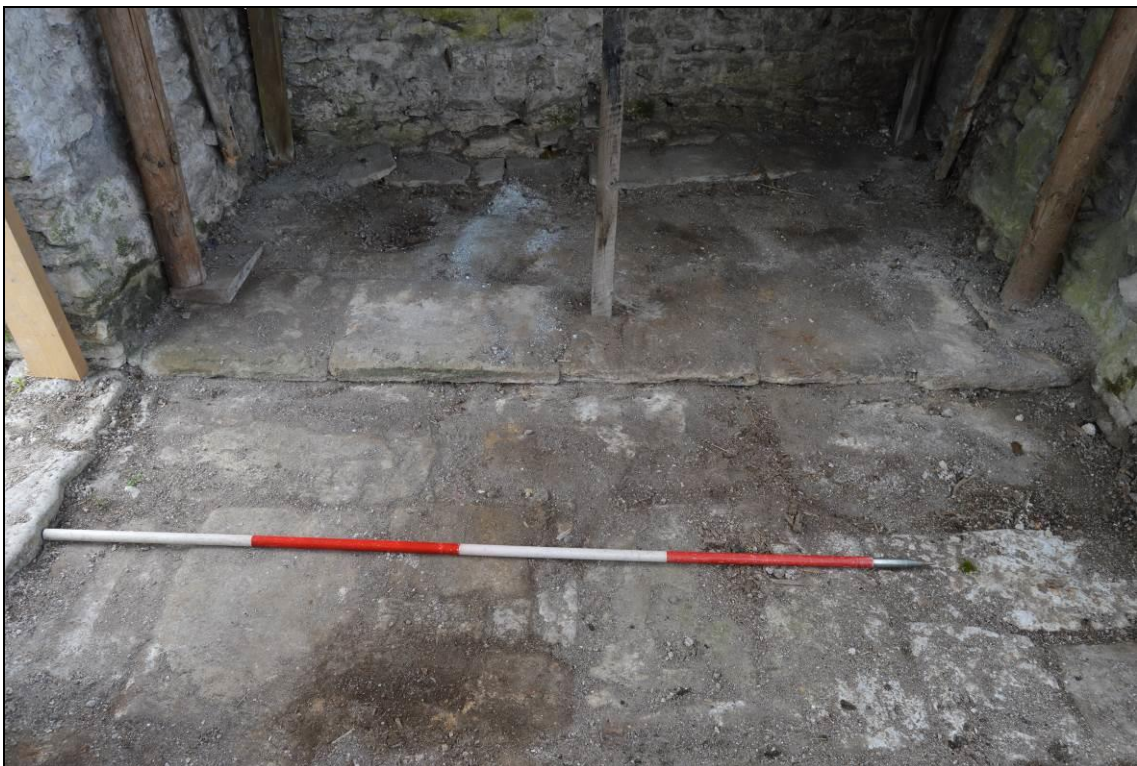
Plate 42: Interior of building 2 with remains of cattle stall flooring (facing west).
