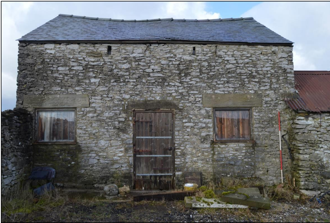
Plate 13: South elevation of building 1, facing north. Scale 2m.
