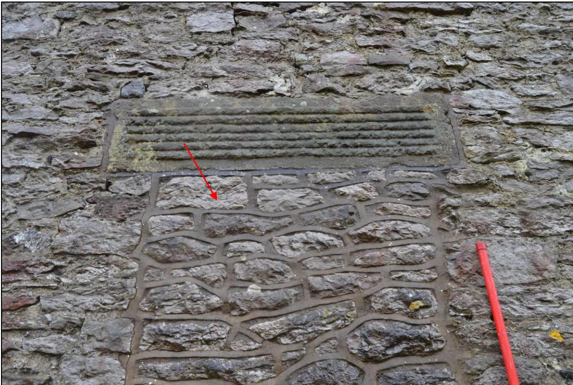
Plate 6: Moulded stone lintel to east doorway in north elevation (facing south). Scale 2m.
