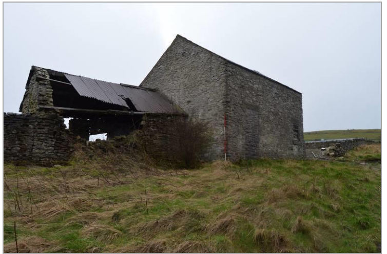
View of Highfields Farm Barn, Stoney Middleton, Derbyshire.
