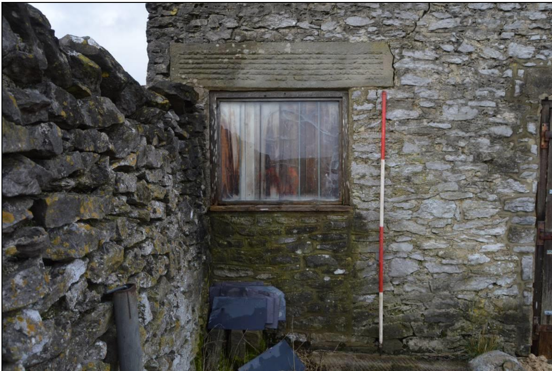
Plate 14: Former west door to the south elevation, facing north. Scale 2m.
