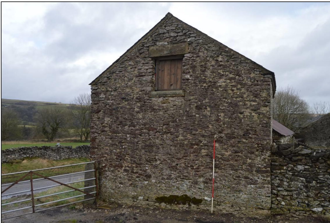
Plate 9: West elevation of the cow house (facing east). Scale 2m.
