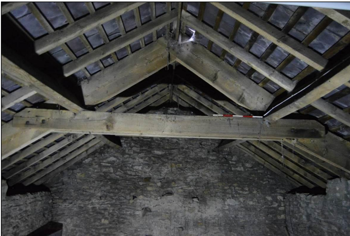
Plate 35: Roof structure of the barn (facing west). Scale 0.5m.
