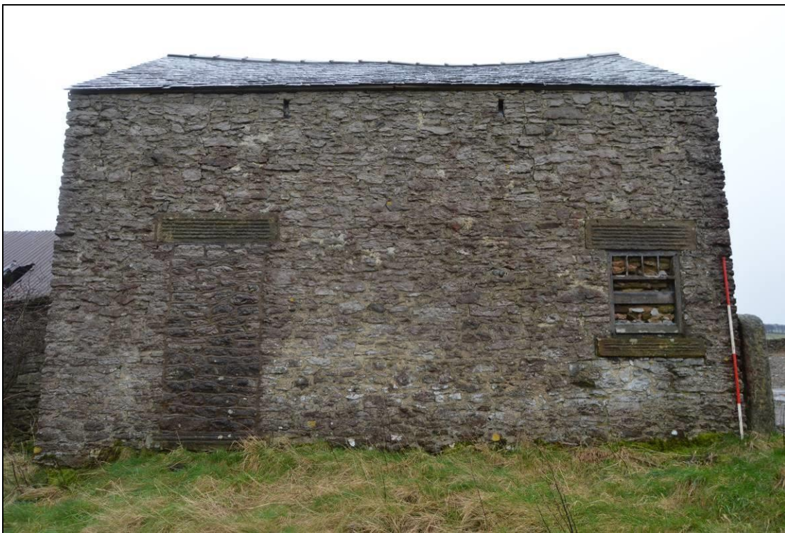
Plate 4: View of the north elevation to building 1 facing south. Scale 2m.
