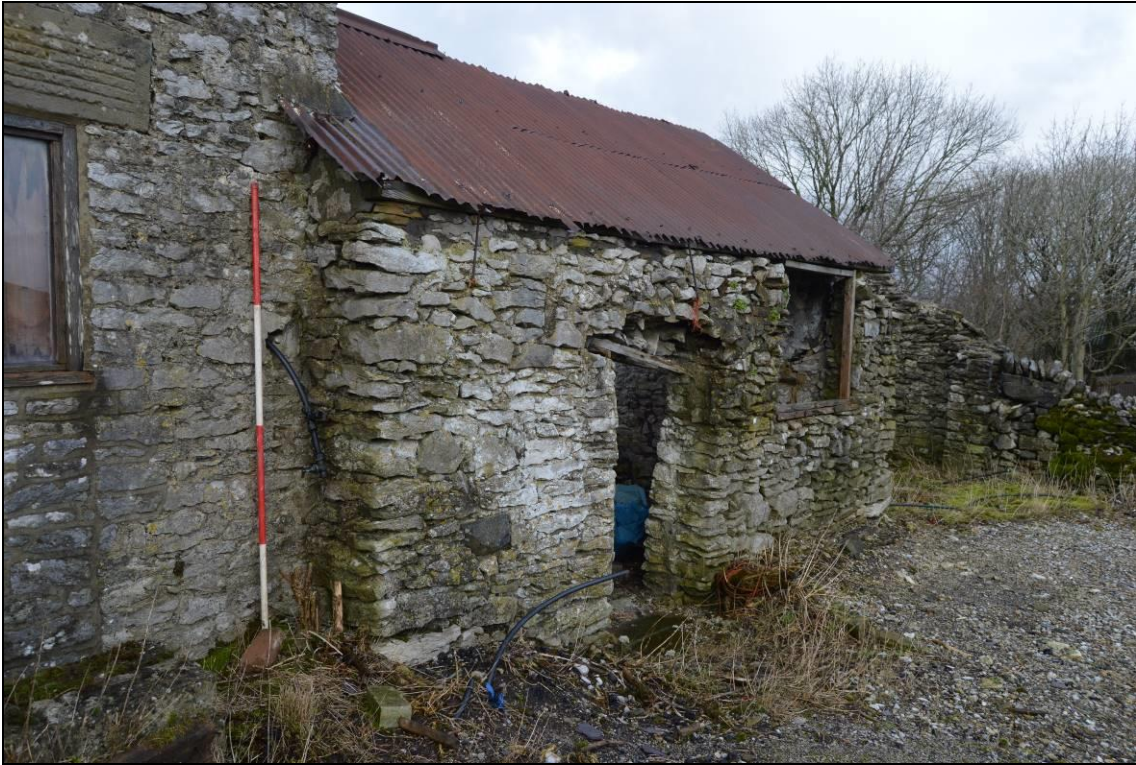
Plate 37: South elevation of building 2 (facing north east). Scale 2m.
