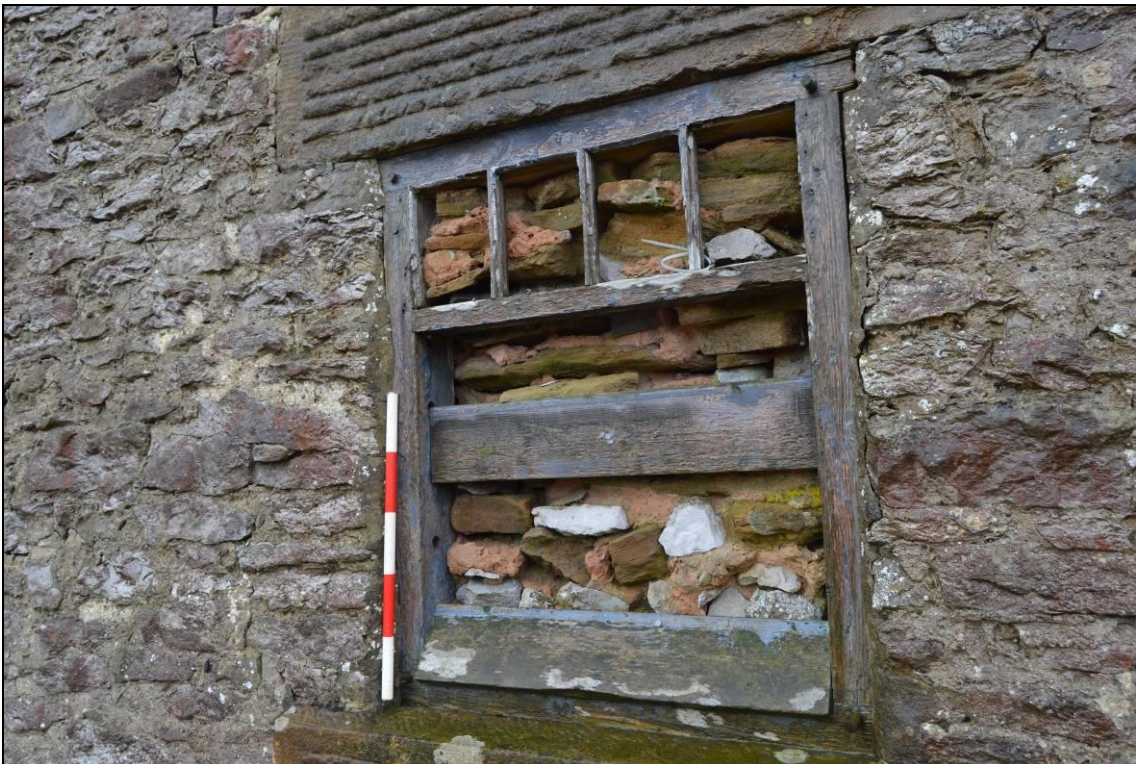
Plate 8: Retained window casement with louvered vents in north elevation (facing south east). Scale 0.5m.
