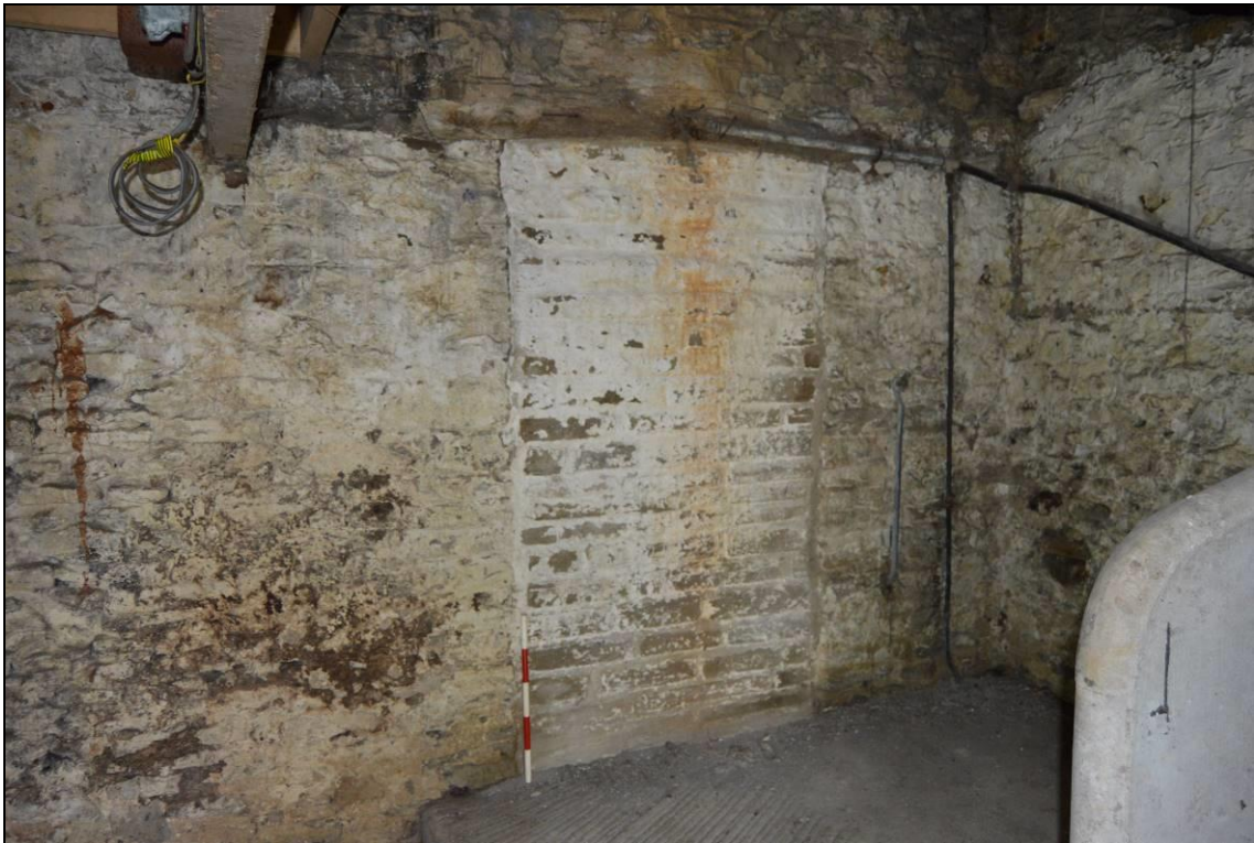
Plate 24: Ground floor of building 1 (facing south east). Scale 0.5m.
