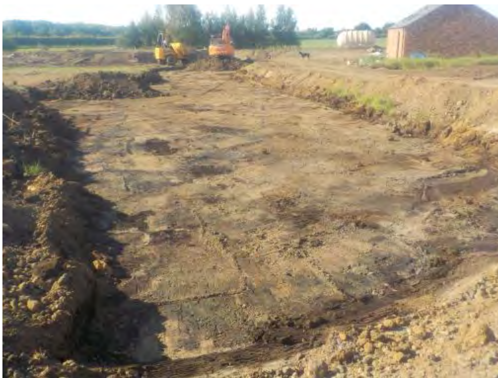
Figure 12. Area 3 Working shot, view to southwest
