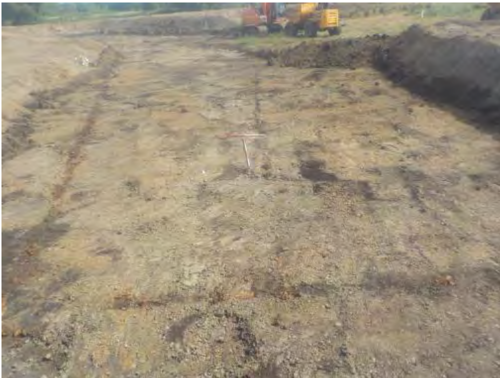
Figure 15. Area 3 working shot, view to northeast
