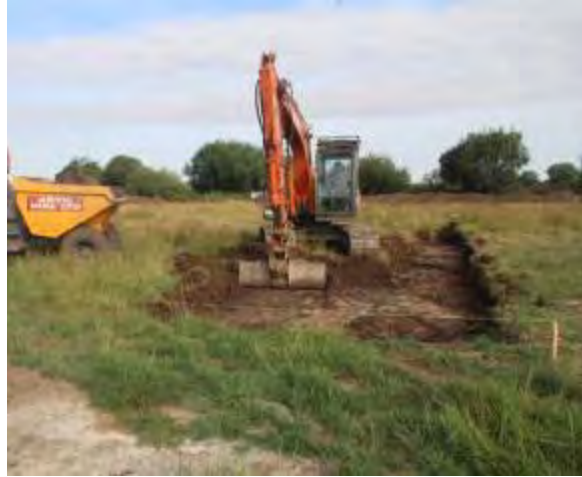
Topsoil strip, phase 1
