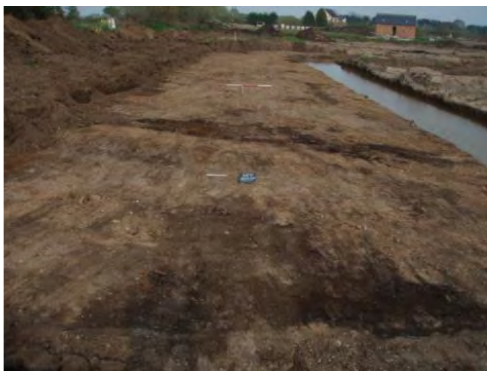
Figure 5. Area shot, view to west
