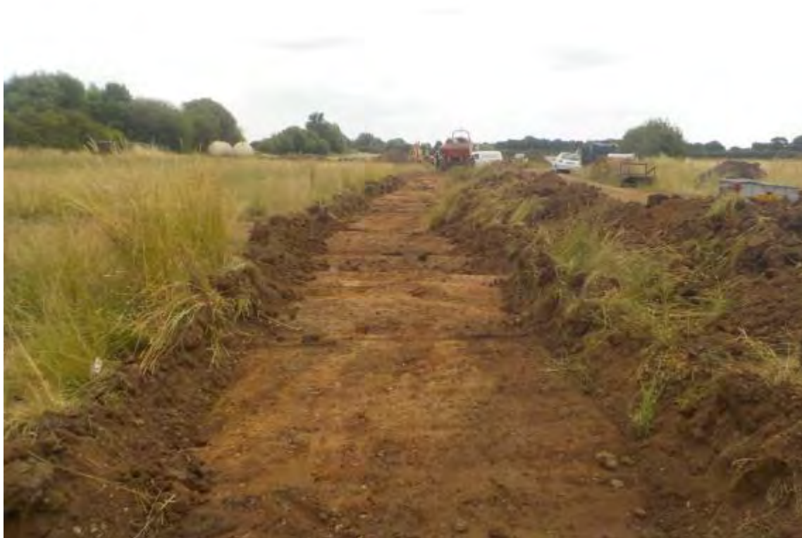
Figure 4. Stripped area, working shot area 1
