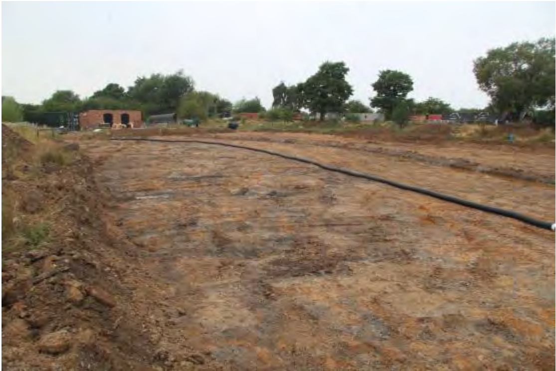
Figure 10. Stripped area 2, view to west.
