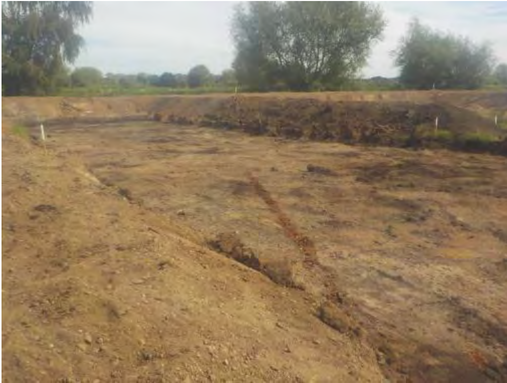
Figure 14. Area 3, view to northeast
