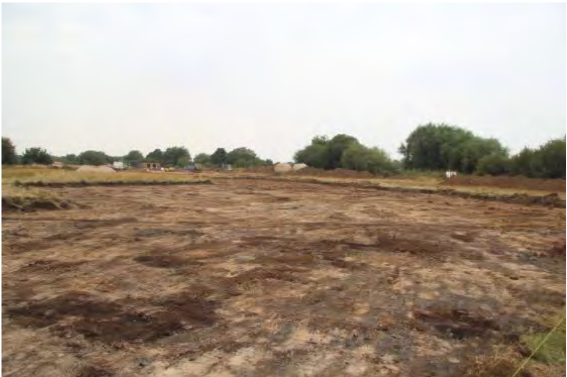
Figure 11. Stripped area 2, view to west
