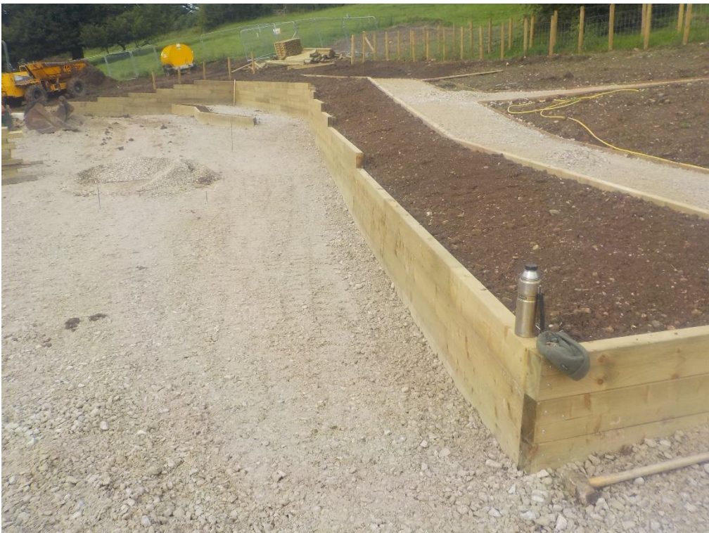
Figure 4: View north-west of the location of unmonitored augur holes.
