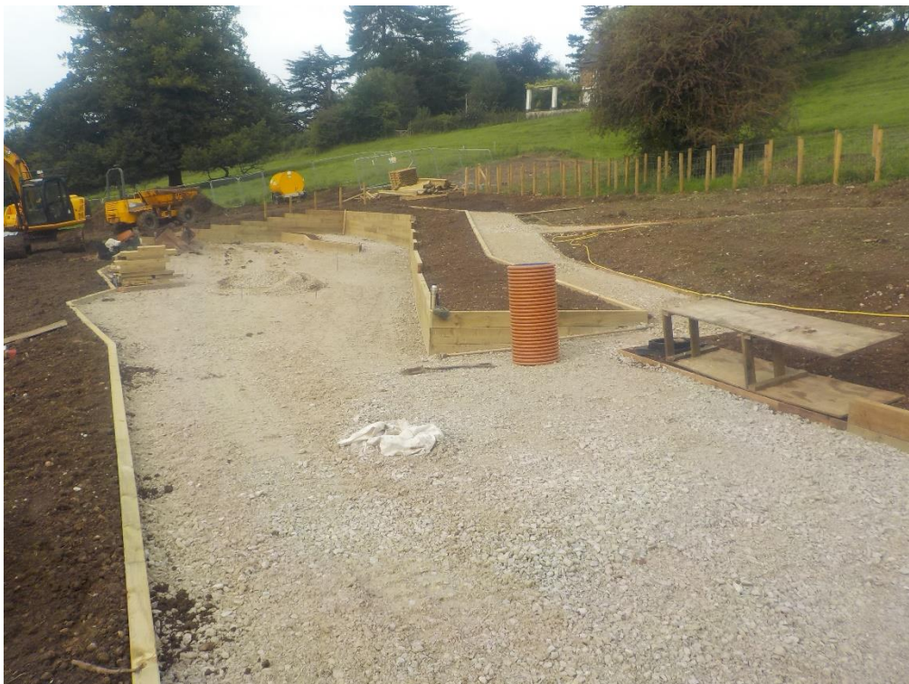
Figure 2: View north-west of constructed paths and retaining walls.
