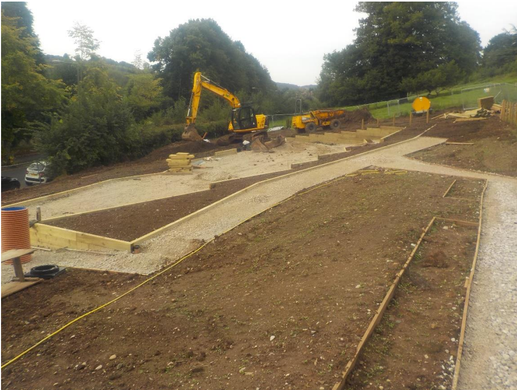
Figure 3: View south-west of constructed paths and retaining walls.
