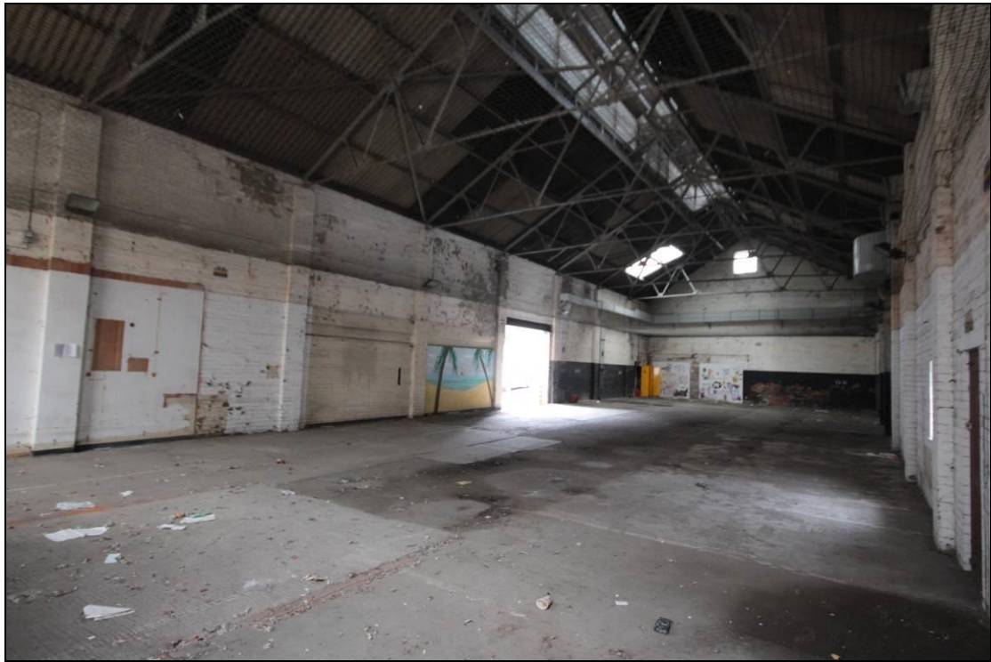
Plate 12: General view of the interior of the building, facing north east.
