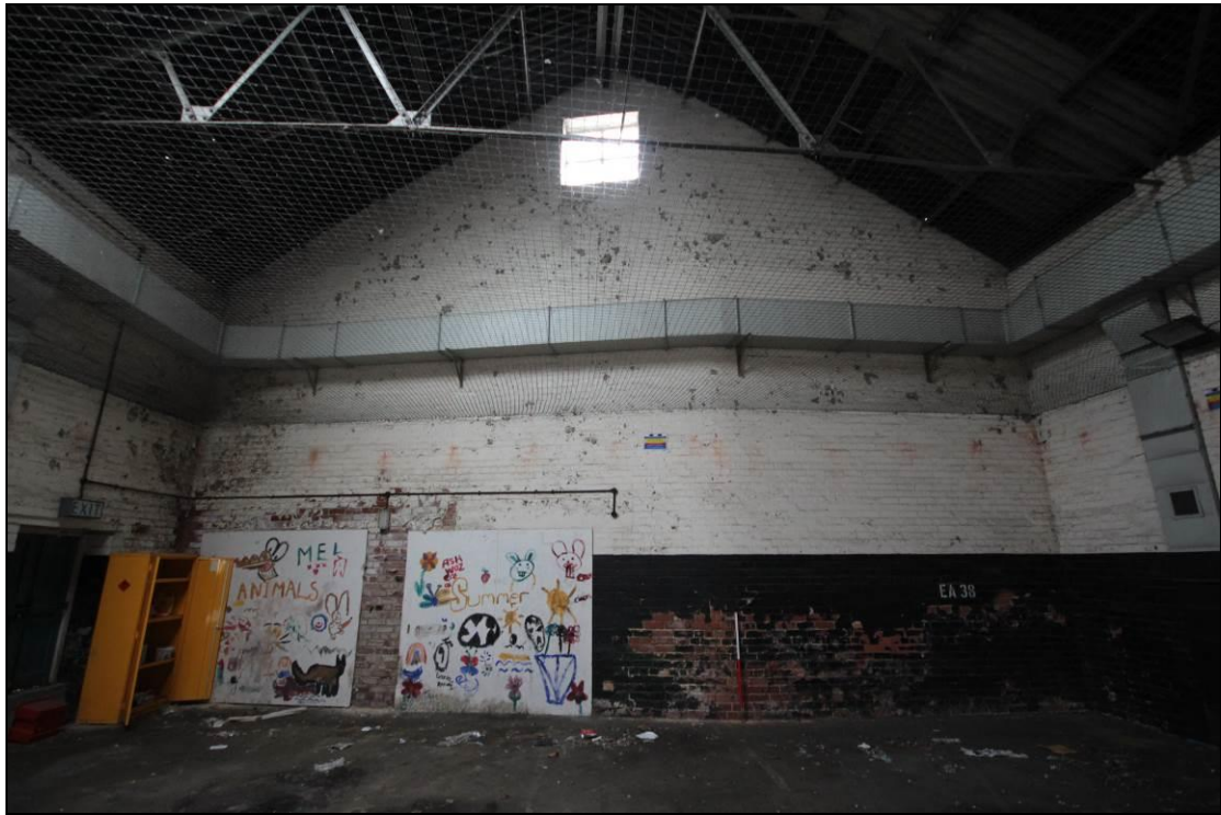
Plate 20: The north eastern wall, facing north east. Scale 1m.
