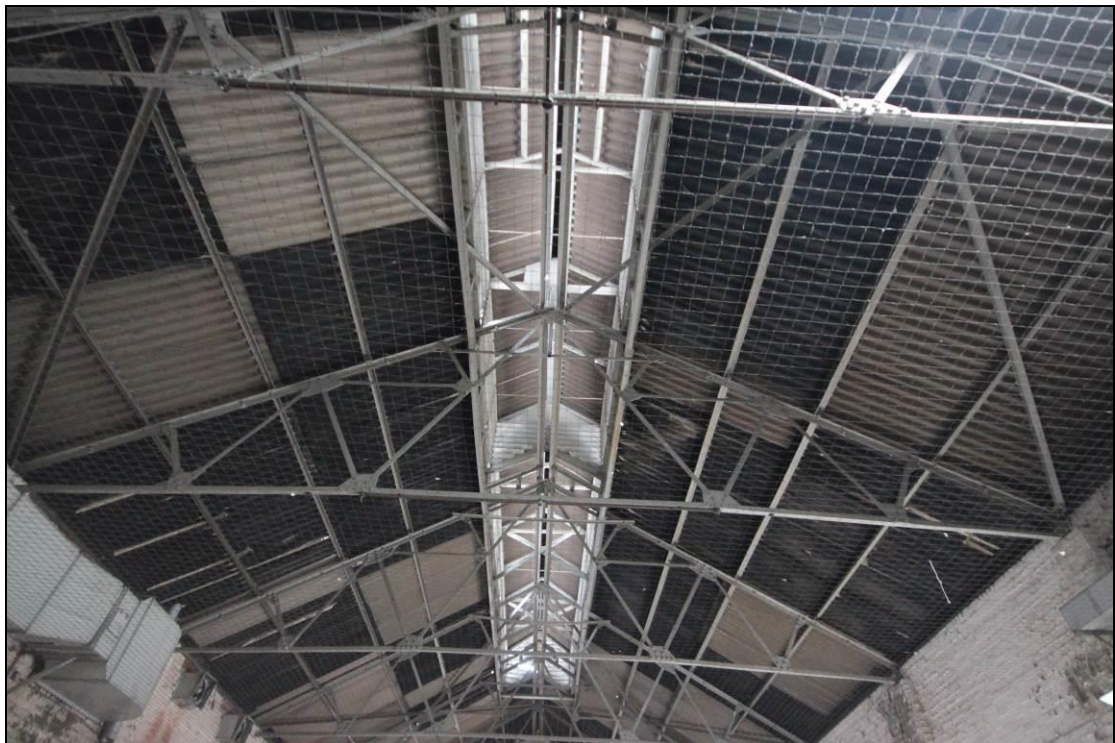
Plate 25: The roof structure of the building, facing south west.
