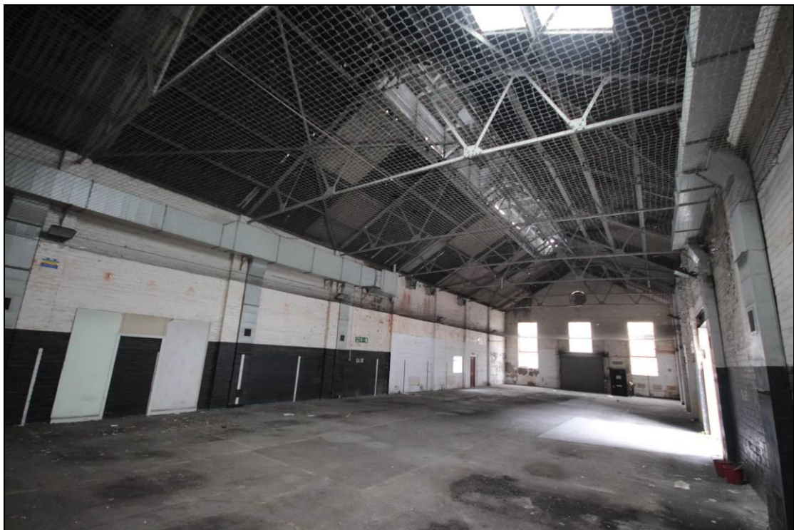
Plate 13: General view of the interior of the building, facing south west.
