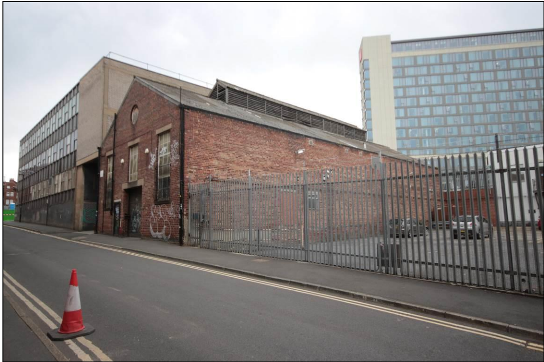
Plate 1: View of the building from the south west, facing north east. Scale 1m.
