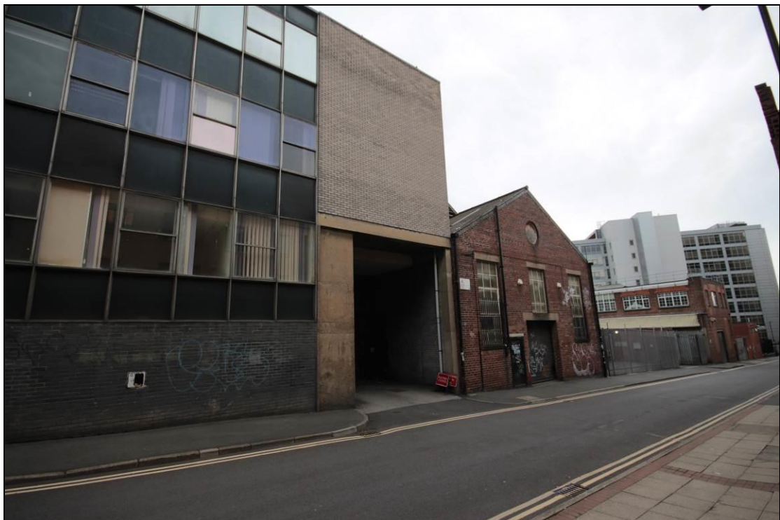
Plate 2: View of the building from the north west, facing south east. Scale 1m.
