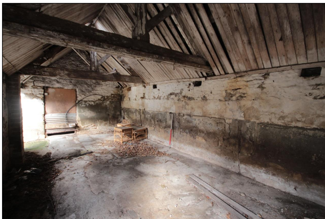
Plate 85: Oblique view of north-east building's interior, with 1m scale.
