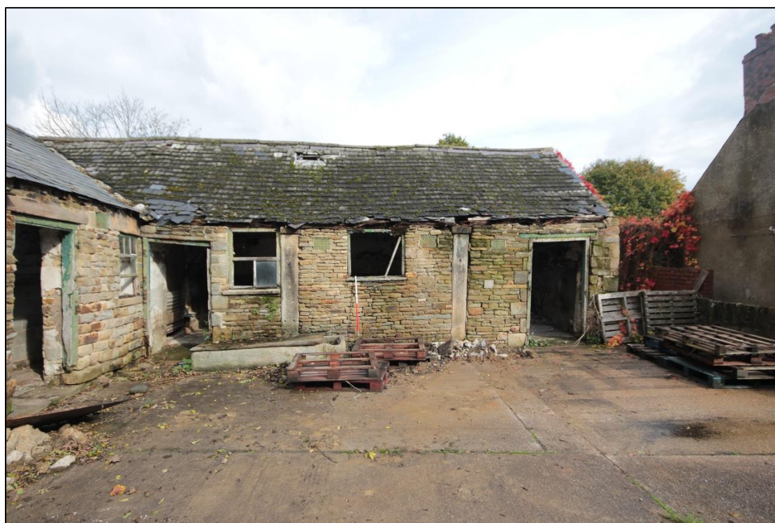
Plate 78: The internal west elevation of the farmyard complex of buildings, featuring plinths from previous shelter shed, with 1m scale.
