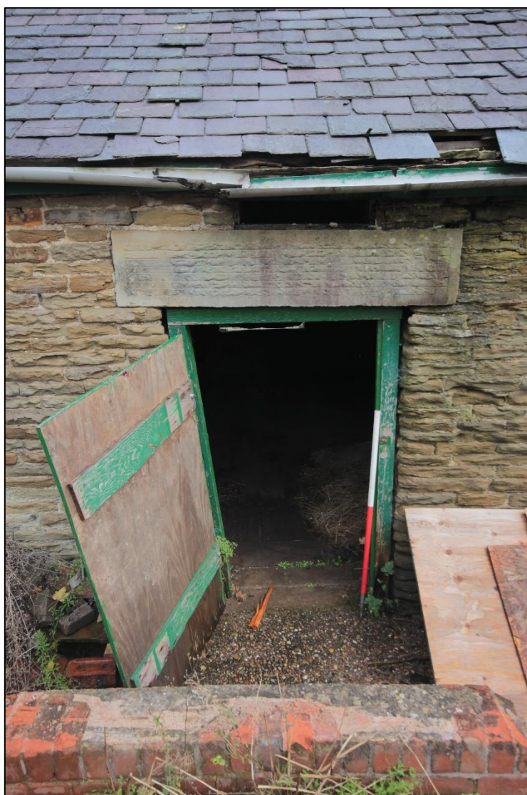
Plate 63: Doorway on the western elevation, taken facing east with 1m scale.
