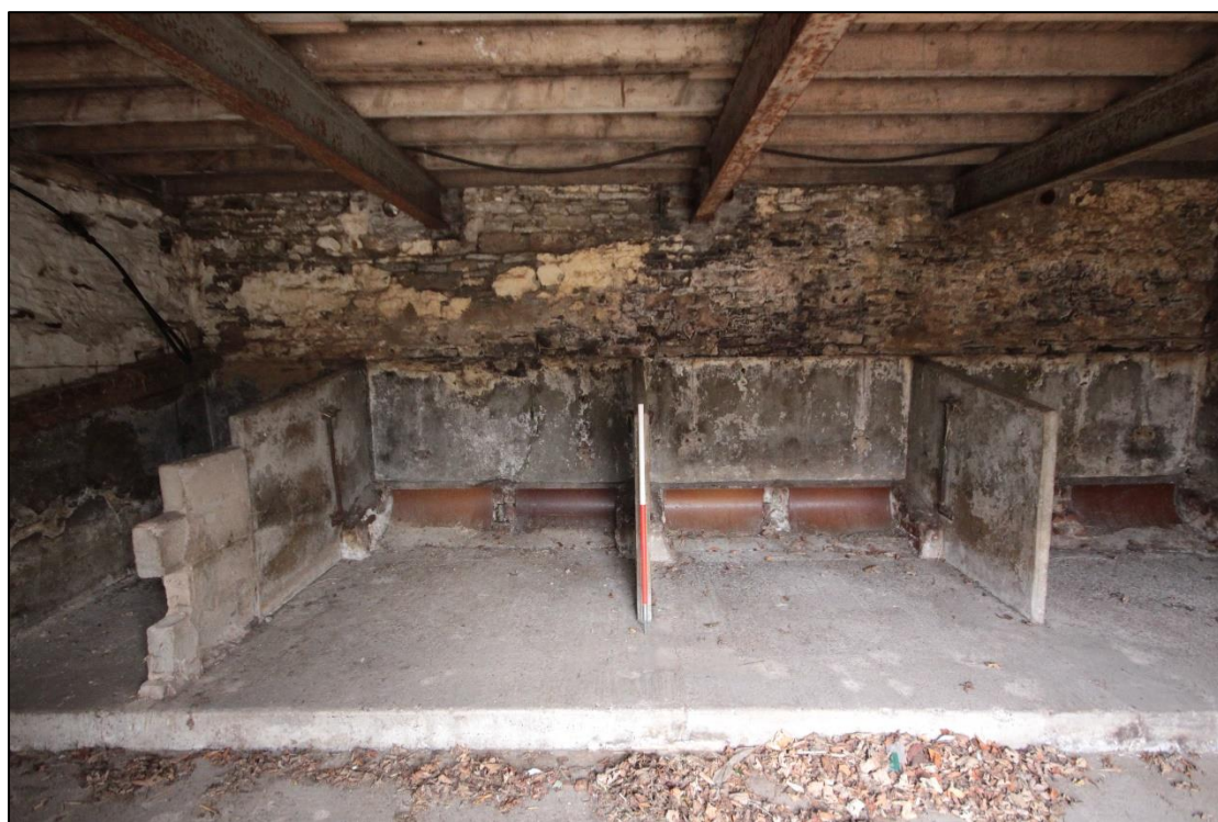
Plate 114: View of the concrete partitions with ceramic trough, with 1m scale.
