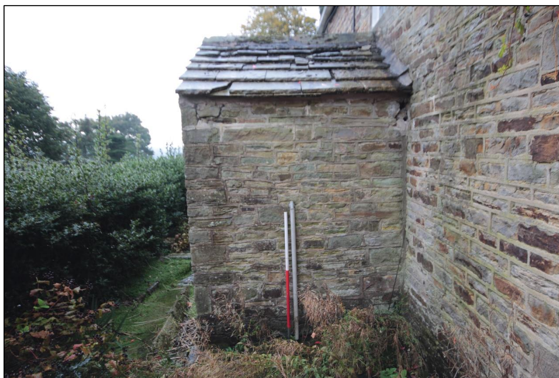
Plate 19: View of the porch facing south-east, with 1m scale.
