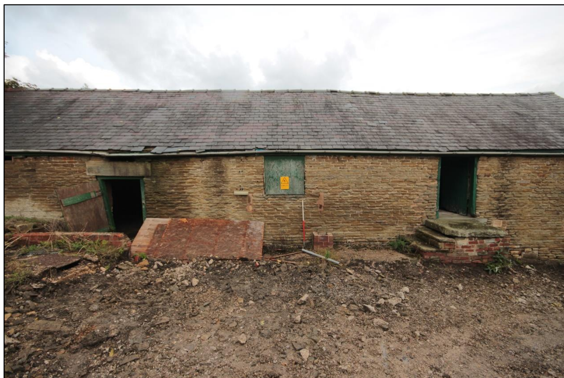
Plate 60: Central view of western elevation, with 1m scale.
