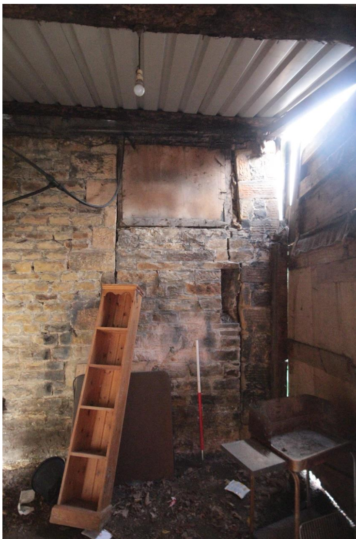
Plate 120: Blocked pitching hole within the end western extension, featuring quoins on the left where the building was connected, with 1m scale.
