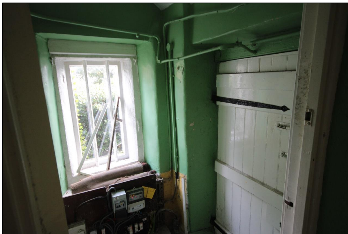
Plate 39: View of the front porch, facing east.
