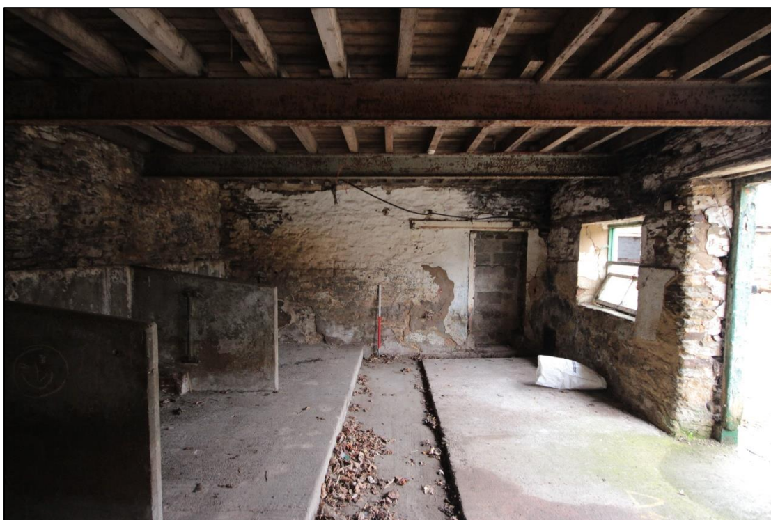
Plate 112: South-east view of central cow house within western wing. Featuring central drainage channel and moulded concrete partitions, with 1m scale.
