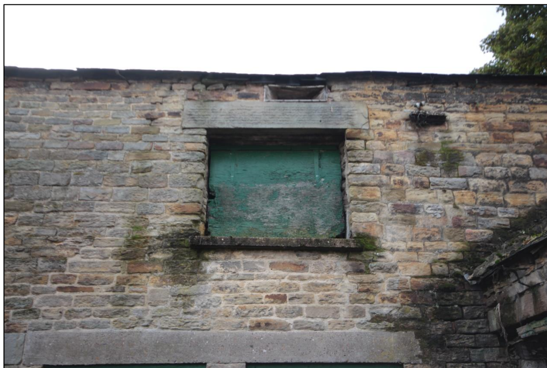
Plate 73: Pitching hole with lintel and sill on the internal eastern elevation.
