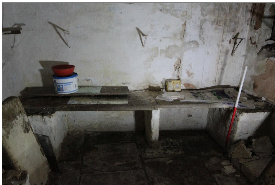
Plate 27: The southern wall of the utility room, with 1m scale.
