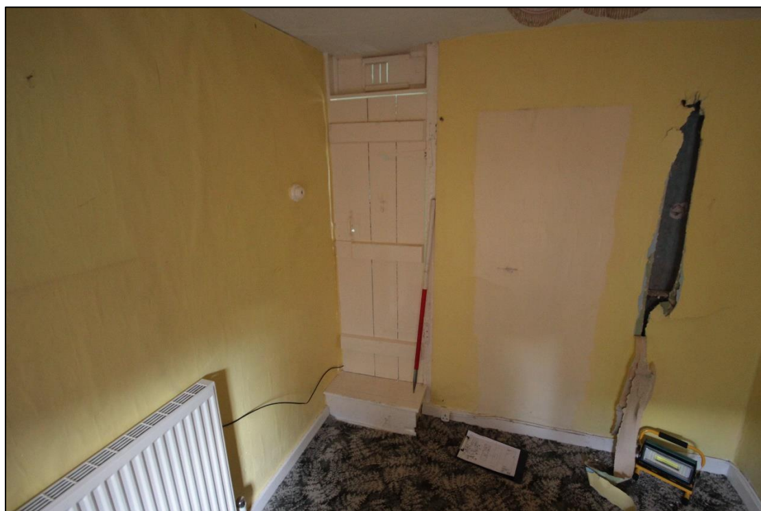
Plate 52: The narrow bedroom door of the small bedroom, with 1m scale.
