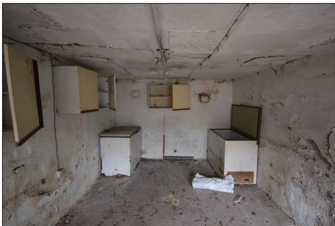
Plate 109: Plain utility room within western wing, with 1m scale.
