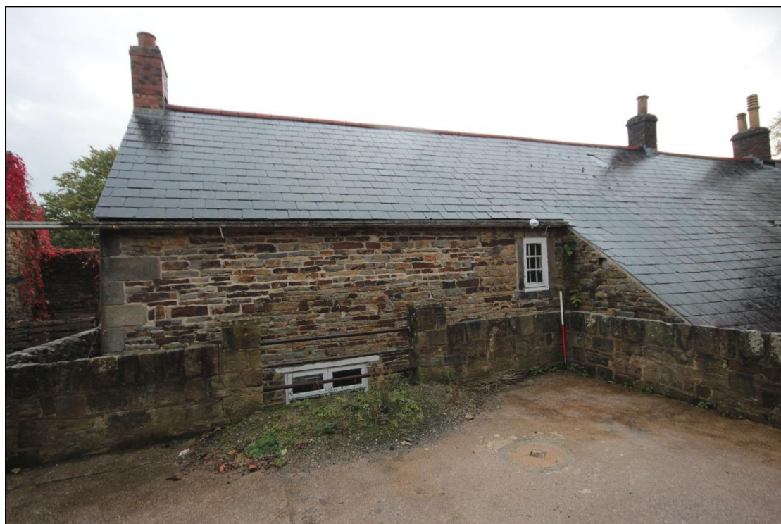
Plate 11: View of the northern extent of the western elevation of the farmhouse. Taken facing east, with 1m scale.
