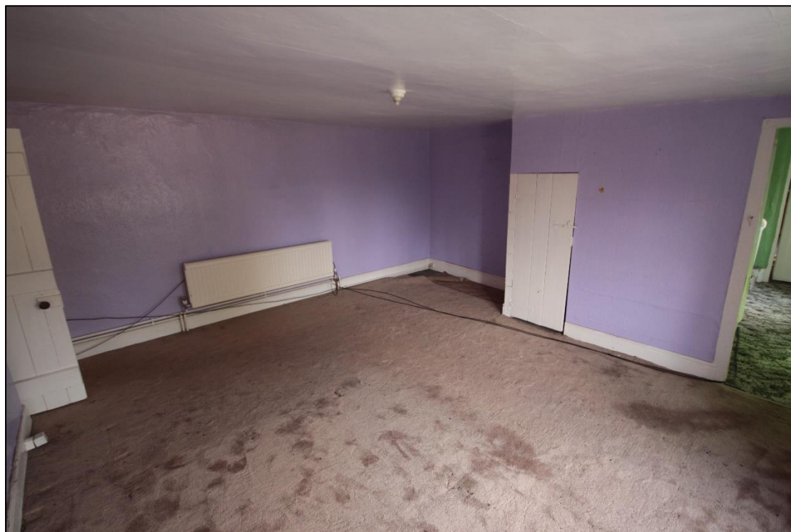
Plate 44: View of the central first floor bedroom, taken facing north-west.
