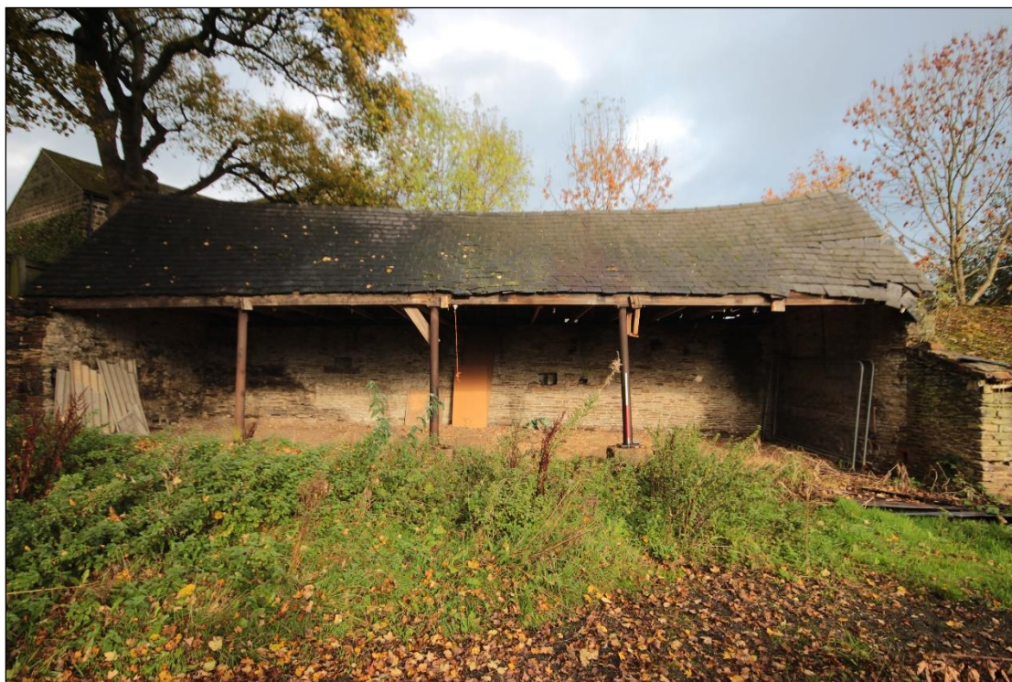
Plate 129: North facing view of the shelter shed, with 1m scale.
