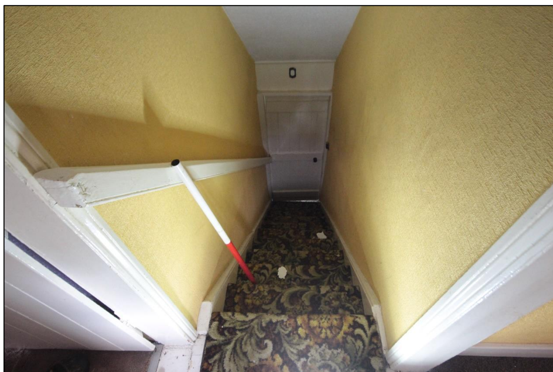
Plate 48: View of the southern staircase, with 1m scale taken facing east.
