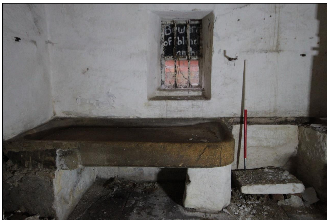
Plate 25: View of the northern wall of the utility room, featuring historic sink, with 1m scale.
