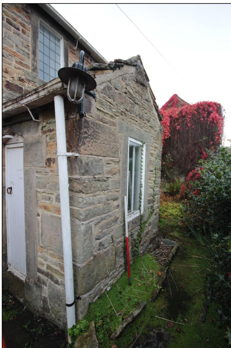
Plate 18: Oblique view of the front porch with 1m scale, facing west.
