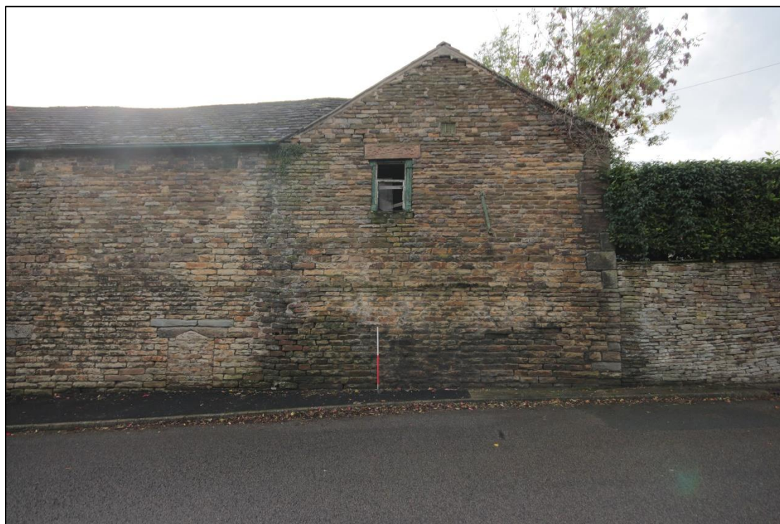
Plate 81: View of the east elevation of the farmyard buildings from the road, taken facing west with 1m scale.
