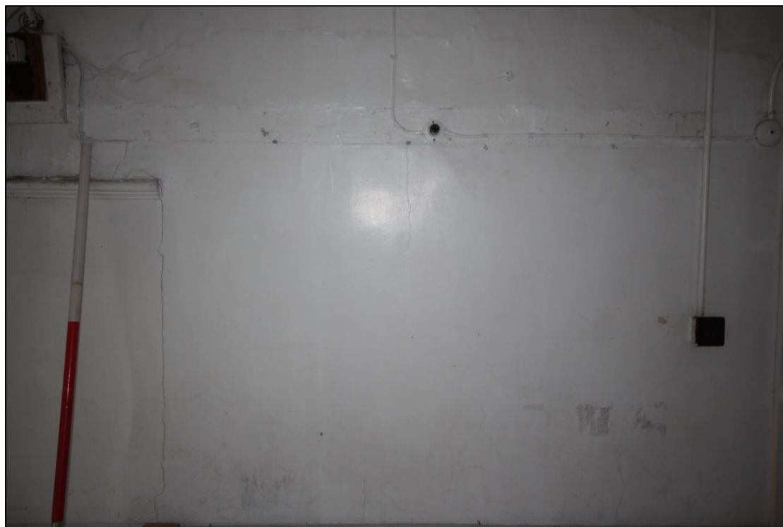
Plate 32: Blocked doorway in the utility room, facing south with 1m scale.
