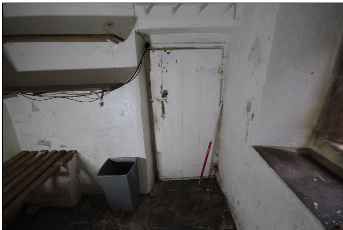
Plate 35: Door on the south wall of the pantry, with 1m scale.
