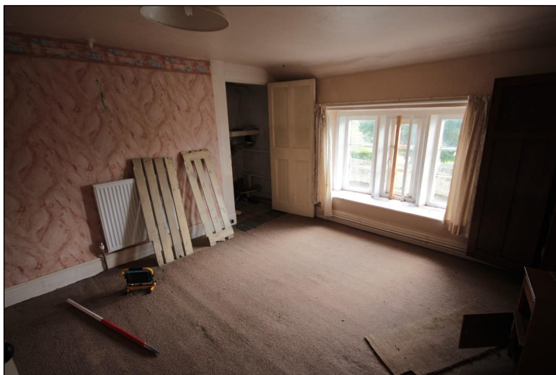
Plate 46: First floor bedroom to the south of the farmhouse, taken facing north.
