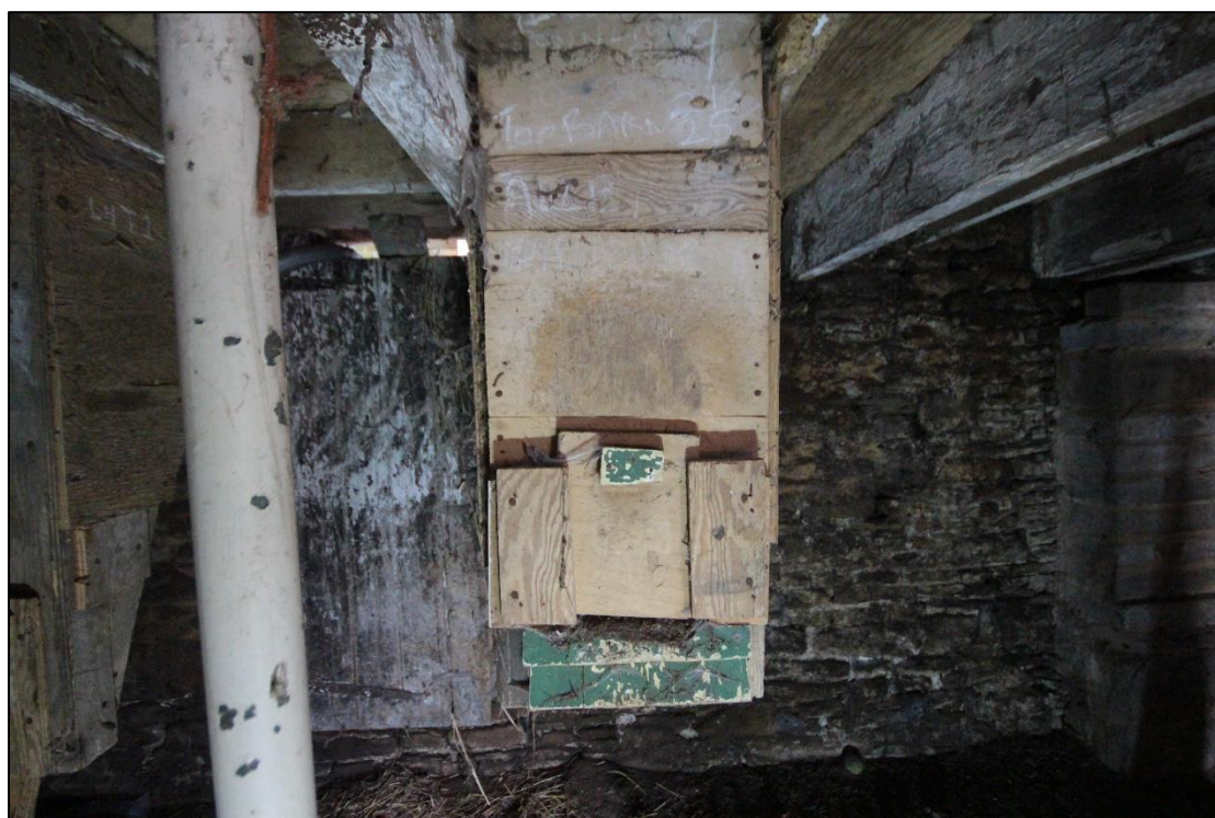
Plate 106: Close view of the timber constructed grain chute.
