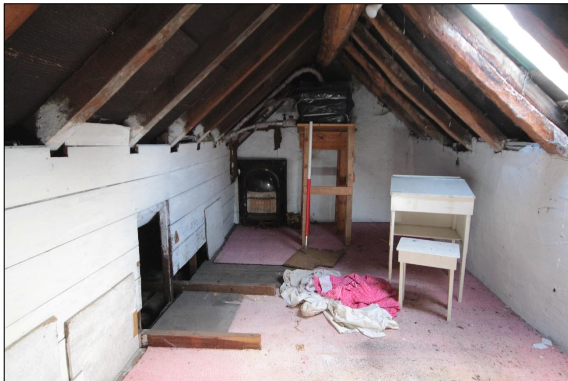
Plate 56: Attic space in the farmhouse, taken facing north with 1m scale.
