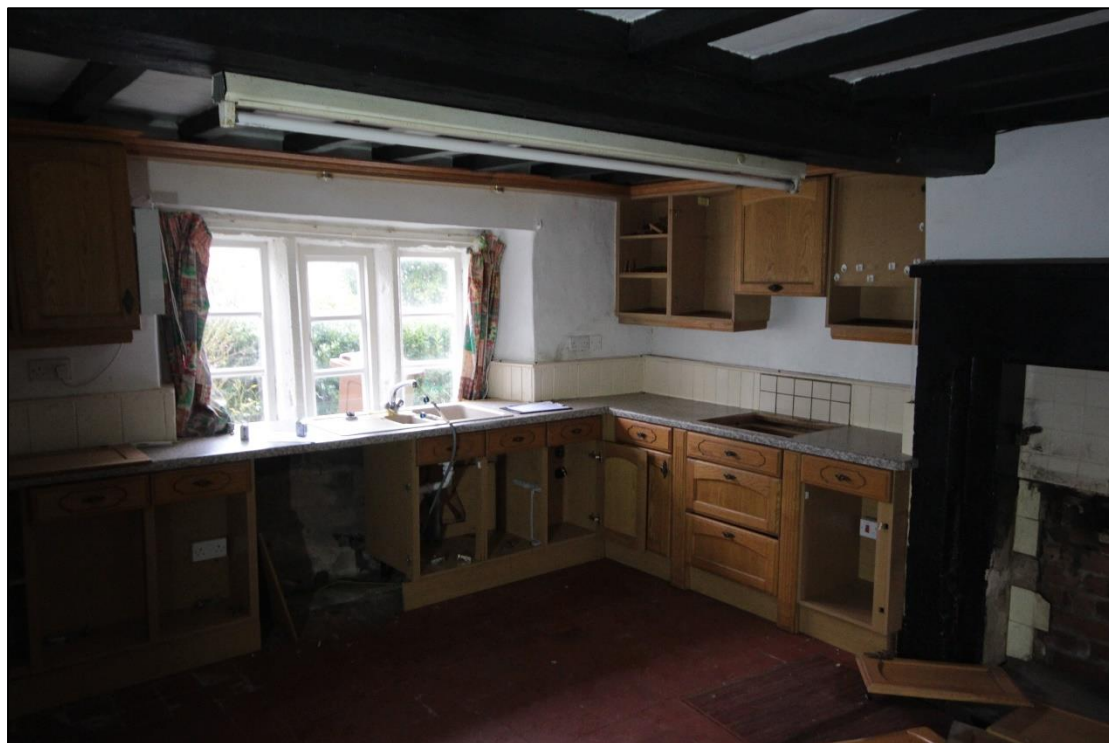
Plate 23: View of the kitchen to the south-east.
