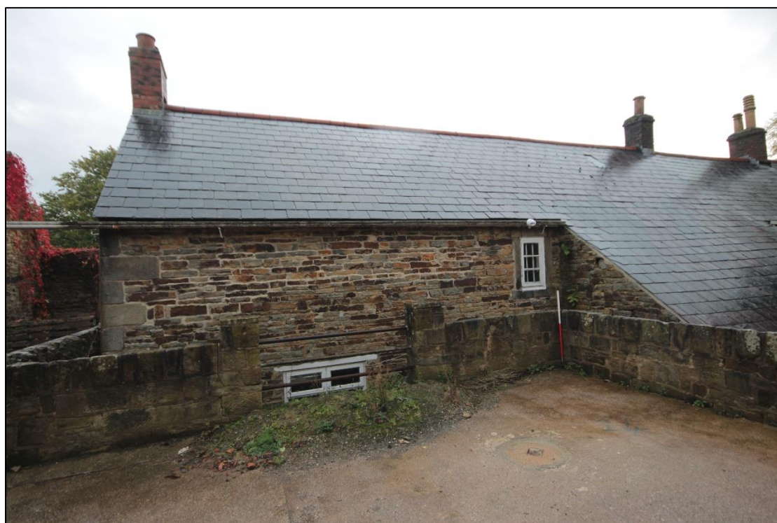
Plate 4: View of the northern extent of the western elevation of the farmhouse. Taken facing east, with 1m scale.
