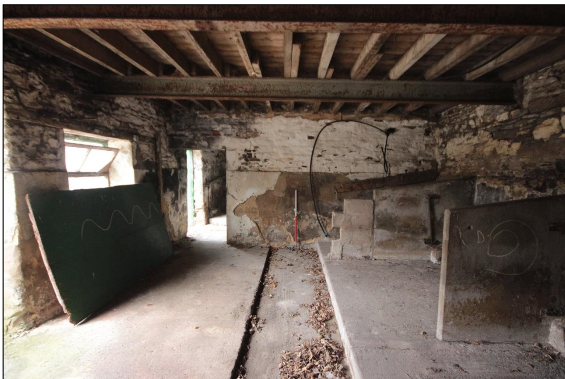
Plate 113: View of the south-east wall within the central cow house of the western wing.
