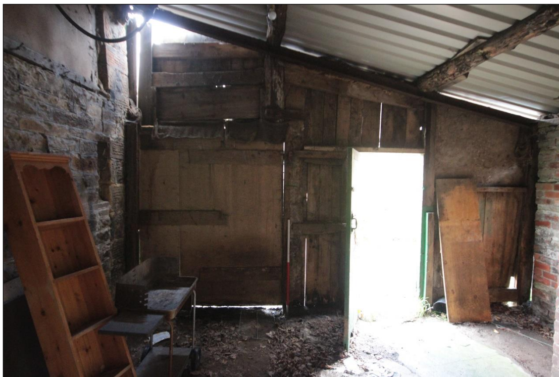
Plate 121: Timber walling on the end extension of the western wing, with 1m scale.
