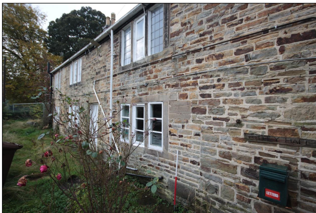
Plate 16: View of the eastern exterior of the farmhouse. Facing north, 1m scale.
