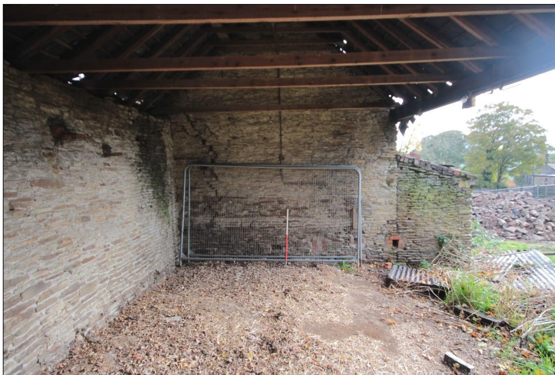
Plate 130: Eastern interior wall of the shelter shed, with 1m scale.
