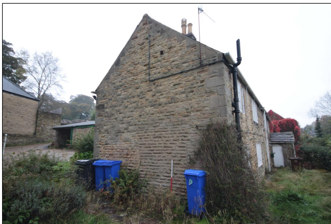
Plate 5: Southern gable of the farmhouse facing north-west, with 1m scale.
