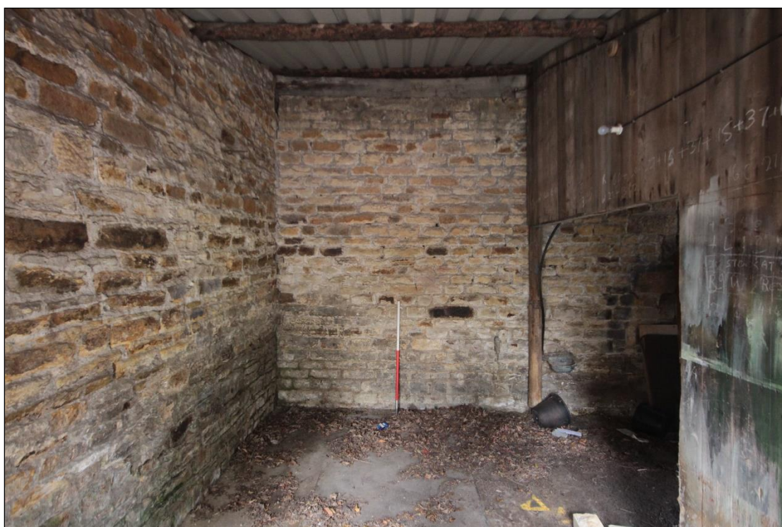
Plate 123: North-west interior wall of the end western extension, with 1m scale.
