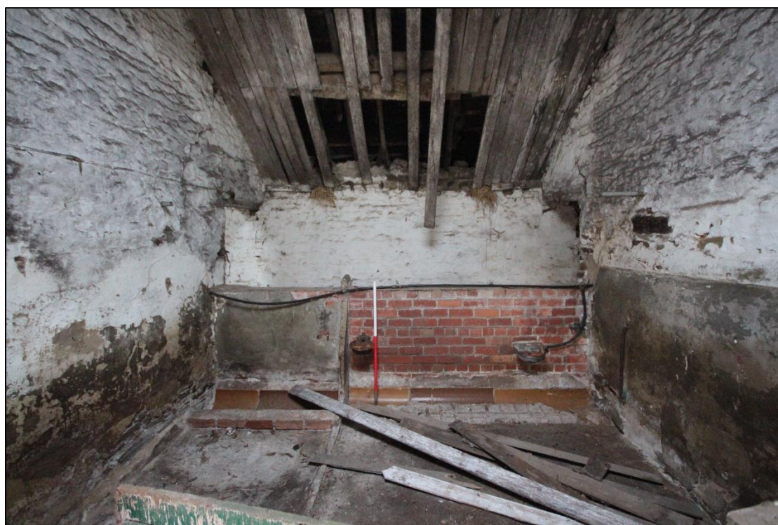
Plate 93: Small area with low brick wall, ceramic trough within the northern wing, with 1m scale.
