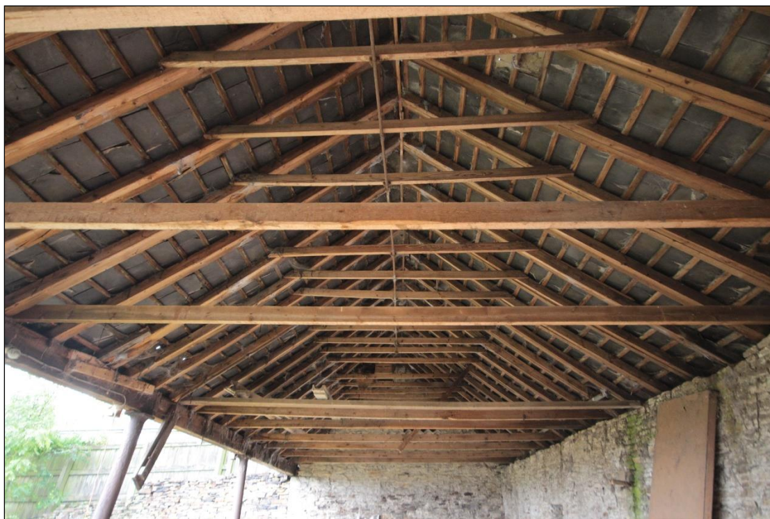
Plate 135: Timber framed roof of the shelter shed, taken facing west.
