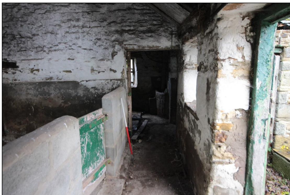
Plate 95: Corridor to the north-east room within the northern exterior, with low concrete moulded wall to the left. 1m scale.
