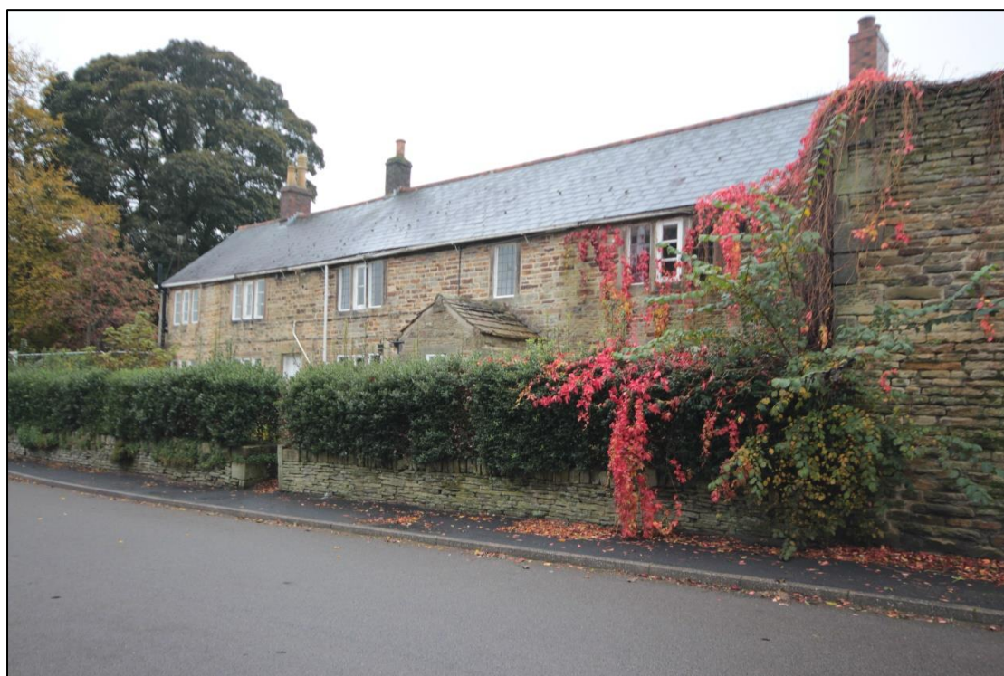
Plate 2: The eastern façade of Totley Hall Farmhouse, taken from the north-east.
