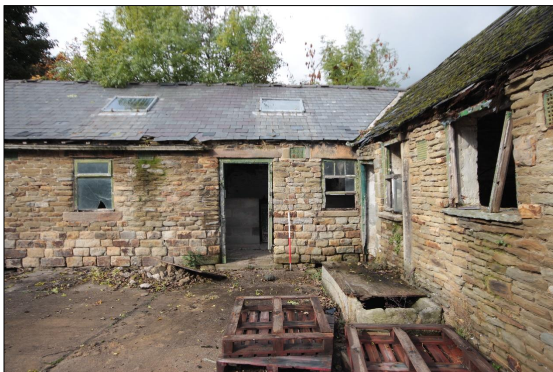
Plate 77: Eastern end of the internal south elevation, with 1m scale.
