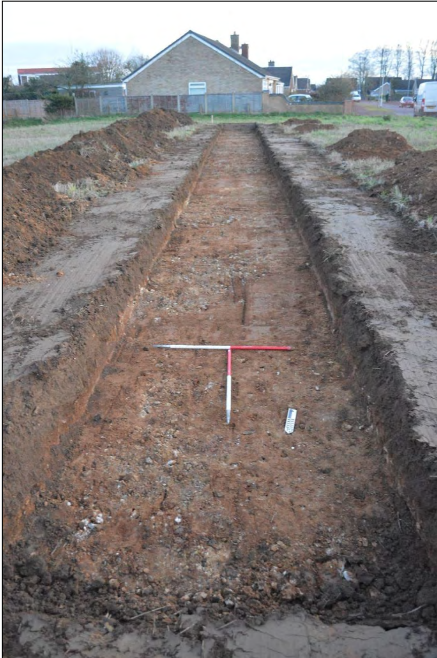
Figure 90: View of Trench 16 looking South-east (Scale = 1 x 1m in 0.5m graduations).
