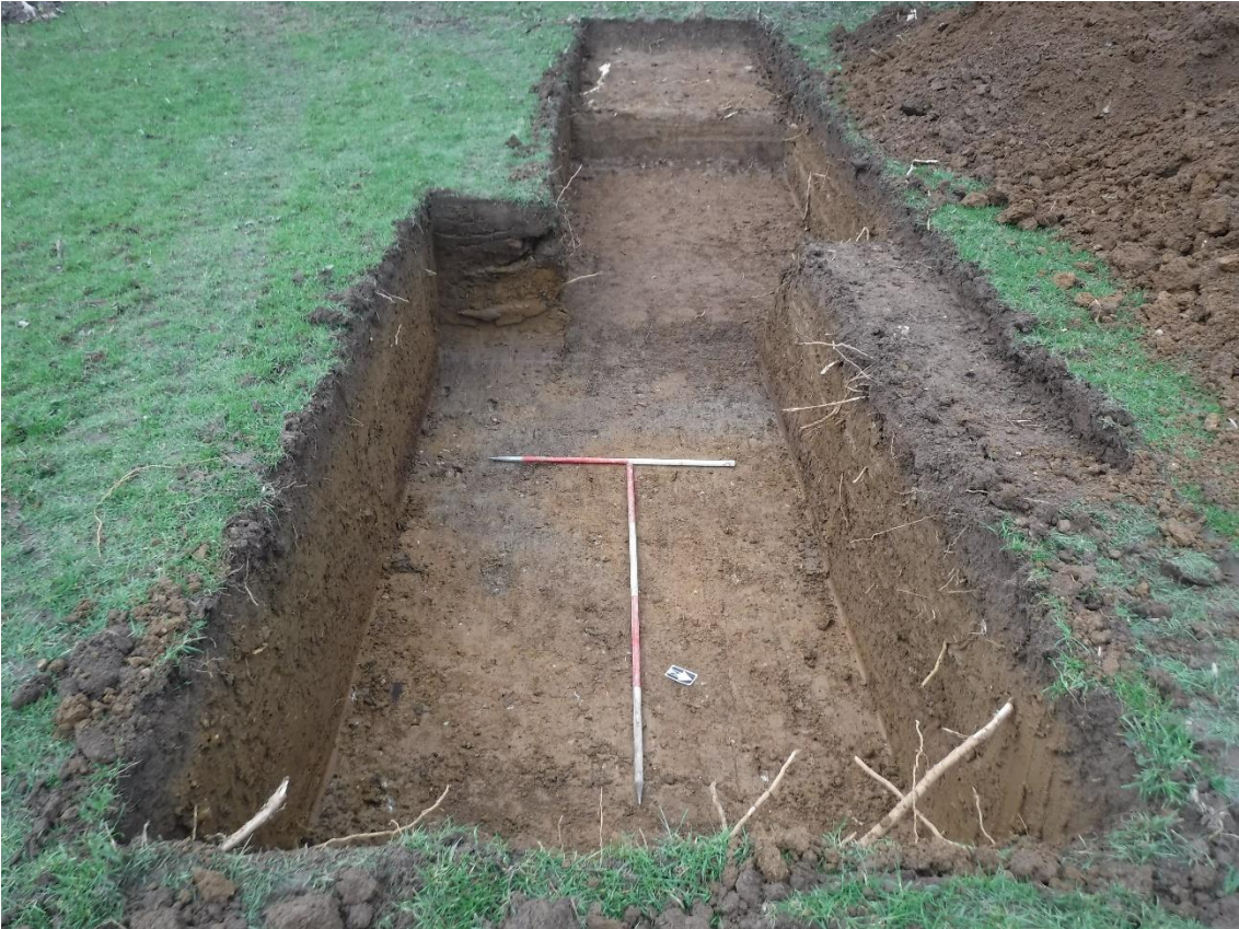
Figure 3. Shot of Trench 1 facing south west
