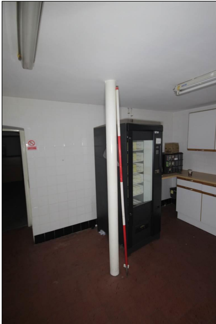
Plate 36: View of one of the cast iron columns within room B9, taken with 2m scale facing south
