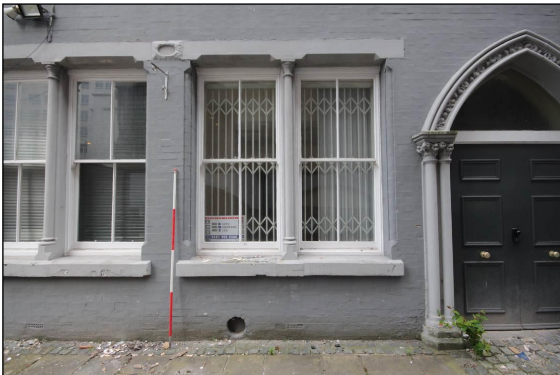
Plate 14: Example of the four-light sash windows with connected sills and chamfered lintels, taken facing north with 2m scale
