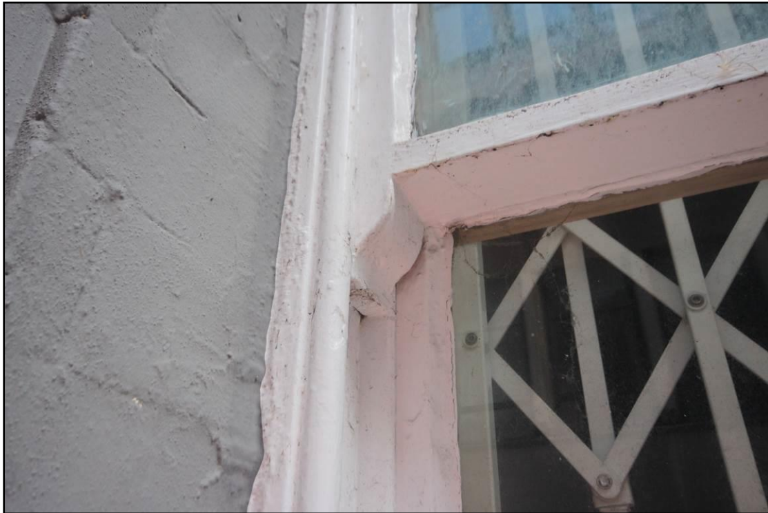
Plate 18: Example of the curved horns seen on the original sash windows of the building
