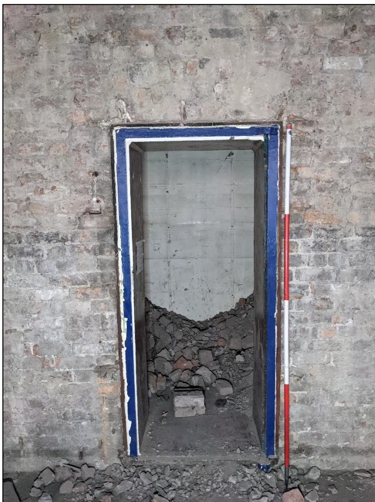
Plate 131: The heavy-duty door frame with segmental arch above within the vault of room SF6, taken with 2m scale facing north
