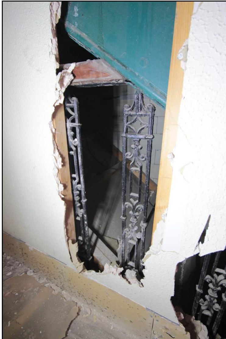
Plate 107: The original central staircase with metal balustrade and timber handrail on the first floor, taken facing north-east
