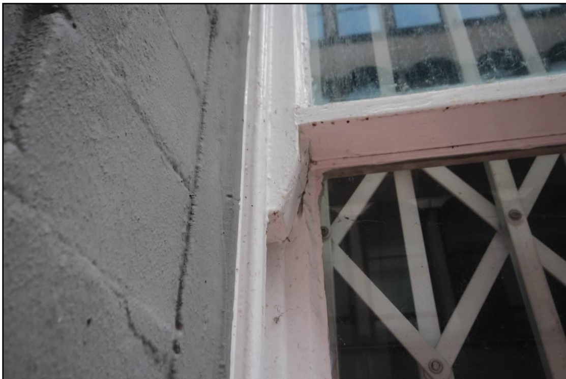
Plate 19: View of the straight horns seen on the narrower sash window, indicating it was likely a later installation
