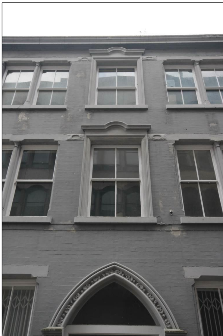
Plate 13: The larger four-light central windows set within decorative architraves on the southern elevation, taken facing north
