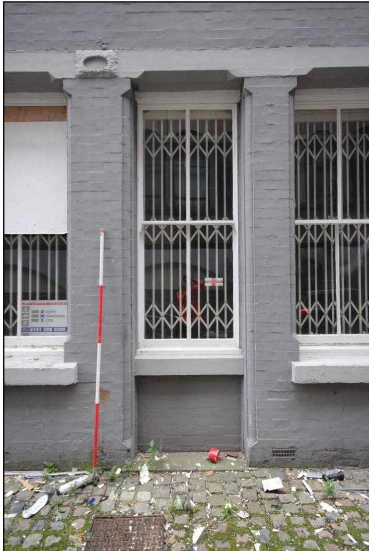
Plate 17: The narrower four-light window, which may have originally been a doorway on the southern elevation, taken with 2m scale facing north
