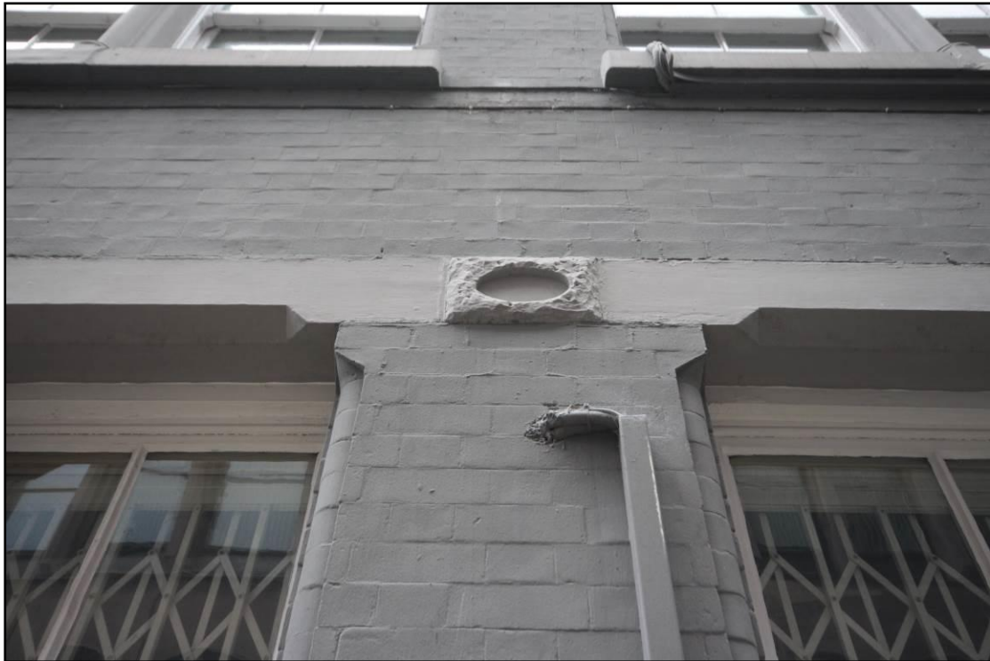
Plate 15: View of one of the rough-tooled stones with oval boss, demarcating the separate rows of sash windows on the southern elevation, taken facing north
