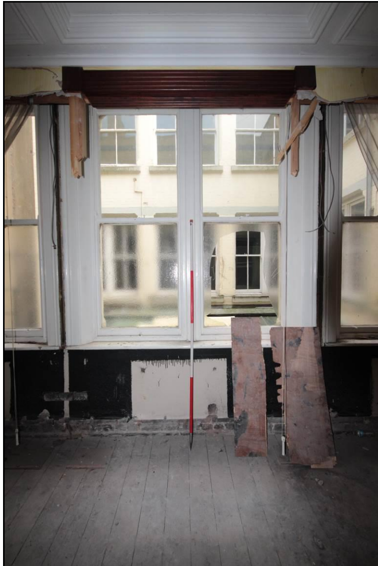
Plate 90: View of the windows with obscure glazing and timber panelling above on the eastern wall of room FF4, taken with 2m scale
