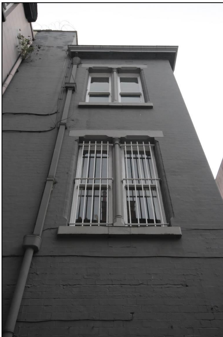
Plate 22: View of the two-light sash windows on the first and second floor of the western elevation, taken facing east
