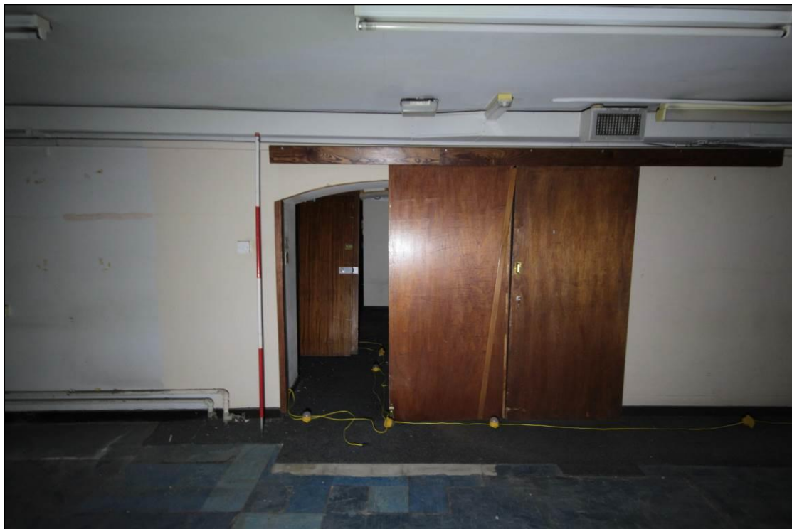
Plate 31: The arched opening with timber sliding door within B6, taken with 2m scale facing north
