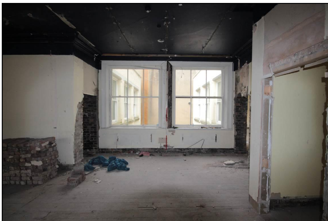
Plate 118: View of the two wide six-light sash windows on the northern wall of room SF2, taken facing north with 2m scale
