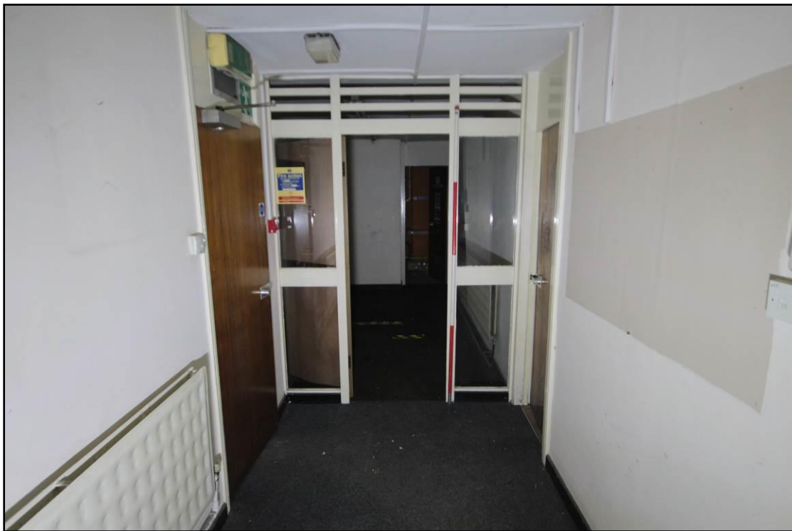
Plate 41: The corridor with timber partition door frame with glazing within the basement, taken facing north with 2m scale
