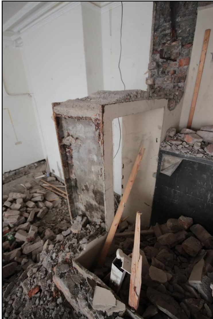
Plate 121: View of the surviving heavy duty metal doorframe of the former vault within room SF3, taken facing south-west
