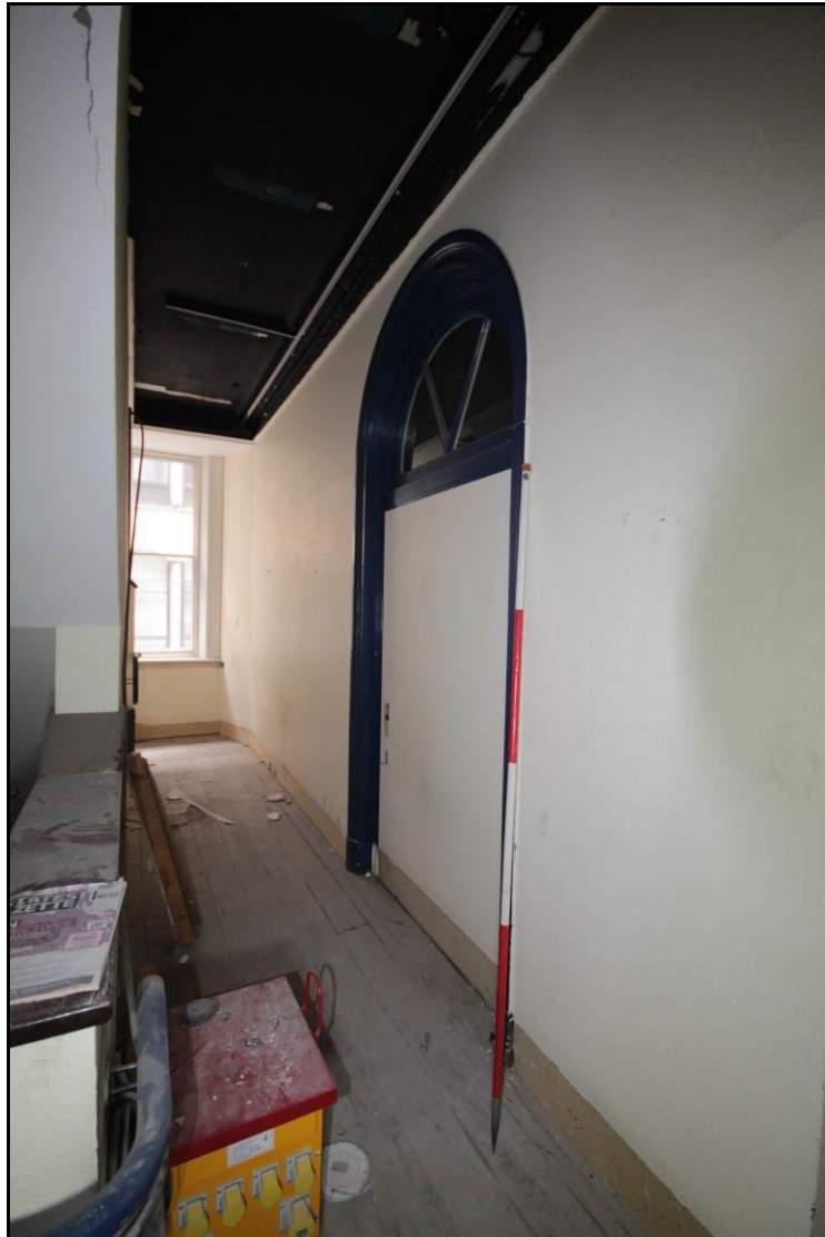
Plate 79: View of the arch with fanlight now blocked connecting the central staircase to FF1, taken with 2m scale facing south
