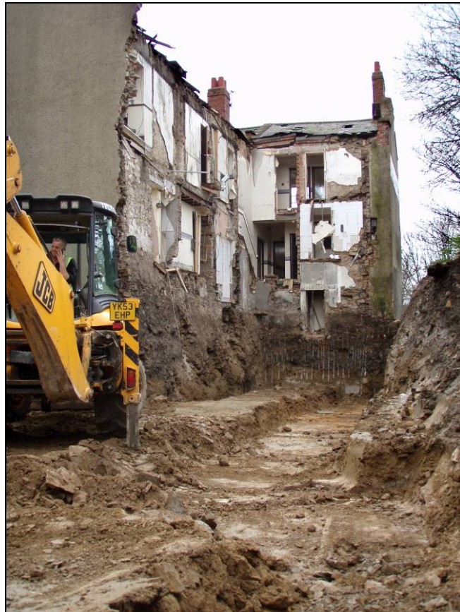
Fig. 5 Rear of the Balmoral hotel showing demolition and depth of excavation.
