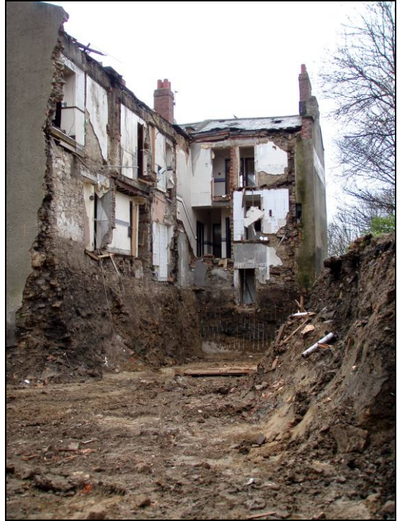
Rear view of the Balmoral during demolition
