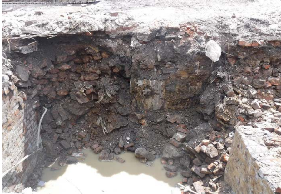
Figure 9: View of corrugated iron shuttering foundation. Facing south-east, no scale.
