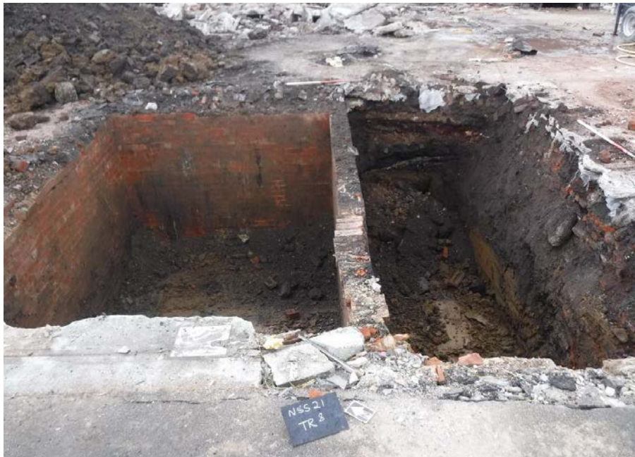
Figure 44: View of Trench 8. Facing north-east, scale 1x1m.
