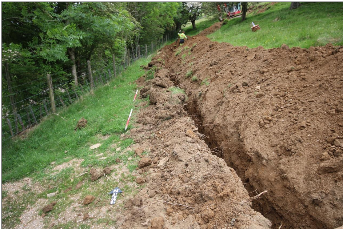
Figure 4: View north of excavated service trench. Scale 2x1m in 0.5m graduations.
