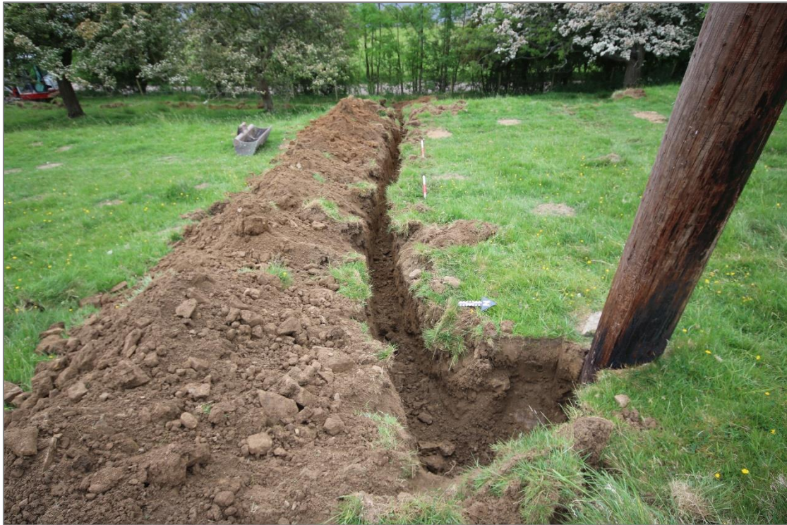
Figure 3: View west of excavated service trench. Scale 2x1m in 0.5m graduations.
