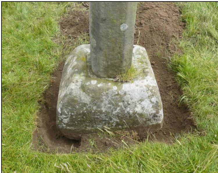
Fig. 4: Excavation around the base to enable lifting. Facing east.
