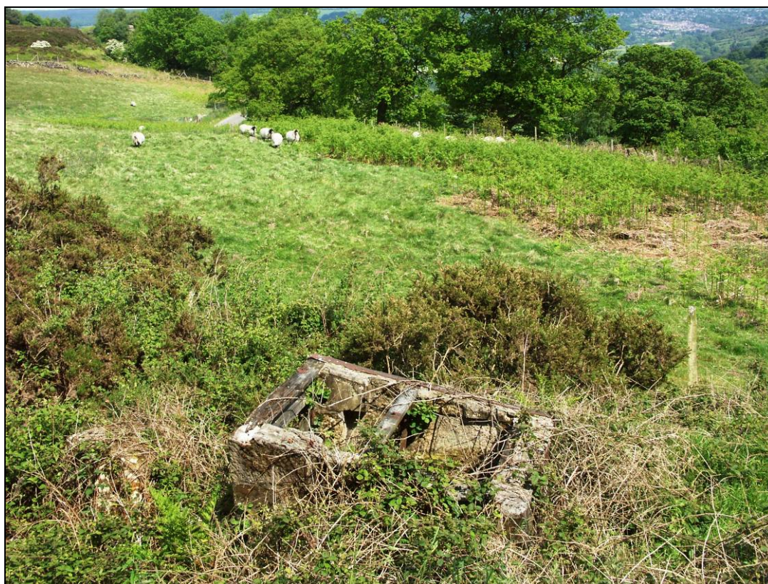
Figure 11: Toilet block beyond the north-east corner of the main building
