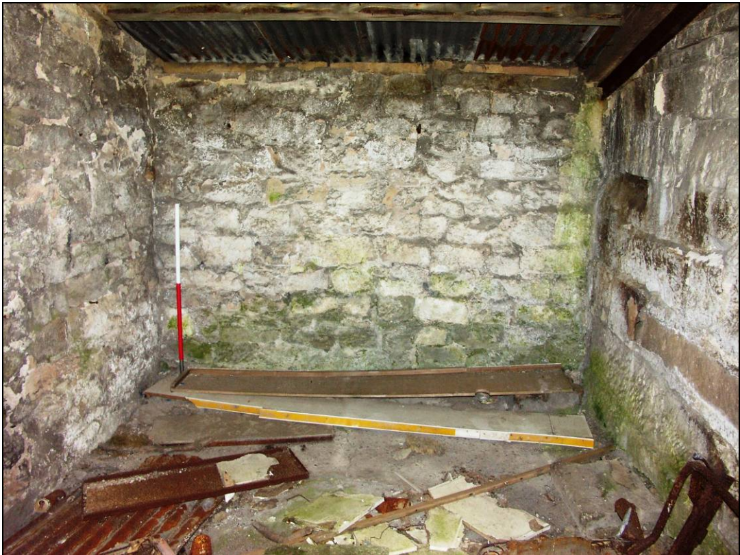
Figure 10: Inside the southern room (looking west)
