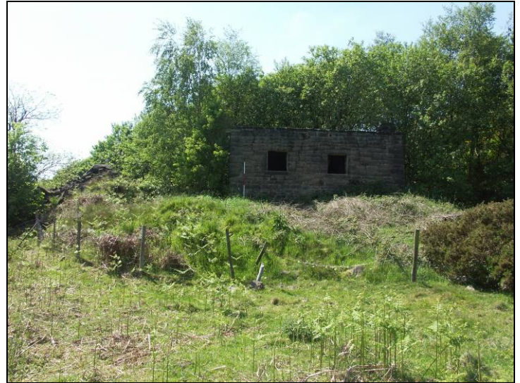
East elevation of redundant shed at Birchover Quarry
