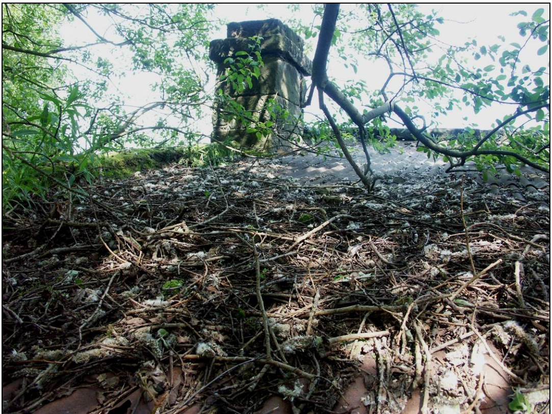
Figure 7: View of the chimney stack and roof (looking north-east)
