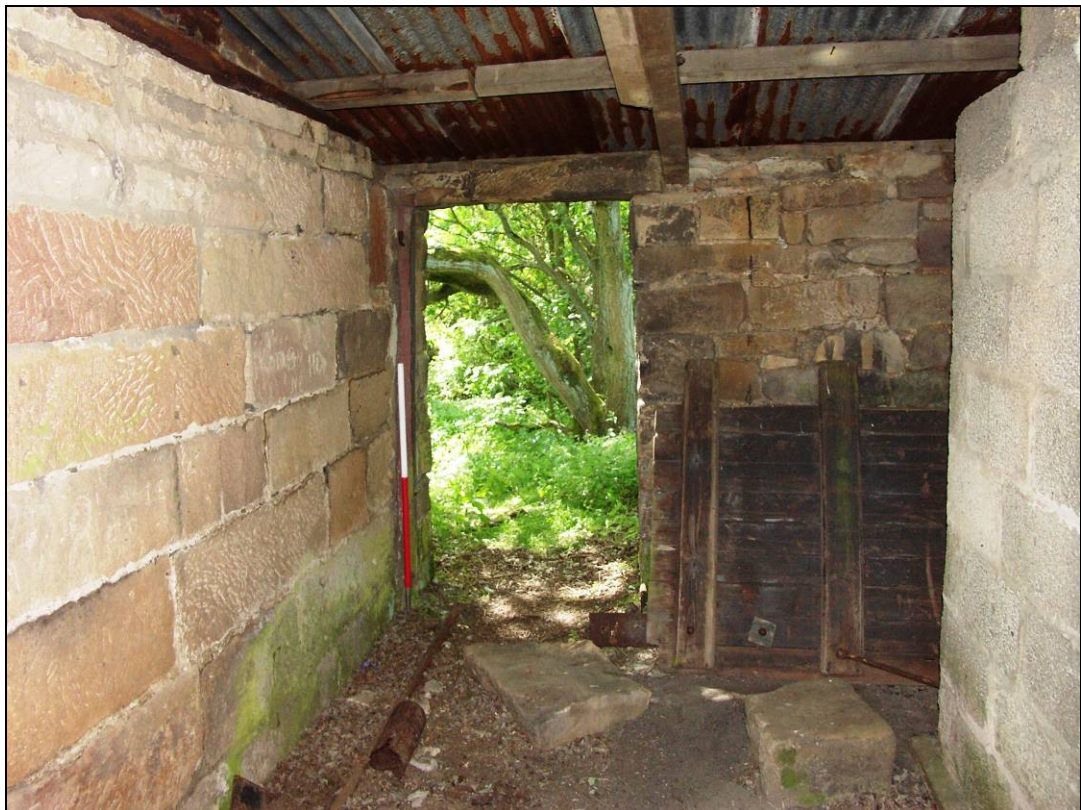
Figure 8: Central hallway (looking west)
