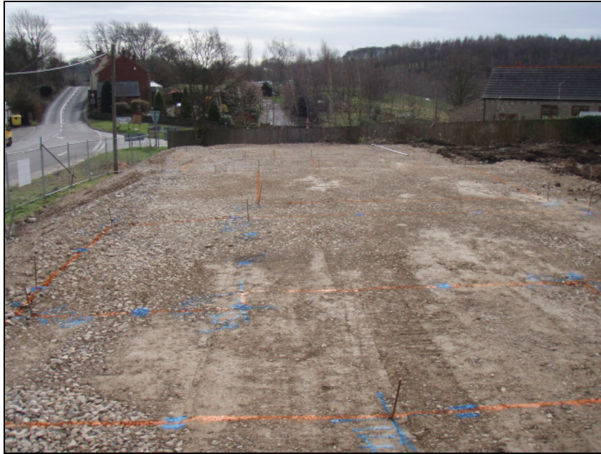
Fig. 7: Area B shown after the bank has been removed and a levelling layer of aggregate deposited ready for construction to begin.
