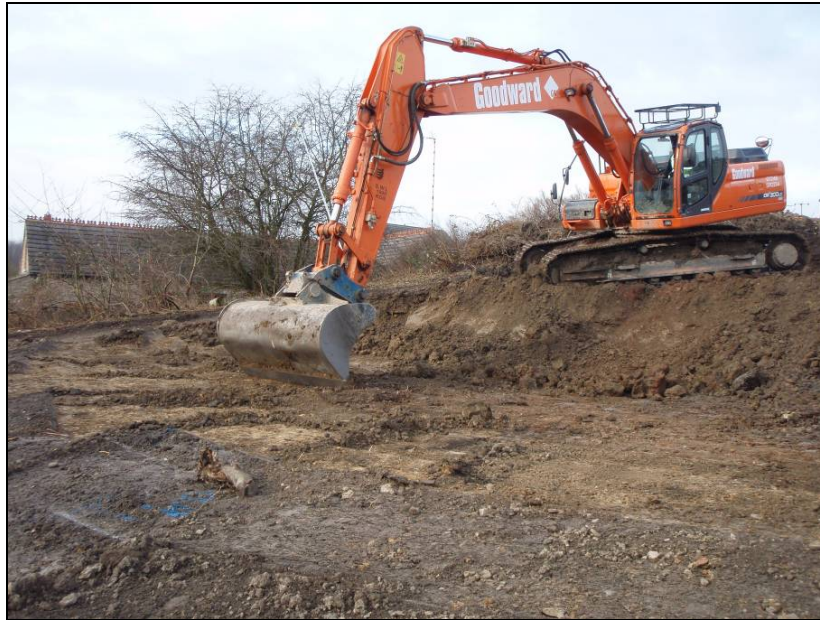
Fig. 4: Working shot of the removal of the soil to form a terrace for Area B.
