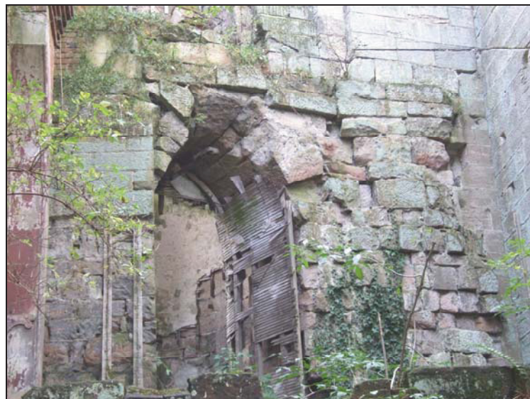
Fig 7 Lower of north elevation showing large central archway
