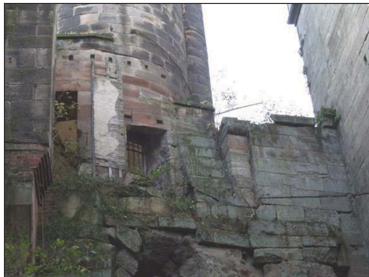
Fig. 9 Central section of north elevation
