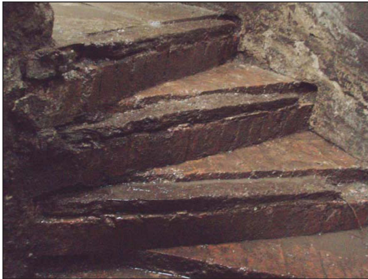
Fig. 21 View of wooden tread plate in situ
