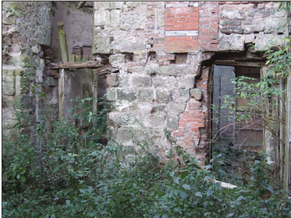
Fig. 4 Lowest storey on east elevation showing doorways to Round Tower on left, mortice holes for original joists and brickwork infilling/repair
