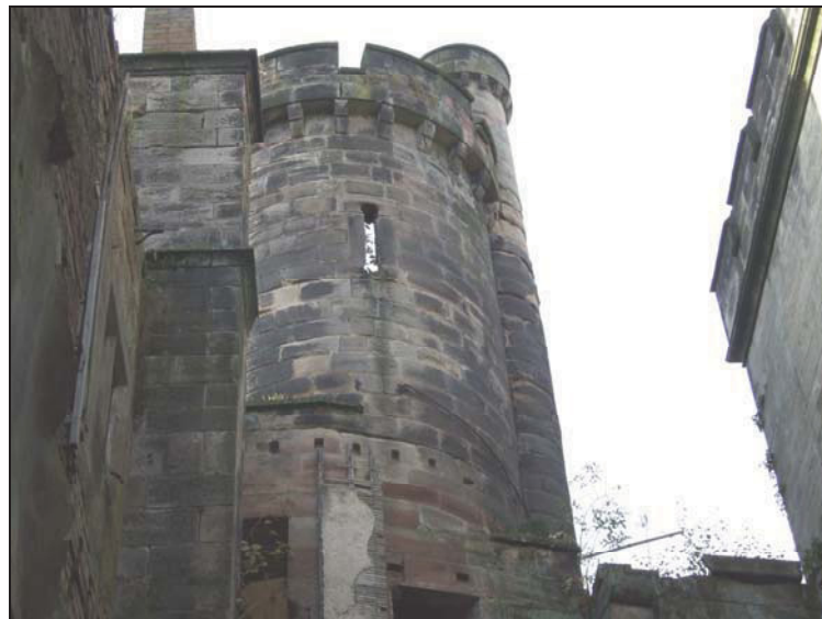
Fig. 10 Upper section of north elevation showing protruding chimney to west
