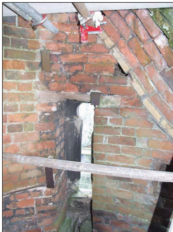
Fig. 14 Interior brick construction with stone cladding visible through the window. The diagonal brick flue can be seen in the top right of shot with a row of heat-retardant bricks at its base.
