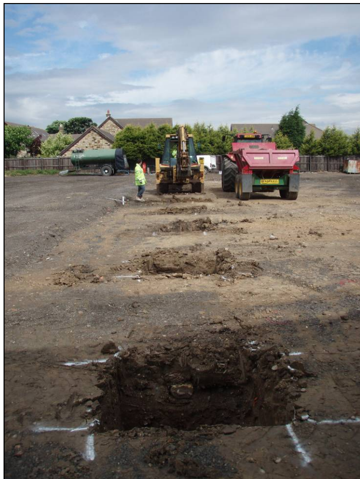
Fig. 7 Row of 1m x 1m foundation pits.
