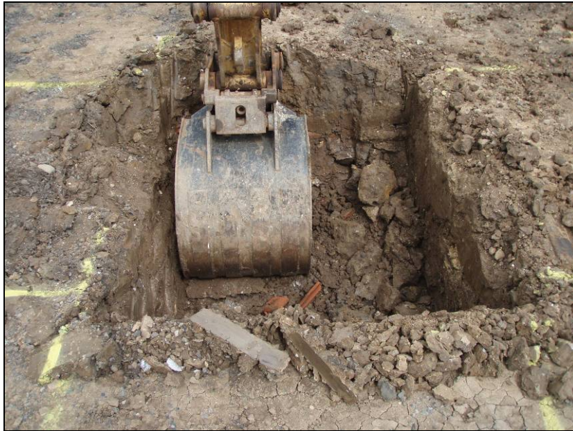
Fig. 6 Excavation of a pit
