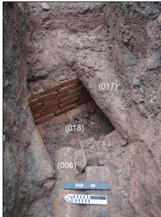
Fig. 10 Photograph of the inside of the culvert (facing east)
