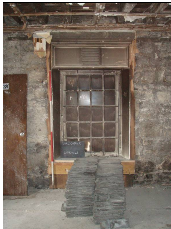
Fig. 11 South elevation ground floor window (internal)
