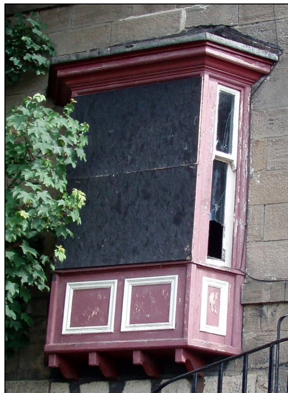
Fig. 9 South elevation bay window
