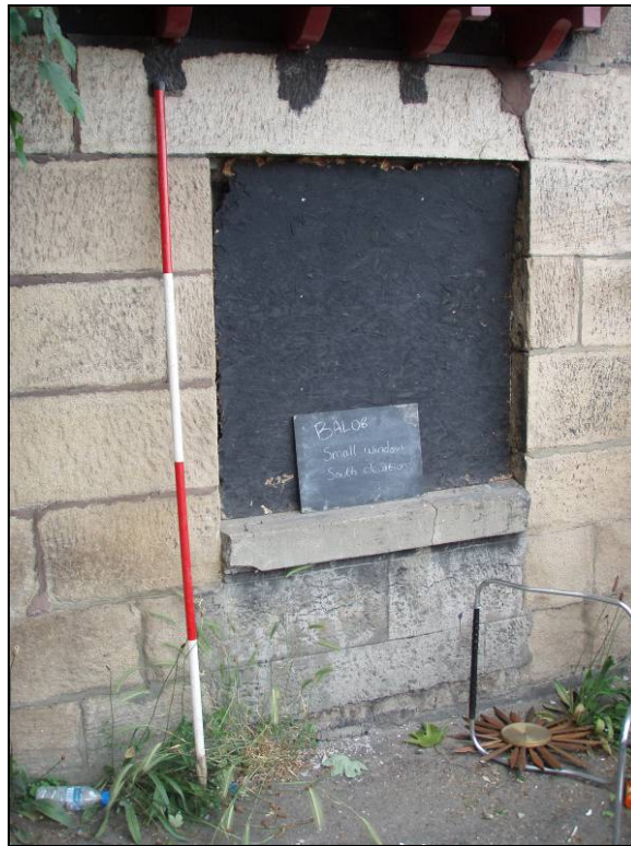
Fig. 10 South elevation, ground floor window
