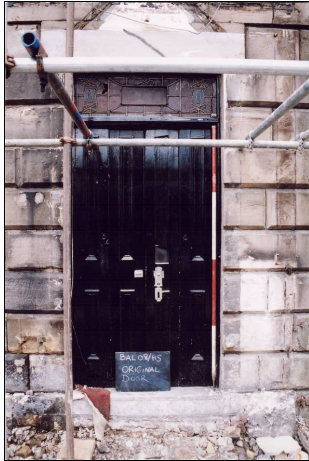
Fig. 16 Original wooden door to the east elevation
