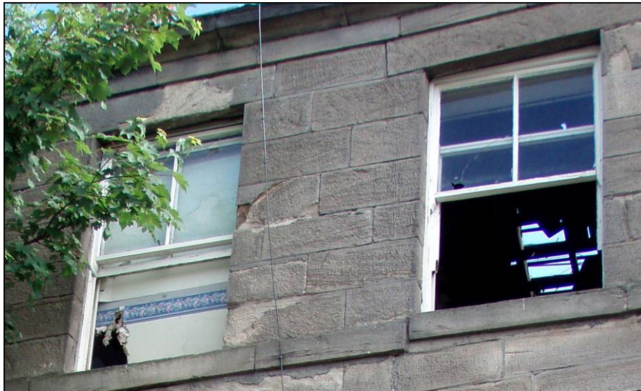
Fig. 7 South elevation Windows to the west side
