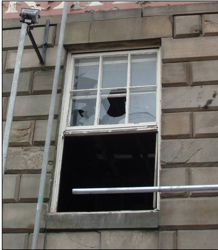
Fig. 6 East elevation, first floor window without moulding
