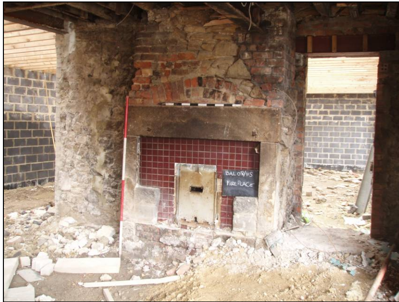
Fig. 12 Fire place with rough brick infill
