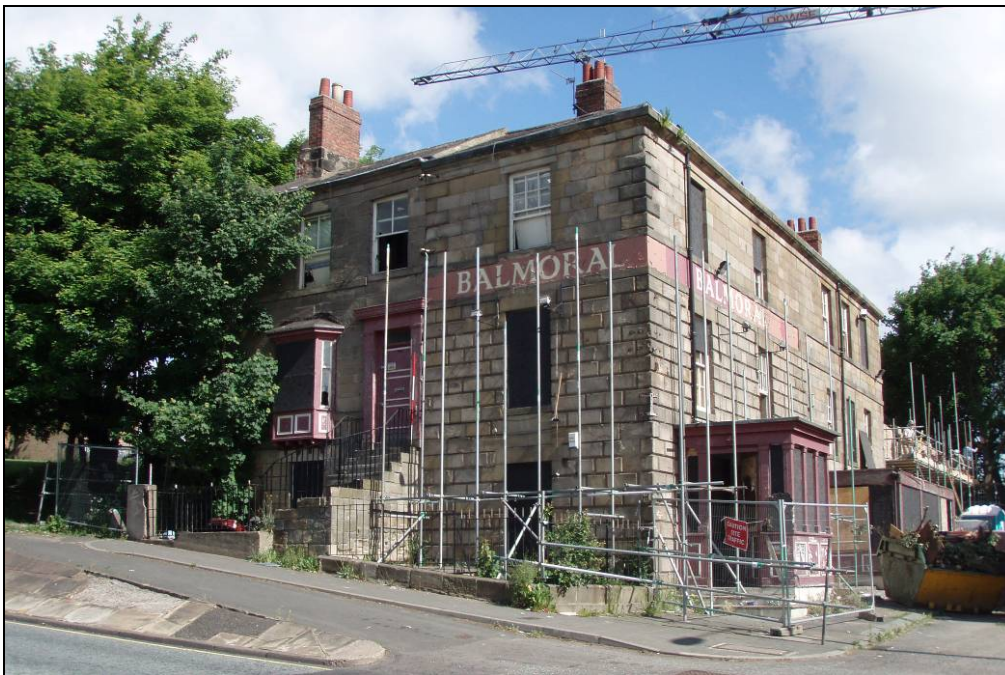
Fig 1. Balmoral profile shot showing south and east elevations.
