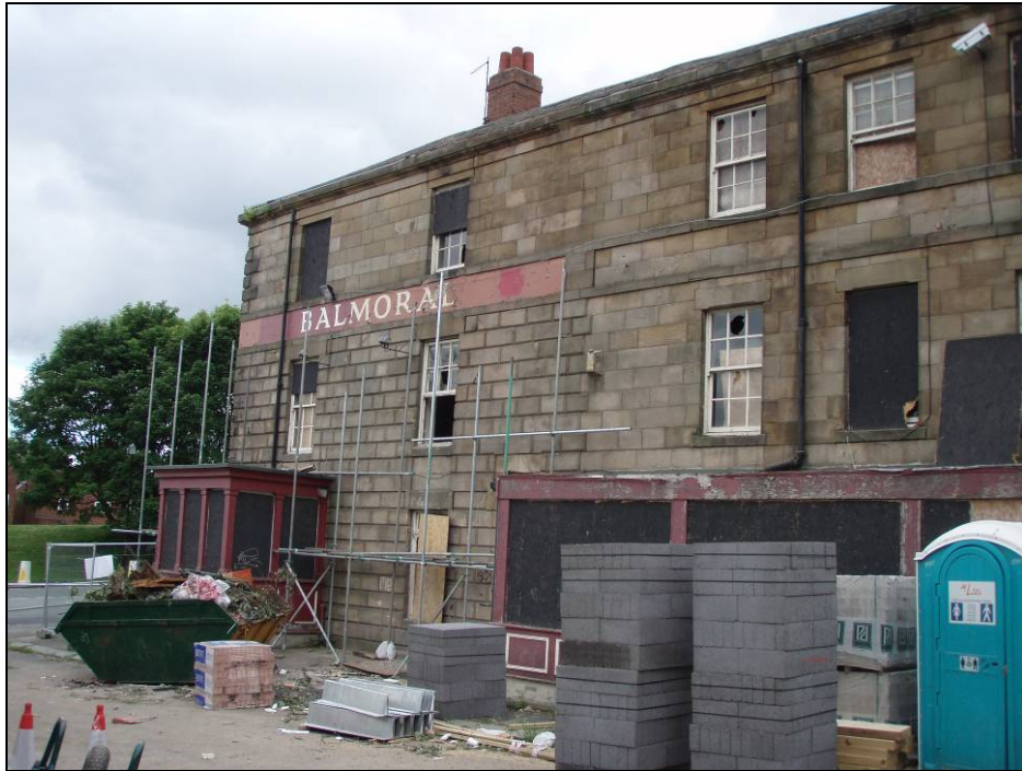
Fig. 13 East elevation showing Ashlar wall and cladding.
