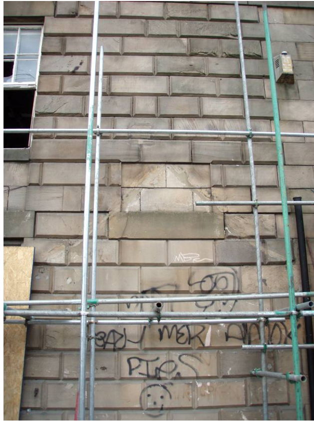
Fig. 14 East elevation 'blocked up door' with lintel
