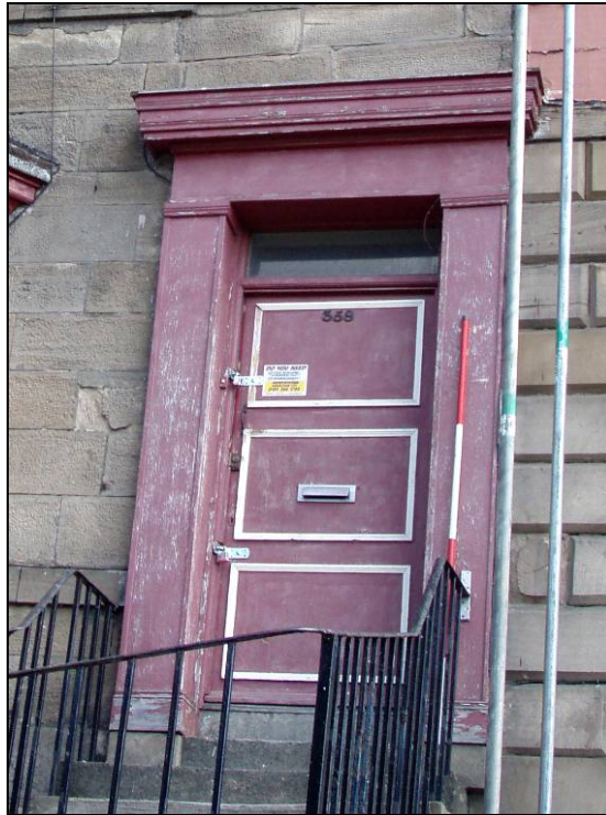
Fig. 19 South elevation entrance.
