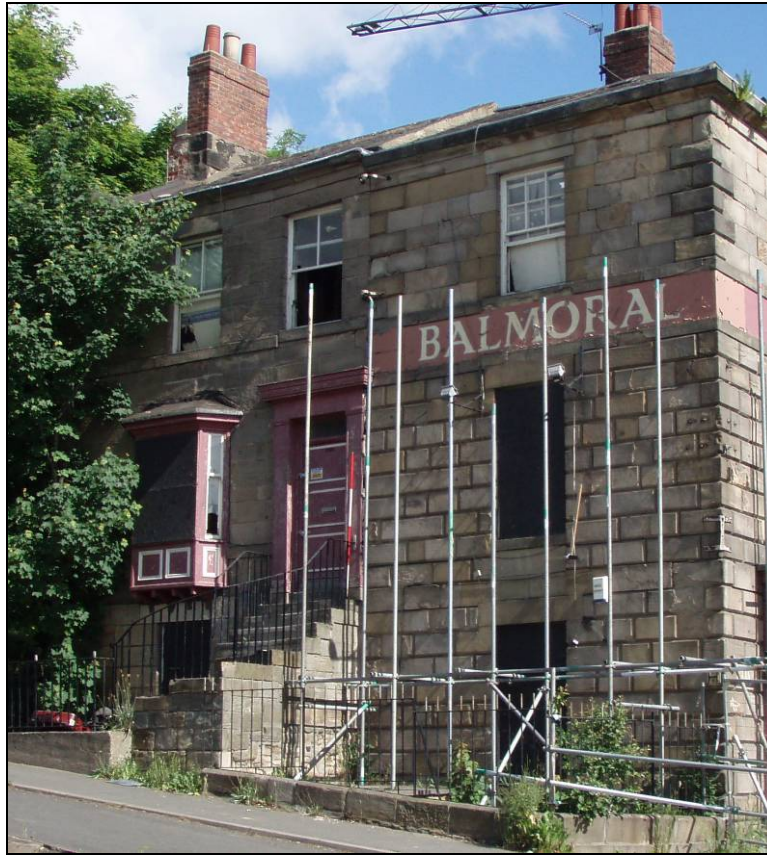
Fig. 15 South elevation wall
