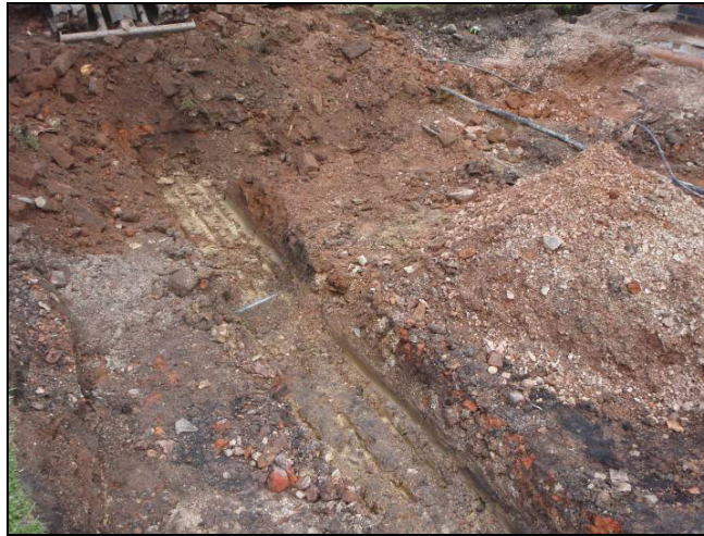
Fig. 23 View of the footings showing the depth of the natural alluvium.
