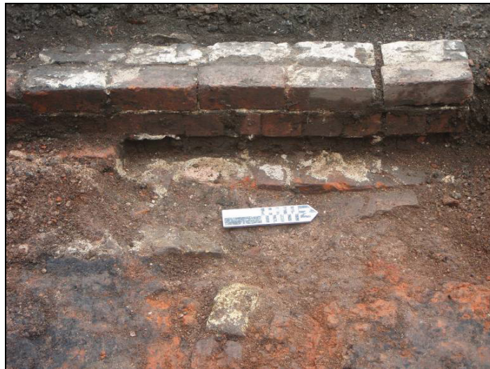
Fig. 7 View of the wall (002) and the earlier floor level (013). Looking west. (Scale: 0.25m)
