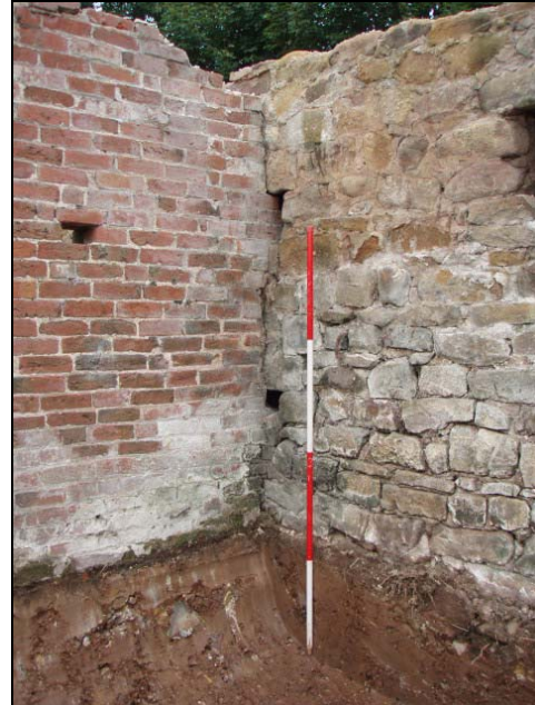
Fig. 64 Red brick wall separating the two rooms of the outbuilding
