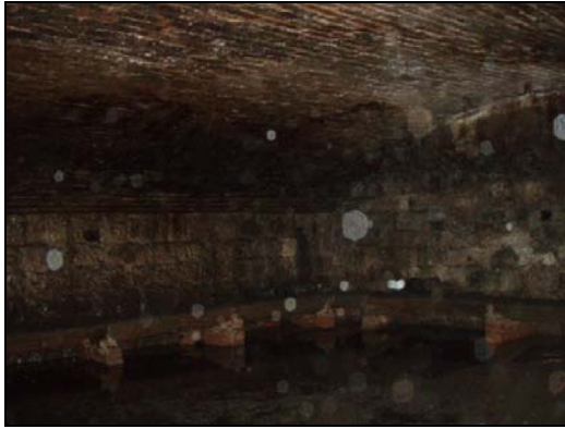
Fig. 61 Brick cellar located underneath Area Three
