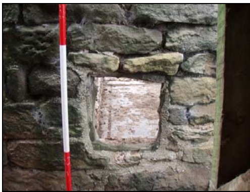
Fig. 49 Small square window in south-east elevation of Area Four
