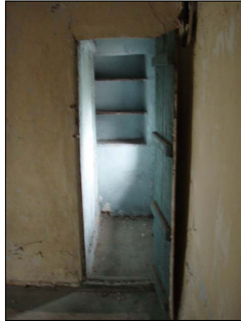
Fig. 60 Storage room off Room 8
