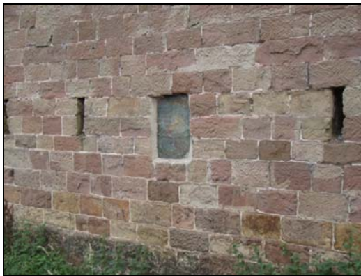
Fig. 11 Modern window in north-east elevation of the barn
