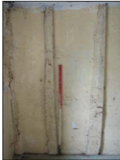
Fig. 58 Plastered wattle and daub forming the north-east wall of Room 7
