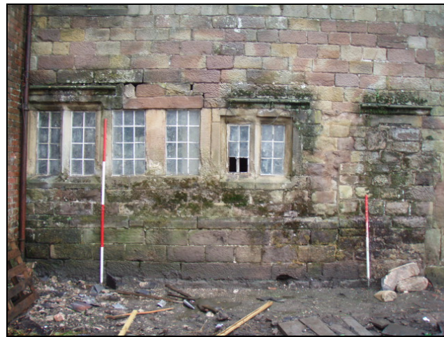
Fig. 33 Lower windows in south-east elevation of original farmhouse.
