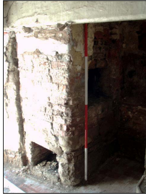
Fig. 53 Red brick bread oven in Room 3
