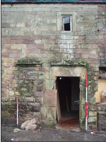
Fig. 36 Door within south-east elevation of farmhouse
