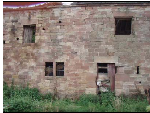
Fig. 12 Windows and doors in north-east elevation of the barn
