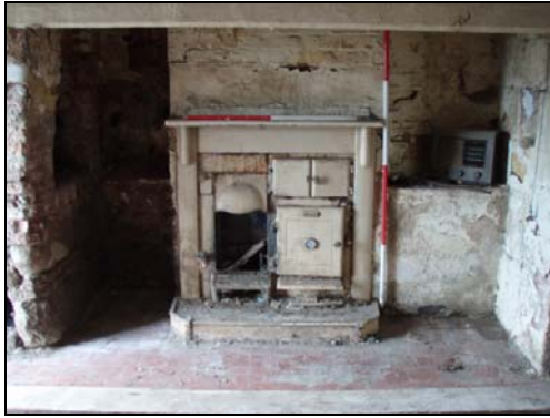
Fig. 52 Range and alcoves in Room 3
