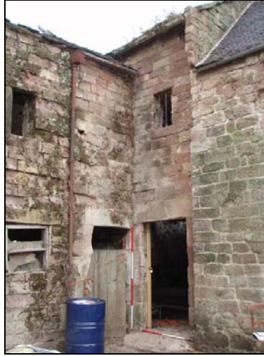
Fig. 20 Additional construction used to join the barn to the farmhouse
