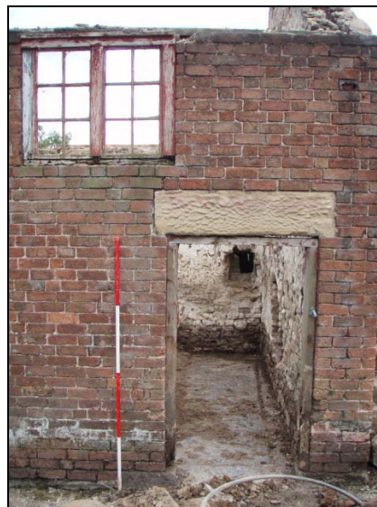
Fig. 46 Door and window within north-west elevation of Area Four
