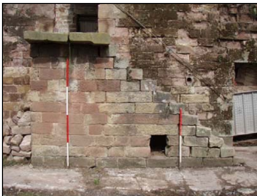
Fig. 18 Stairway on south-east elevation of the barn
