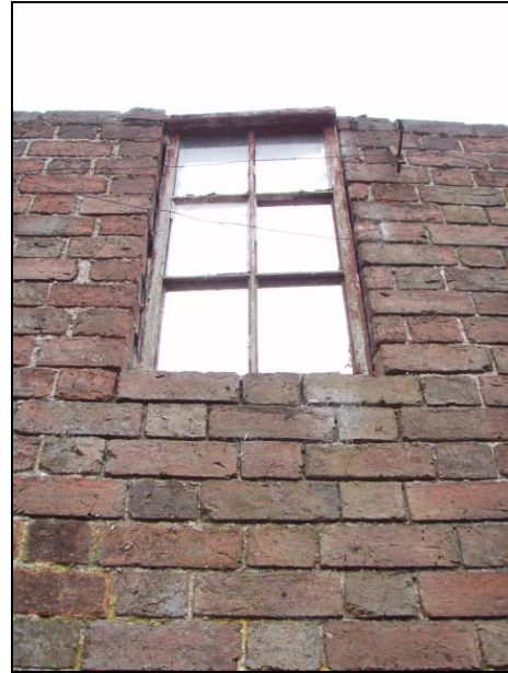
Fig. 45 Flemish style bricks construction of north-west elevation of Area Four
