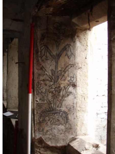
Fig. 56 Painted plaster on window jamb within Room 5
