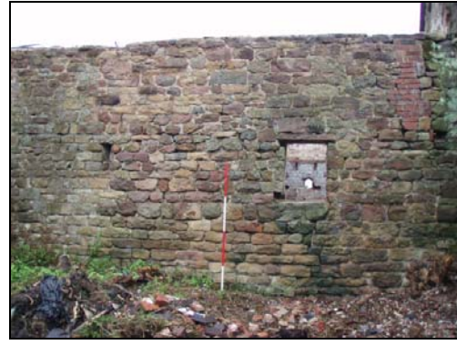
Fig. 48 South-east elevation of Area Four
