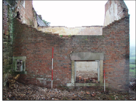
Fig. 43 South-west elevation of red brick extension
