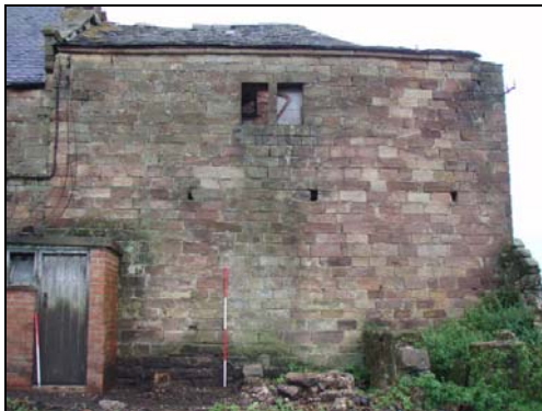
Fig. 21 South-east elevation of the barn
