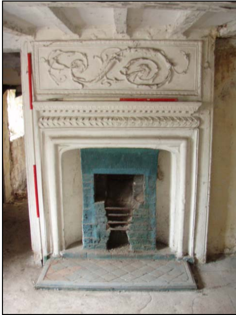
Fig. 59 Fireplace within Room 8
