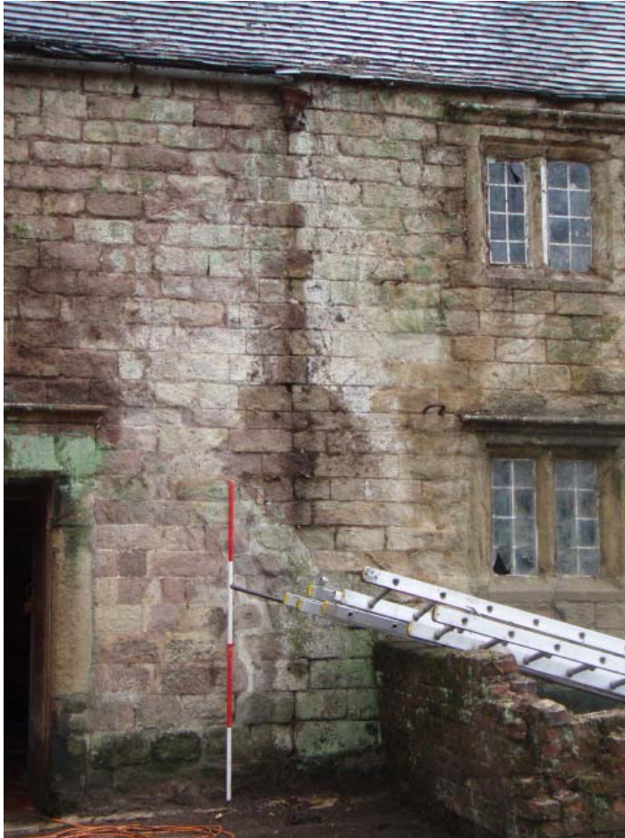
PLATE 2: BOND IN NORTH-WEST WALL SHOWING EXTENSION OF FARMHOUSE
