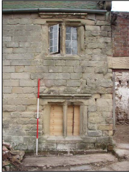
Fig. 26 Windows in north-west wall of the original farmhouse
