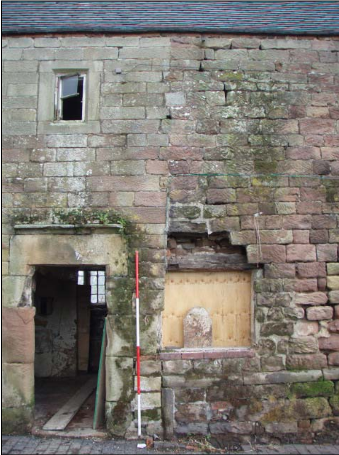
PLATE 3: BOND IN SOUTH-WEST WALL SHOWING EXTENSION OF FARMHOUSE
