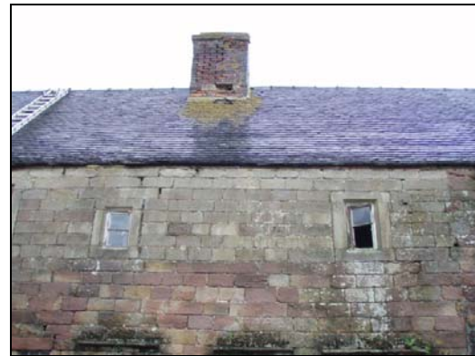
Fig. 35 Upper floor windows in south-east wall
