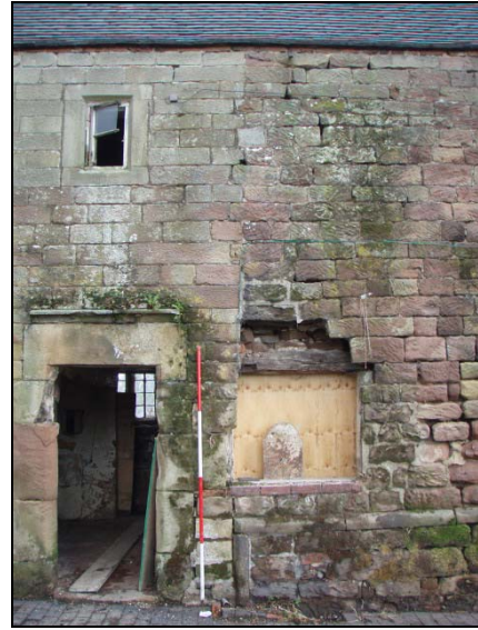
Fig. 25 Vertical bond between farmhouse and later addition on south-east wall
