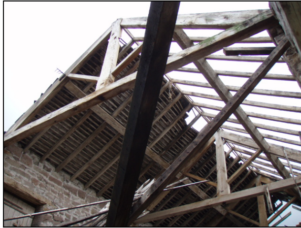
Fig. 51 King-post truss roof within the barn (Area One)
