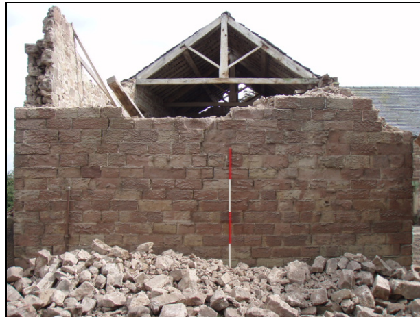
Fig. 13 North-west elevation, undergoing demolition, of the barn
