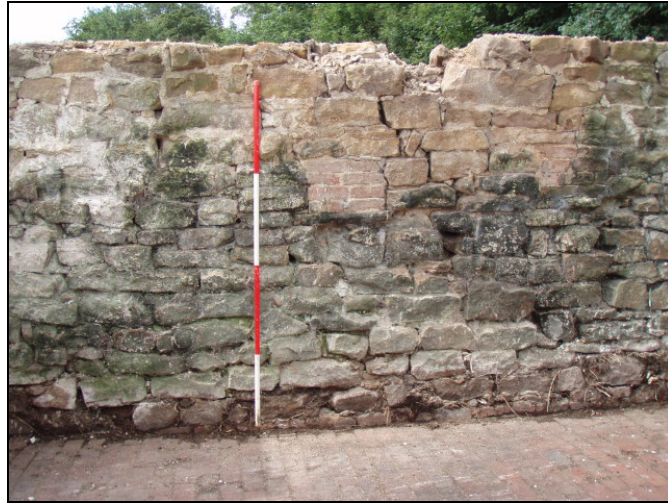
Fig. 65 South-west elevation with sealed window in centre of photograph
