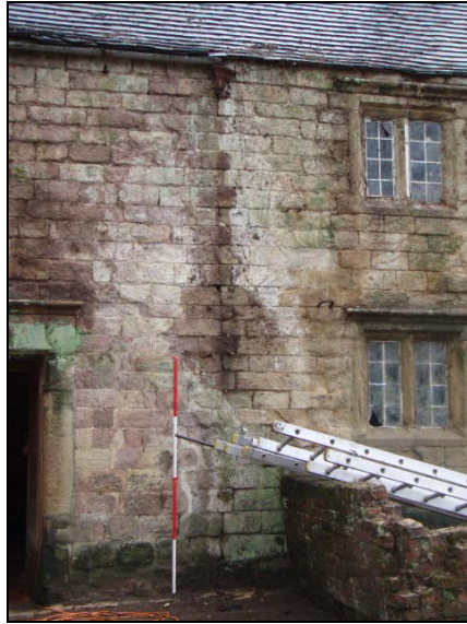
Fig. 24 Different coloured sandstone blocks and vertical bond between farmhouse and later addition added onto north-west wall
