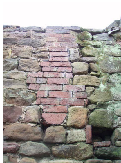
Fig. 50 Area of red bricks within south-east elevation of Area Four
