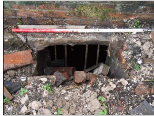
Fig. 41 Cellar grate located underneath the north-east elevation of Area Three
