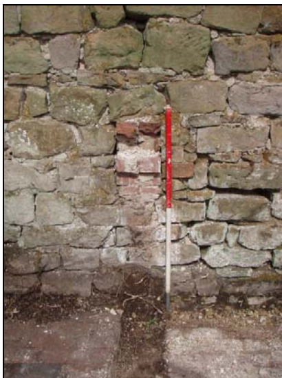
Fig. 66 Red brick dividing wall within north-west wall of outbuilding
