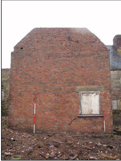
Fig. 42 South-east elevation of red brick extension
