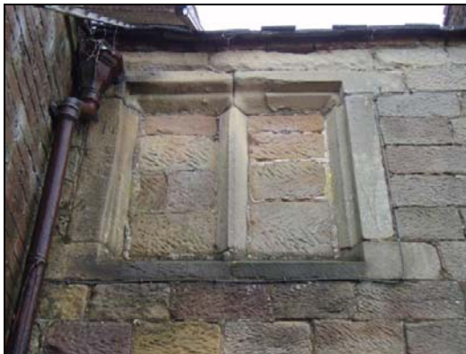
Fig. 34 Sealed upper floor window in south-east wall
