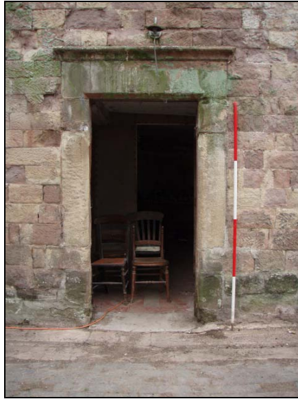
Fig. 30 Door within the north-west wall of the farmhouse extension
