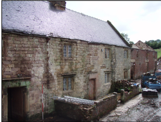
Fig. 23 North-west elevation of Farmhouse
