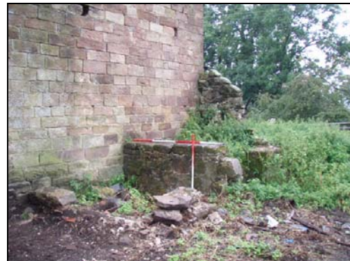
Fig. 22 Piggery located on the south-east elevation of the barn
