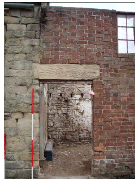
Fig. 32 Bond between the farmhouse (Area 2) and the red brick extension (Area 4).
