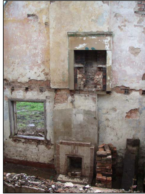
Fig. 62 Interior of Area Three showing the two fireplaces and the position of the first floor
