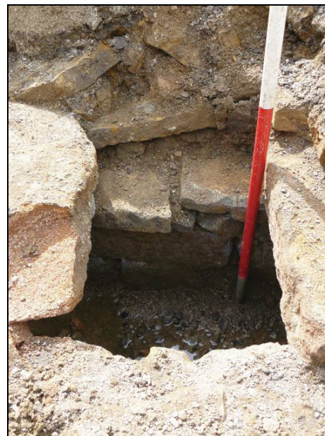
Fig. 11 Sandstone blocks forming the wall of the culvert
