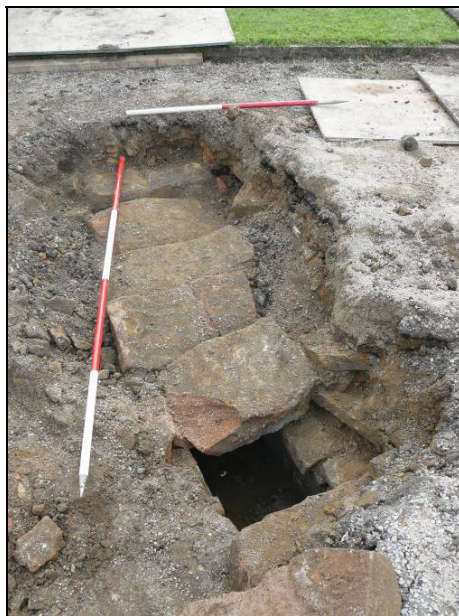
Fig. 10: Sandstone blocks forming the capstone of the culvert
