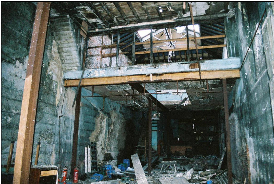
Fig. 24 Internal structure of 172/3 from the ground floor looking through to ceiling
