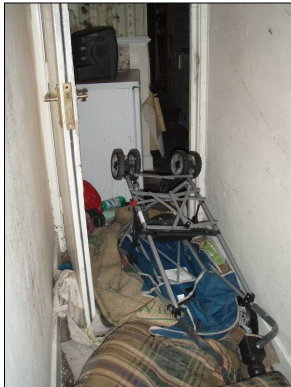
Fig. 32 Access passage to first floor staircase
