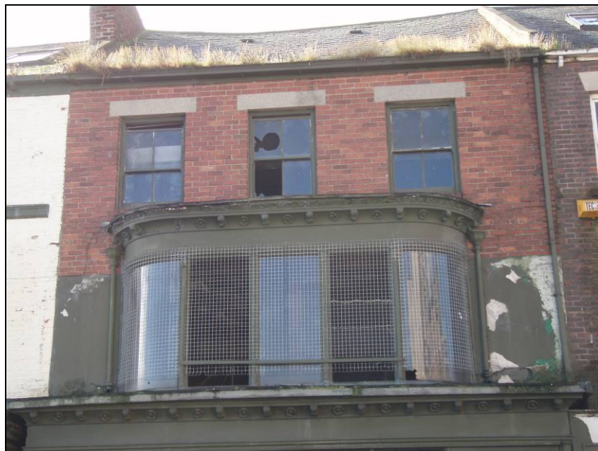
Fig. 22 First floor bay window and second floor sash windows 172/3
