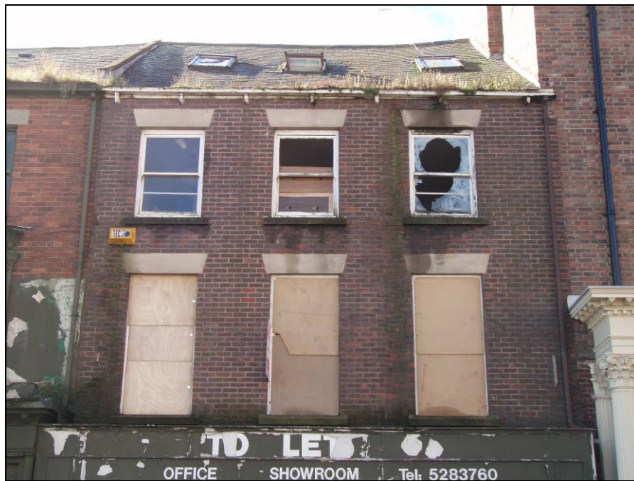
Fig. 28 First and second floor sash windows 174/5
