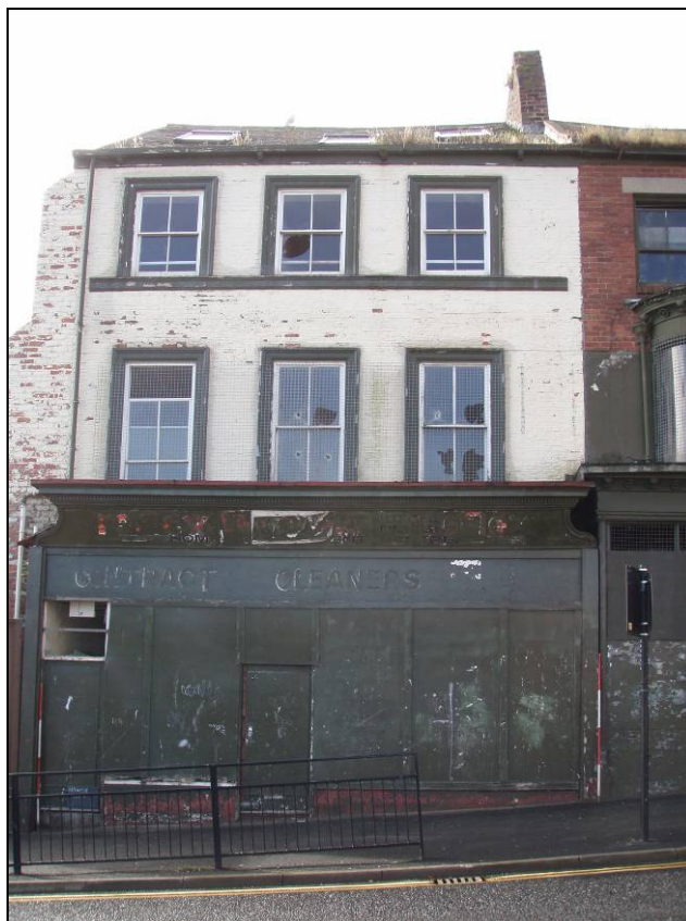
Fig. 16 170/1 High Street west north elevation
