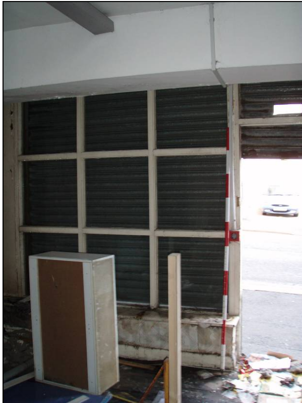
Fig. 29 North elevation (internal) showing shop frontage 174/5
