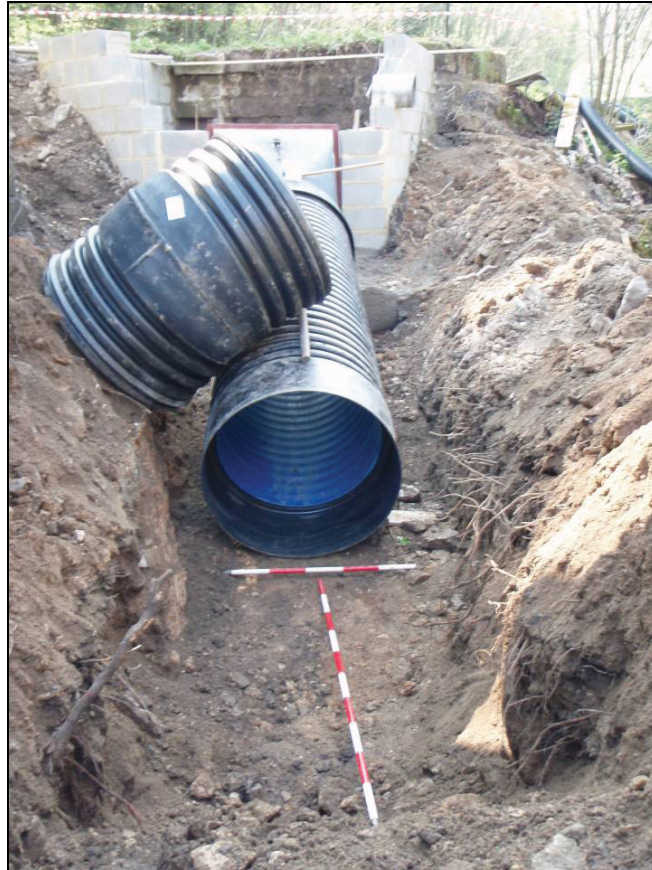
Fig. 13 Intake Tank and initial section of laid pipeline. Facing south
