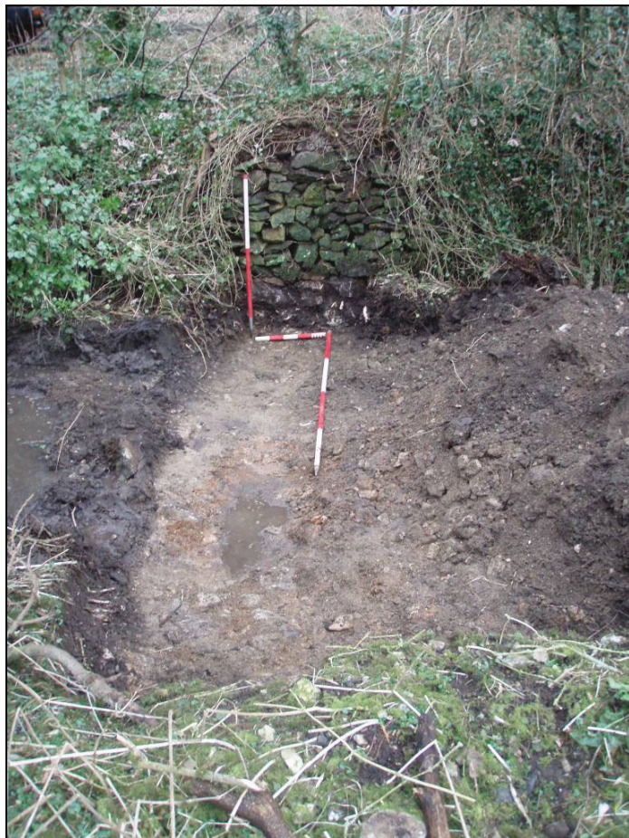
Fig.9 An intact section of the eastern mill race wall.
