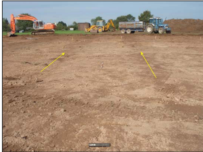
Fig. 5 Linear features (5 and 6) of context (003) highlighted by yellow arrows (facing north-west)
