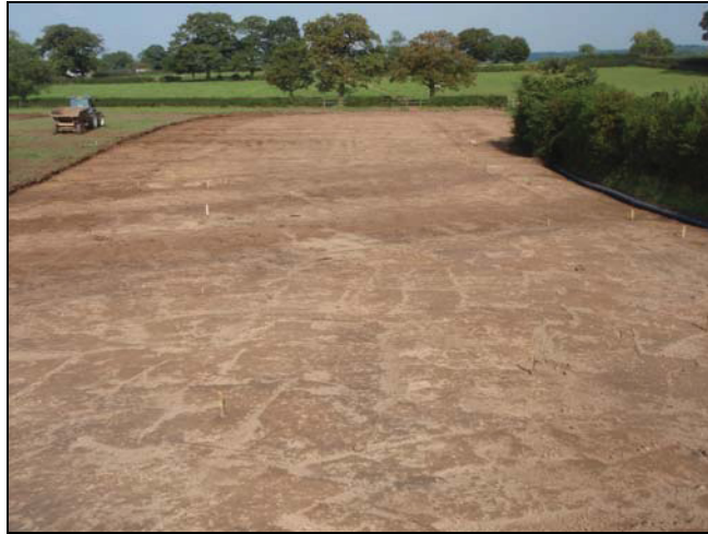
Fig. 2: Area of excavation after topsoil strip (facing north-east)
