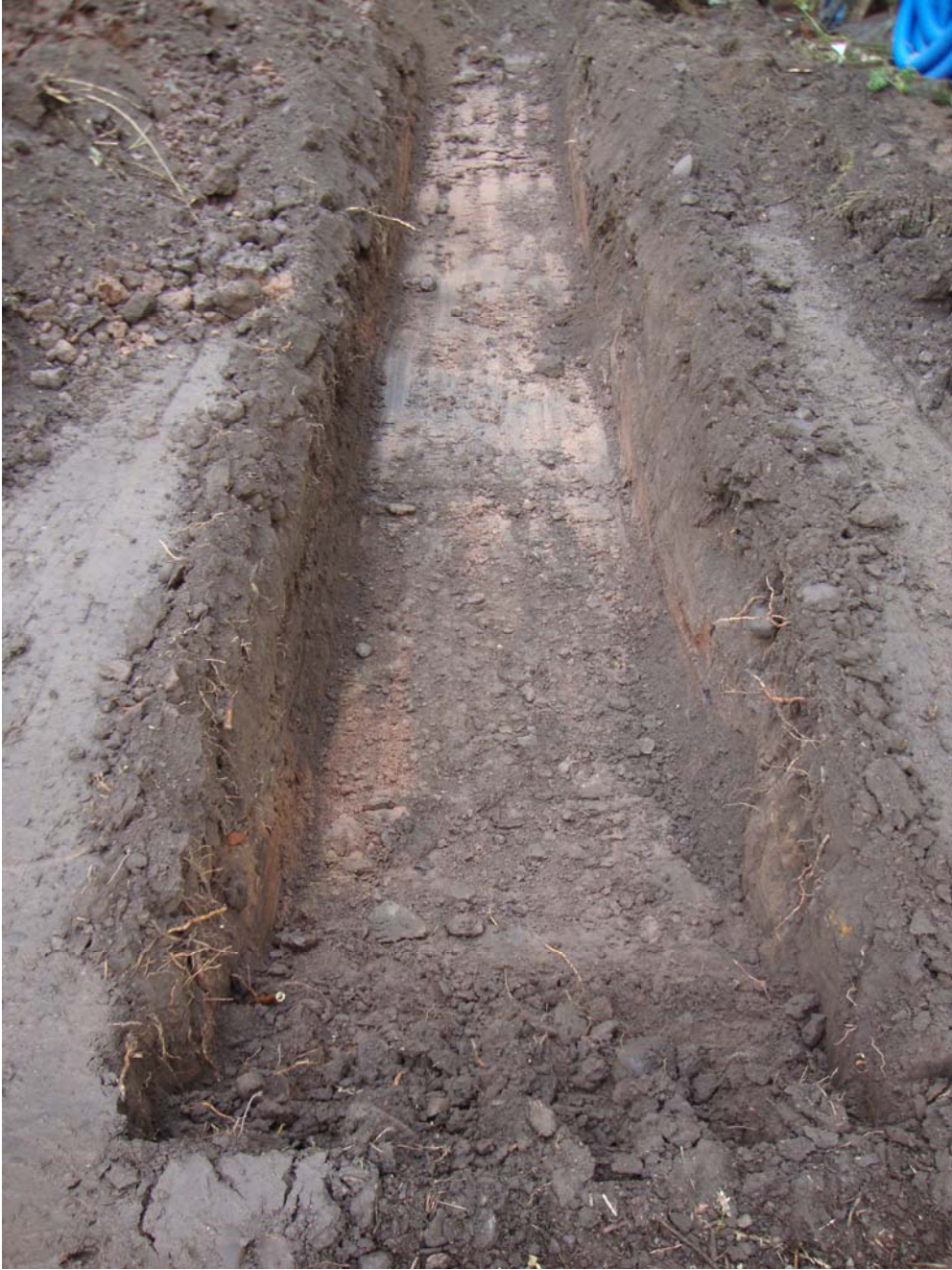
Figure 4: Excavated service trench to the front of the site
