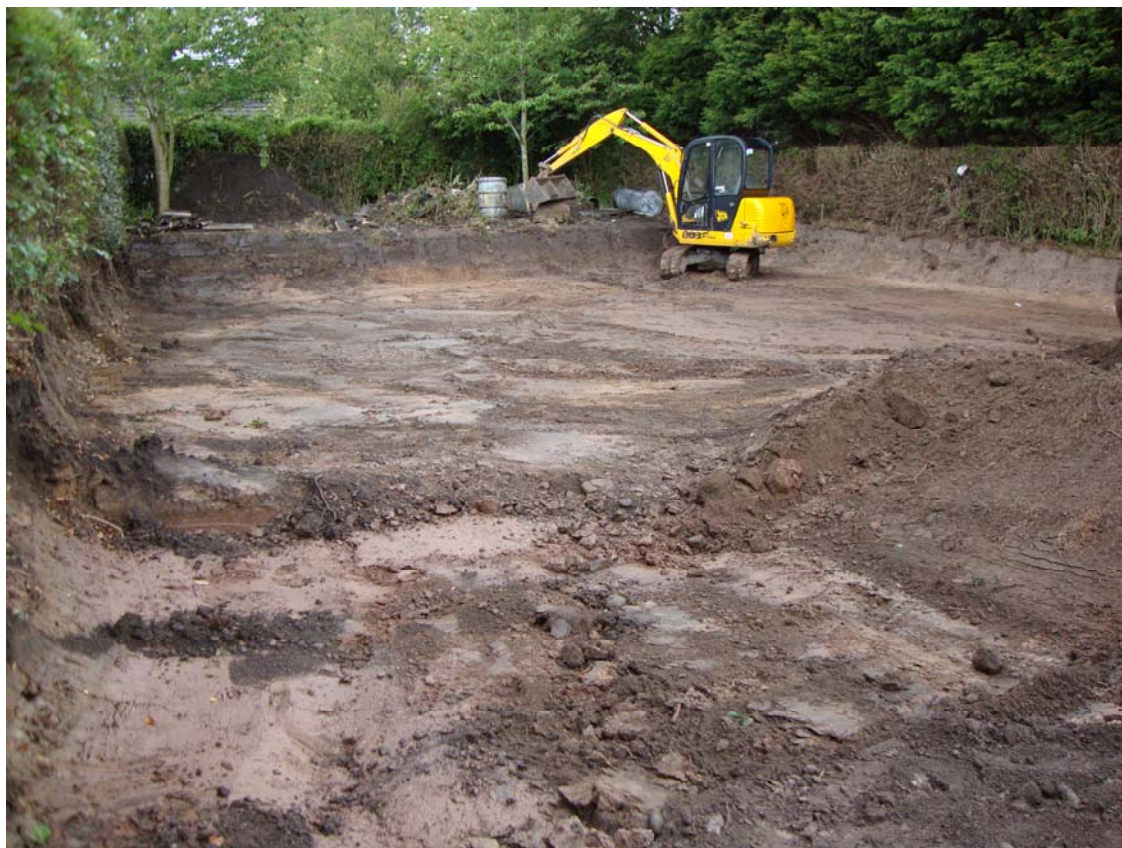
Figure 3: The site after levelling and excavation
