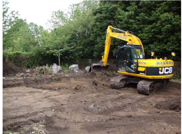
Excavation on site at Tarbits
