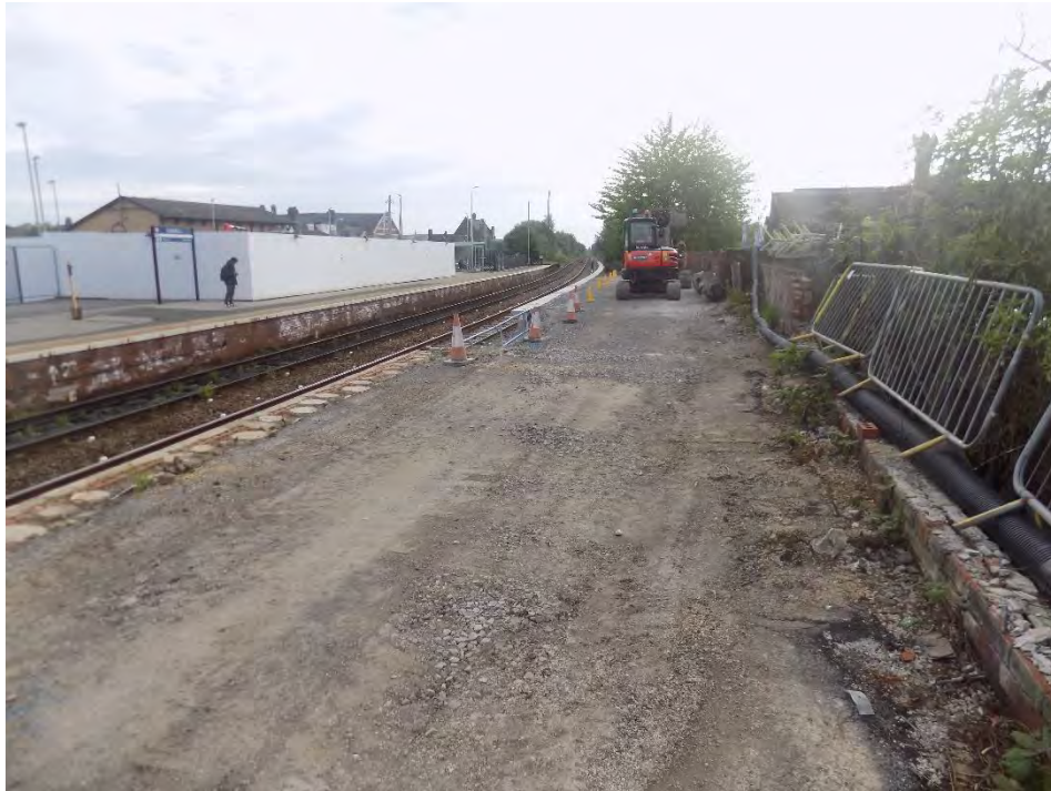
Figure 4. Platform 2, overview of watching brief area piling mat, looking east
