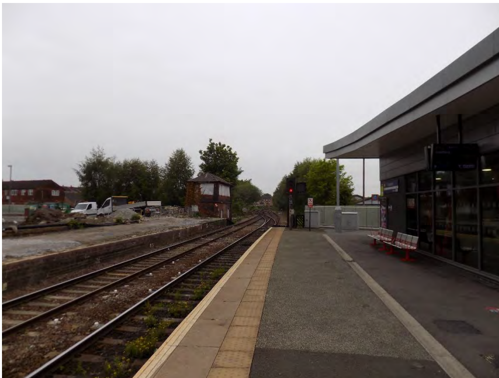
Figure 3. Overview of Castleford Railway Station from Platform 1, looking west towards disused signal box
