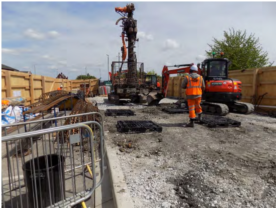
Figure 5. Piling in progress on Platform 1, looking west
