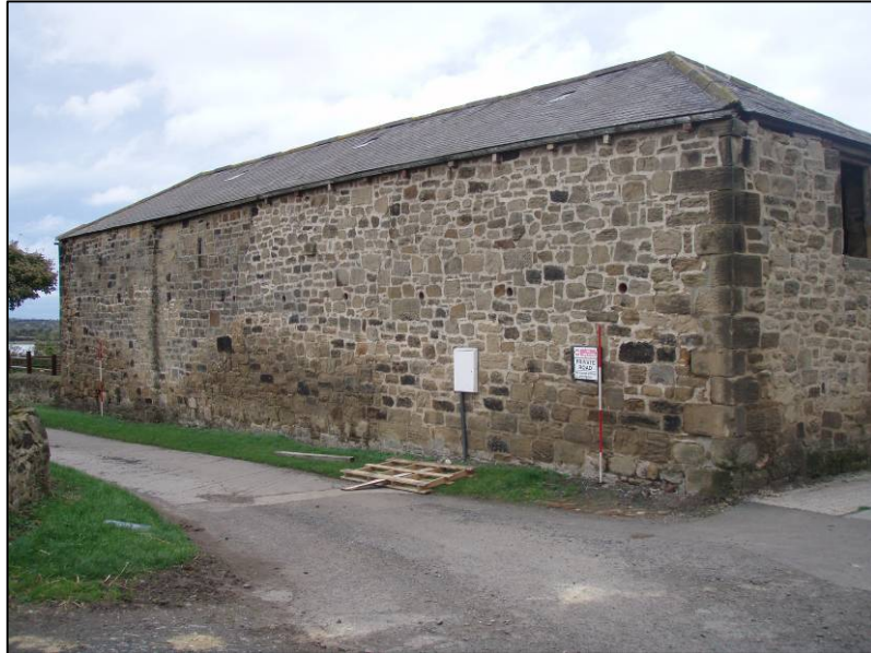
Fig. 19 Phase II west facing elevation, exterior.
