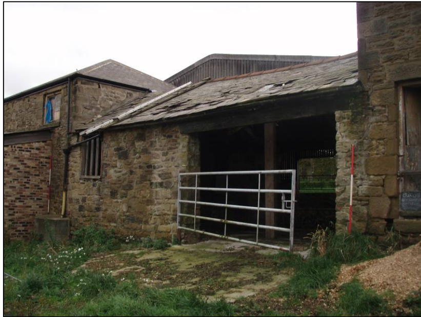
Fig. 23 Phase III North facing elevation, exterior.
