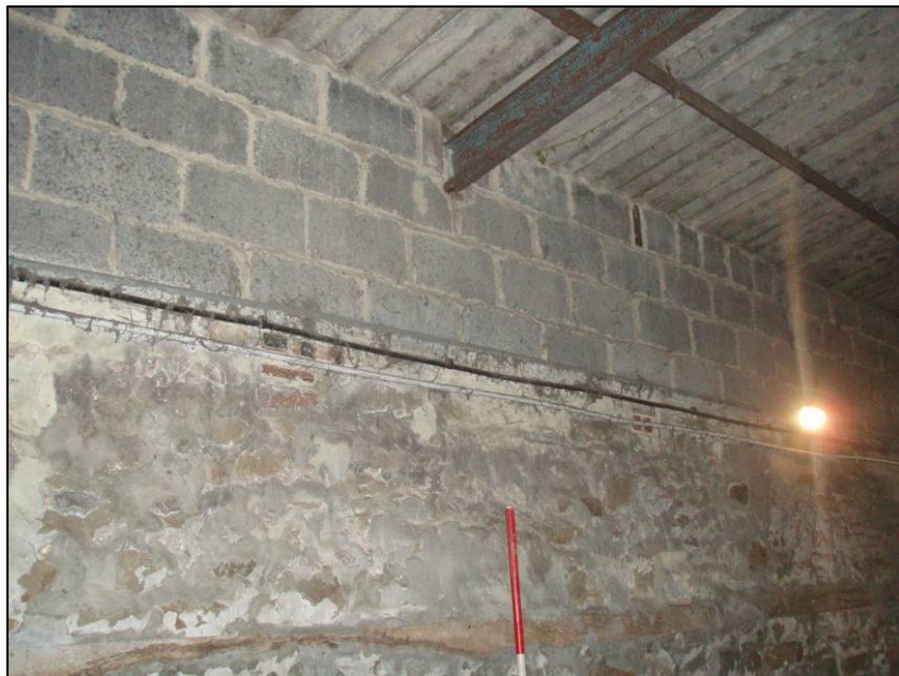
Fig. 34 Interior of room 6 showing remodelling of roof.
