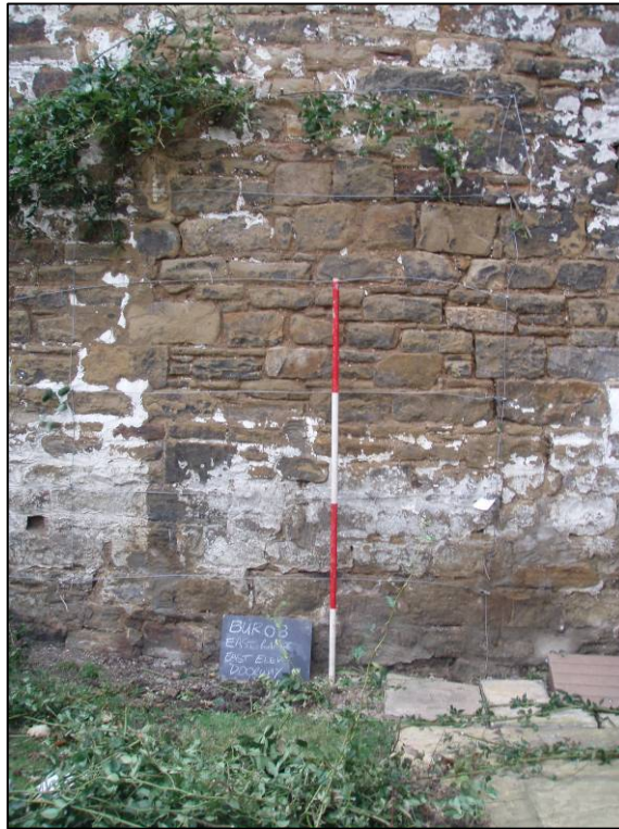
Fig. 25 Phase II east facing elevation, exterior doorway.
