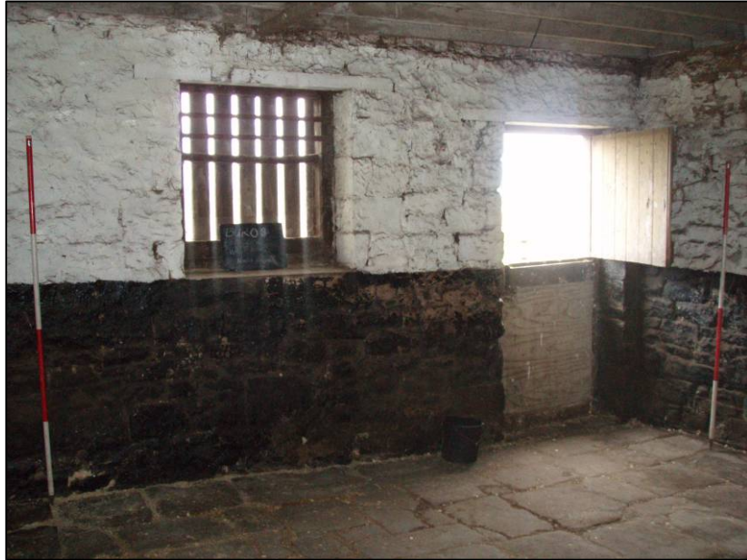
Fig. 33 Interior of room 3 looking east.
