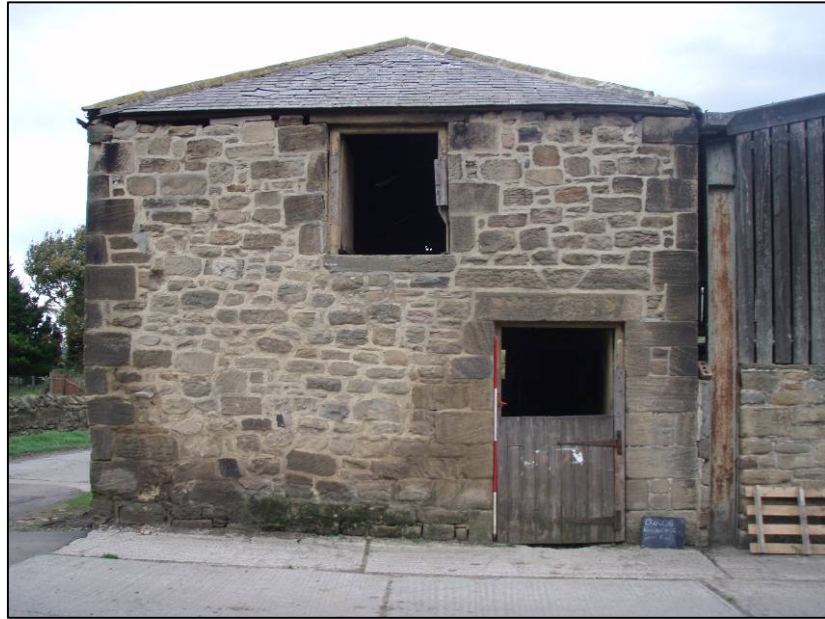
Fig. 17 Phase II south facing elevation, west side exterior.
