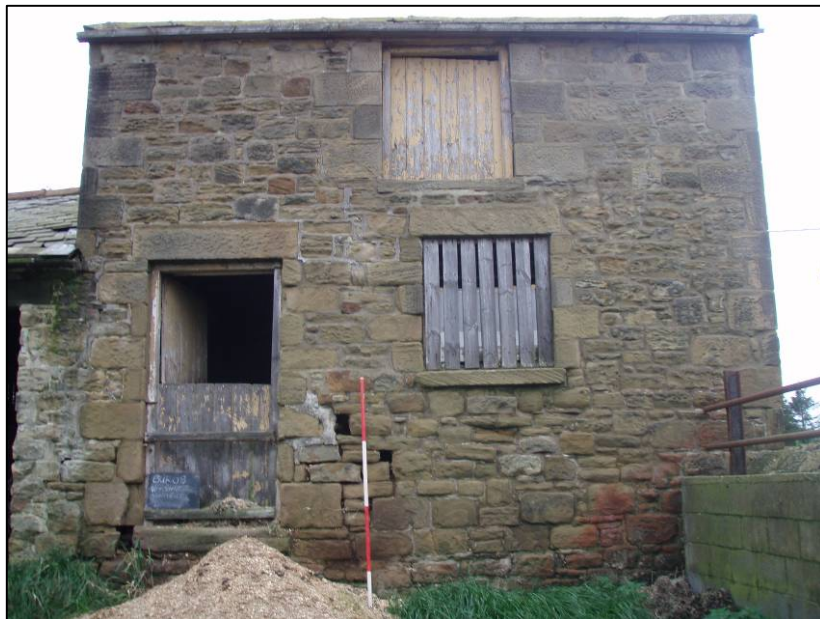
Fig. 22 Phase II north facing elevation, exterior.
