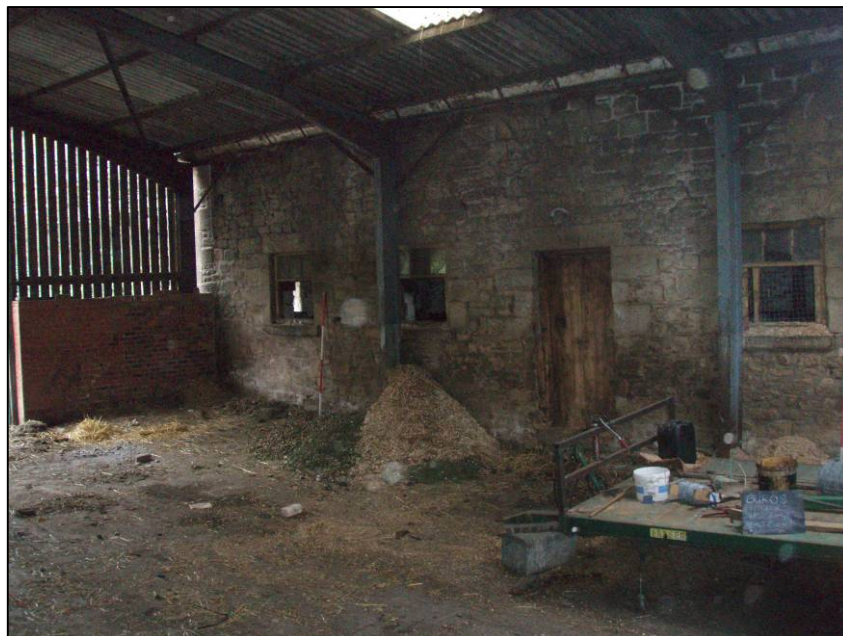
Fig. 26 Phase II east facing elevation, interior.
