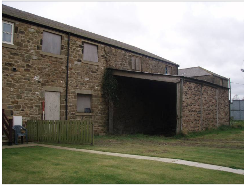
Fig. 21 Modern lean to on north elevation.
