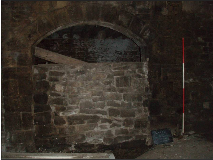
Fig. 29 Phase I in-filled archway.
