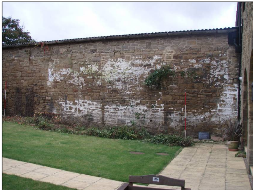
Fig. 24 East facing elevation, exterior.
