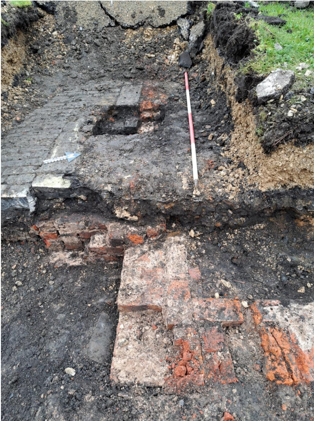
Figure 22: Photograph showing the extension to Trench 12, looking north-west. Foreground: walls {1218}/{1219}; background right: doorway {1220}/{1221}; background left: surface (1207). Scale 1x2m in 0.5m graduations.
