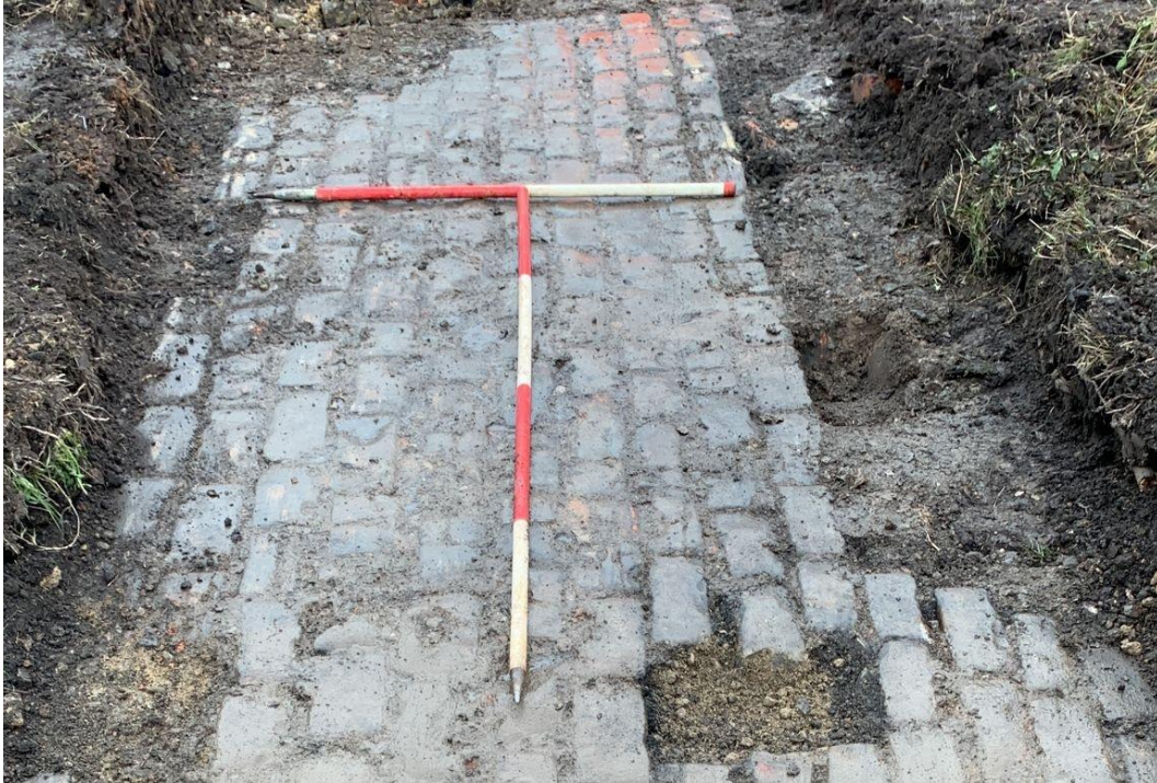
Figure 15: Photograph showing the truncated remains of Crown Street (804), looking north-west. Scale 1x1m and 1x2m in 0.5m graduations.
