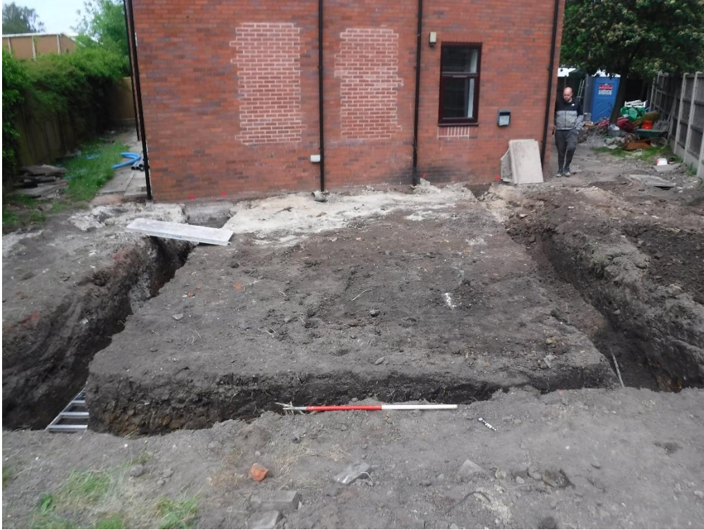
Figure 5. Completed foundation trench and ground reduction, looking northeast (scale: 1x1m)
