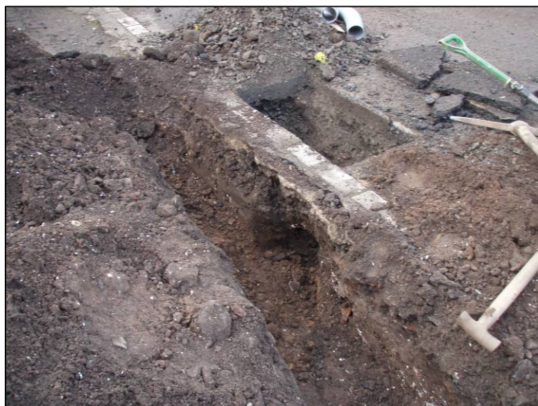
Fig. 4 Trench for ducting to be laid.
