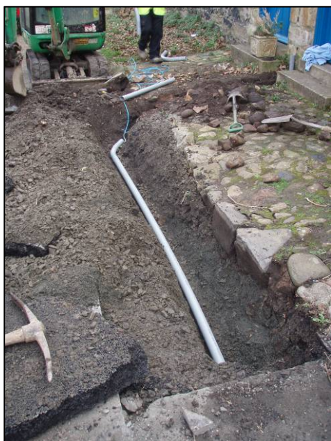
Fig. 5 Trench to the west of St Cuthberts Square
