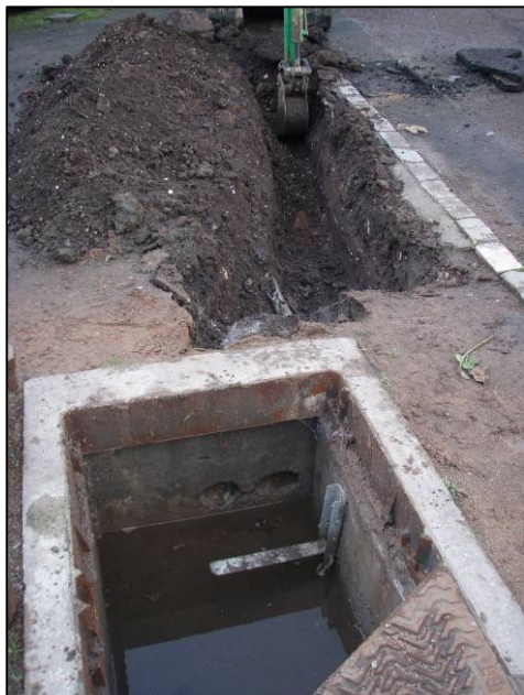
Fig. 3 Service box and Trench to the east of St Cuthberts Square
