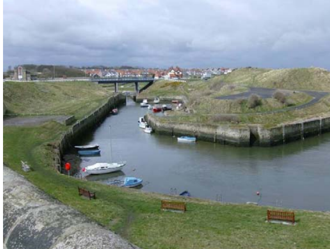
Figure 7.8 Seaton Sluice harbour; the sluice is below the road bridge (author)
