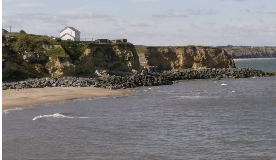
Figure 7.1 Rock armour at the base of cliffs north of Seaham (author)
