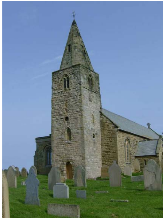
Figure 8.7 St Bartholomew's Church, Newbiggin (author)
