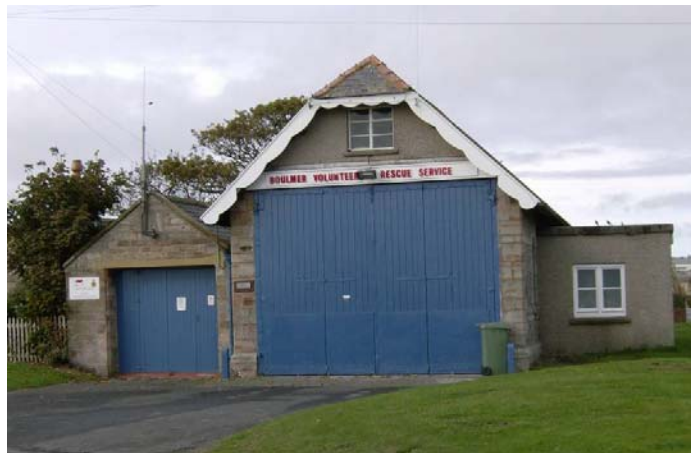
Figure 8.15 Boulmer Volunteer Rescue Service building (author)
