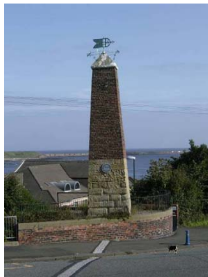
Figure 7.15 The East Lawe Beacon, South Shields (author)
