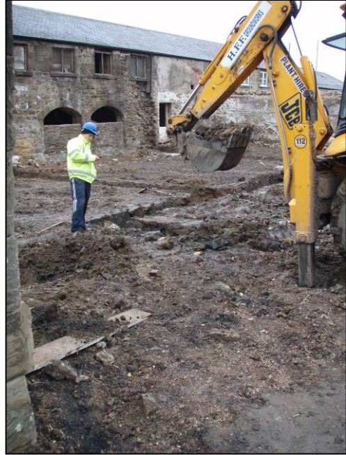
Groundworks at Burradon
