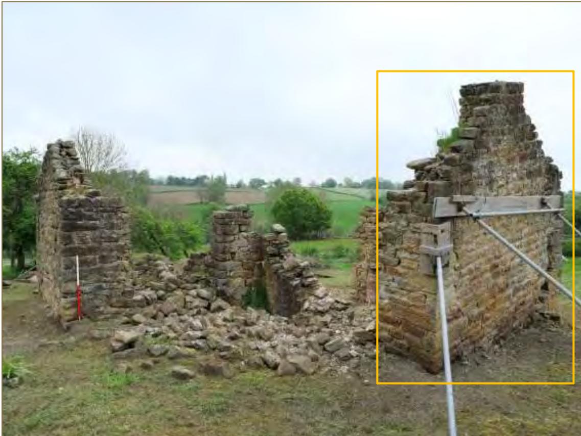
Photograph 14: The south elevation (looking north east). Scale 1m. (File: HBR_18)
