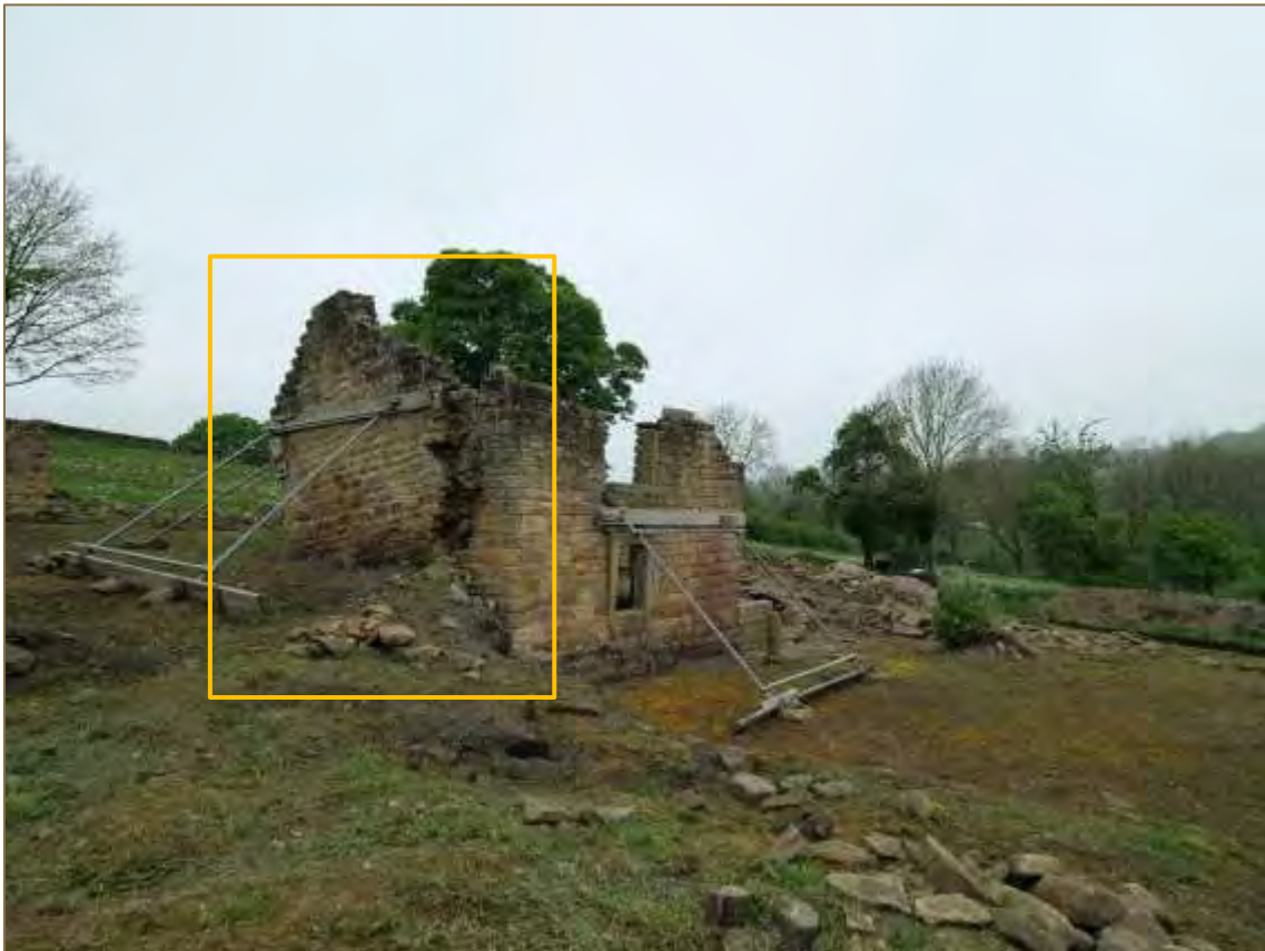
Photograph 13: Oblique view of the south elevation (looking north west). (File: HBR_132)
