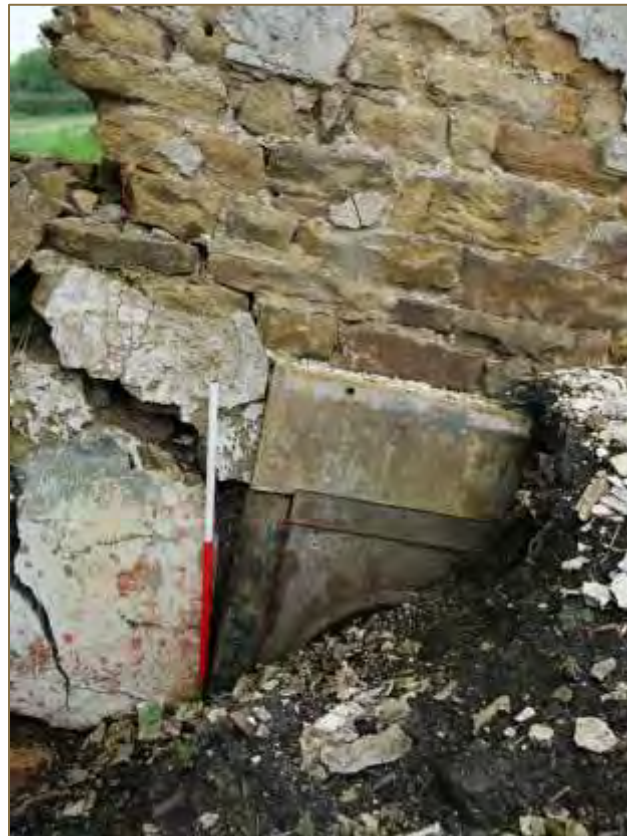
Photograph 24: The interior (looking south). Scale 1m. (File: HBR_299)
