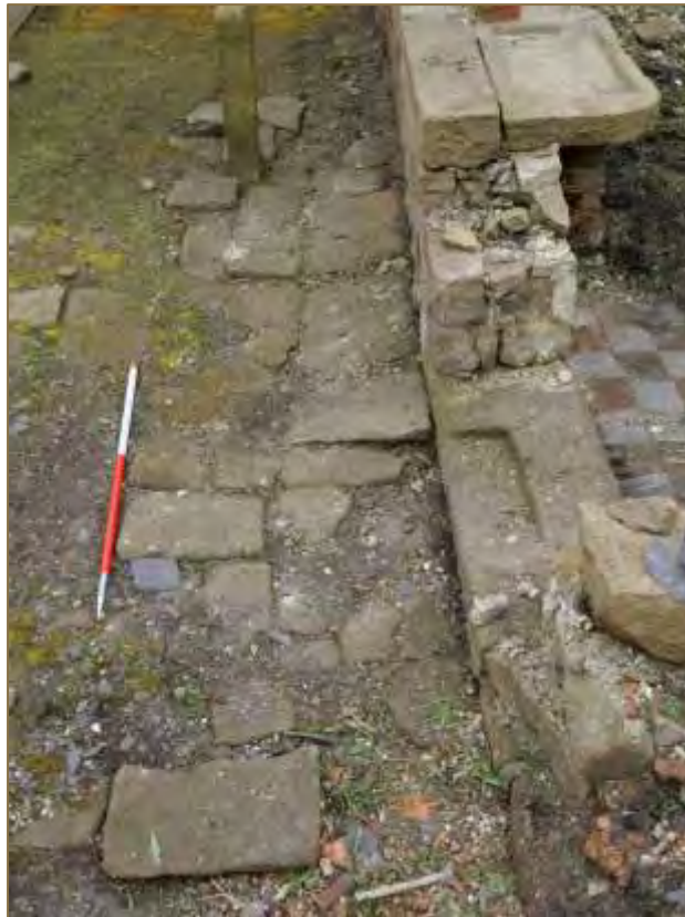
Photograph 11: The east elevation with stone step to entrance and paved area to front (looking south), and sink. Scale 1m. (File: HBR_75)
