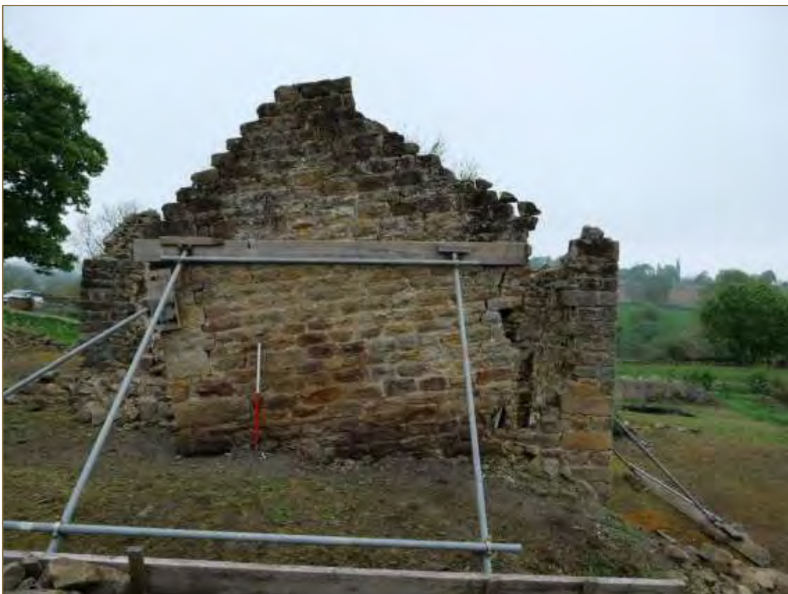
Photograph 15: The south elevation of (looking north). Scale 1m. (File: HBR_152)
