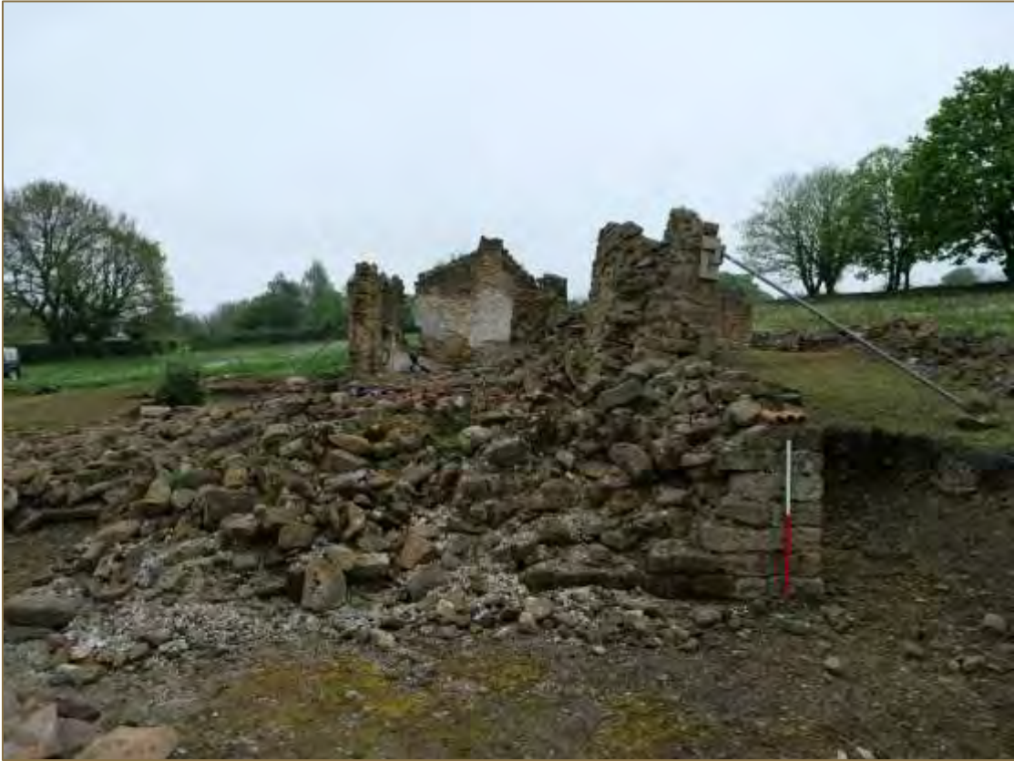
Photograph 19: The north elevation (looking west). Scale 1m. (File: HBR_152)
