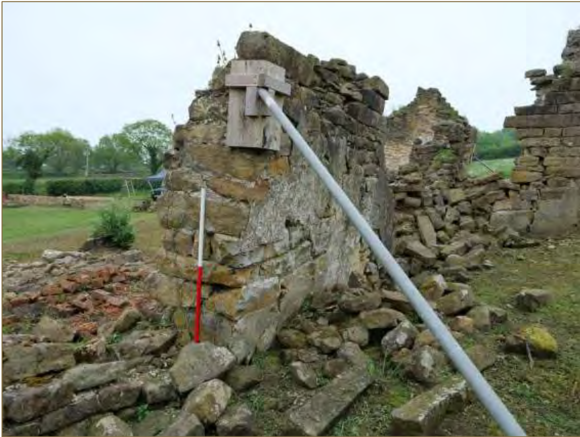
Photograph 17: The west elevation (looking south). Scale 1m. (File: HBR_152)
