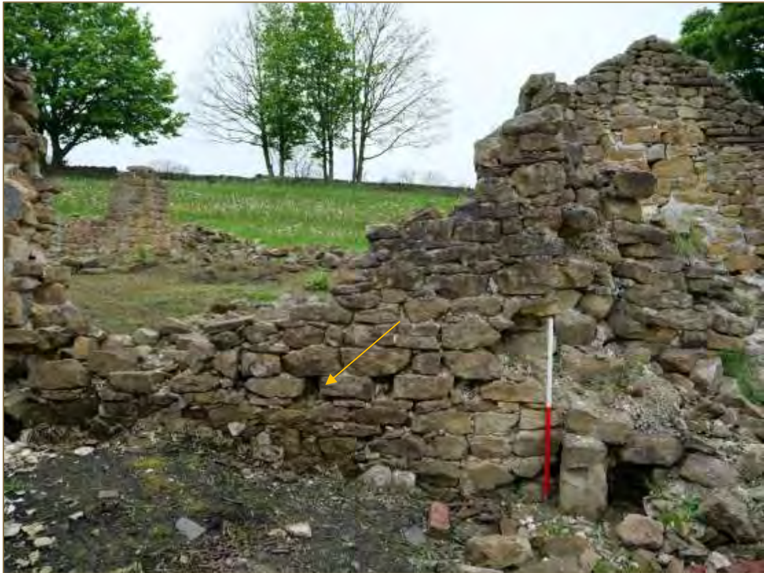
Photograph 25: The interior (looking north), showing beam slots. Scale 1m. (File: HBR_314)
