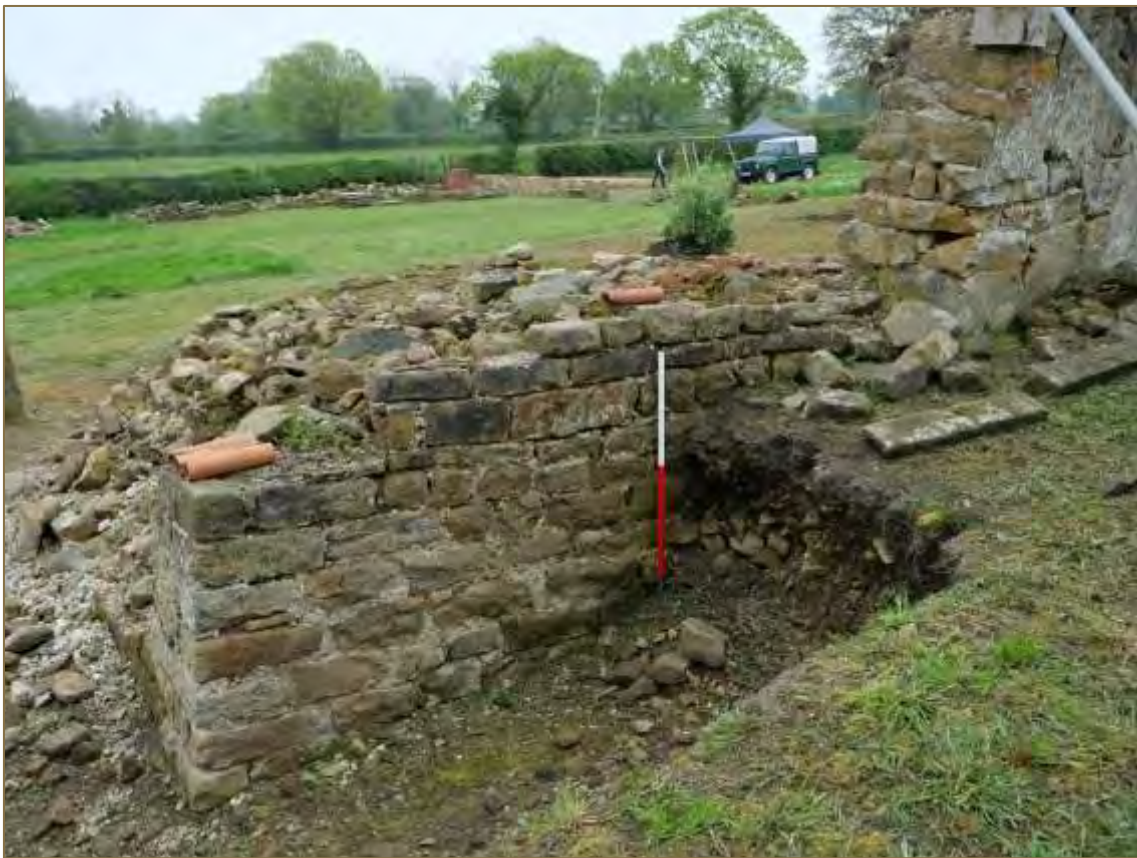
Photograph 18: The west elevation (looking east). Scale 1m. (File: HBR_152)
