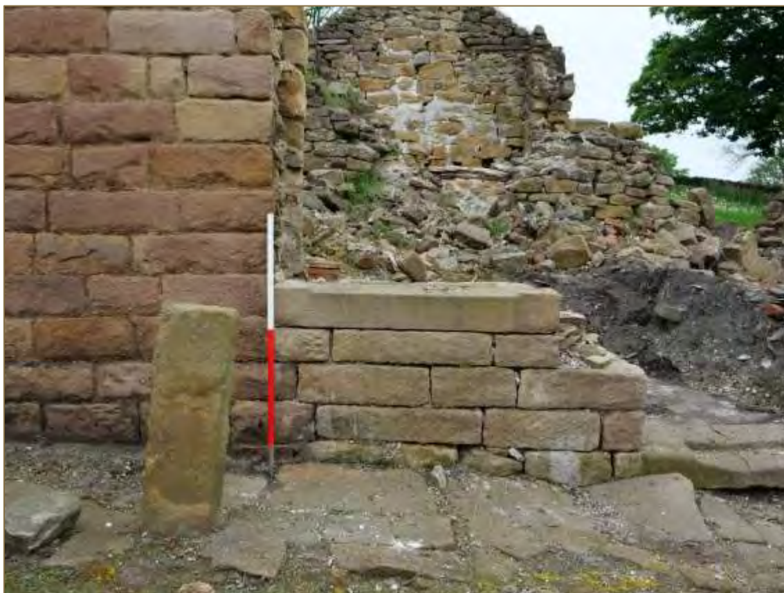
Photograph 10: The in-situ cill to the centre range aperture. Scale 1m. (File: HBR_112)
