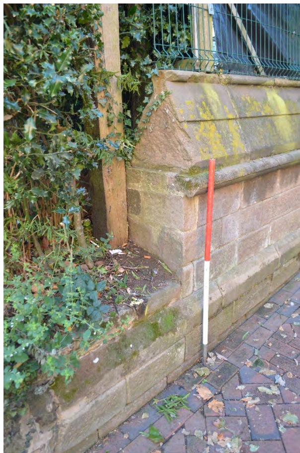
Photograph 6. Easterly end of middle and upper course of wall, looking south-west. Scale in 0.5m graduations.
