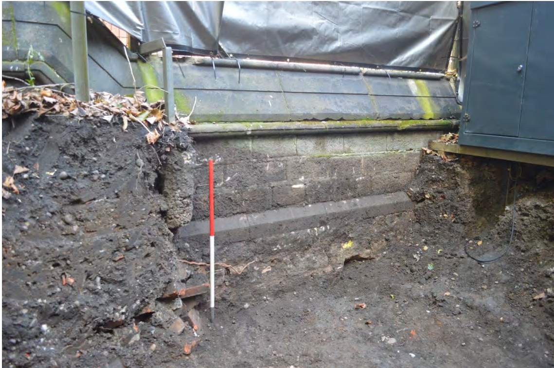
Photograph 3. South elevation of the wall, with footings revealed after archaeological excavation, looking north-east. Scale in 0.5m graduations.
