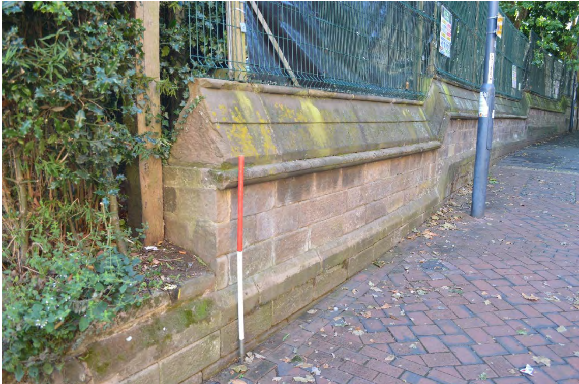
Photograph 7. Easterly end of middle and upper course of wall, looking south-west. Scale in 0.5m graduations.
