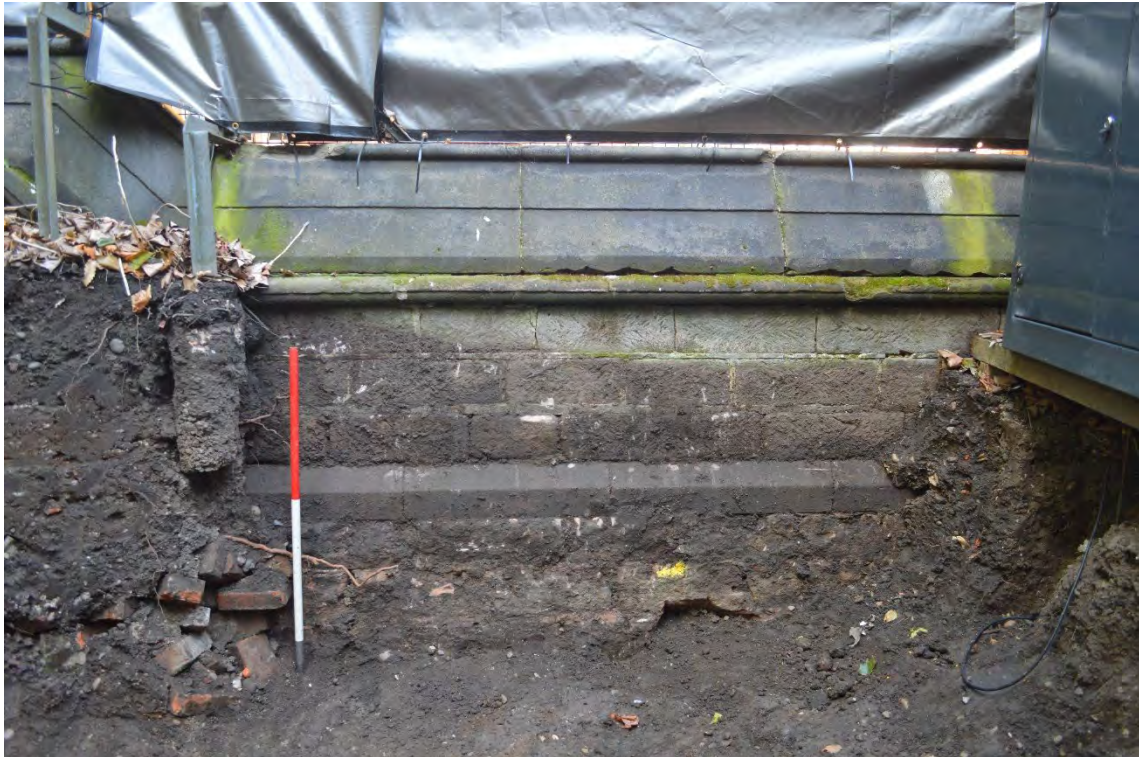
Photograph 1. South elevation of the wall, with footings revealed after archaeological excavation, looking north. Scale in 0.5m graduations.
