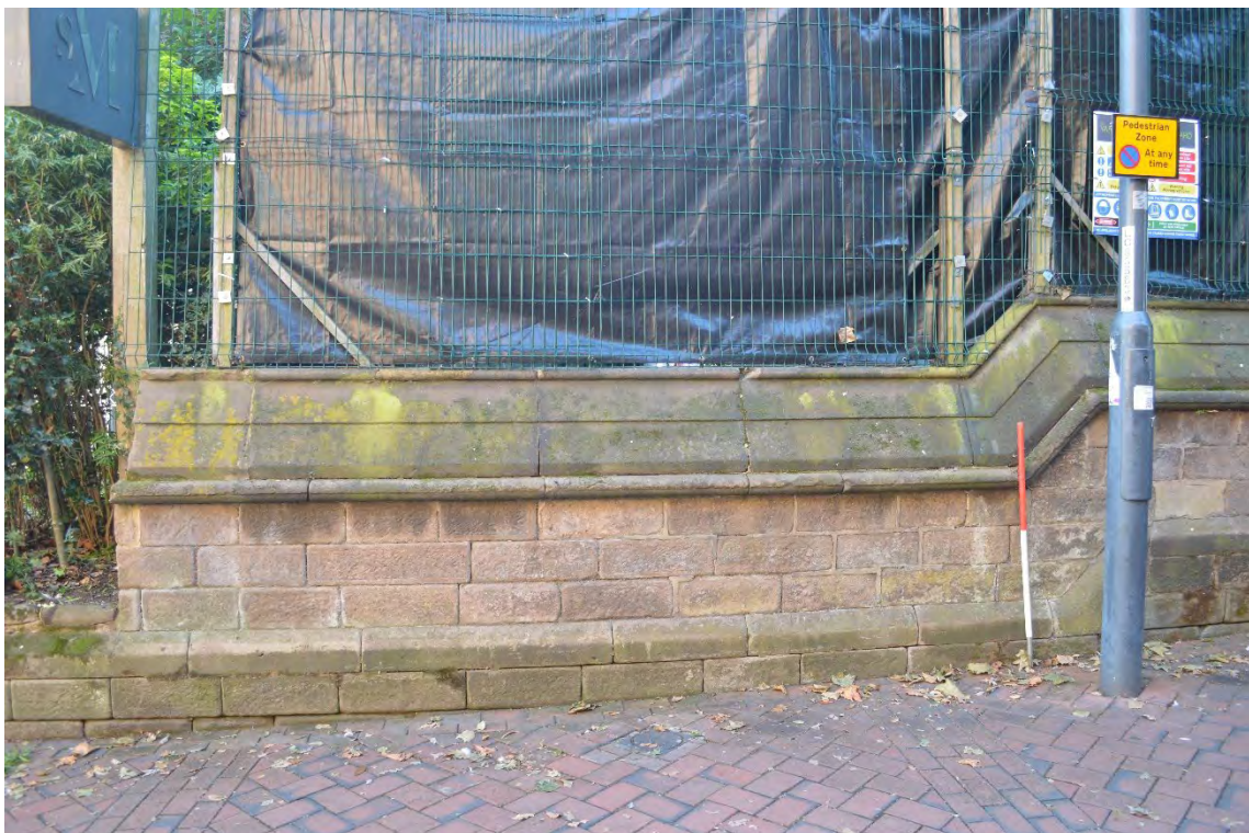
Photograph 4. North elevation of wall, taken from St Peter's Churchyard Street, looking south. Scale in 0.5m graduations.
