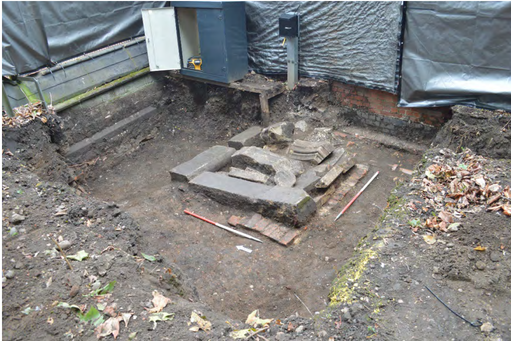
Figure 5. View north-east of brick structure {306} backfilled stone (308) and (307) and wall {313} (scale = 2 x 1m in 0.5m graduations)
