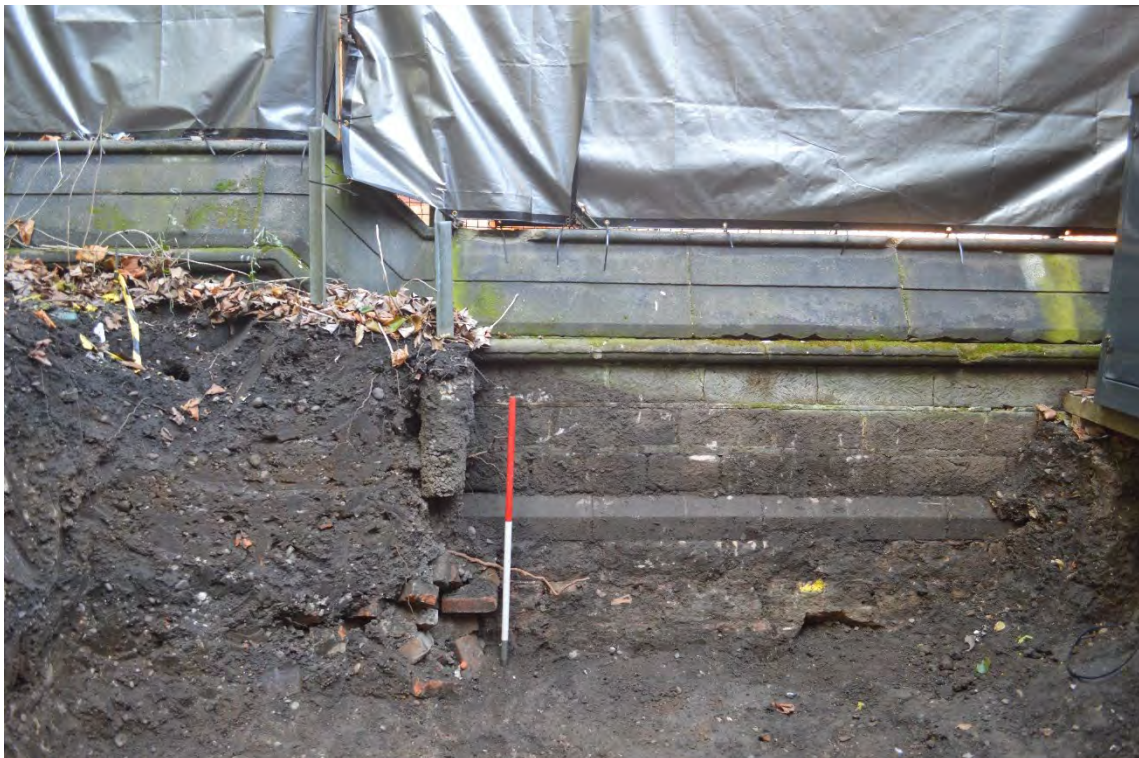
Photograph 2. South elevation of the wall, with footings revealed after archaeological excavation, looking north. Scale in 0.5m graduations.
