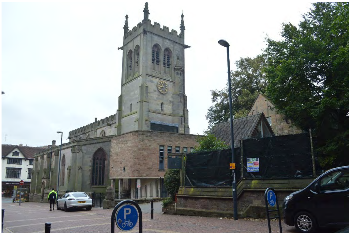
Photograph 16. North elevation of wall, panning upwards to church tower, looking north-west.
