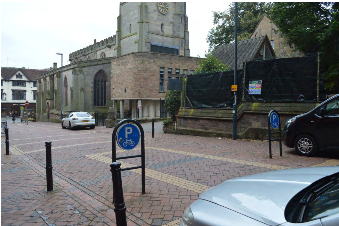
Photograph 14. Oblique location shot of north elevation of wall, with St Peter's Church in background, looking north-west
