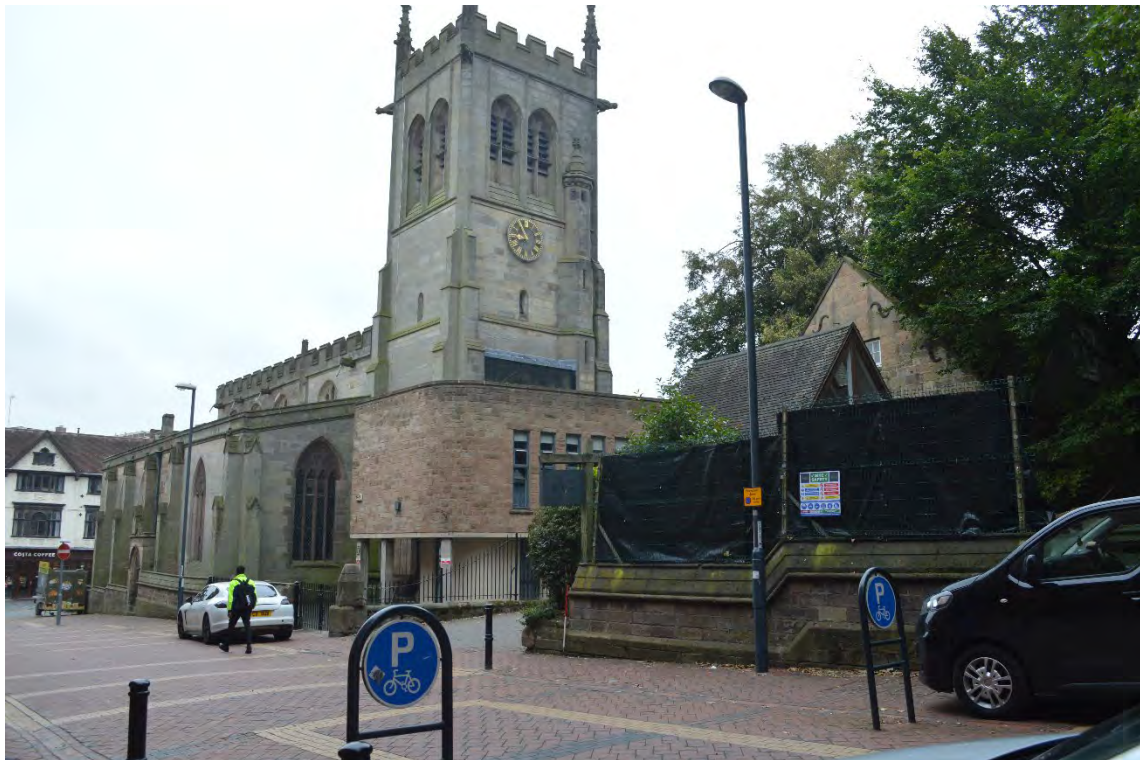
Photograph 15. North elevation of wall, panning upwards to church tower, looking north-west.
