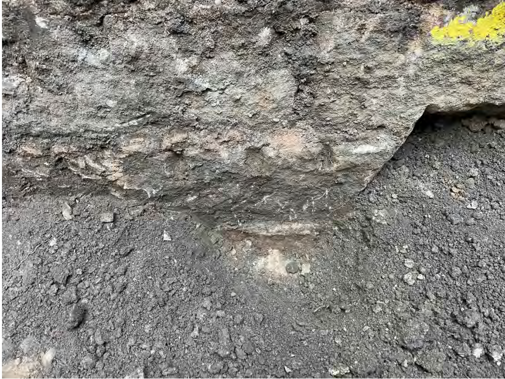
Figure 14. View of wall foundation (no scale)
