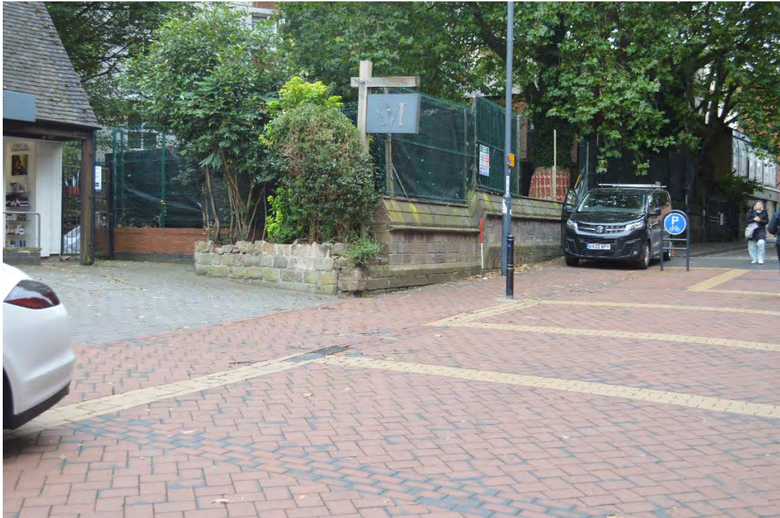
Photograph 13. Eastern end of wall section (north elevation), in context with St Peter's Churchyard Street, looking southwest. Scale in 0.5m graduations.
