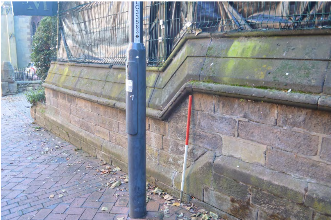
Photograph 8. North elevation of wall, with St Peter's church in background, looking south-east. Scale in 0.5m graduations.
