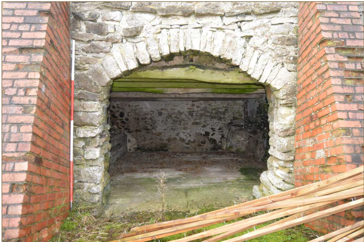
Photograph 20. Detail view of the wide livestock entrance aperture in the east elevation of the barn (looking west). Scale 2m. (File: HBR_106)
