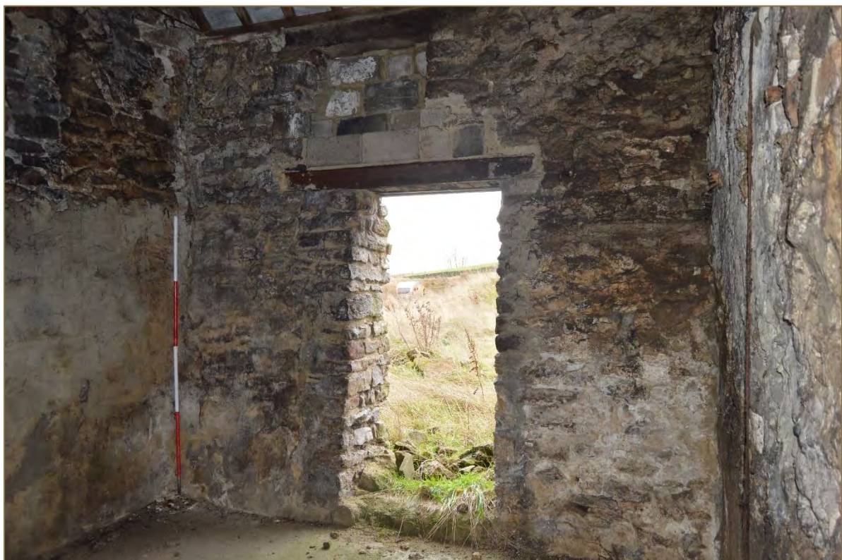
Photograph 43: View of G3/F3, with detail of apertures on the south wall (looking south east). Scale 2m. (File: HBR_167)
