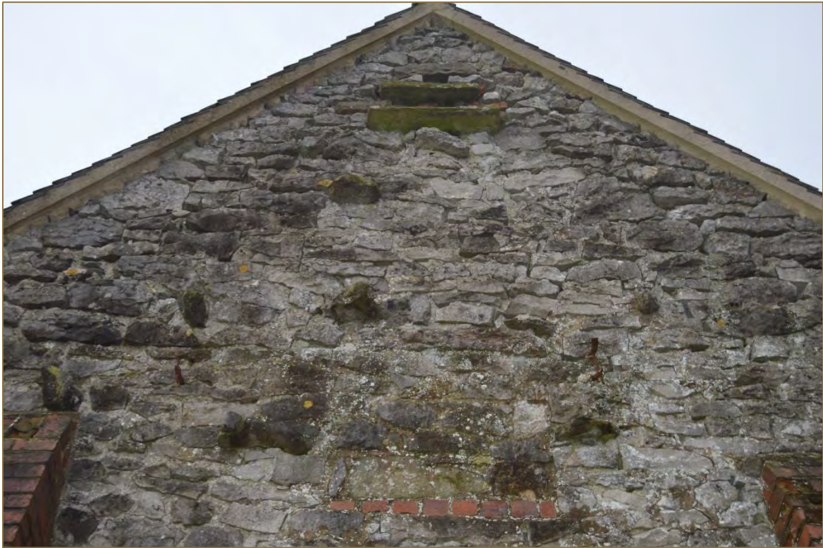
Photograph 22. Detail of the gable with the bird perches and opening on the east elevation of the barn (looking west). (File: HBR_74)
