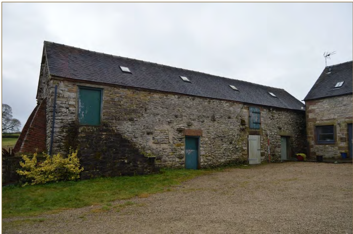
Photograph 9. Overall view of the barn (looking south west). Scale 2m. (File: HBR_16)
