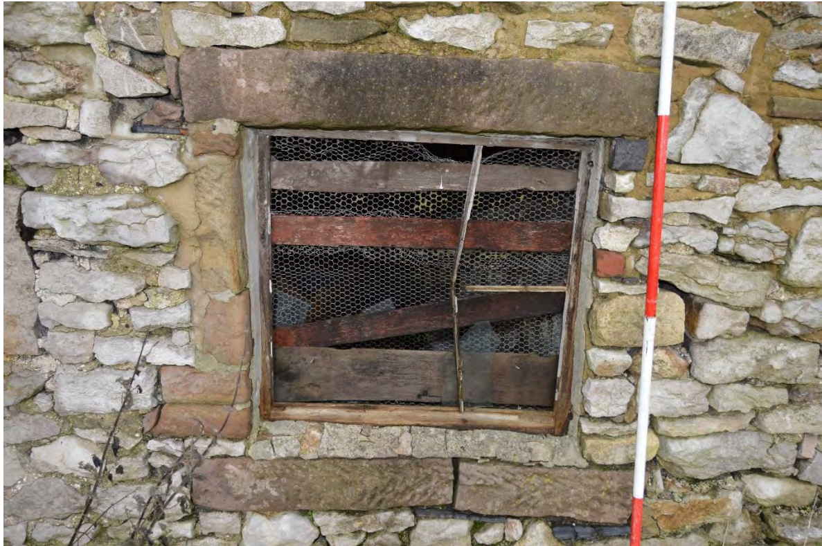
Photograph 29. View of the single window aperture in the barn's south elevation (looking north). Scale 2m. (File: HBR_165)
