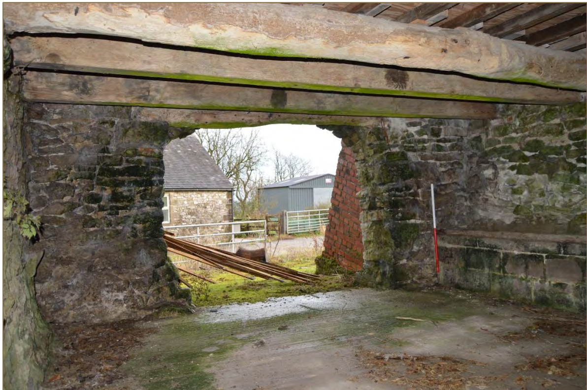
Photograph 36: View of the ground floor interior of the barn (G1), towards the wide opening in the east wall (looking east). Scale 1m. (File: HBR_80)
