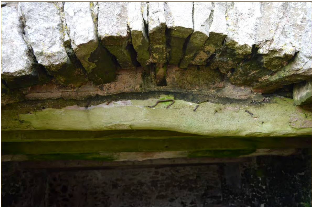
Photograph 23. Detail of the east elevation archway and internal timberwork arrangement (looking west). Scale 2m. (File: HBR_97)
