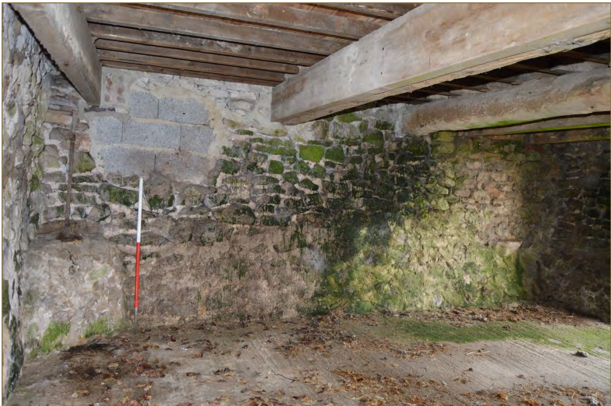
Photograph 39: View of the north wall of the ground floor room (G1) of the barn (looking north). Scale 1m. (File: HBR_89)
