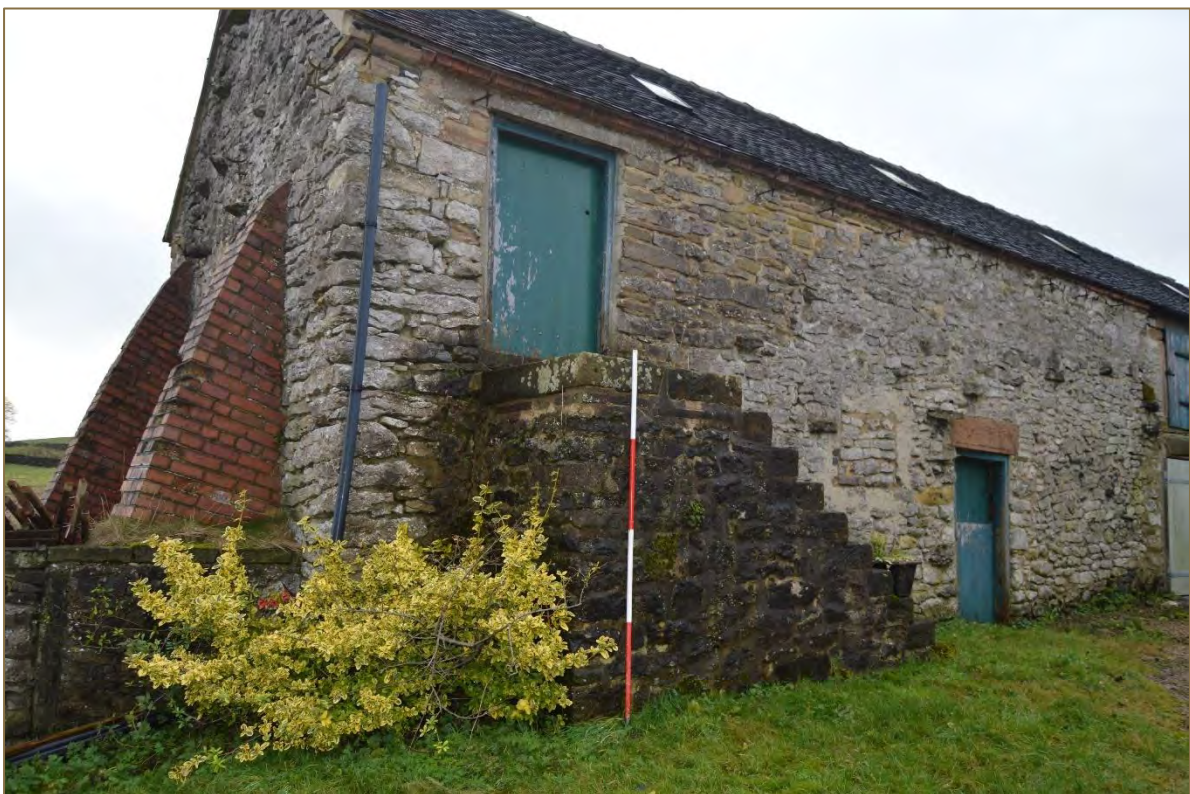
Photograph 16. View of to the barn's eastern bay in the north elevation (looking south west). Scale 2m. (File: HBR_58)
