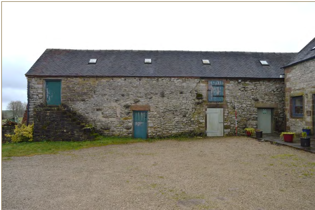
Photograph 10. Perpendicular view of the barn's north elevation (looking south) which forms the south side of the farmyard. Scale 2m. (File: HBR_17)
