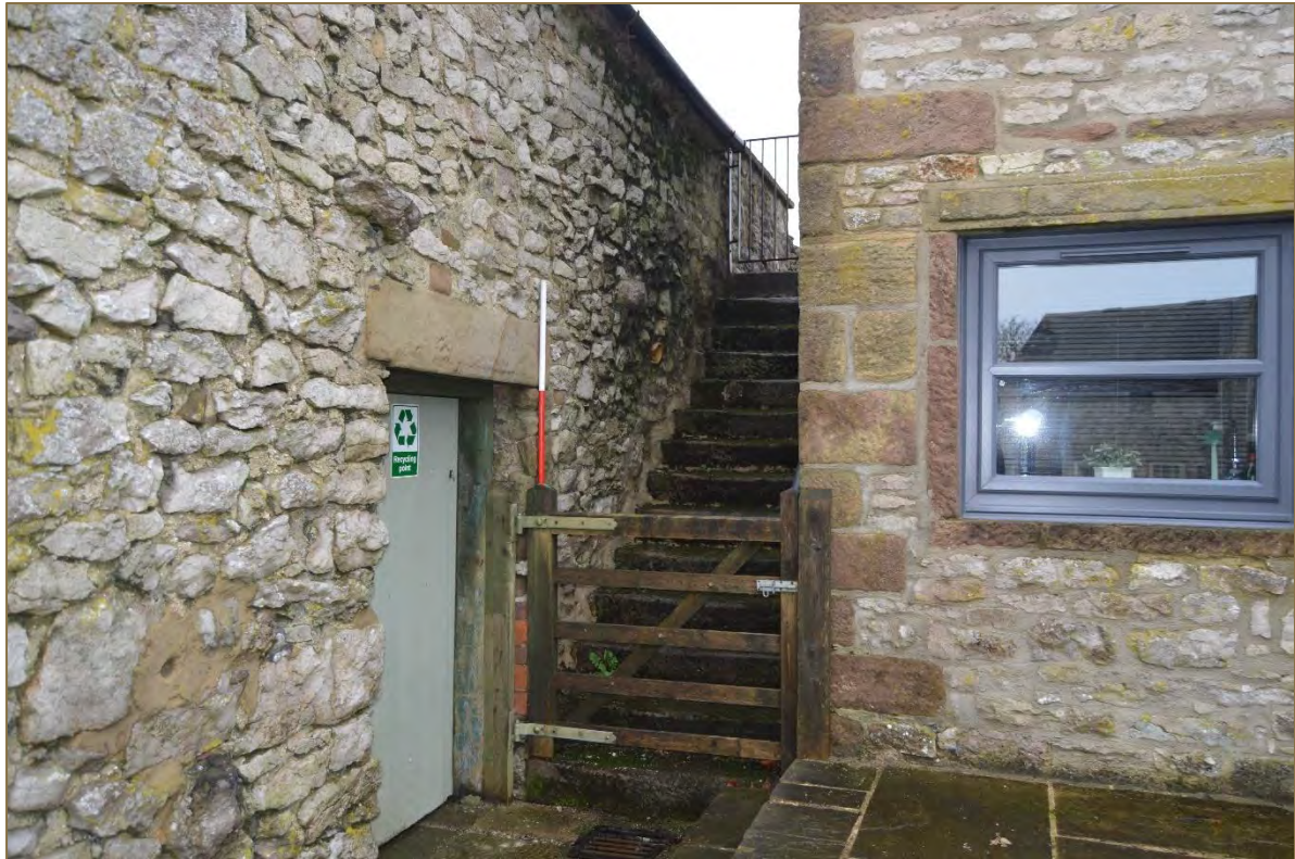
Photograph 11. View of the westernmost ground floor doorway in the north elevation (looking south west). Note the adjacent building and steps conforming to the rising topography. Scale 2m. (File: HBR_21)
