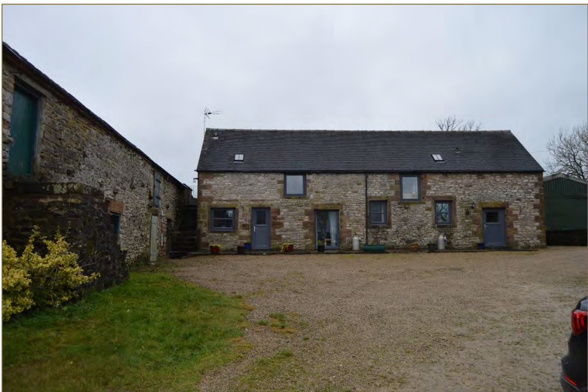
Photograph 4. View of the converted farm building adjacent the barn (left), from the east side of the farmyard (looking west). (File: HBR_6)
