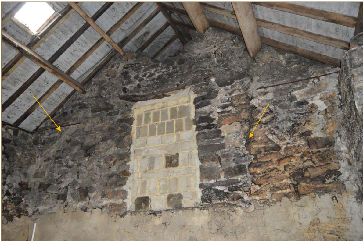
Photograph 47: View of G3/F3, with detail of the east dividing wall, featuring blocked first floor doorway above the plastering at ground level. Other structural features are indicated (looking north east). (File: HBR_164)
