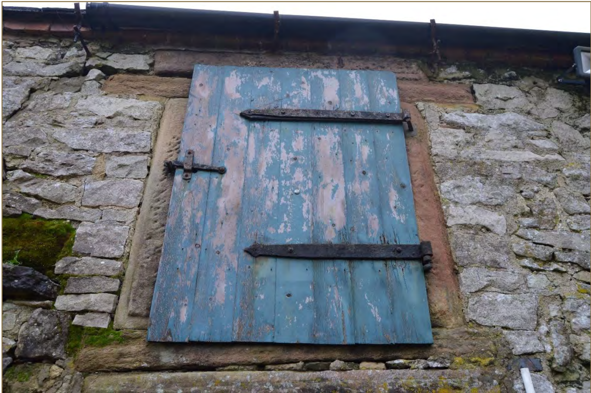
Photograph 15. Detail view of the pitching door in the the barn's north elevation (looking south). Scale 2m. (File: HBR_42)
