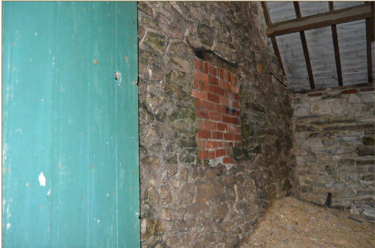
Photograph 52: Internal view of the east gable wall within the first floor of the barn. Note the bricked-up aperture formerly in the east elevation (looking south east). (File: HBR_255)
