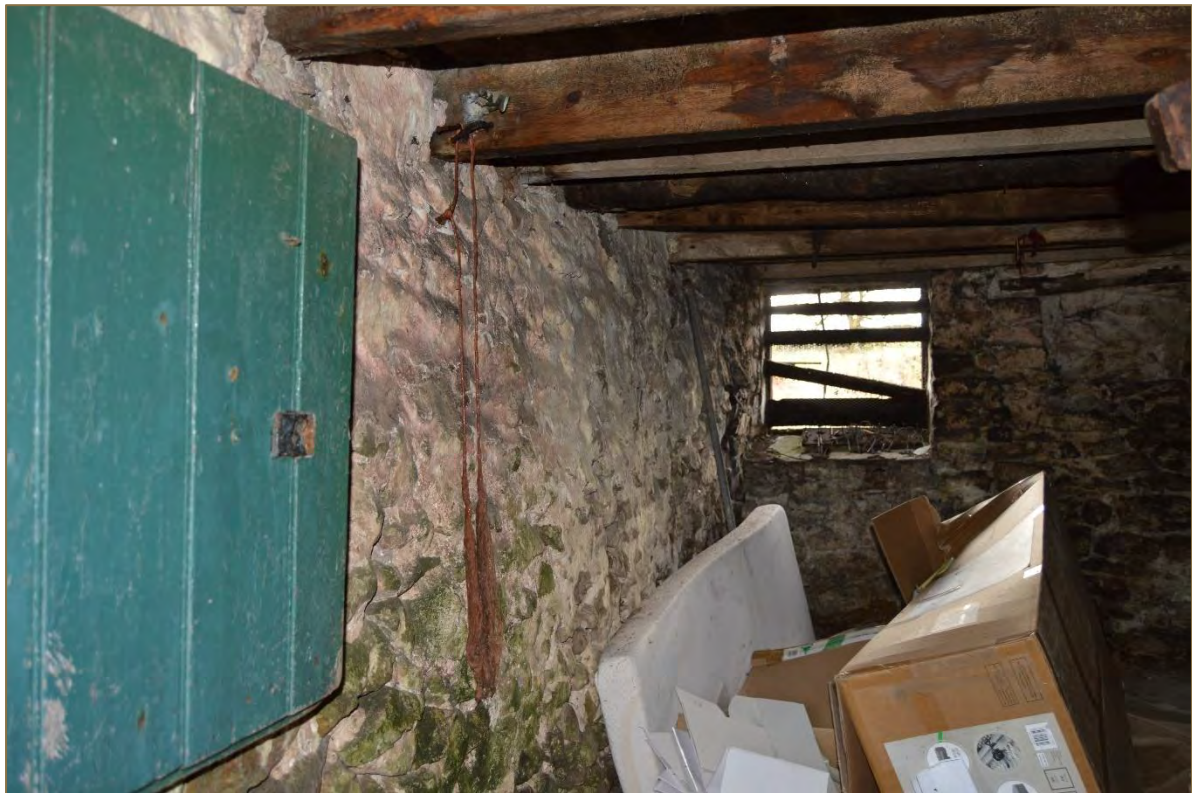
Photograph 42: View of the ground floor room G2, with the single window aperture in the south wall (looking south). Scale 2m. (File: HBR_136)
