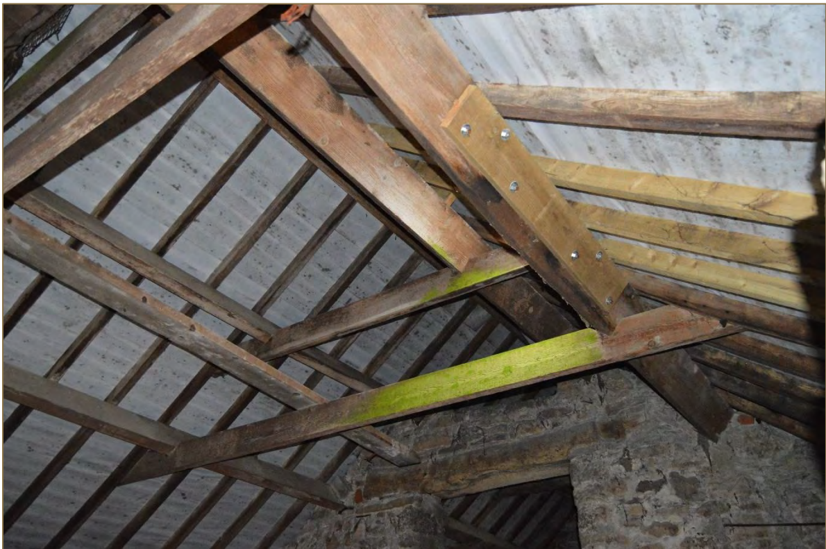
Photograph 55: View of the roof structure over the first floor hayloft (F1) of the barn (looking south west). (File: HBR_258)
