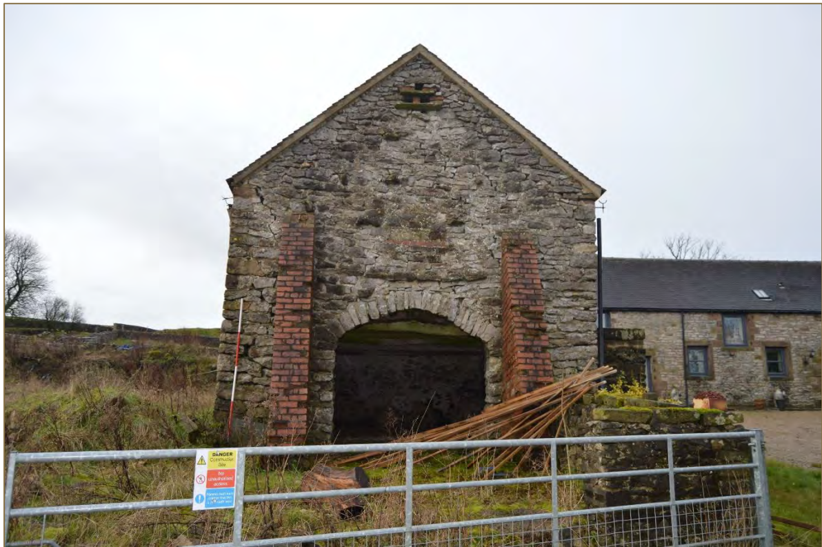
Photograph 18. Perpendicular view of the barn's east elevation (looking west). Scale 2m. (File: HBR_69)
