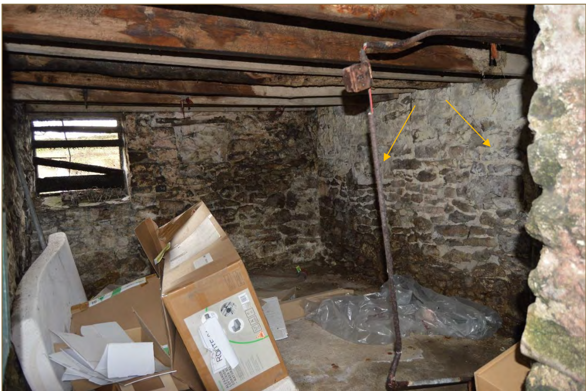
Photograph 41: View of the ground floor room G2, with blocked aperture features observed in the west wall (looking south). (File: HBR_134)
