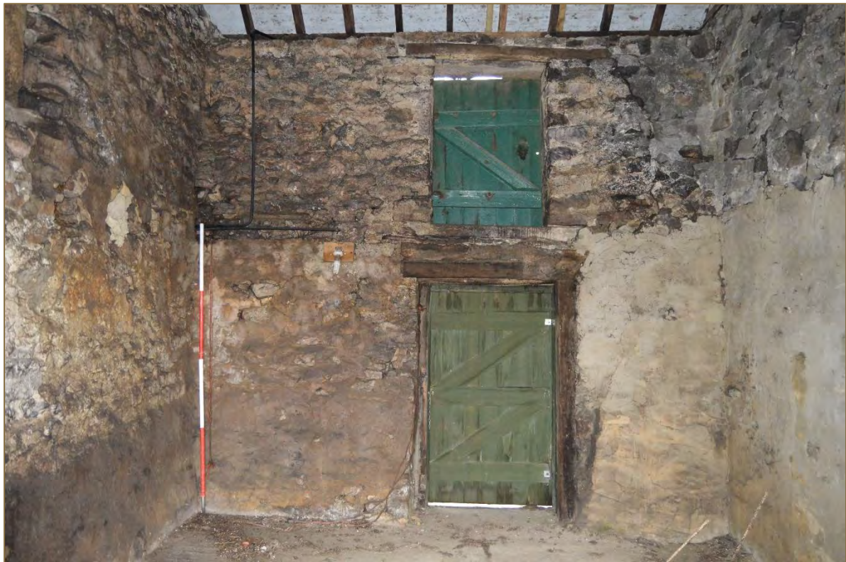
Photograph 58: View of the north wall of the barn's ground and non-extant first floor level (G3/F3) (looking north). Scale 2m. (File: HBR_157)
