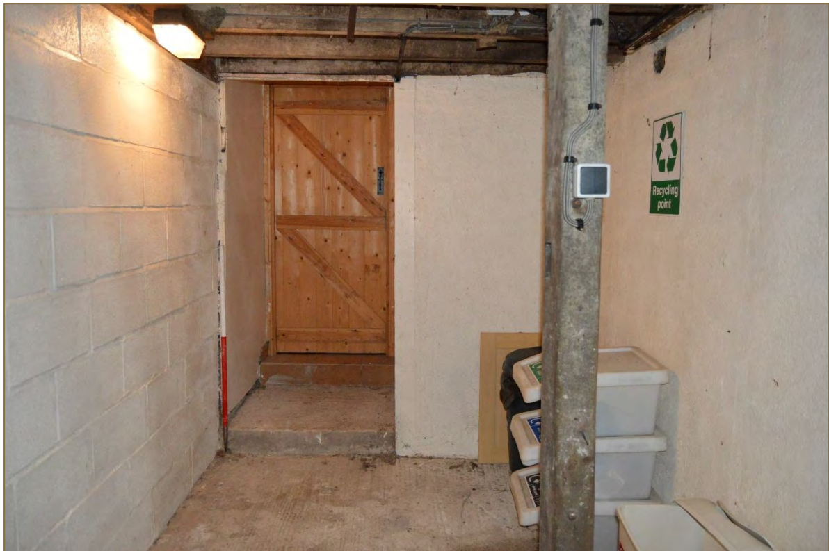
Photograph 50: View of the barn's ground floor westernmost, room (G4) which has been renovated for modern communal use (looking west). Scale 2m. (File: HBR_143)
