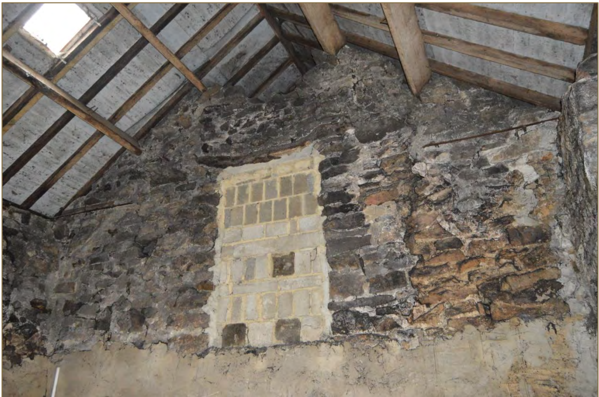
Photograph 57: View of the east dividing wall of the barn's non-extant first floor level, F3, inside G3 (looking east). Scale 2m. (File: HBR_164)
