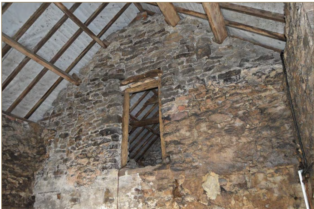
Photograph 59: View of the west wall of the barn's non-extant first floor level (G3/F3) (looking west). (File: HBR_155)
