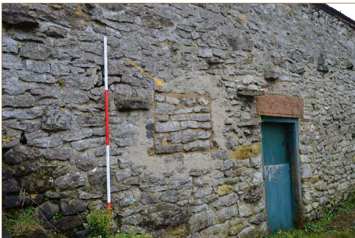
Photograph 14. View of the eastern extent of the barn's north elevation, (looking south west). Scale 2m. (File: HBR_18)
