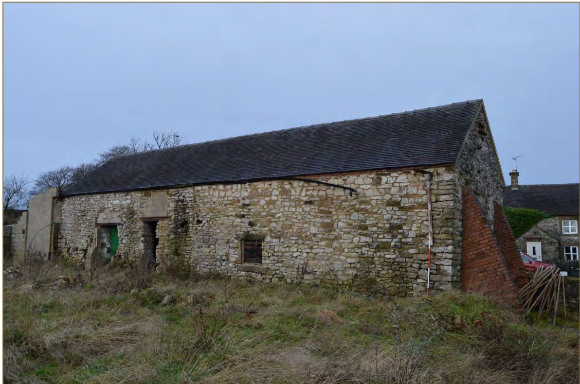
Photograph 24. Overall oblique view of the barn's south elevation (looking north west). Scale 2m. (File: HBR_119)
