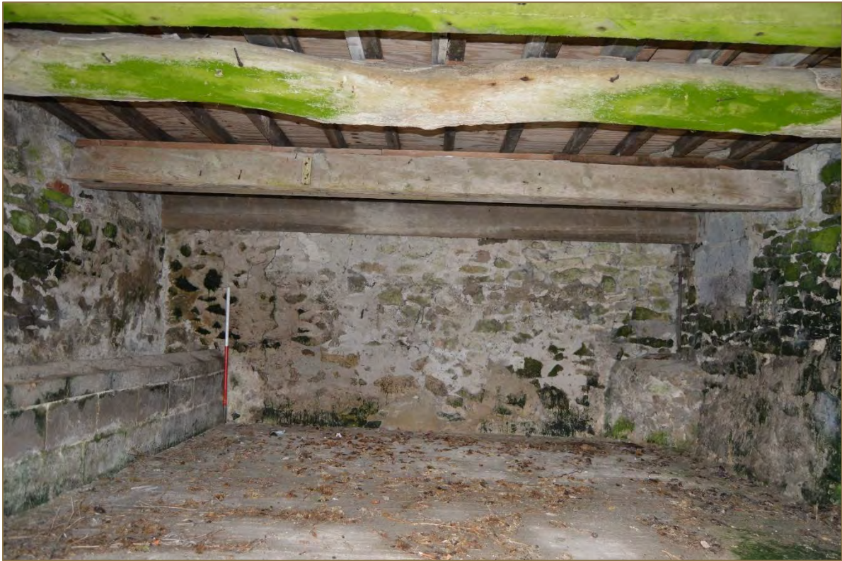
Photograph 38: View of the west wall of the ground floor room (G1) of the barn (looking west). Scale 1m. (File: HBR_83)
