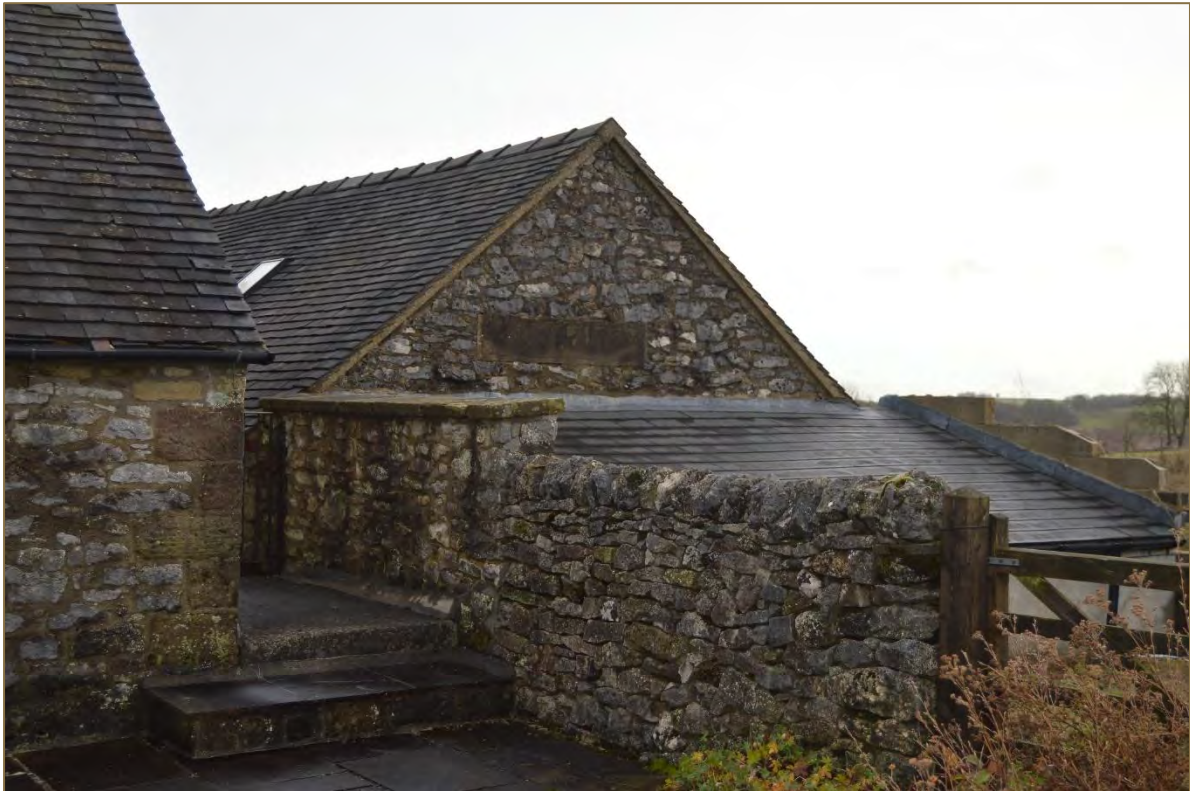
Photograph 34. Oblique view of the barn's west elevation (looking south east). (File: HBR_127)
