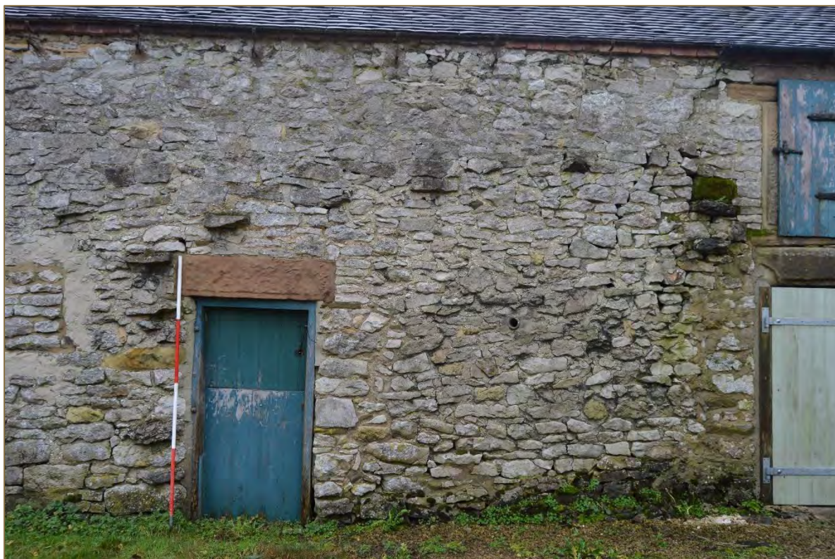
Photograph 13. View of the centre bay and doorways in the barn's north elevation (looking south). Scale 2m. (File: HBR_24)
