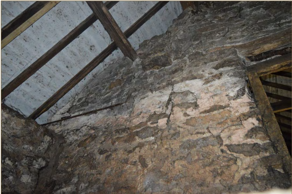
Photograph 60: Restricted view of the barn's first floor eastern wall from the ground floor room (G4/F4)(looking east). (File: HBR_149)
