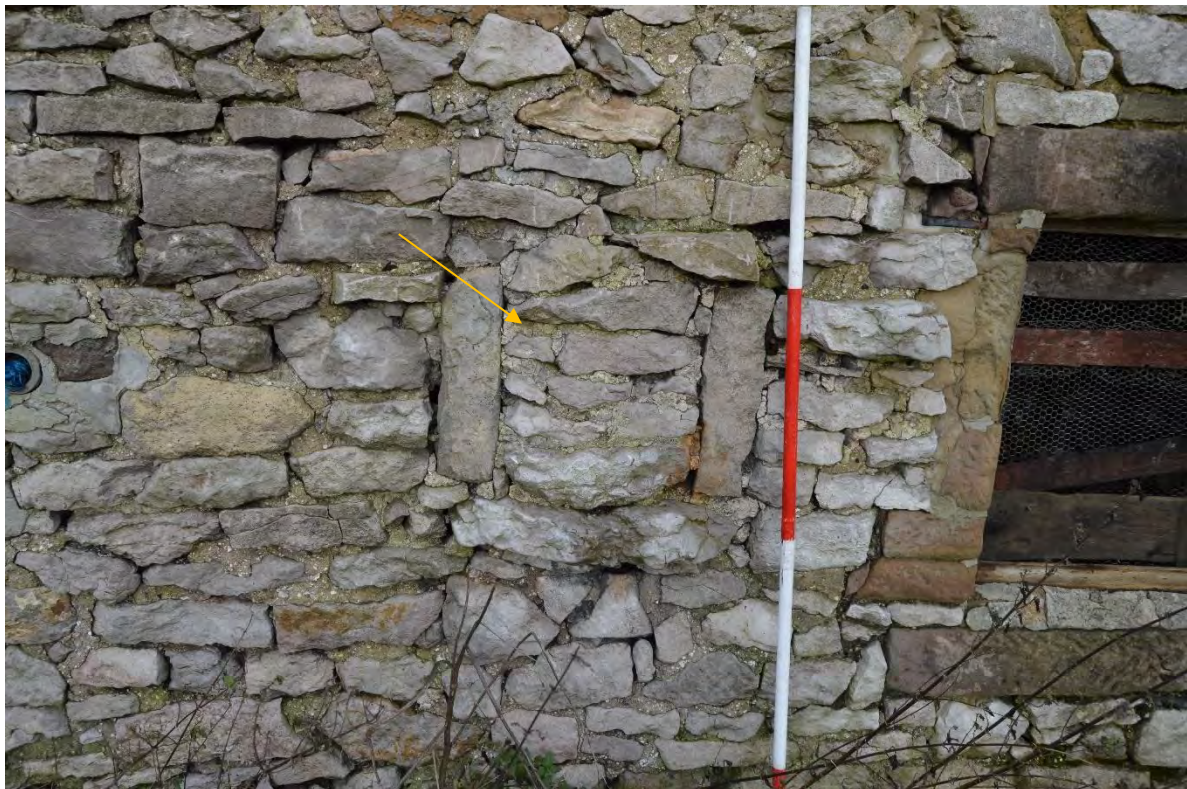
Photograph 30. View of the blocked aperture (indicated) in the barn's south elevation (looking north). Scale 2m. (File: HBR_149)
