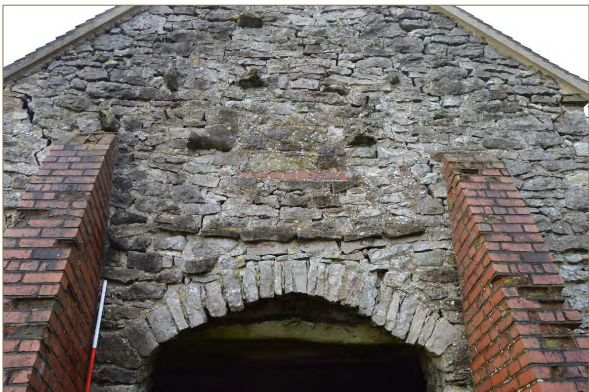
Photograph 21. Detail view of the upper extent with arrangement of protruding tie stones on the east elevation of the barn (looking west). (File: HBR_105)
