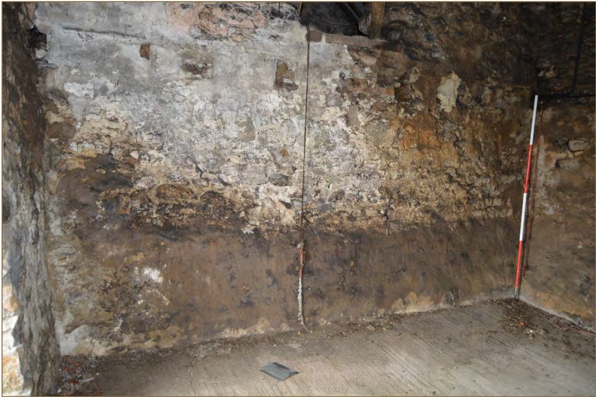
Photograph 46: View of G3/F3, with detail of the west wall, featuring blocked first floor joist slots with doorway above (looking north west). Scale 2m. (File: HBR_153)
