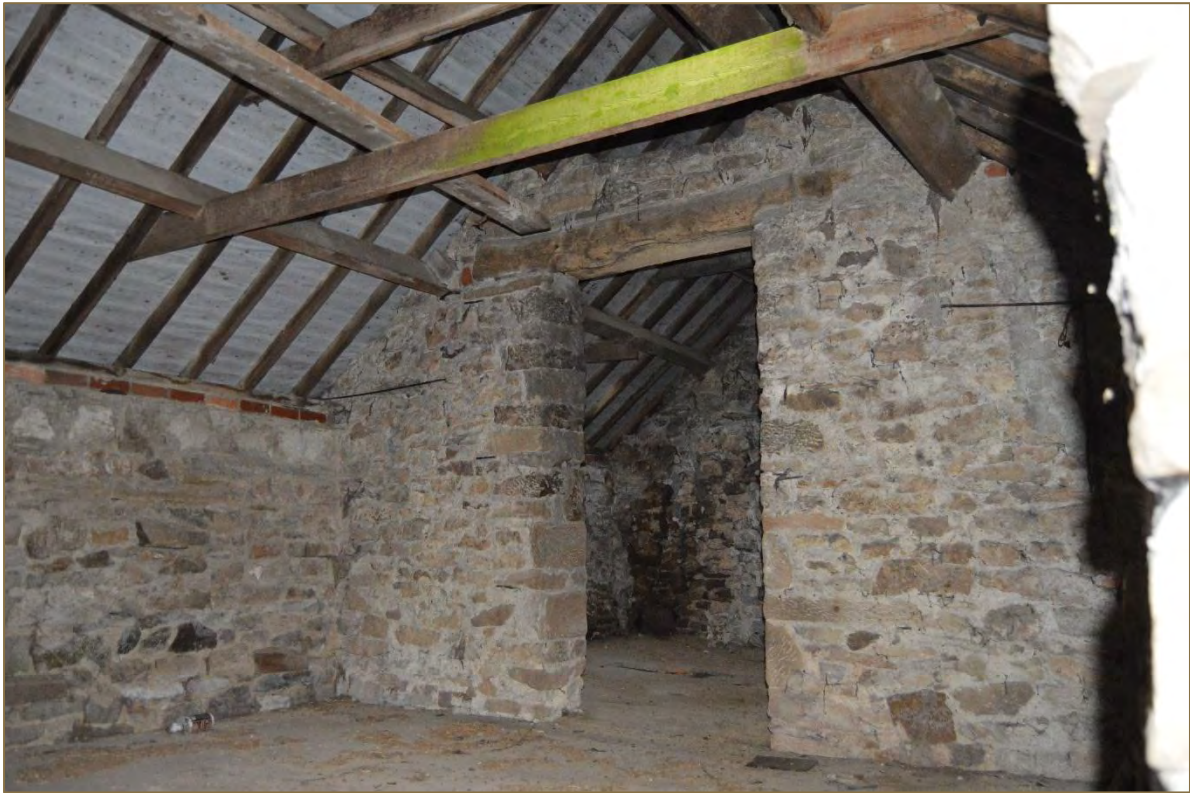
Photograph 54: View of west dividing wall with access to the adjoining room (F2) on the first floor of the barn. (File: HBR_252)
