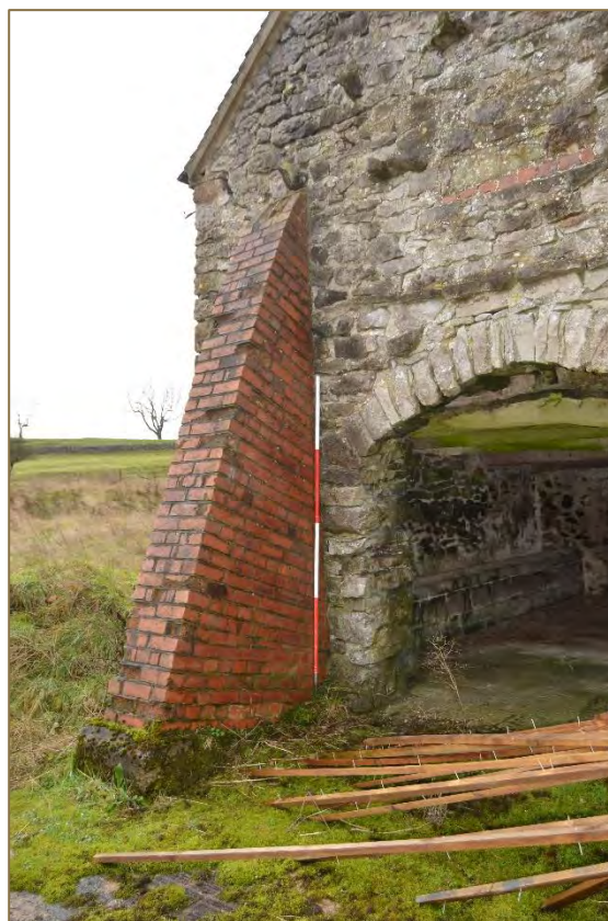
Photograph 19. View of the left hand brick pier on the east elevation of the barn (looking south west). Scale 2m. (File: HBR_114)
