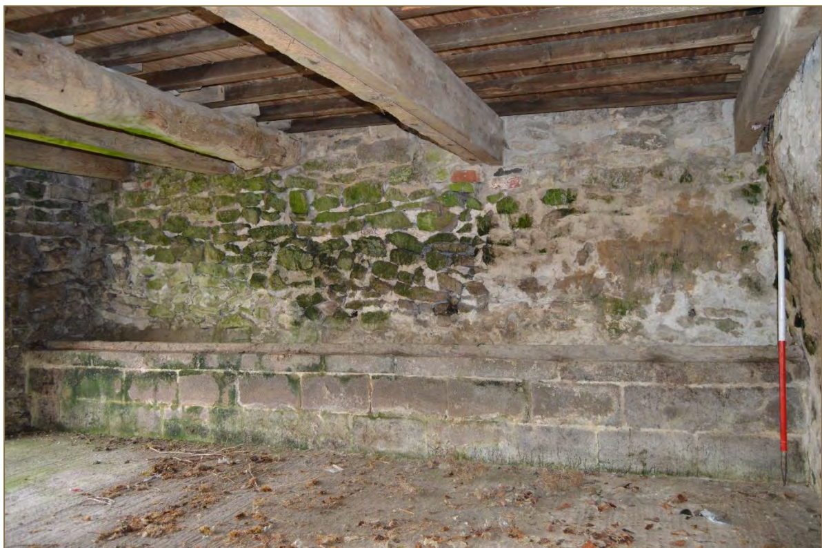
Photograph 37: View of the south wall of the ground floor room (G1) of the barn with modern cow trough (looking south). Scale 1m. (File: HBR_83)
