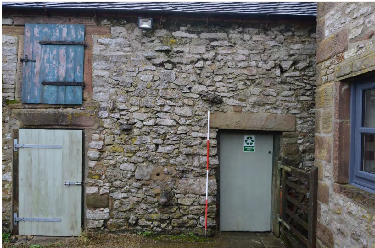
Photograph 12. Perpendicular view of the western bays of the barn's south elevation (looking south). Scale 2m. (File: HBR_27)
