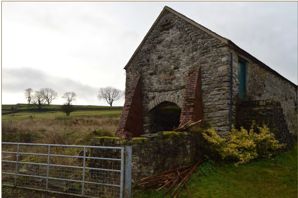
Photograph 17. Oblique view of the barn's east elevation (looking south west). Scale 2m. (File: HBR_70)
