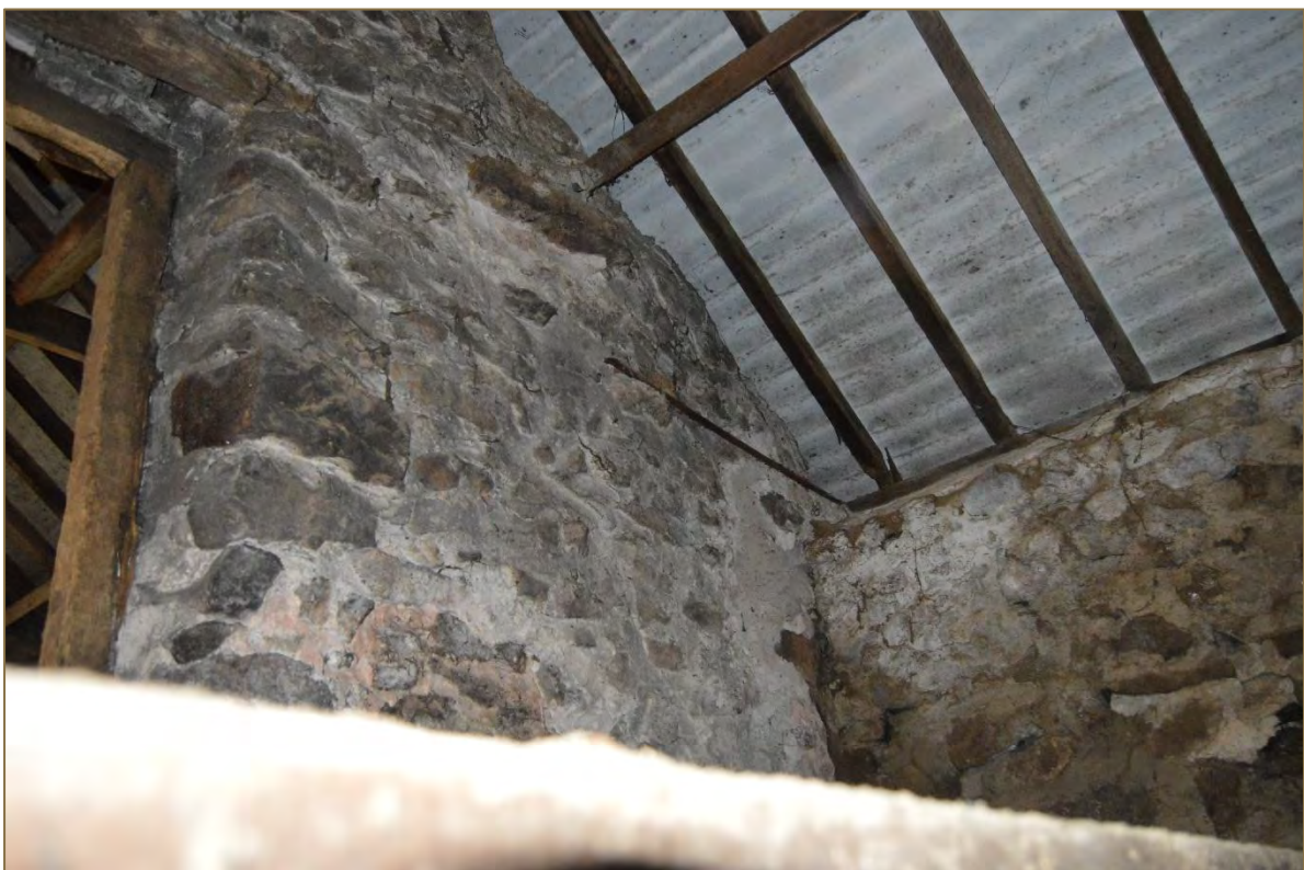
Photograph 61: Restricted view of the barn's first floor eastern and southern wall from the ground floor room (G4/F4)(looking south east). (File: HBR_151)
