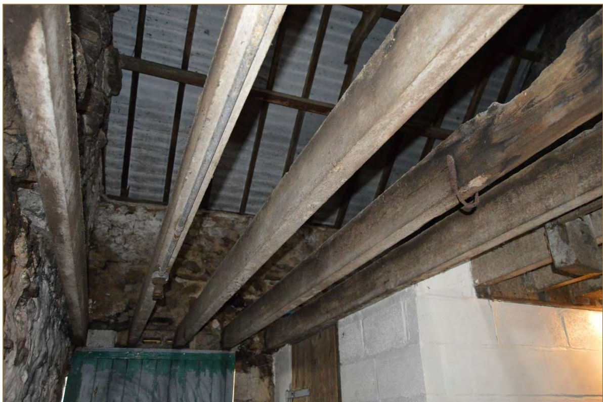
Photograph 51: View of the barn's ground floor westernmost room (G4) showing the remaining first floor joists (looking south). Scale 2m. (File: HBR_139)
