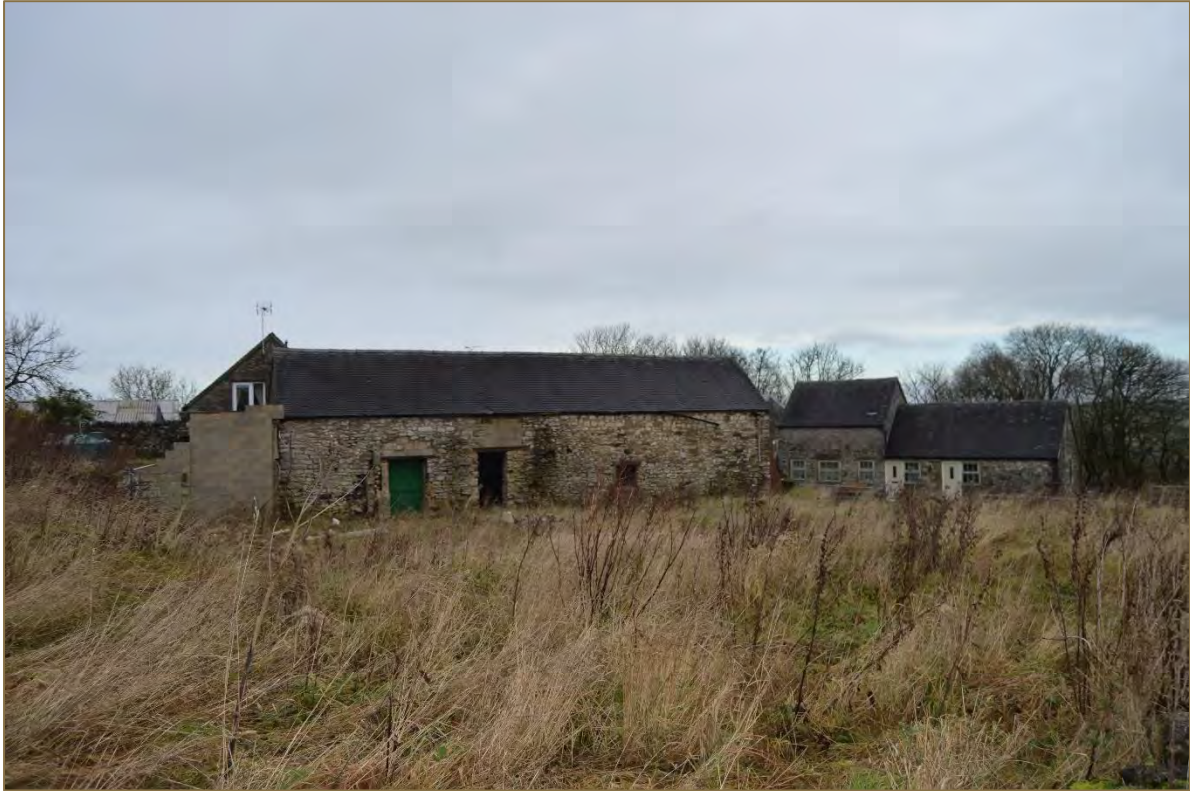
Photograph 7. View of the barn and its settings from south perimeter of the farmyard (looking north). Scale 2m. (File: HBR_11)
