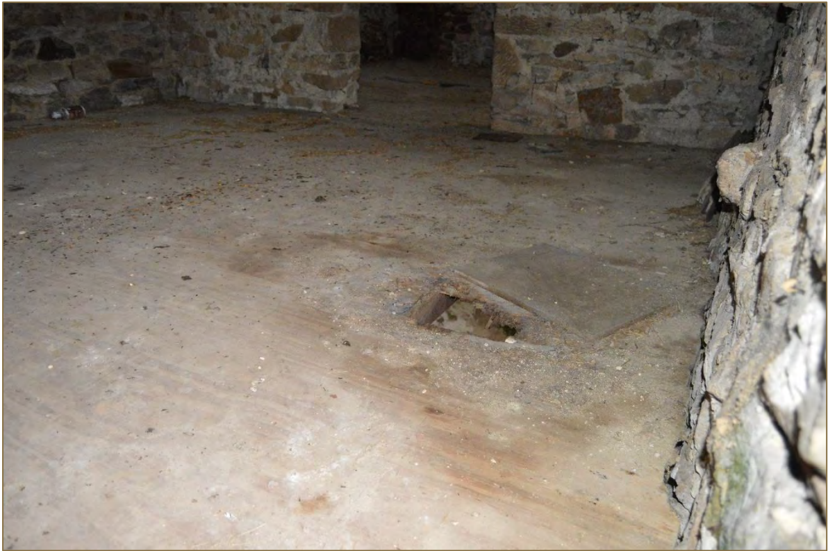
Photograph 56: View of the plywood flooring of the first floor hayloft (F1) of the barn and through into the next room (F2) (looking south west). (File: HBR_254)
