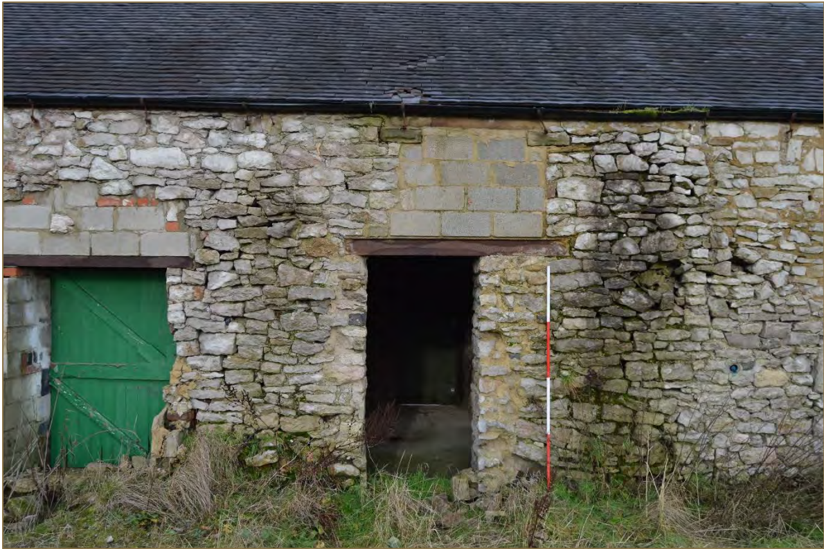
Photograph 27. View of the easternmost doorway in the barn's south elevation (looking north). Scale 2m. (File: HBR_124)
