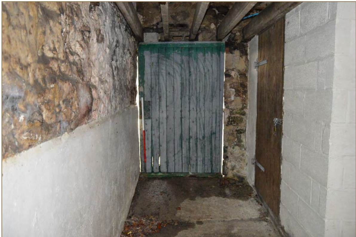
Photograph 48: View of the barn's ground floor, westernmost room (G4) which has been renovated for modern communal use (looking south). Scale 2m. (File: HBR_138)
