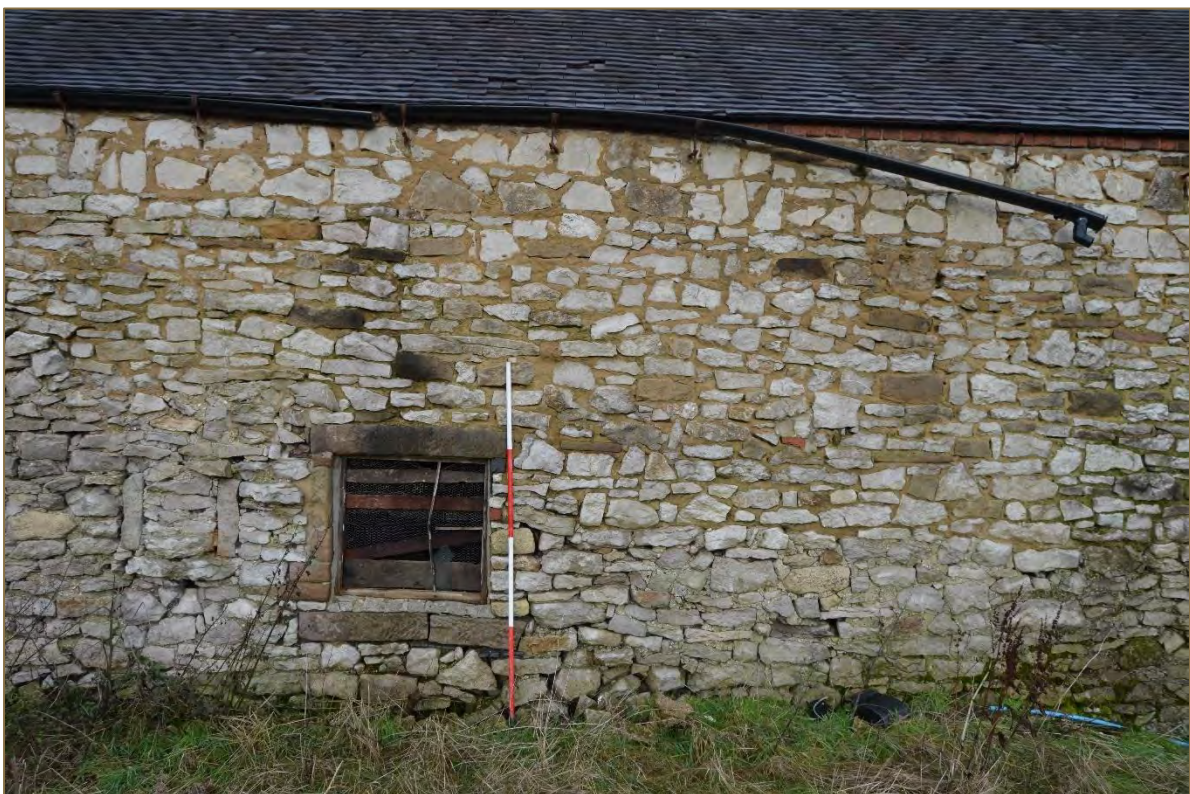
Photograph 28. View of the single window aperture in the barn's south elevation (looking north). Scale 2m. (File: HBR_338)
