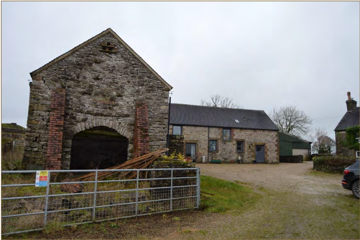
Photograph 5. View of the barn and its settings from the south gate of the farmyard (looking west). (File: HBR_7)
