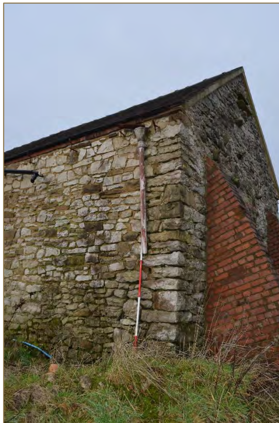
Photograph 32. View of the barn's south east corner with (looking north west). Scale 2m. (File: HBR_107)
