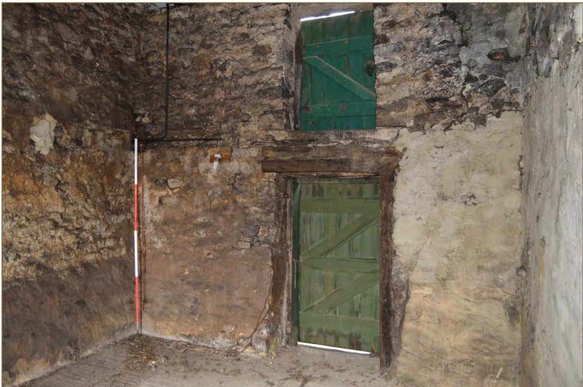
Photograph 45: View of G3/F3, with detail of apertures on the north wall (looking north west). Scale 2m (File: HBR_158)
