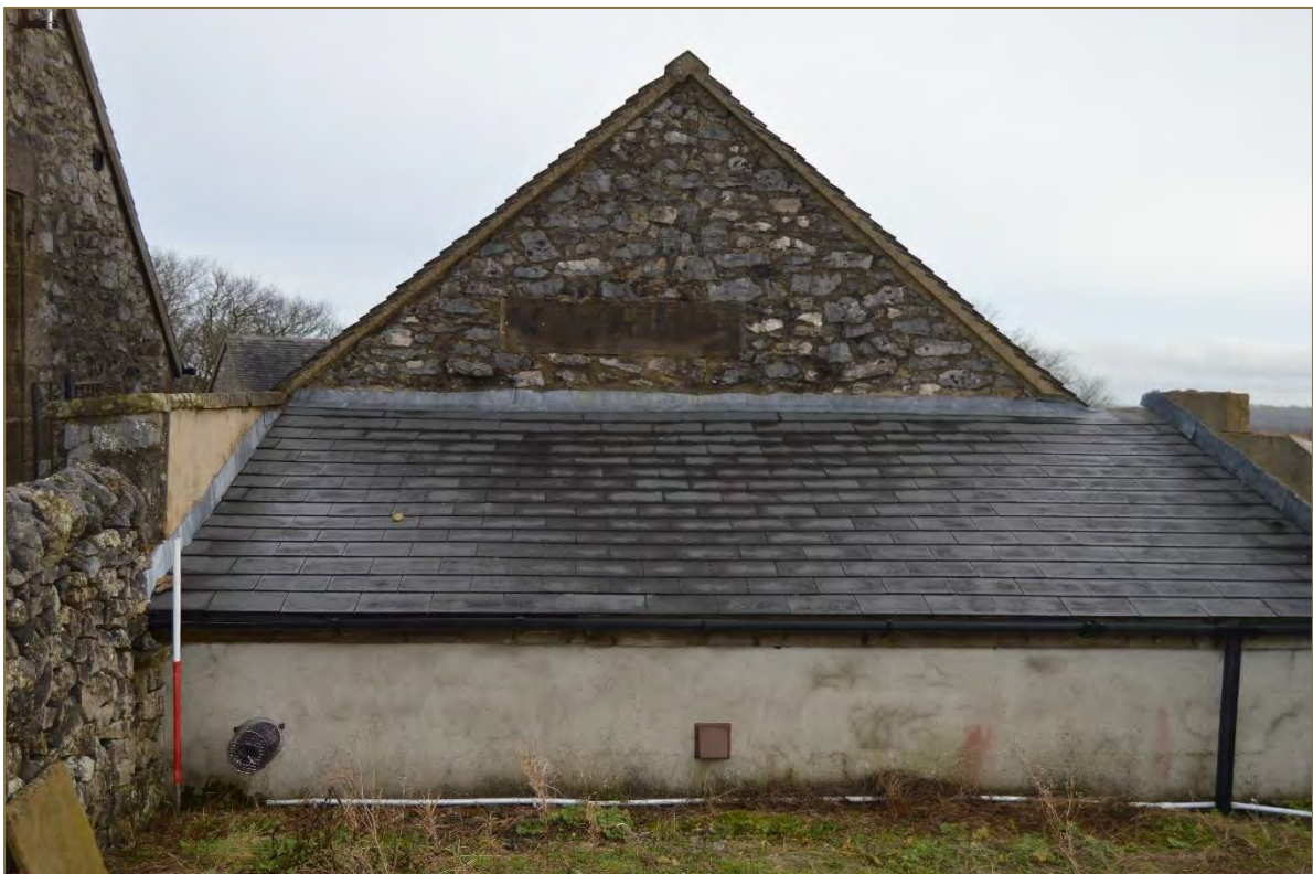
Photograph 35. View of the barn's west elevation (looking east). Scale 1m. (File: HBR_128)
