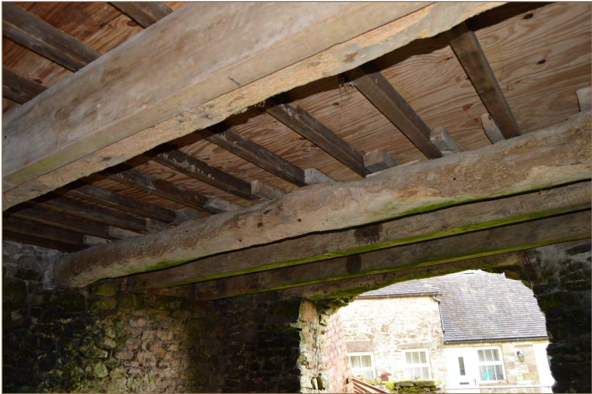
Photograph 40: View of the ceiling structure above the barn's easternmost ground floor room (G1) (looking north east). (File: HBR_173)
