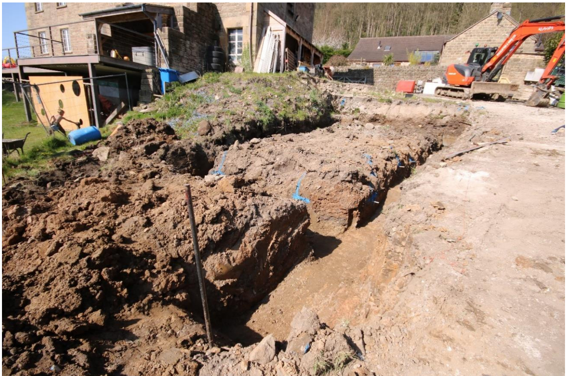
Figure 2: Looking NW towards the building foundation trench
