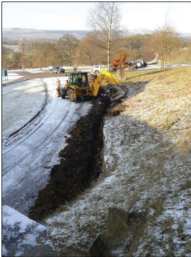
Fig. 3: Trench initial excavation. Facing north-west.
