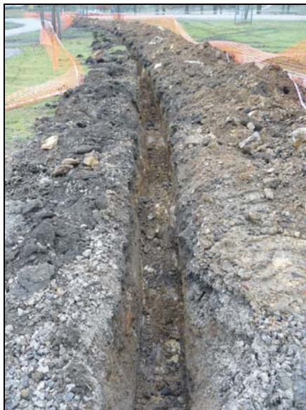
Fig. 4: Trench in managed grassland Facing west.
