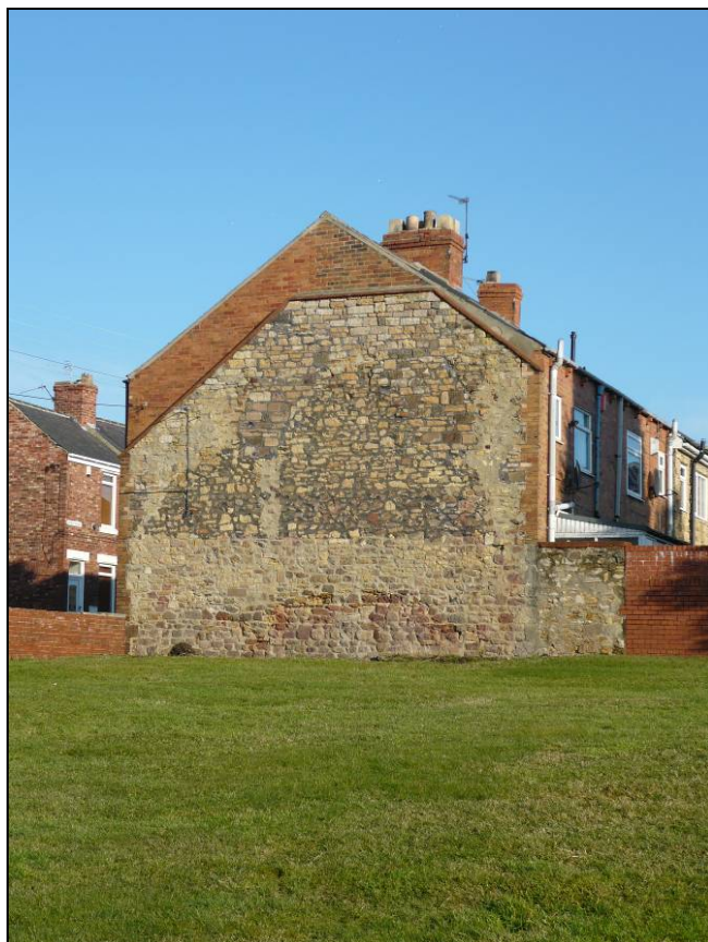
Fig. 16 evidence of the former 19 th century buildings
