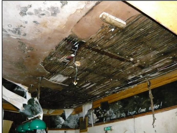
Fig. 21 Internal ground floor ceiling
