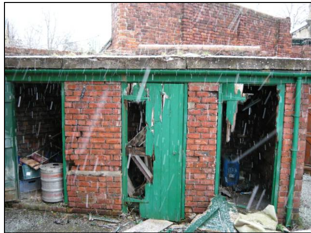
Fig. 19 Brick built sheds to the east of the building
