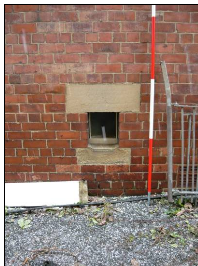
Fig. 20 Small window on the south elevation
